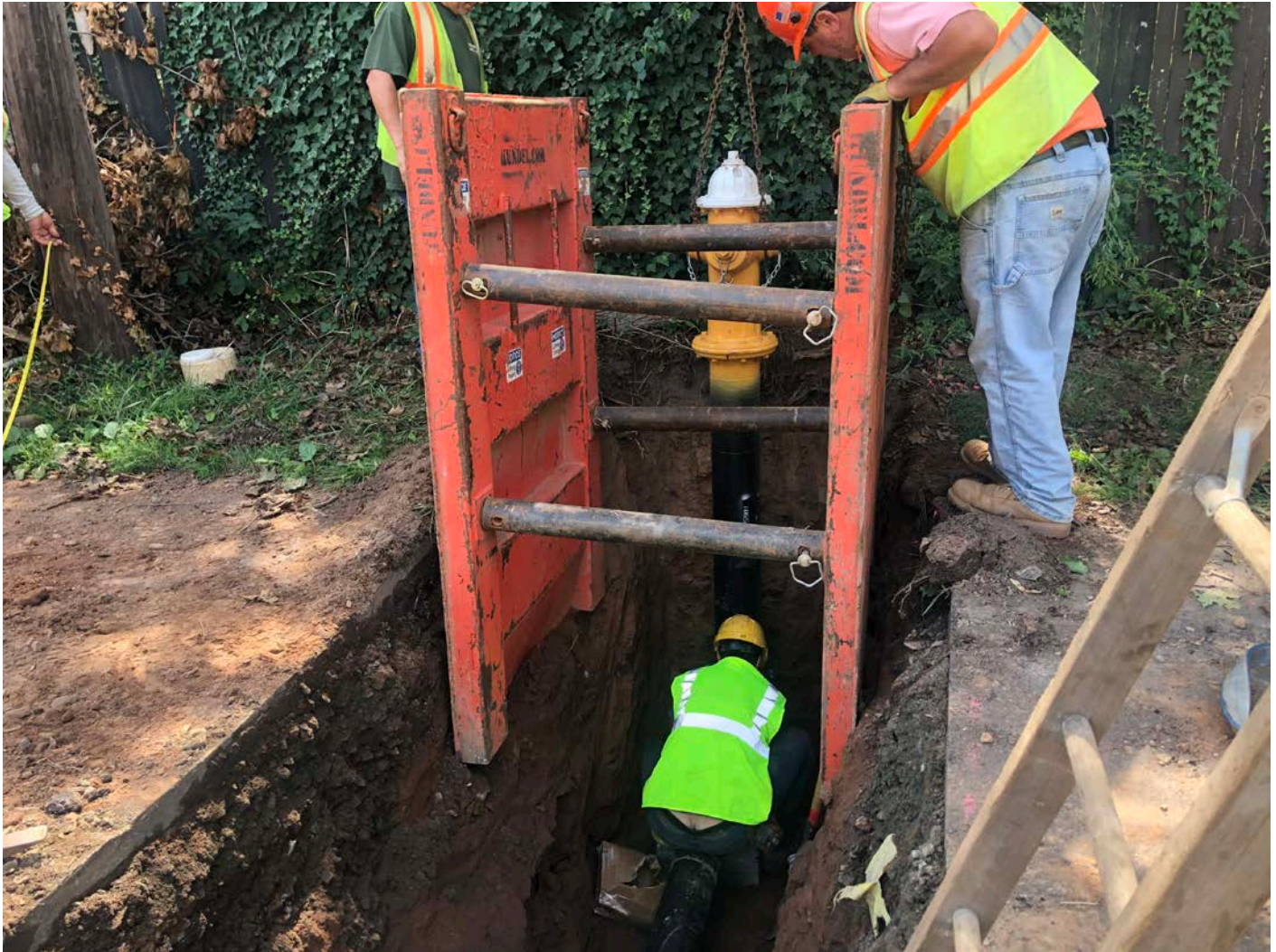
Picture 10: Ludlow installing a new hydrant at Station 401+37, Maiden Lane, Durham. View to the south.
