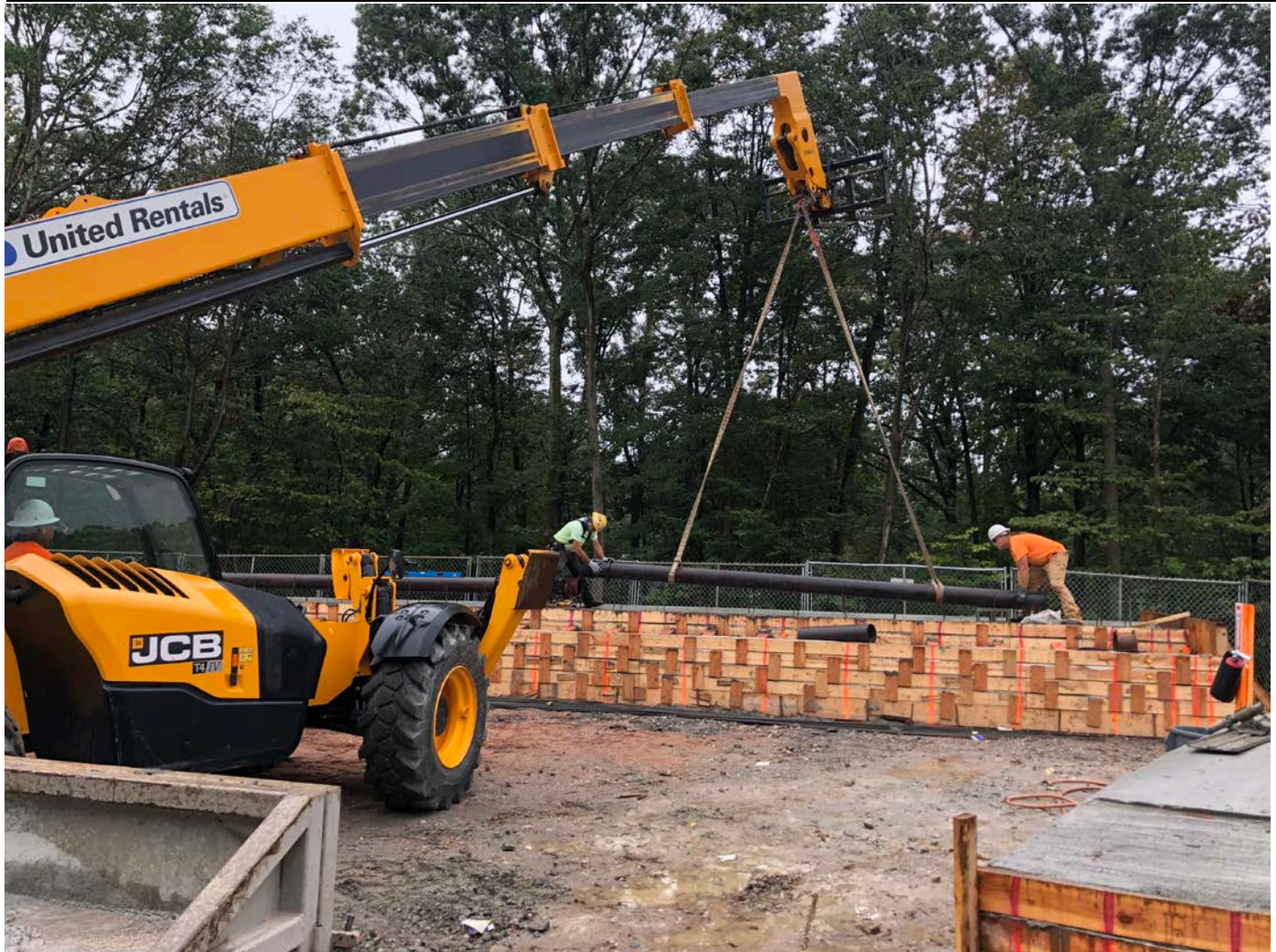
Picture 7: DN Tanks placing 8" DIP on one of the narrow water tank side panels. Water tank work zone, east of the Shared Access Driveway, Middletown. View to the south.
