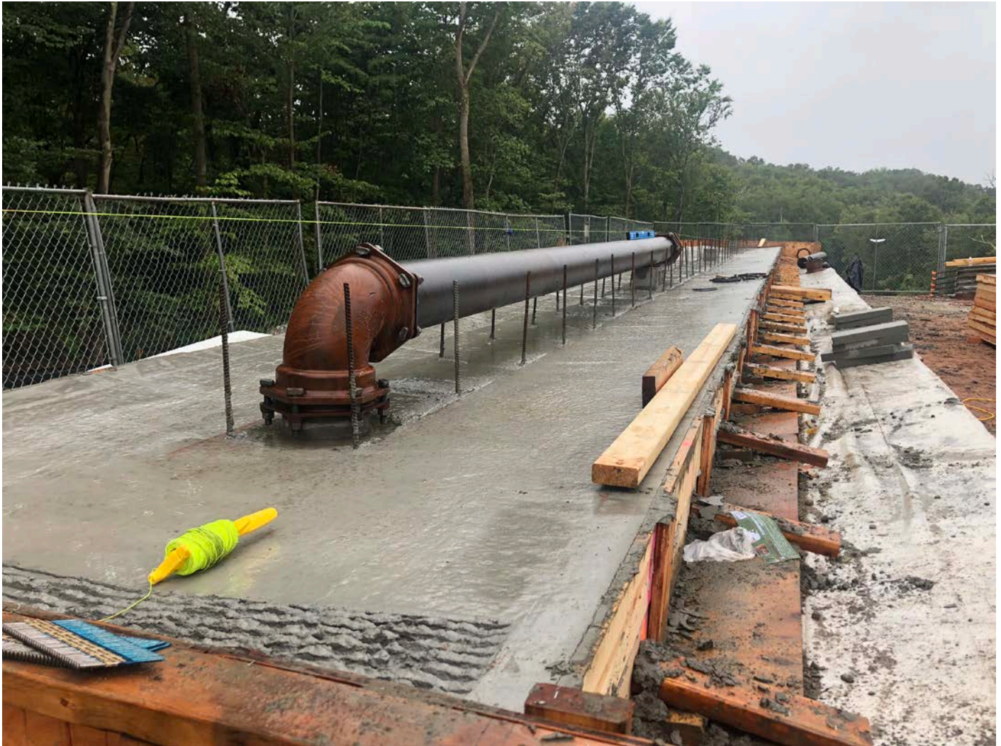
Picture 2: 8" DIP installed on one of the narrow water tank side panels. Water tank work zone, east of the Shared Access Road, Middletown. View to the west.
