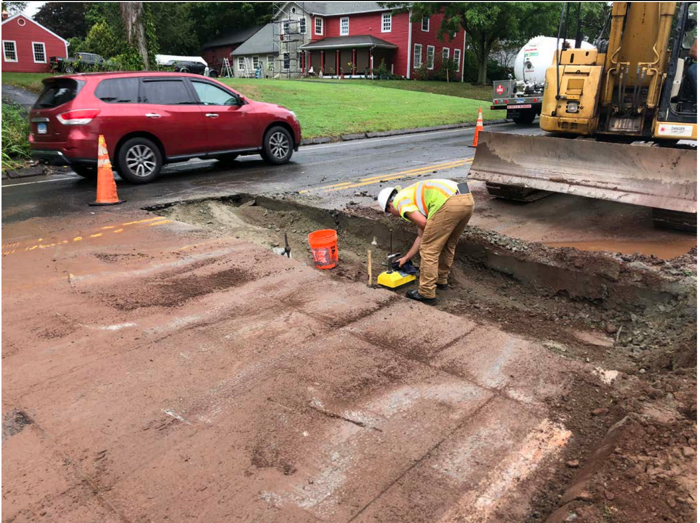
Picture 6: JTC collecting soil compaction data at Station 198+10, Main Street, Durham. View to the northwest.
