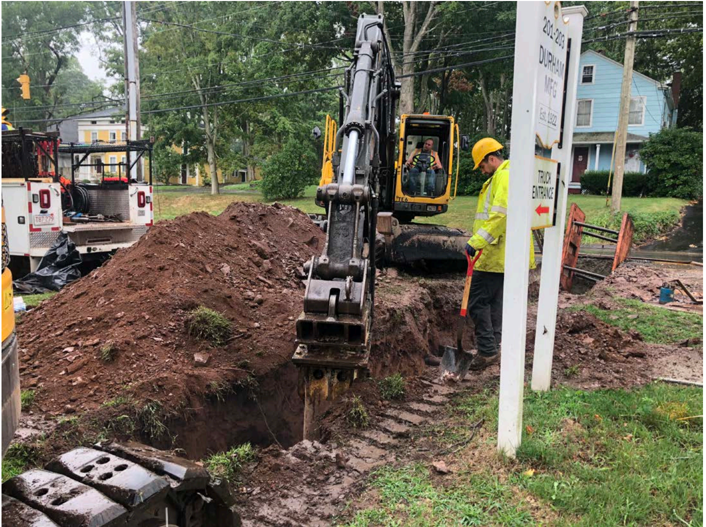
Picture 4: Ludlow hammering rock as they excavate a trench for the installation of 4" DIP at Station 198+10. 201-203 Main Street, Durham. View to the west.
