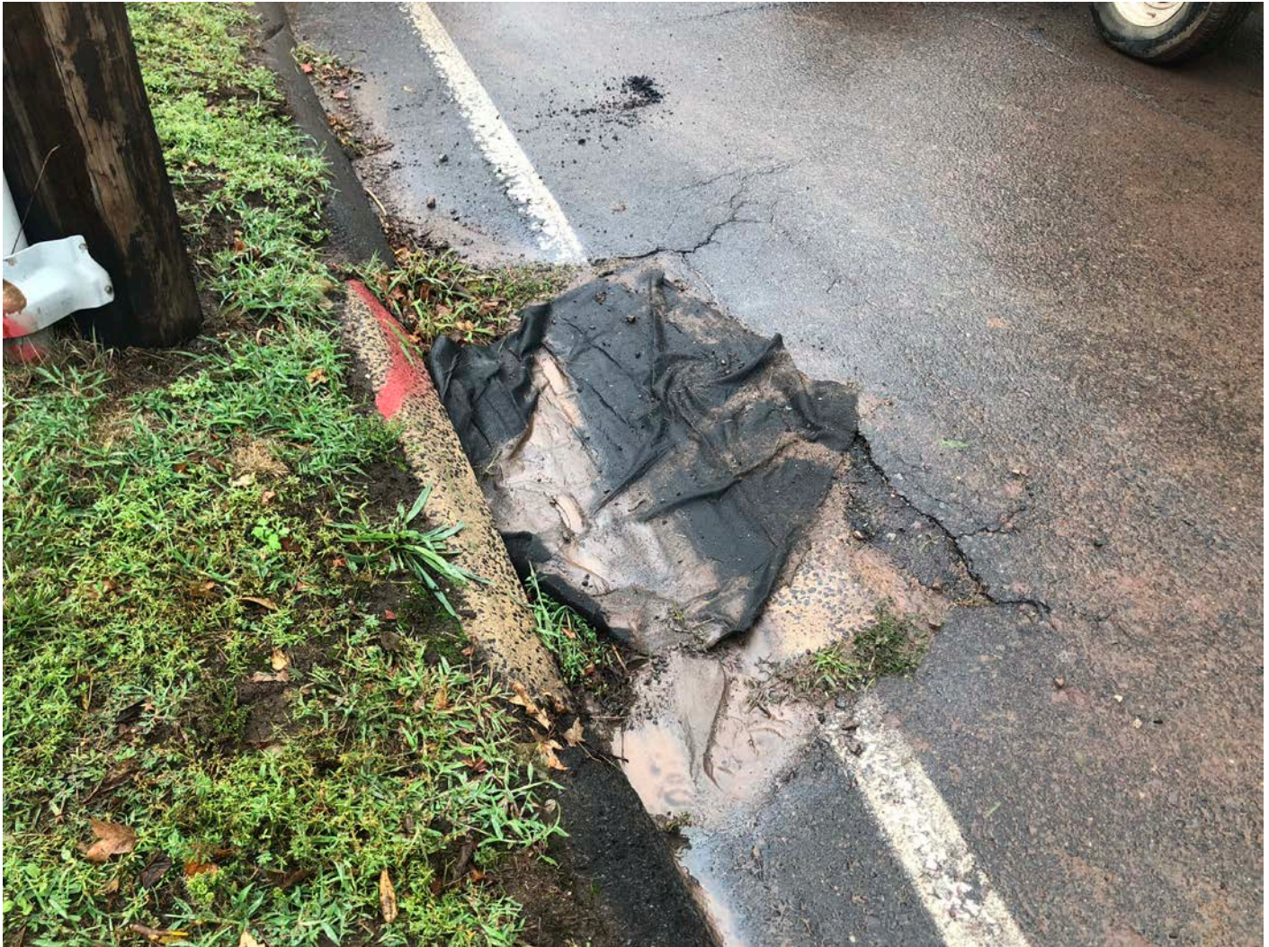
Picture 8: Filter fabric placed over storm drain on Main Street downgradient of the excavation at Station 198+10. Main Street, Durham.
