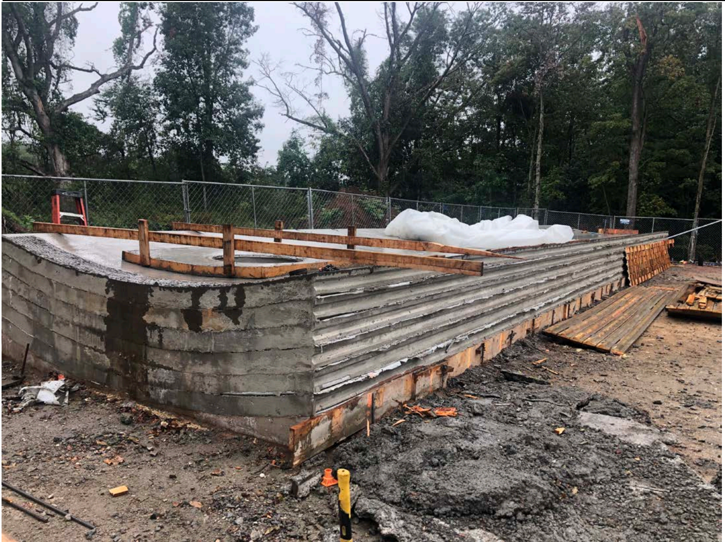
Picture 3: Wide water tank side panels with the wooden forms partially removed. Water tank work zone, east of the Shared Access Road, Middletown. View to the south.
