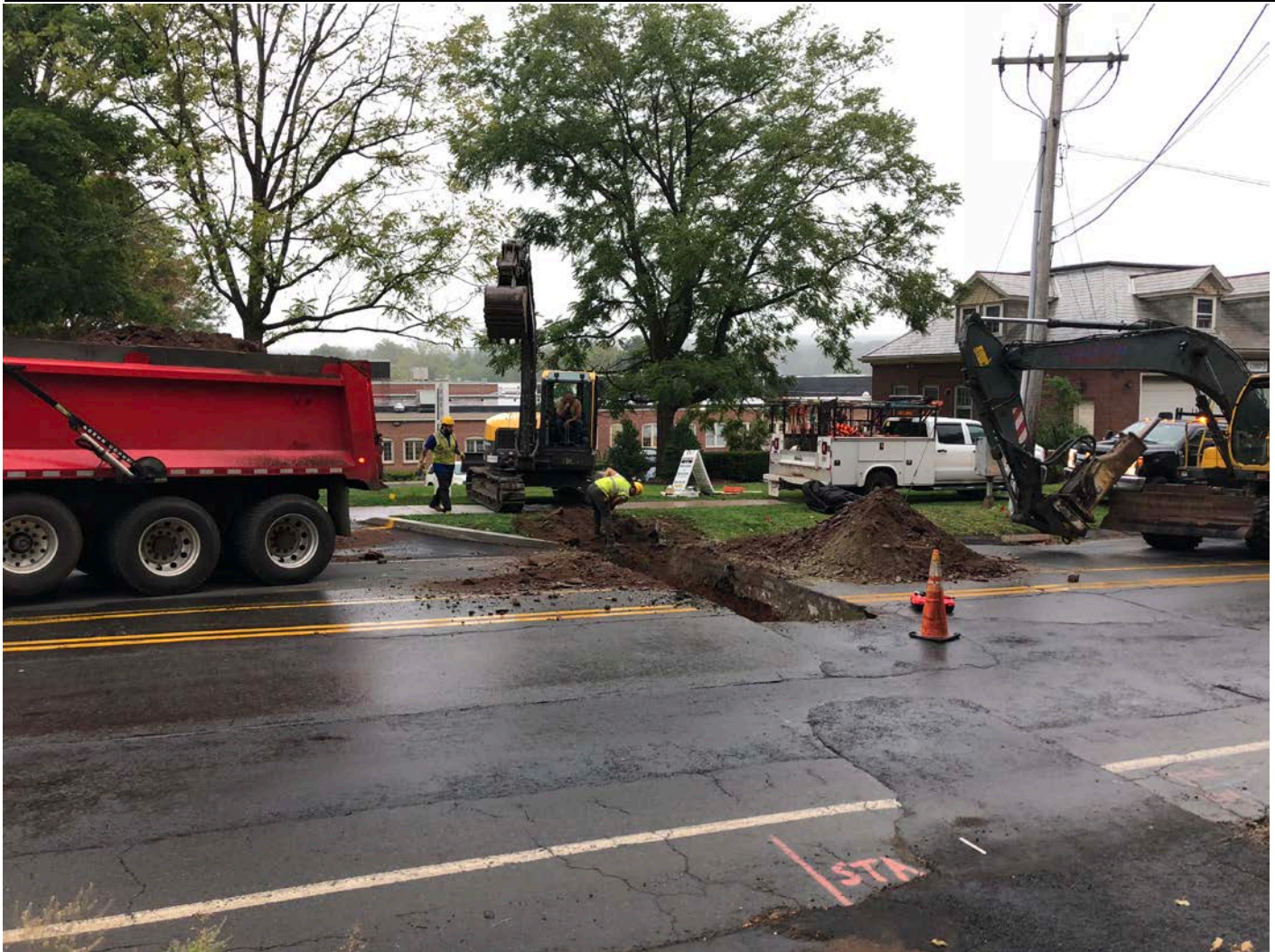
Picture 1: Ludlow installing 4" DIP at Station 198+10, Main Street, Durham. View to the east.
