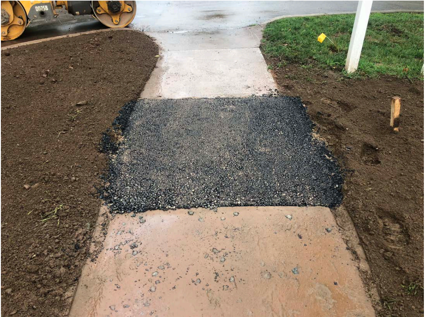
Picture 9: Sidewalk at Station 198+10 temporarily repaired with hot patch. Main Street, Durham. View to the south.
