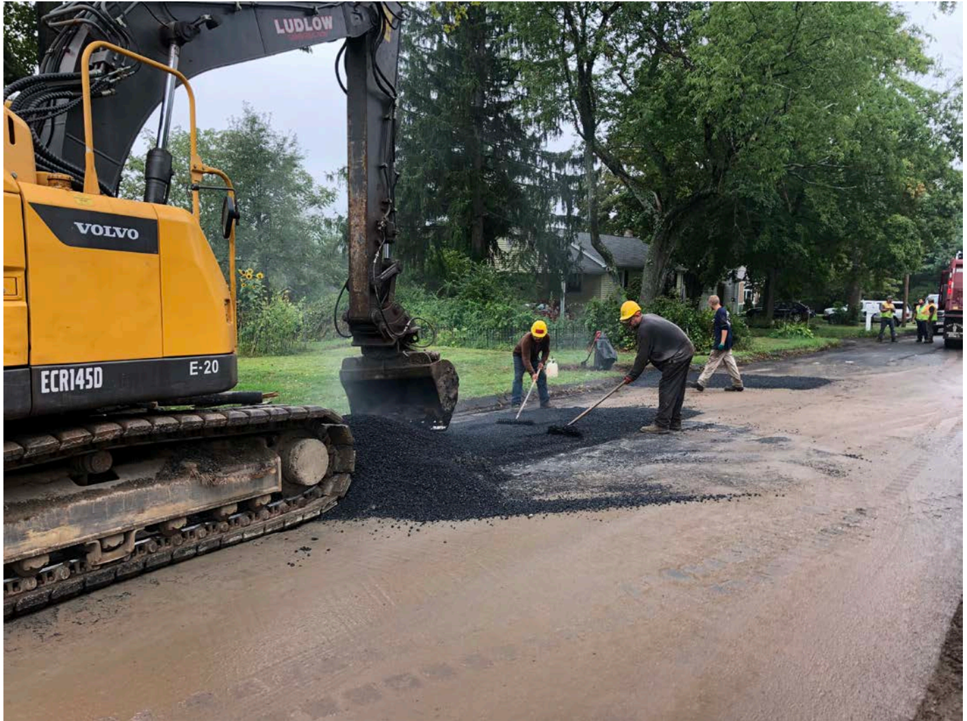
Picture 10: Ludlow placing hot patch on the trench that was excavated today for the installation of 8" DIP. Maple Avenue, Durham. View to the southwest.
