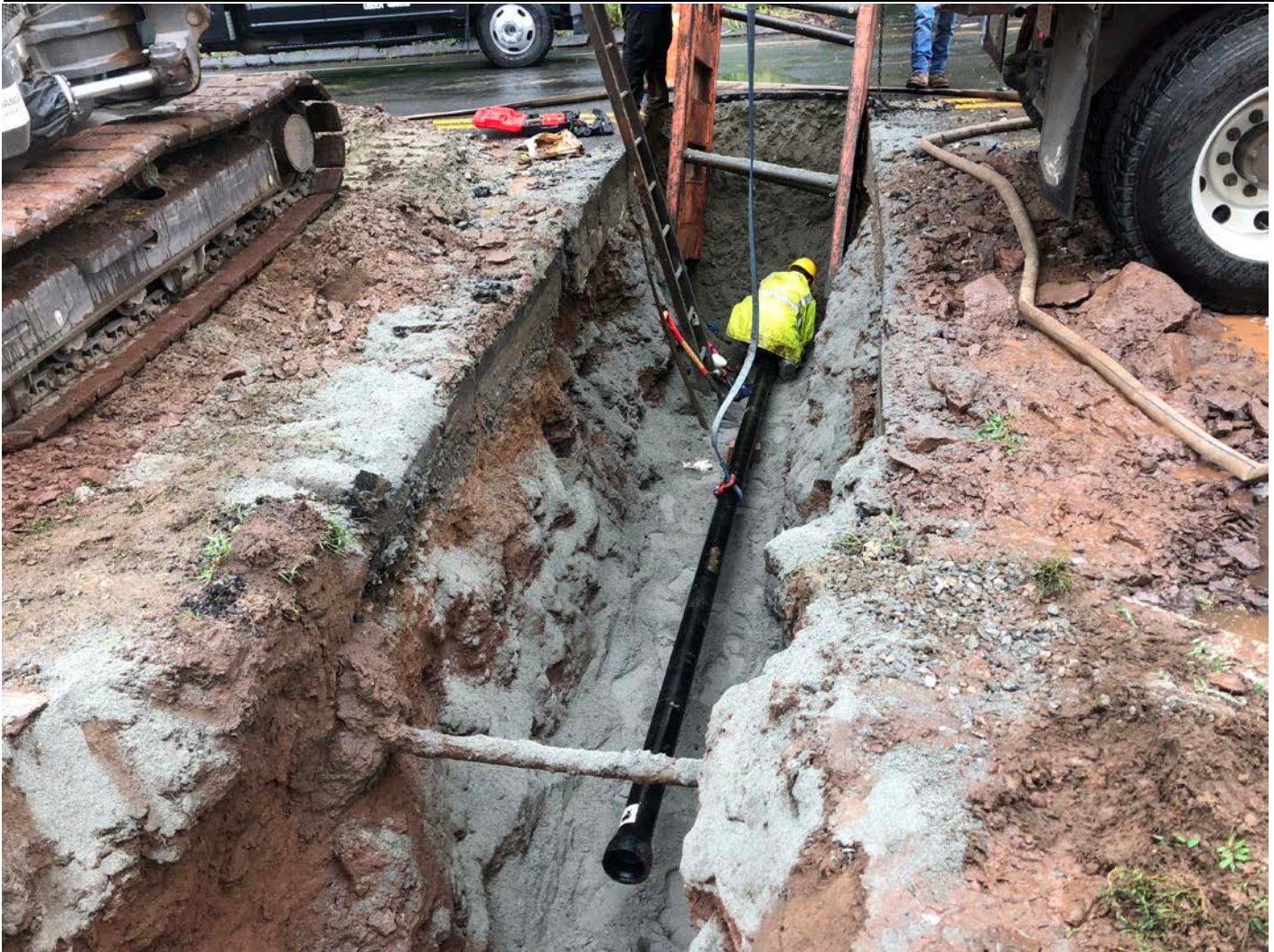
Picture 5: Ludlow installing 4" DIP at Station 198+10. 201-203 Main Street, Durham. View to the west.
