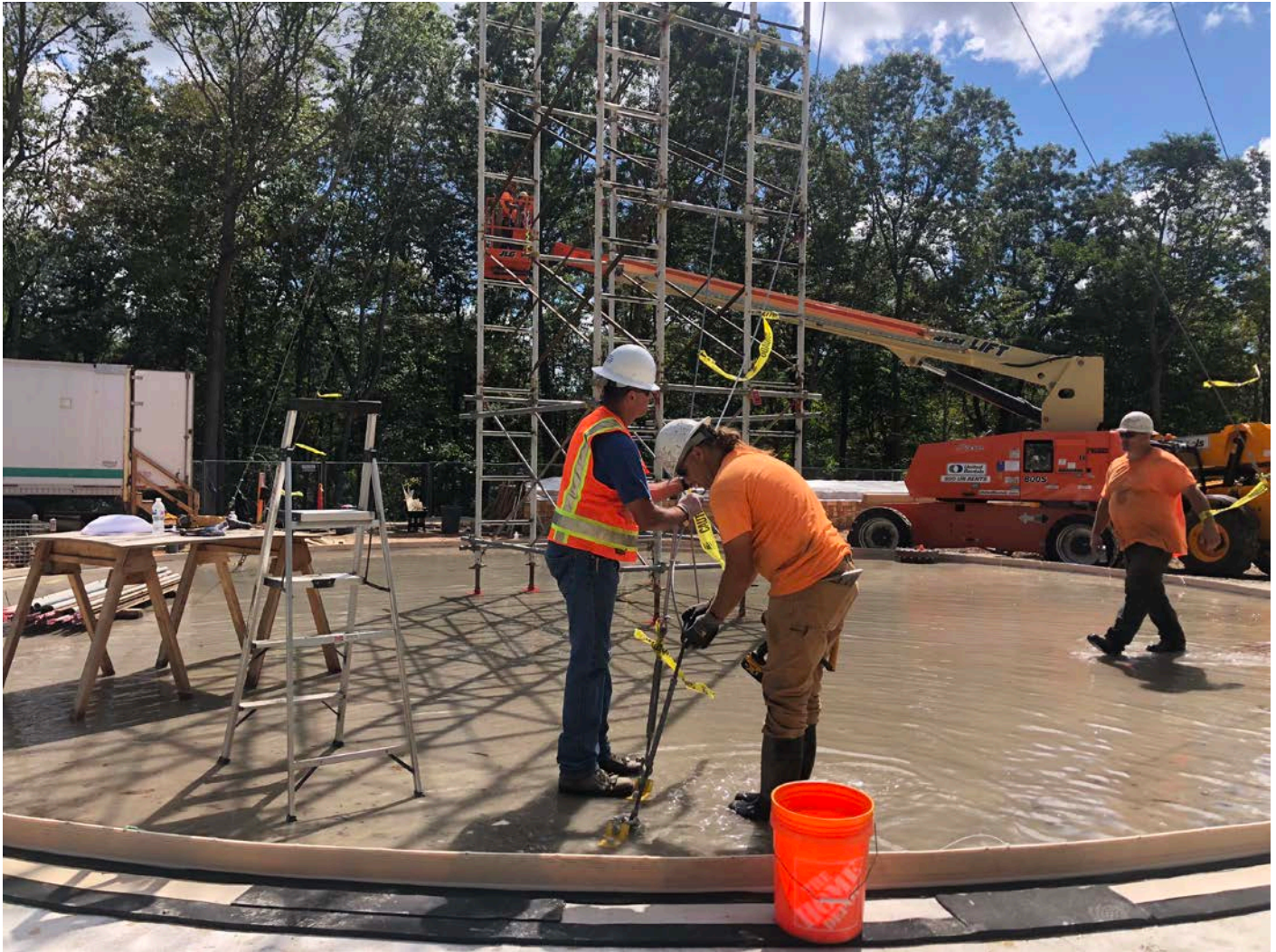
Picture 8: DN Tanks installing one of the center tower guidewires on the base of the water tank. Water tank work zone, east of the Shared Access Driveway, Middletown. View to the southeast.
