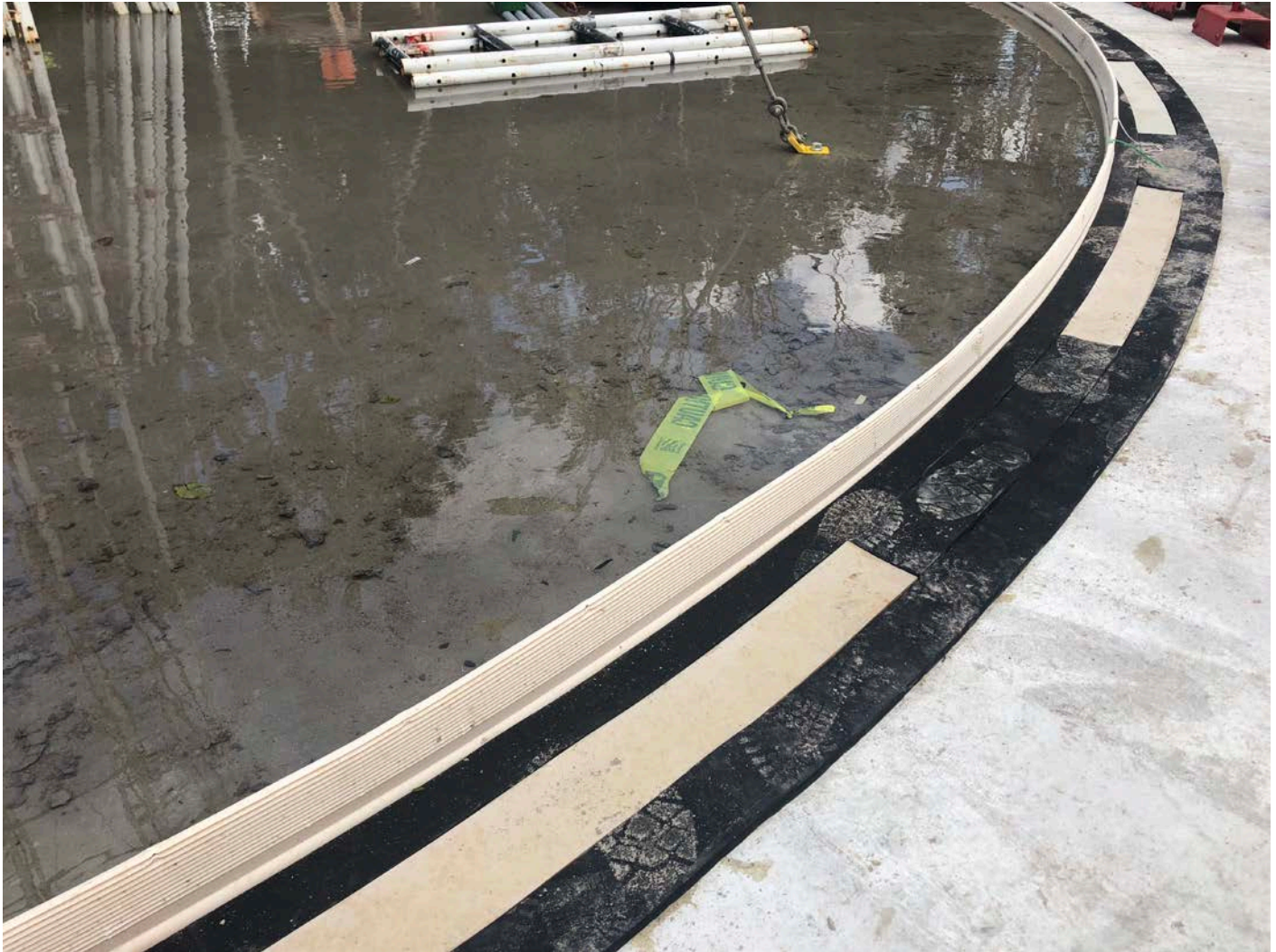
Picture 2: Foam padding after having been glued into place along the outer perimeter of the PVC water stop yesterday on the water tank base. Water tank work zone, east of the Shared Access Driveway, Middletown.
