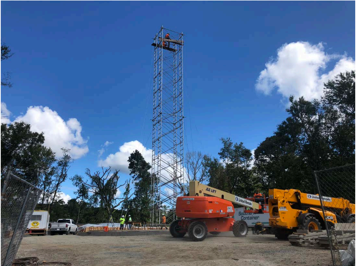
Picture 7: DN Tanks continuing to erect the center tower on the base of the water tank. Water tank work zone, east of the Shared Access Driveway, Middletown. View to the east.
