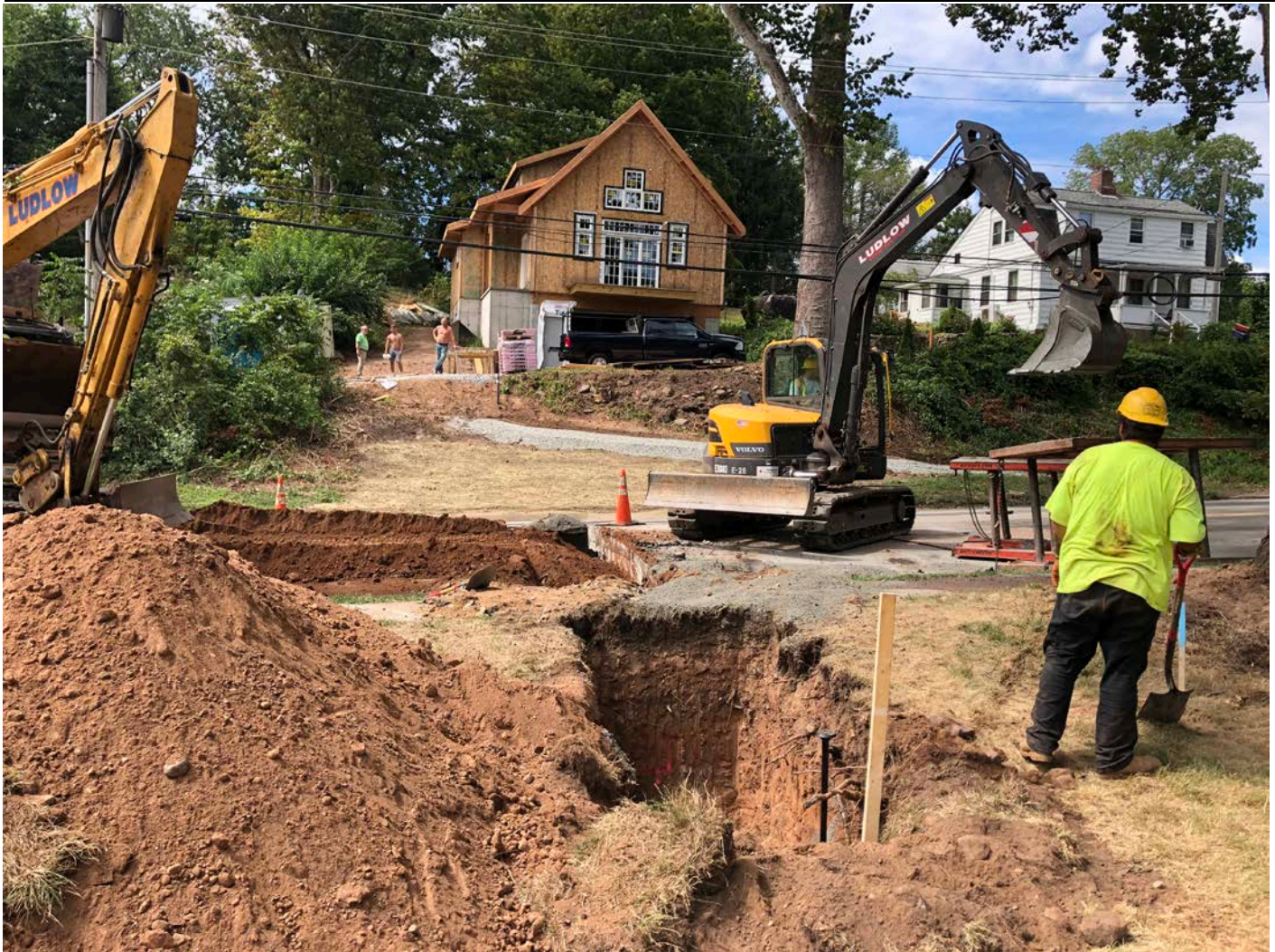
Picture 6: Ludlow installing a curb stop at Station 205+55, Main Street, Durham. View to the west.
