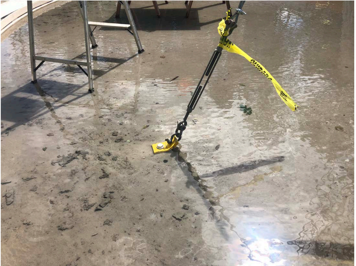
Picture 4: One of the center tower guidewires temporarily bolted to the water tank base. Water tank work zone, east of the Shared Access Driveway, Middletown.
