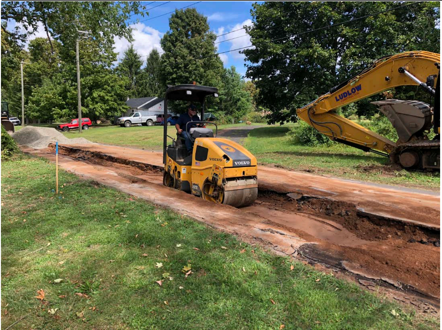
Picture 5: Ludlow compacting fill in the trench on Maple Avenue, Durham after the installation of 8" DIP. View to the northeast.
