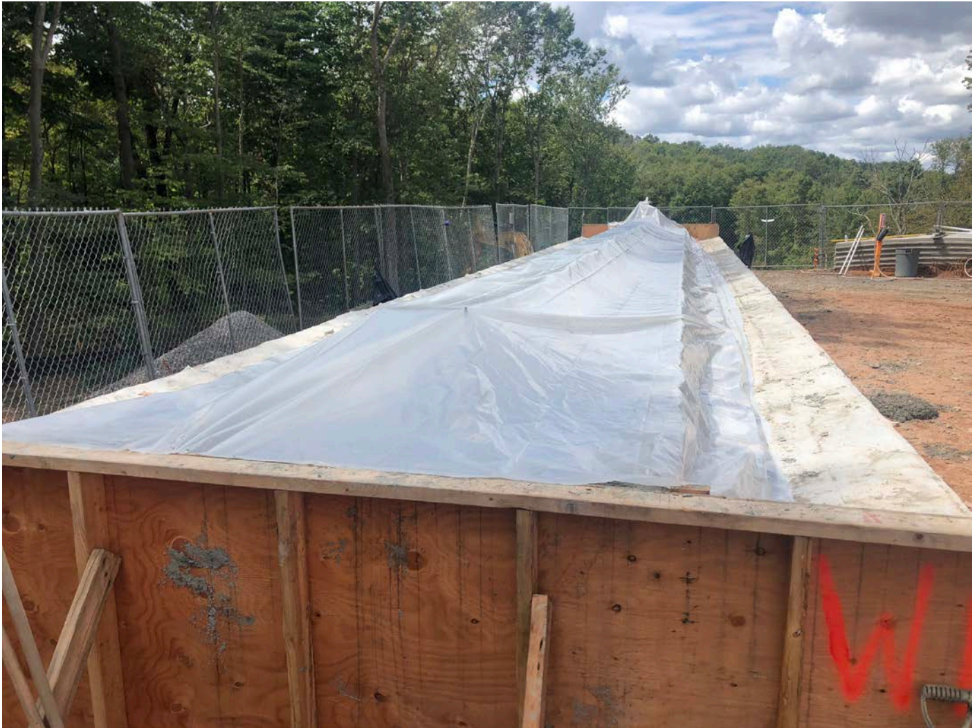
Picture 1: The narrow side panel form for the water tank, having been poured earlier in the day. Poly sheeting has been placed over the setting concrete. Water tank work zone, east of the Shared Access Driveway, Middletown. View to the west.
