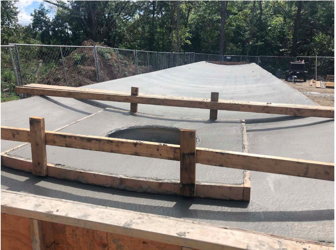
Picture 3: The wide side panel form for the water tank with a manway cast into it; poured earlier in the day. Water tank work zone, east of the Shared Access Driveway, Middletown.
