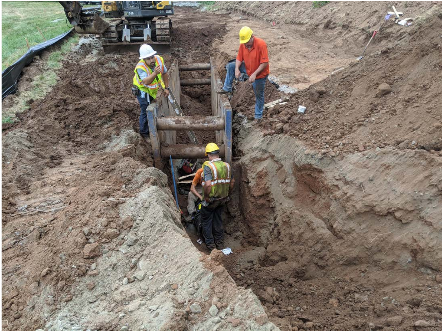
Picture 6: Ludlow Construction working on joining a 20' section of 12" DIP south of the stream crossing, Maple Avenue, Stations 904+50 to 902+03.5. View to the north.
