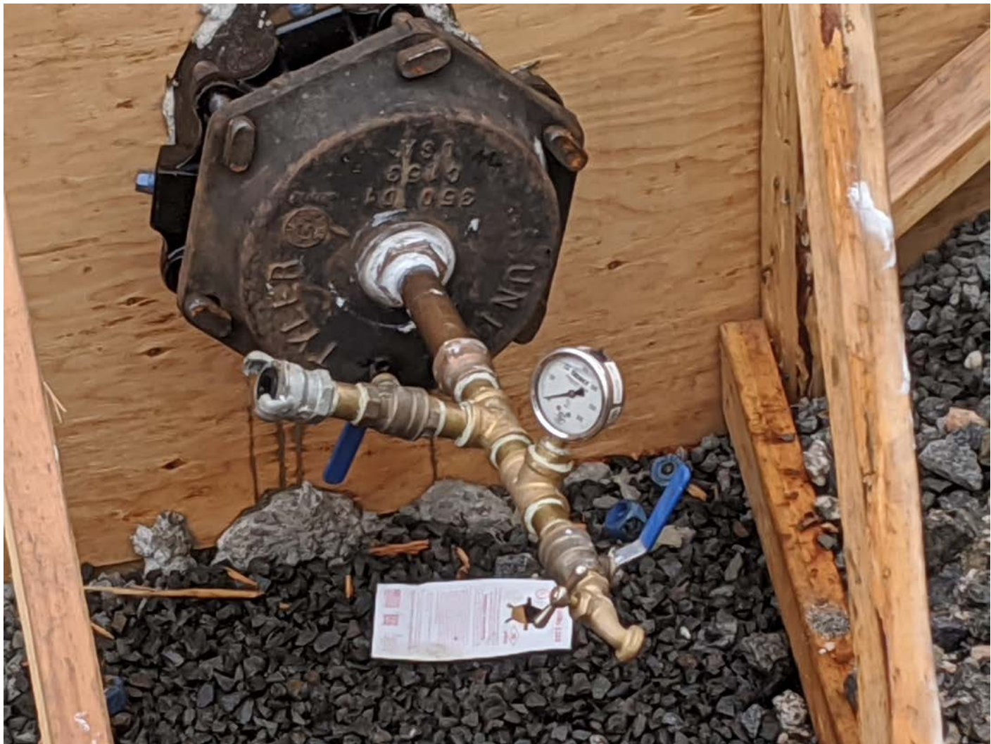
Picture 4: Pressure gauge attached to the water tank piping, Shared Access Driveway. View to the north.
