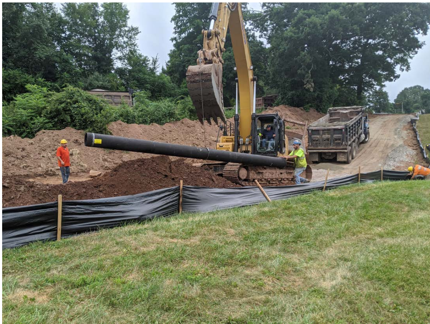
Picture 2: Ludlow construction installing a 20' section of DIP south of the stream crossing, Maple Avenue, Station 904+50 to 902+03.5. View to the east.
