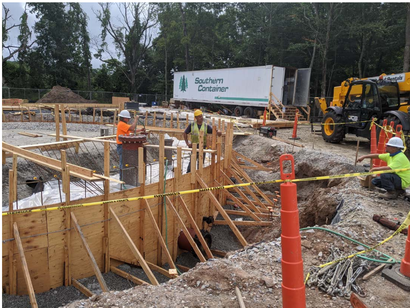
Picture 3: Ludlow Construction and DN Tanks preparing for the pressure testing of the water tank piping, Shared Access Driveway, View to the southeast.
