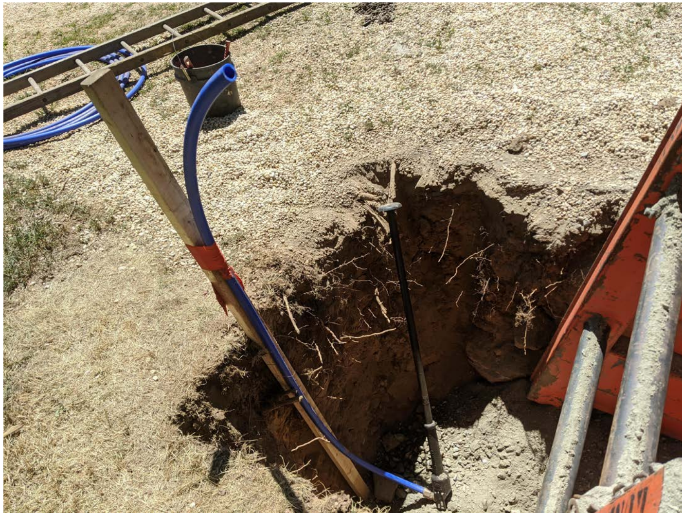
Picture 8: Curb stop installed at the station 182+50 located at 289 Main Street, Main Street, Station 182 + 50. View to the south.
