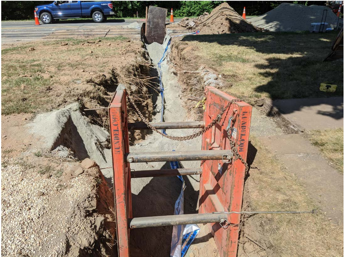
Picture 7: Trench line at station 182+50 backfilled with pea gravel and lined with caution tape, Main Street, Station 182+50. View to the west.
