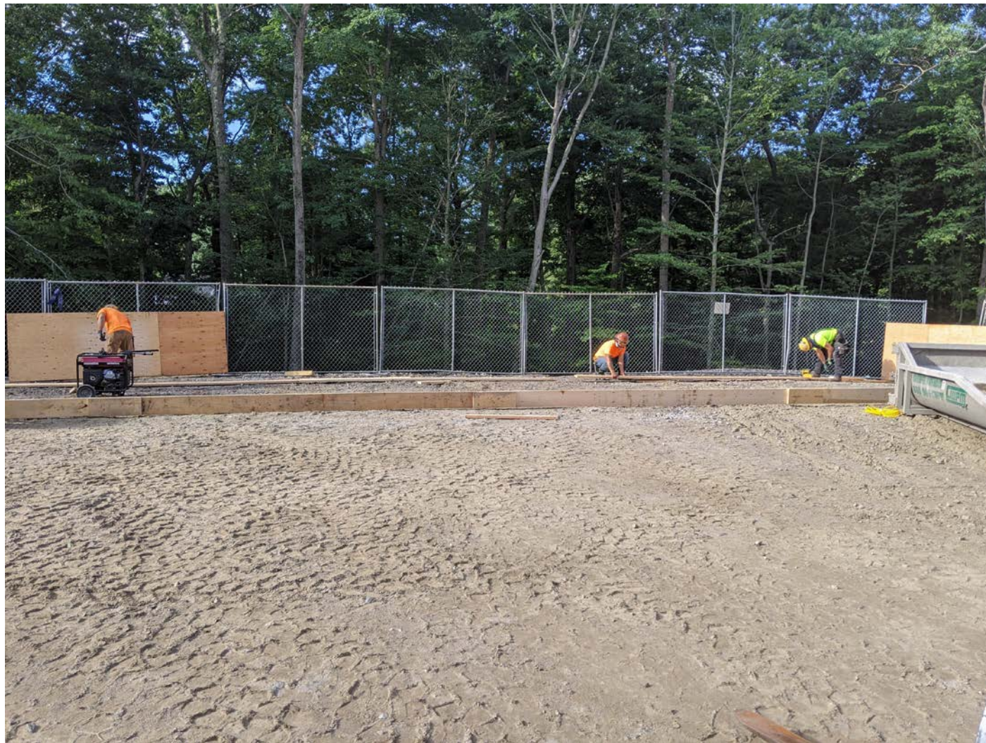
Picture 5: DN tanks working on the concrete forms for the water tank, Shared Access Driveway. View to the east.
