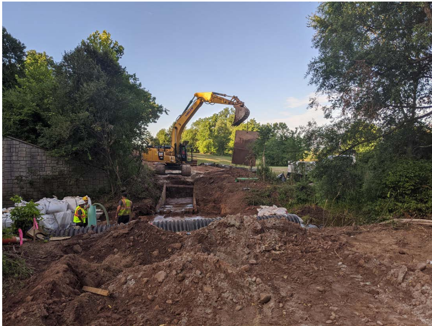
Picture 1: Ludlow construction removing shoring from the excavation area, Station 905 + 00. View to the south.
