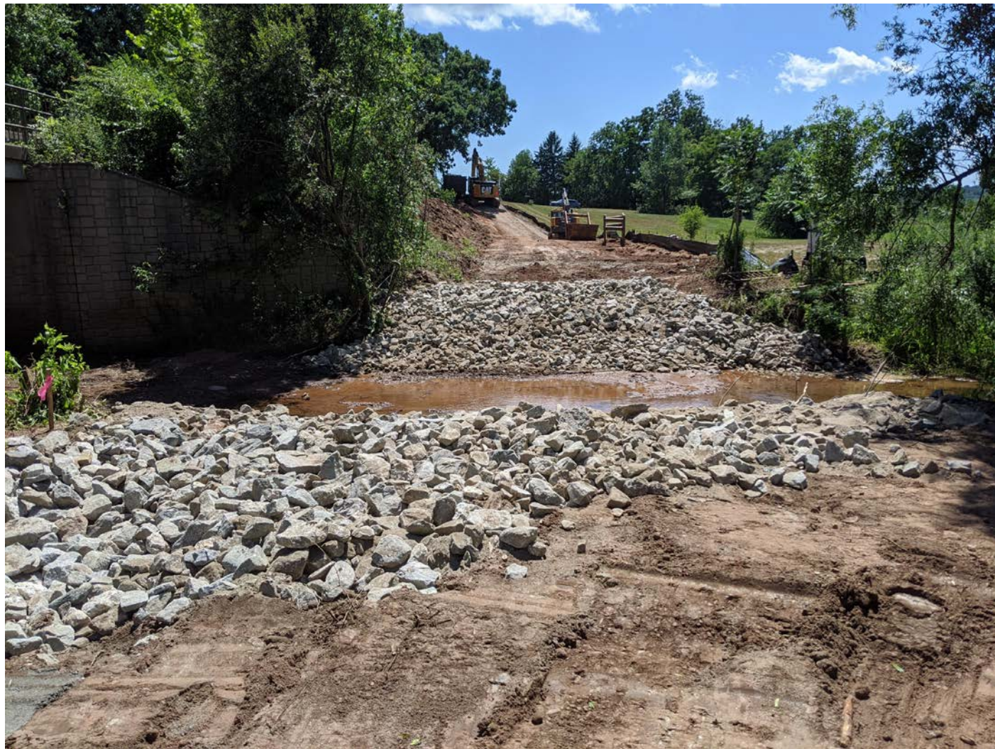
Picture 9: Rip rap placed on the banks of Allyn Brooke, Maple Avenue, Station 905 + 00. View to the south.
