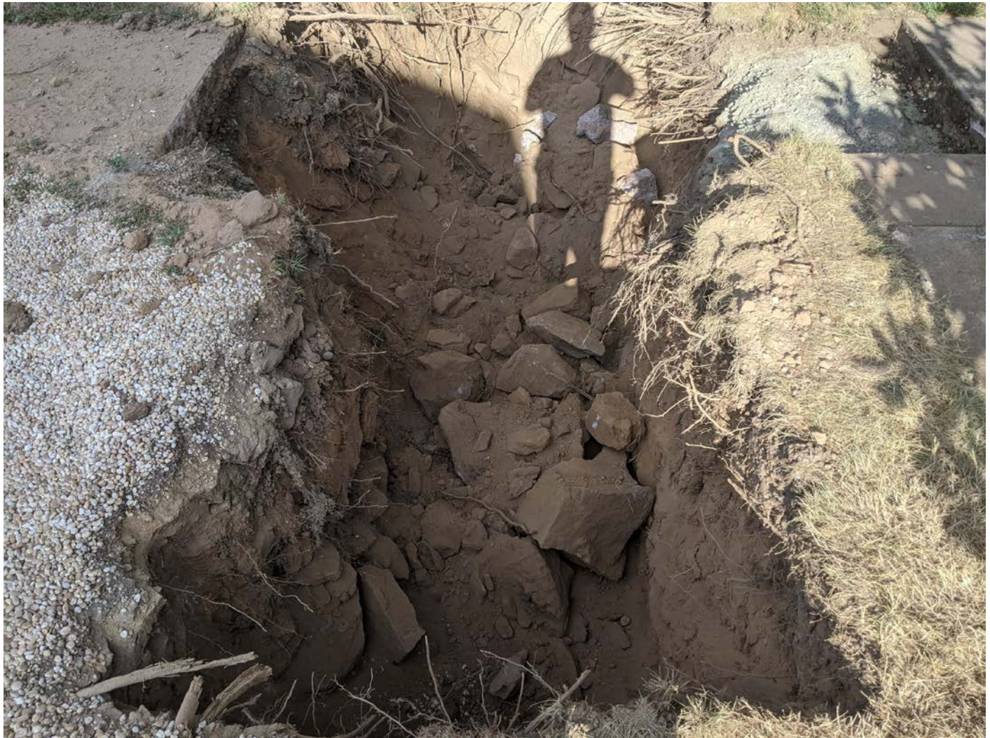
Picture 4: View of the ledge encountered in the trench line at station 182+50 on Main Street, Main Street, Stations 182+50. View to the west.
