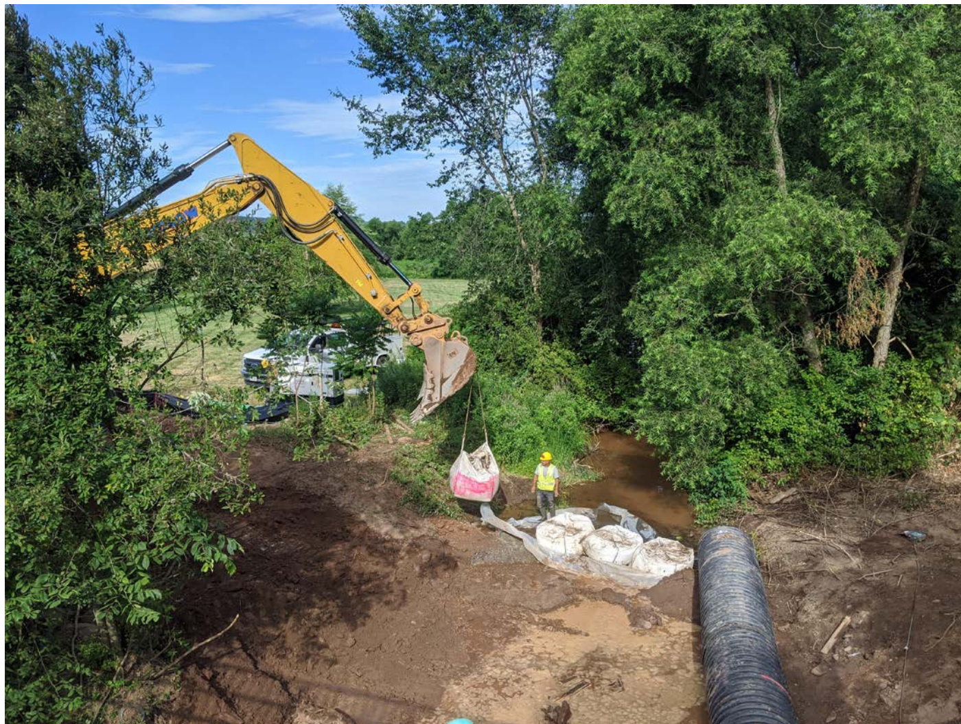
Picture 2: Ludlow construction removing sandbags from the stream bed, Maple Avenue, Station 905 + 00. View to the west.
