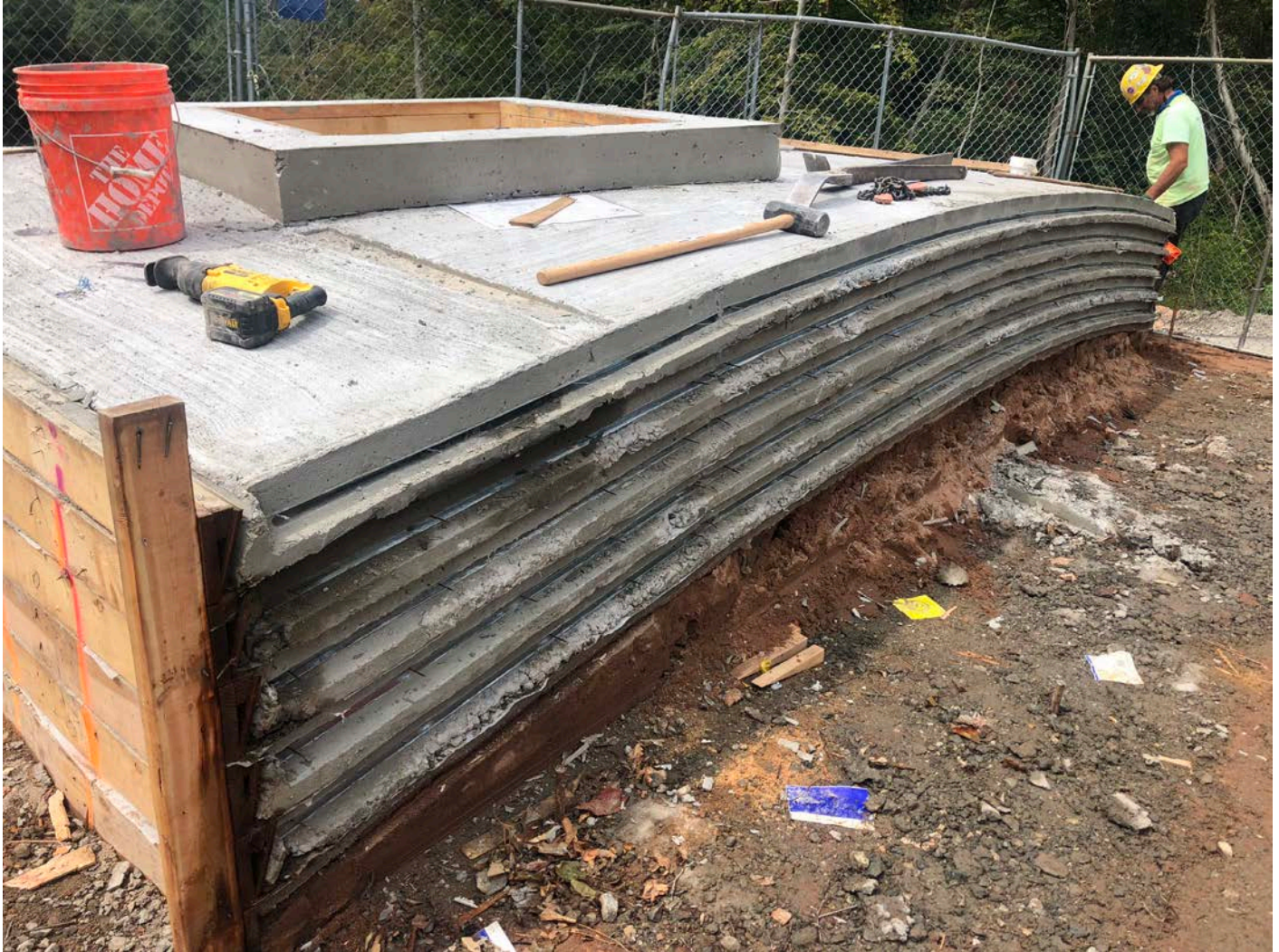
Picture 8: Water tank dome panels with the side of the concrete form removed. Water tank work zone, east of the Shared Access Driveway, Middletown. View to the northwest.
