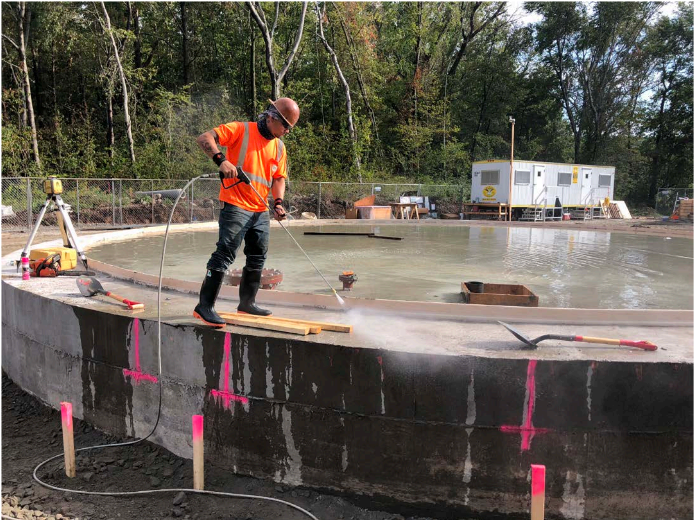
Picture 3: DN Tanks using pressure washer to clean concrete from top of PVC water stop on the water tank base. Water tank work zone, east of the Shared Access Driveway, Middletown. View to the north.
