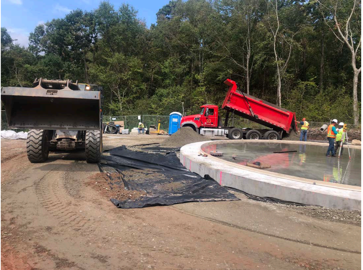
Picture 9: Ludlow placing geotextile fabric covered with gravel to finish the installation of the 6" underdrain pipe they just installed around the periphery of the water tank base. Water tank work zone, east of the Shared Access Driveway, Middletown. View to the north.
