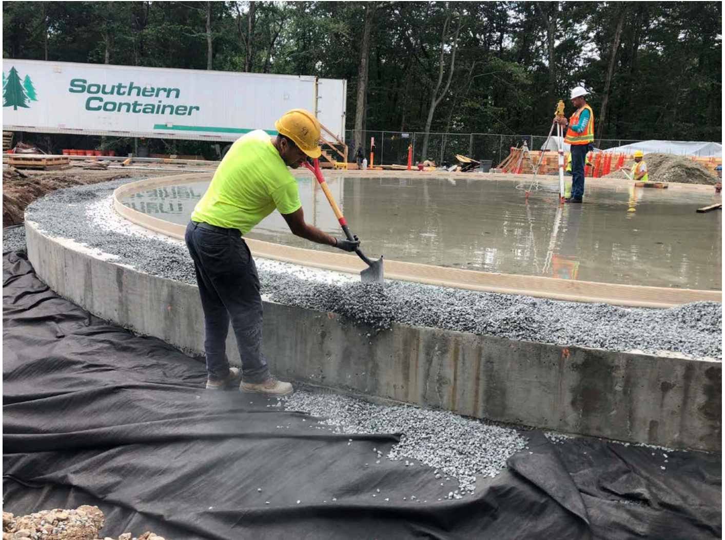
Picture 6: Ludlow placing geotextile fabric covered with stone over the 6" underdrain pipe they just installed around the periphery of the water tank base. Water tank work zone, east of the Shared Access Driveway, Middletown. View to the south.
