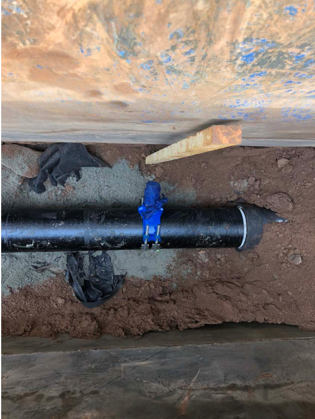
Picture 10: 1.5" corporation stop installed by Ludlow on Maple Avenue, Durham at Station 934+68.
