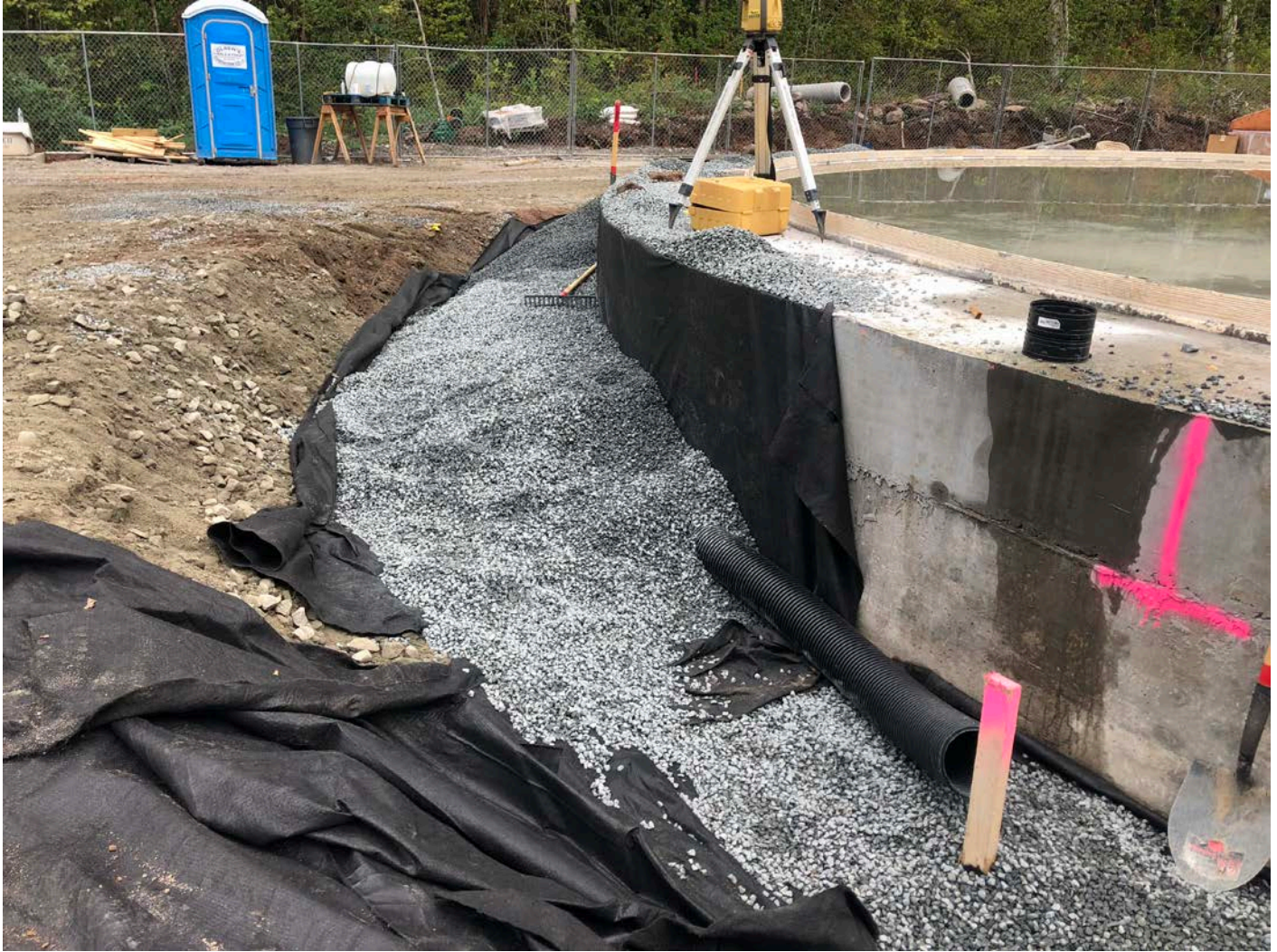
Picture 4: Ludlow installing 6" plastic underdrain pipe around the periphery of the water tank base. Water tank work zone, east of the Shared Access Driveway, Middletown. View to the north.
