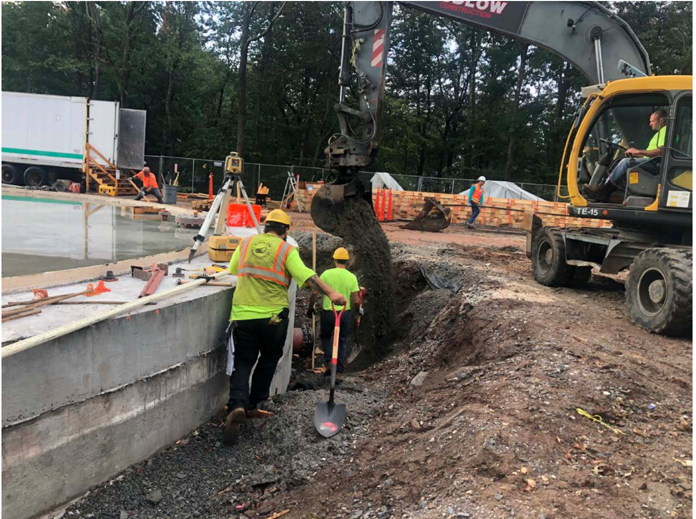
Picture 2: Ludlow placing fill around the periphery of the water tank base. Water tank work zone, east of the Shared Access Driveway, Middletown. View to the south.
