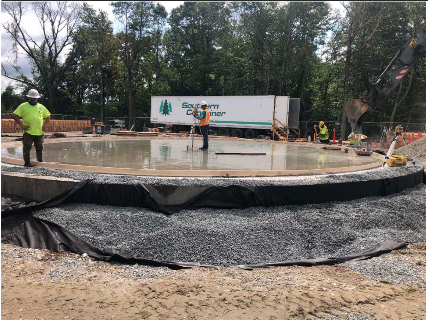
Picture 7: Another view of the geotextile fabric covered with stone that was placed over the 6" underdrain pipe that Ludlow installed around the periphery of the water tank base. Water tank work zone, east of the Shared Access Driveway, Middletown. View to the west.
