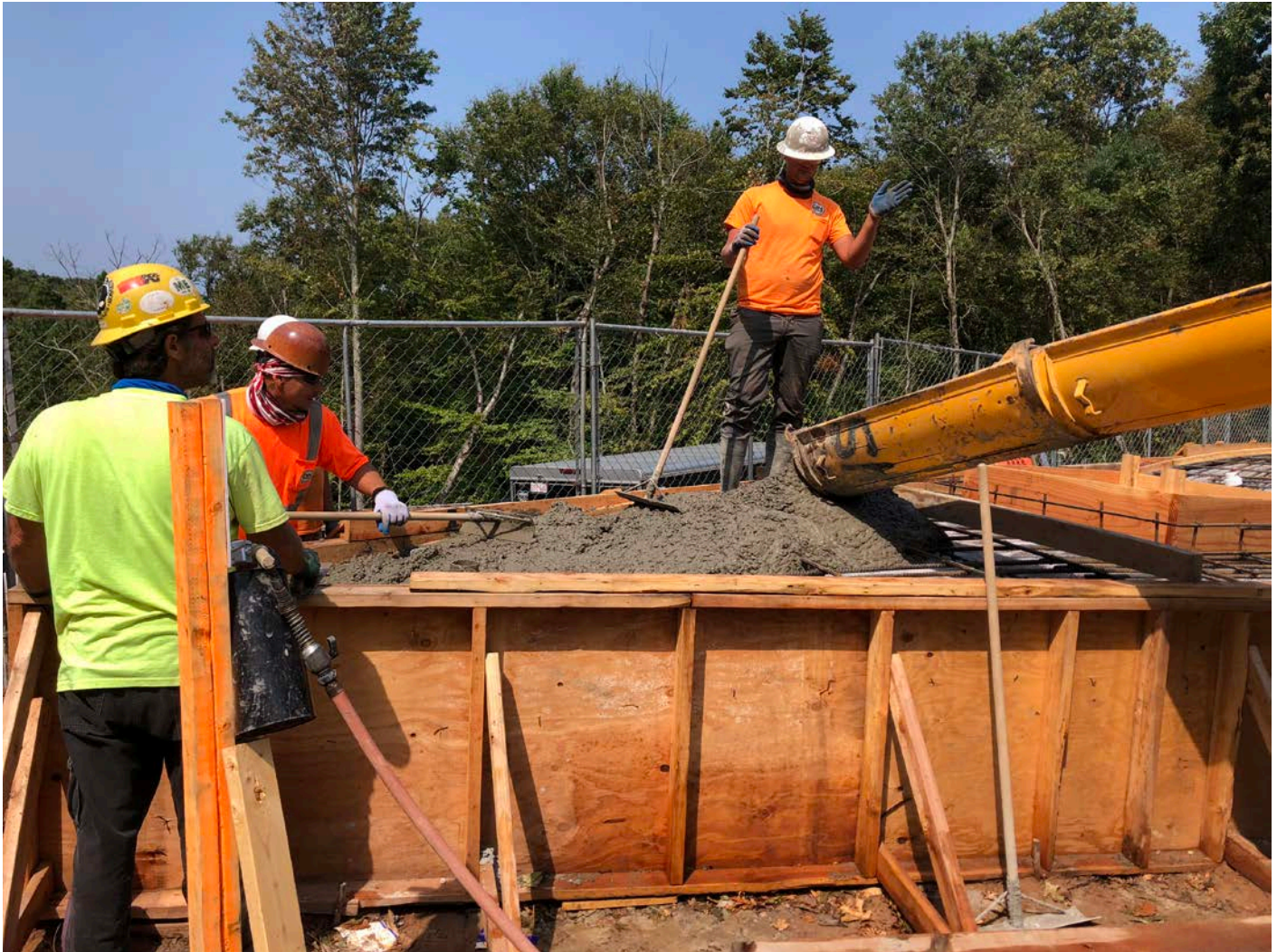
Picture 7: DN Tanks placing concrete on one of the water tank dome panel forms. Water tank work zone, east of the Shared Access Driveway, Middletown.
