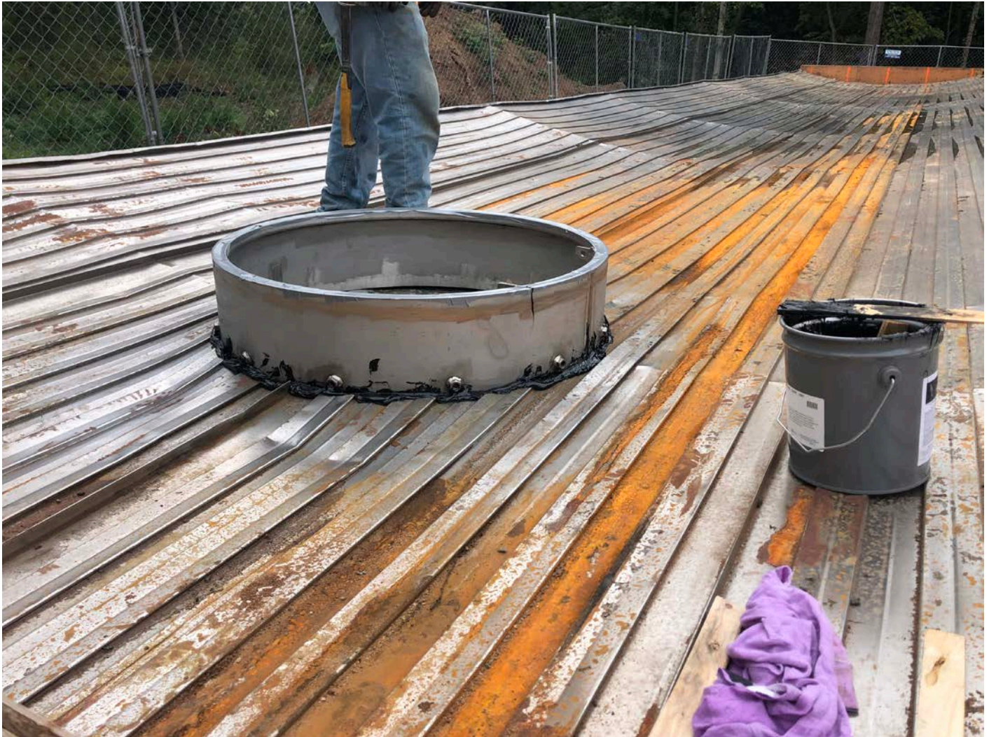
Picture 4: DN Tanks placing a manway on the wide side panel concrete form. Water tank work zone, east of the Shared Access Driveway, Middletown.
