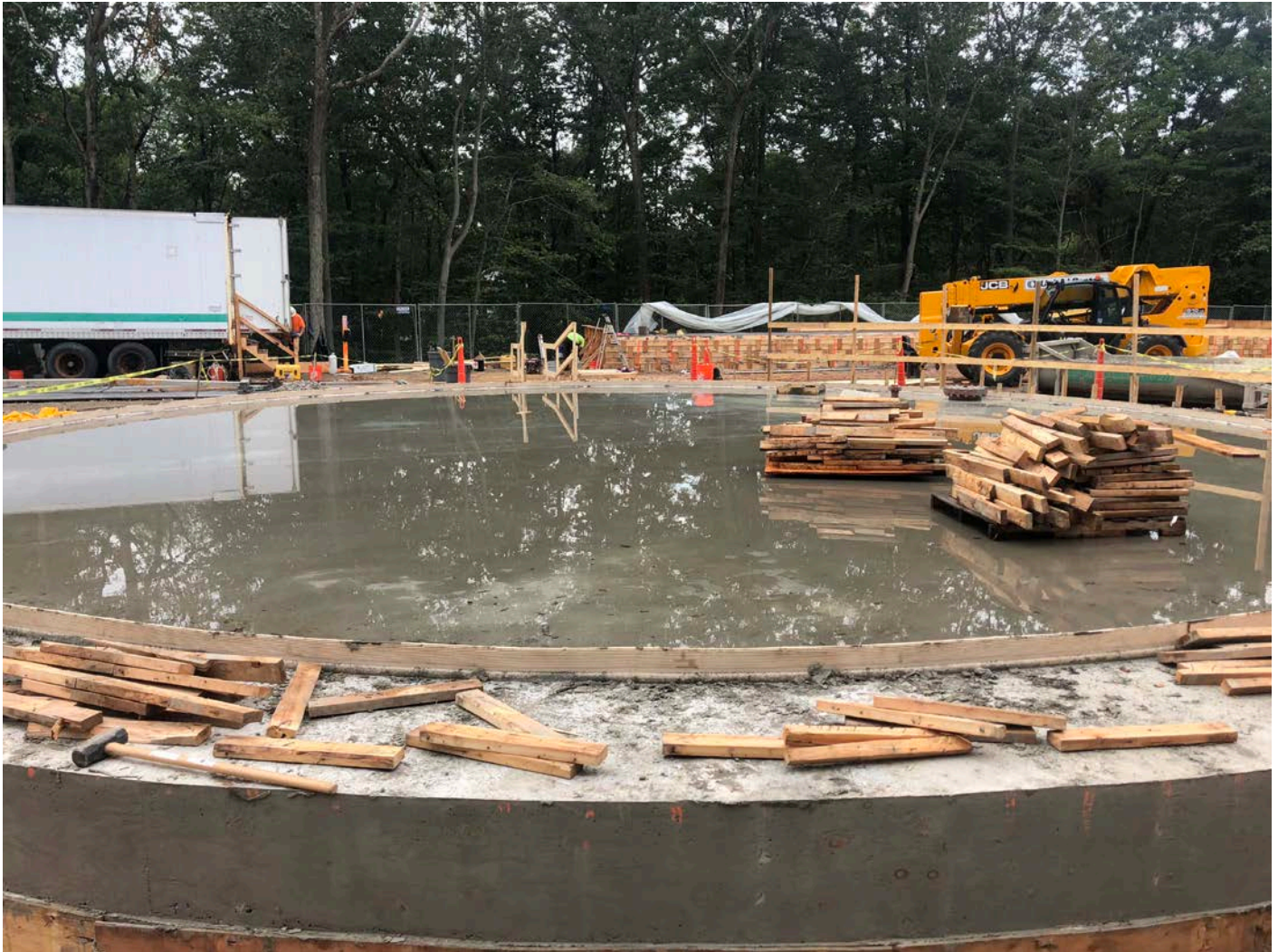
Picture 3: The top of the water tank base with a layer of water on top of it to slow the cure of the concrete. Water tank work zone, east of the Shared Access Driveway, Middletown. View to the south.
