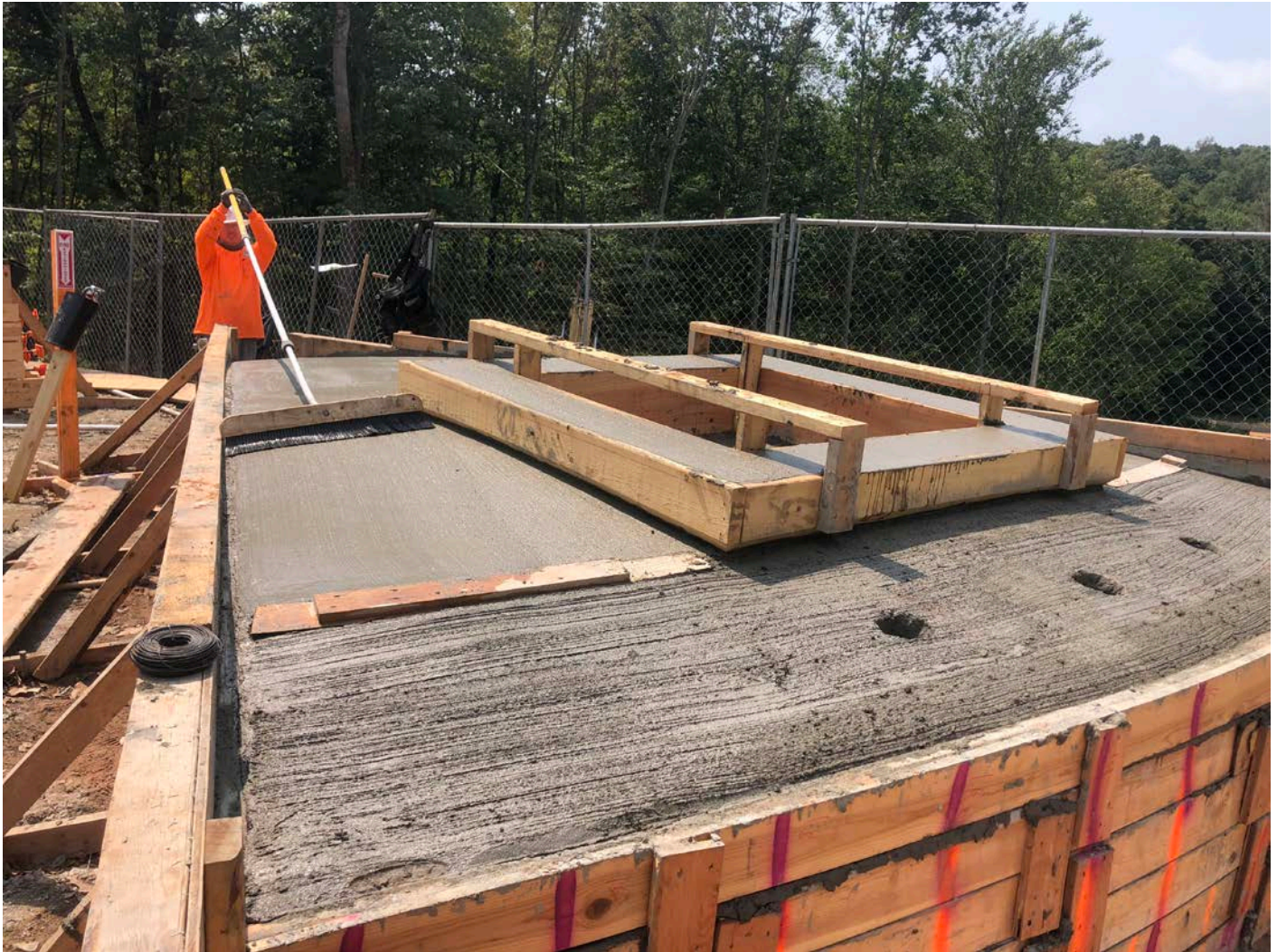
Picture 10: DN Tanks finishing the surface of freshly-placed concrete on one of the water tank dome panel forms. Water tank work zone, east of the Shared Access Driveway, Middletown. View to the south.
