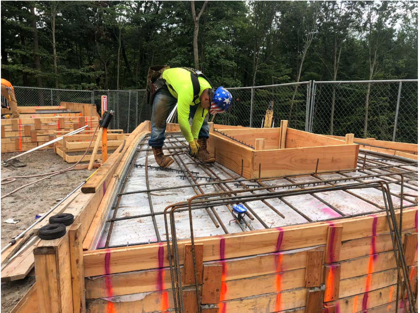
Picture 5: Northeastern Steel placing and fastening rebar on one of the water tank dome forms. Water tank work zone, east of the Shared Access Driveway, Middletown. View to the south.
