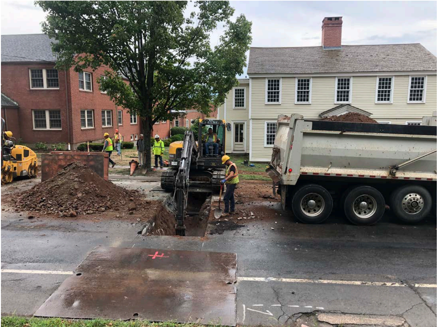
Picture 2: Ludlow installing a curb stop at Station 200+22 (199 Main Street, Durham). View to the east.
