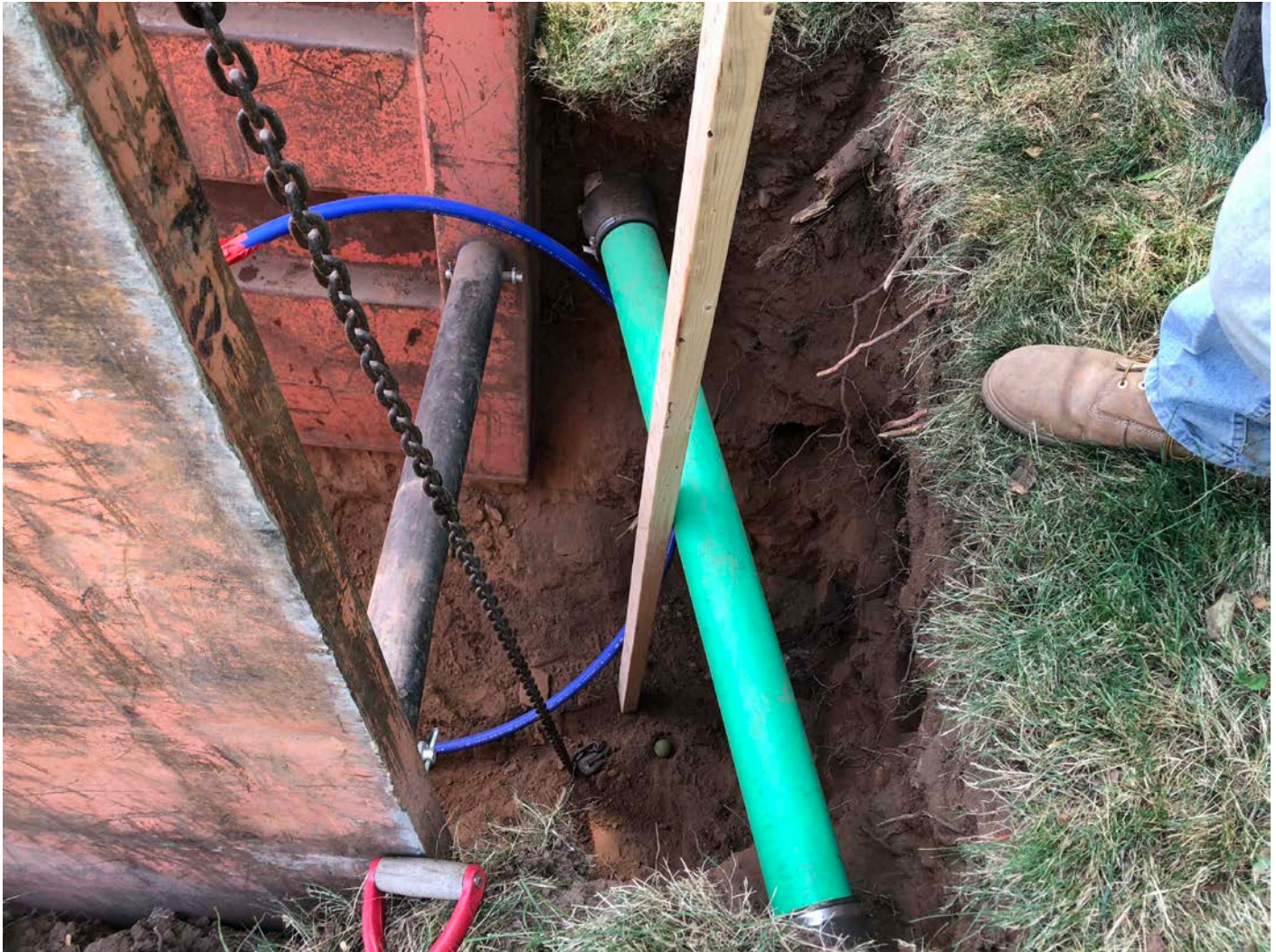
Picture 8: PVC drainpipe that was damaged and repaired by Ludlow at 202 Main Street, Durham during the installation of a curb stop.
