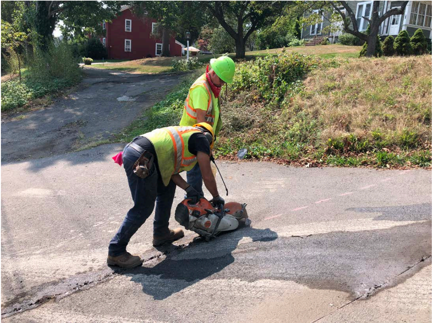
Picture 9: Ludlow saw cutting pavement at 196 Main Street, Durham (Station 201+36) for the installation of a curb stop. View to the southeast.
