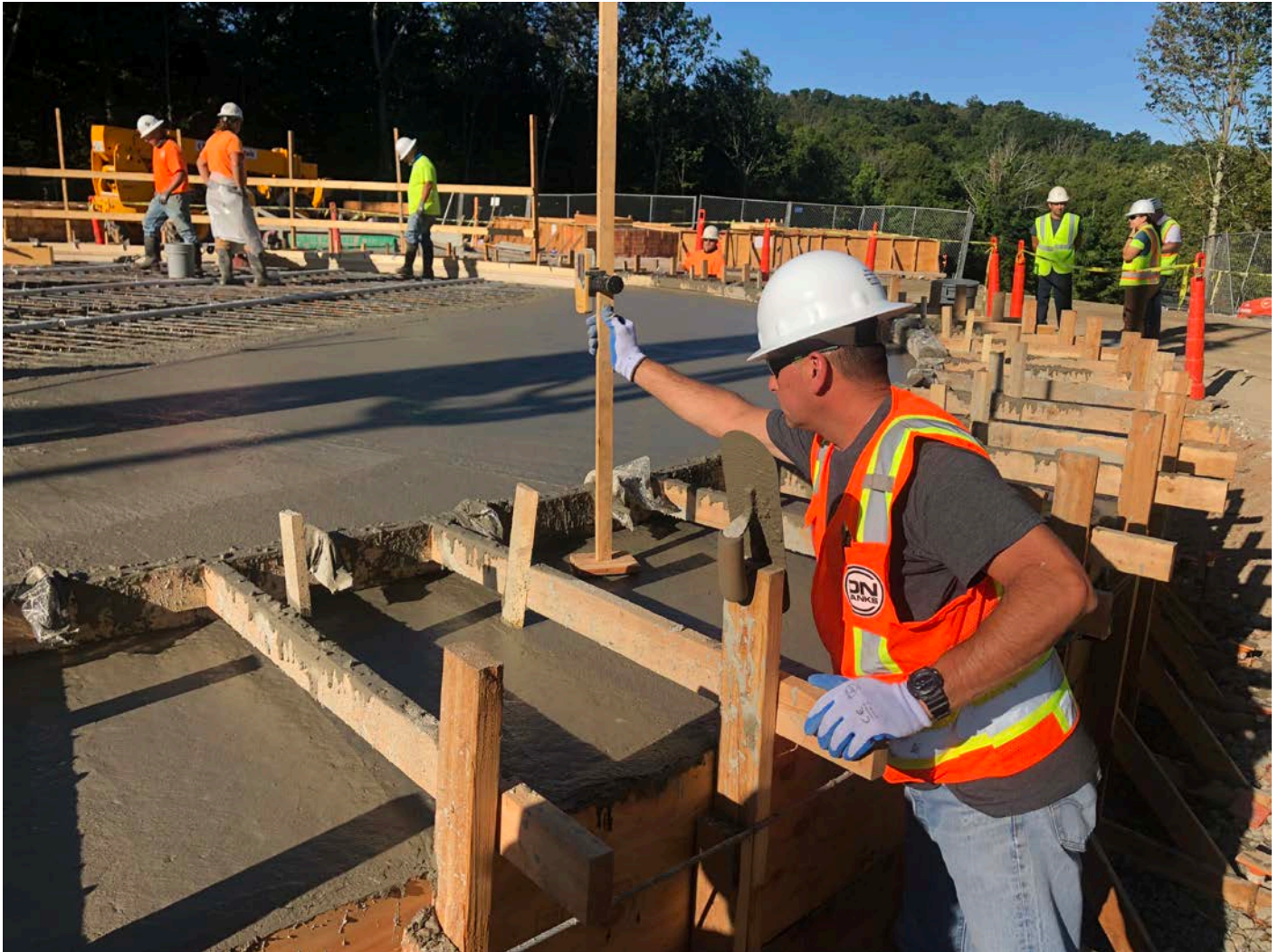
Picture 5: DN Tanks checks the elevation of the freshly-placed concrete for the water tank base. Water tank work zone, east of the Shared Access Driveway, Middletown. View to the south.
