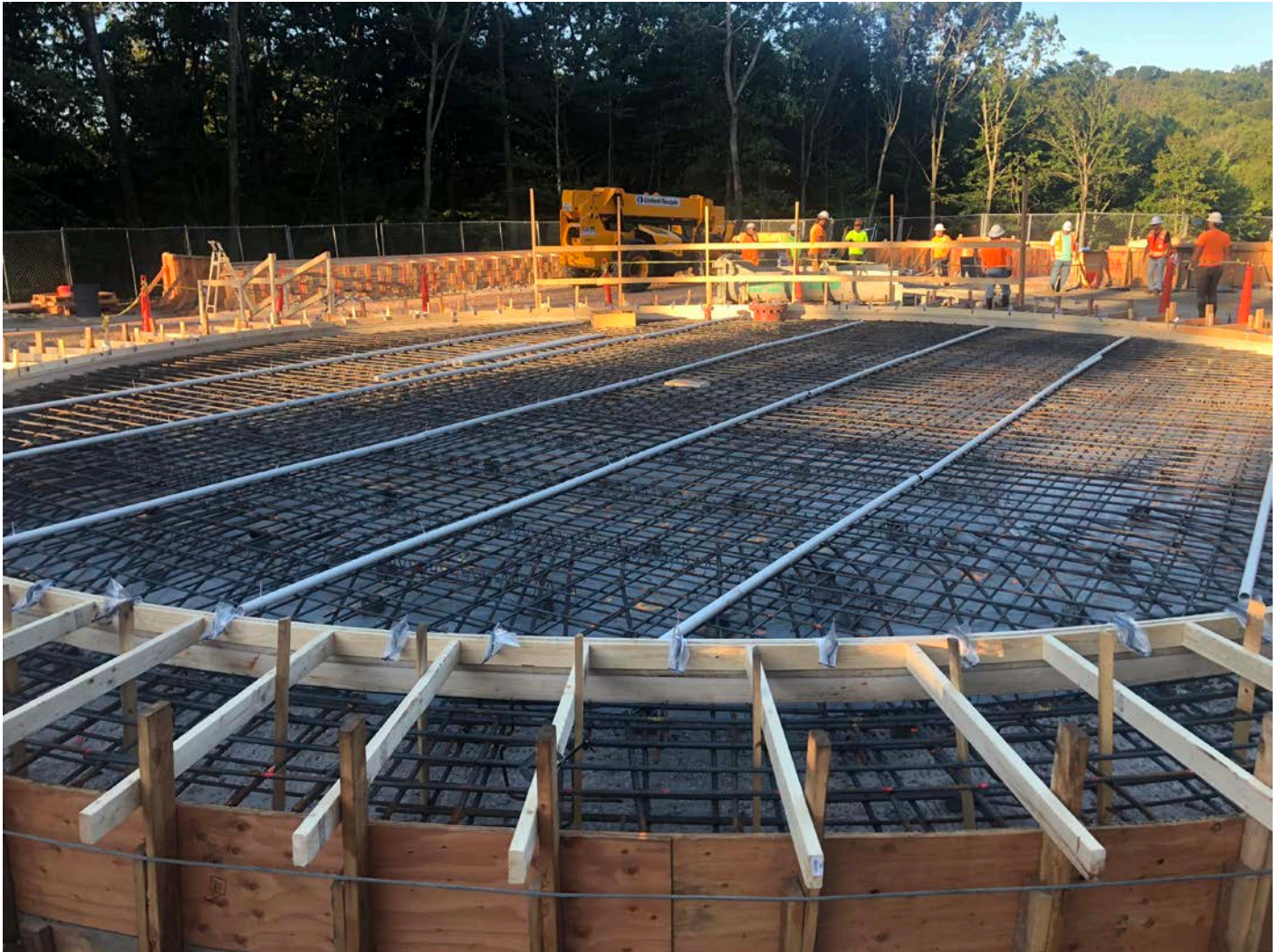
Picture 1: Water tank base laid out with rebar, water stop clamped in place, and PVC pipe temporarily placed to guide the power bull float once concrete has been poured. Water tank work zone, east of the Shared Access Driveway, Middletown. View to the west.
