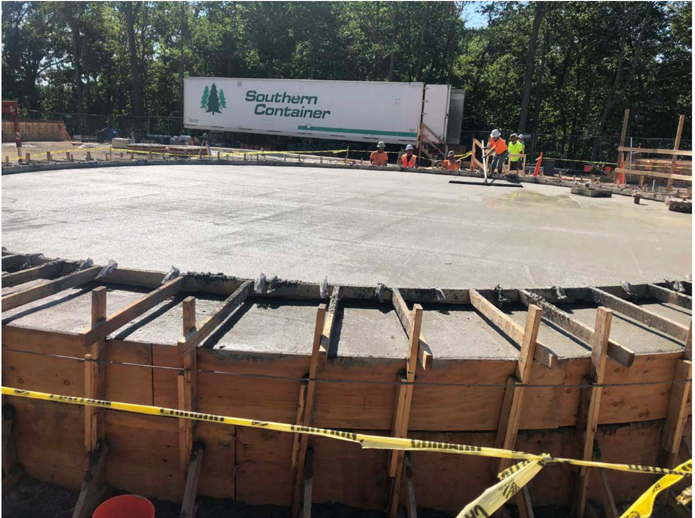
Picture 8: DN Tanks finishing smoothing of surface of the freshly-place concrete at the water tank base. Water tank work zone, east of the Shared Access Driveway, Middletown. View to the south.
