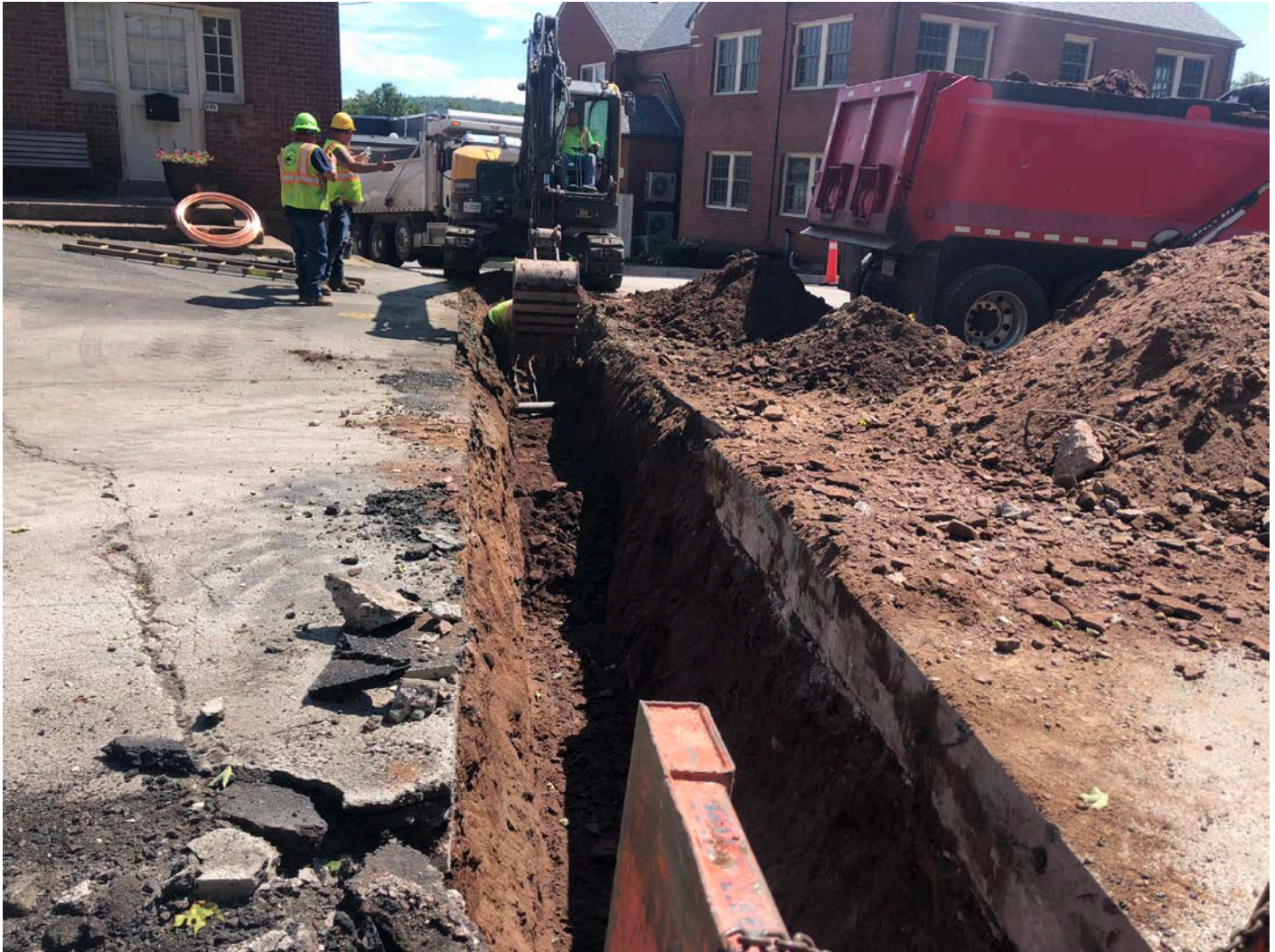
Picture 9: Ludlow installing a curb stop at 205 Main Street (Station 199+12). Main Street, Durham. View to the east.
