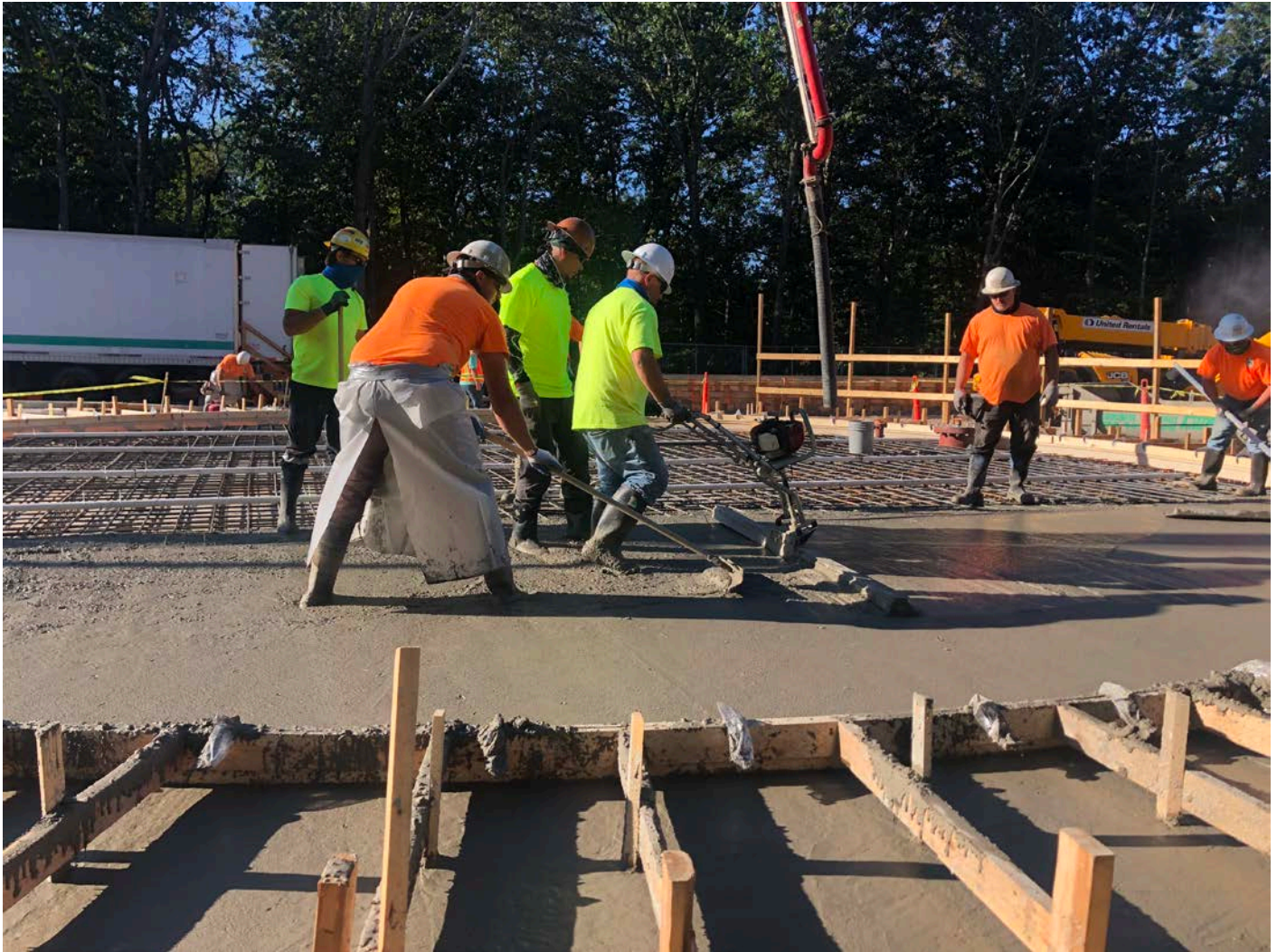
Picture 4: DN Tanks using the power bull float to smooth and level freshly-poured concrete for the water tank base. Water tank work zone, east of the Shared Access Driveway, Middletown. View to the south.
