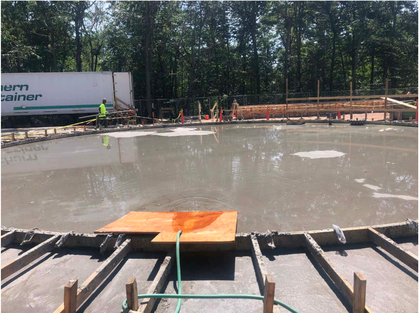
Picture 10: Freshly-placed concrete at the water tank base, with a layer of water placed over it in order to slow the cure. Water tank work zone, east of the Shared Access Driveway, Middletown. View to the south.
