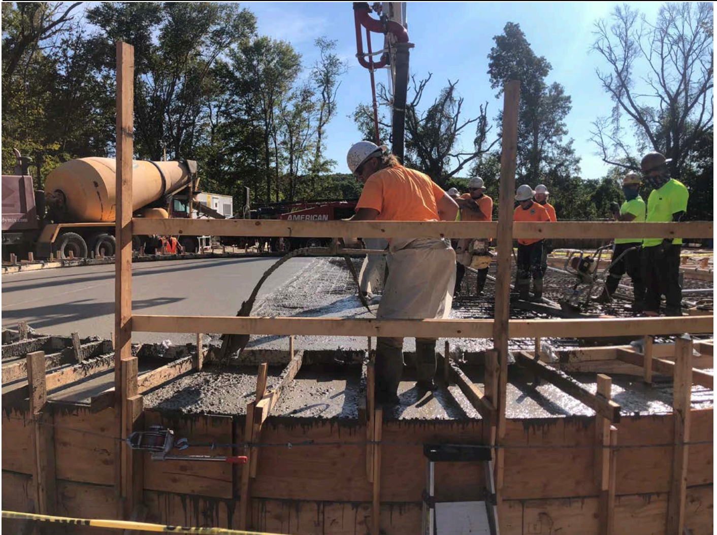
Picture 7: DN Tanks vibrating freshly-placed concrete at the water tank base. Water tank work zone, east of the Shared Access Driveway, Middletown. View to the east.
