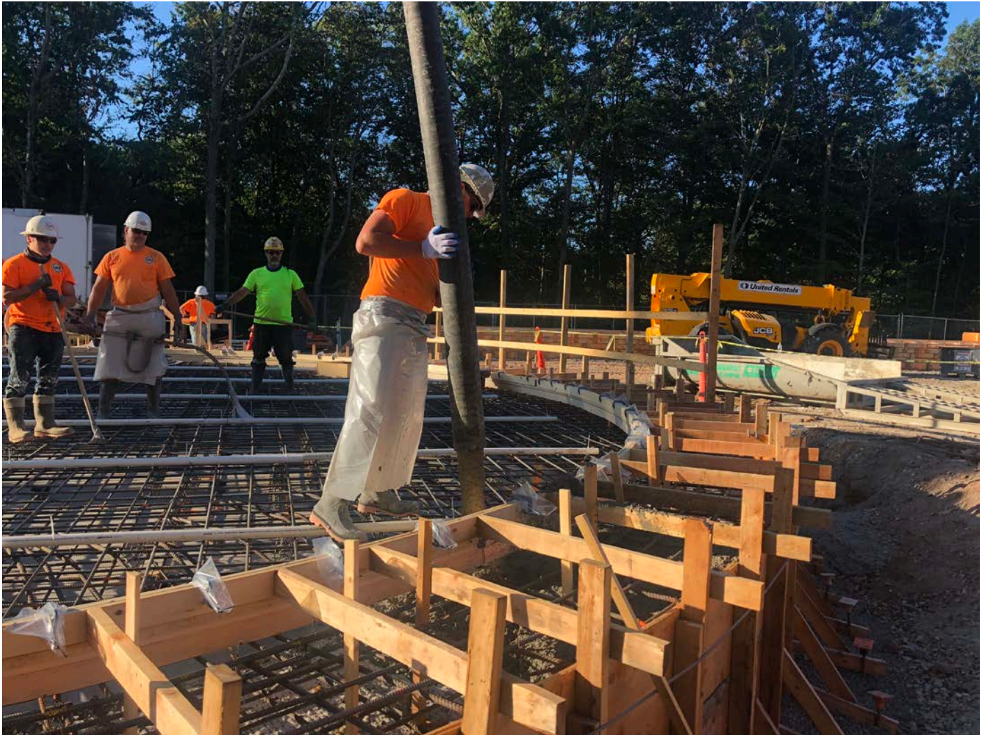
Picture 2: DN Tanks beginning to pour concrete for the water tank base. Water tank work zone, east of the Shared Access Driveway, Middletown. View to the south.
