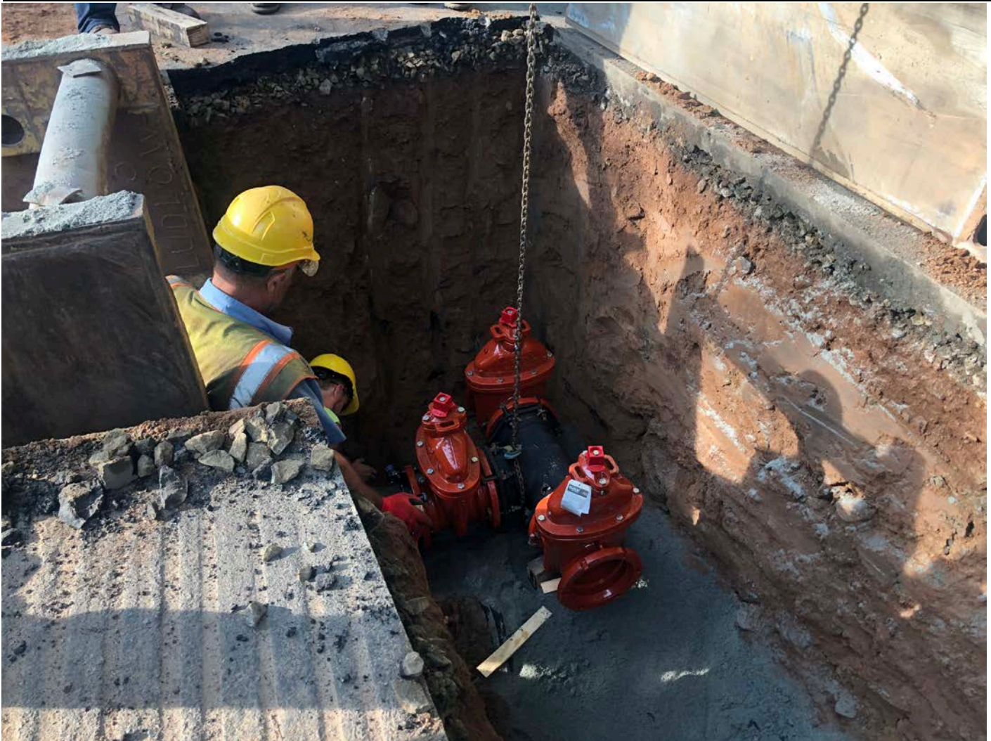
Picture 3: Ludlow installing three 8" gate valves and gate boxes at Station 940+52. View to the south.
