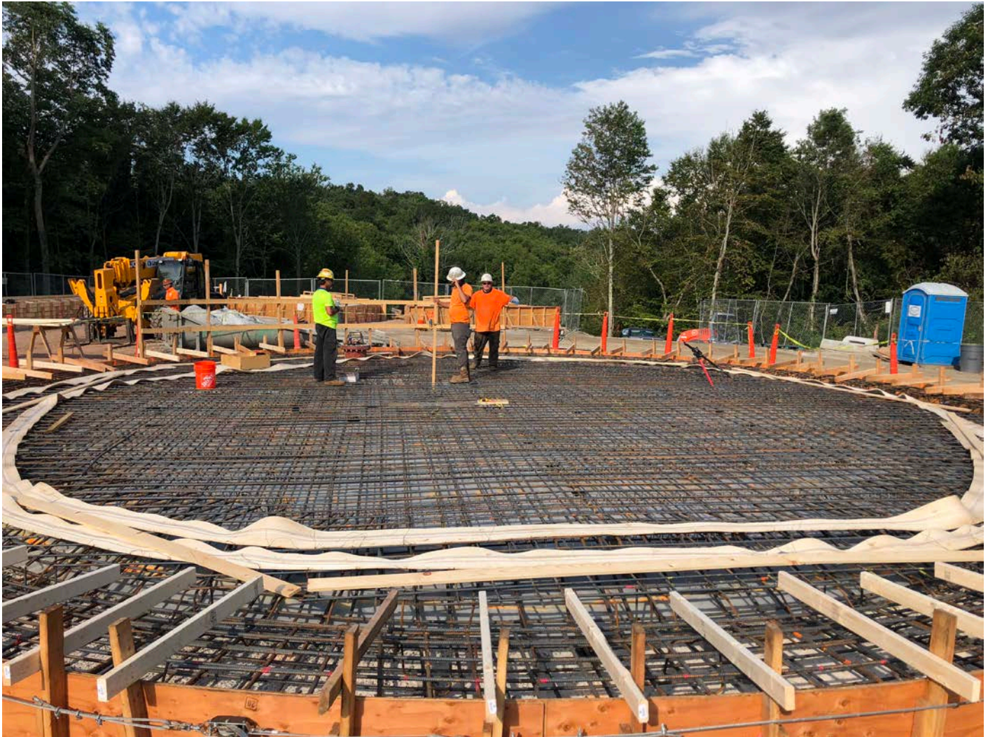
Picture 4: Ludlow preparing the water tank footprint for the pouring of concrete for the water tank base tomorrow morning. East of the Shared Access Driveway, Middletown. View to the west.
