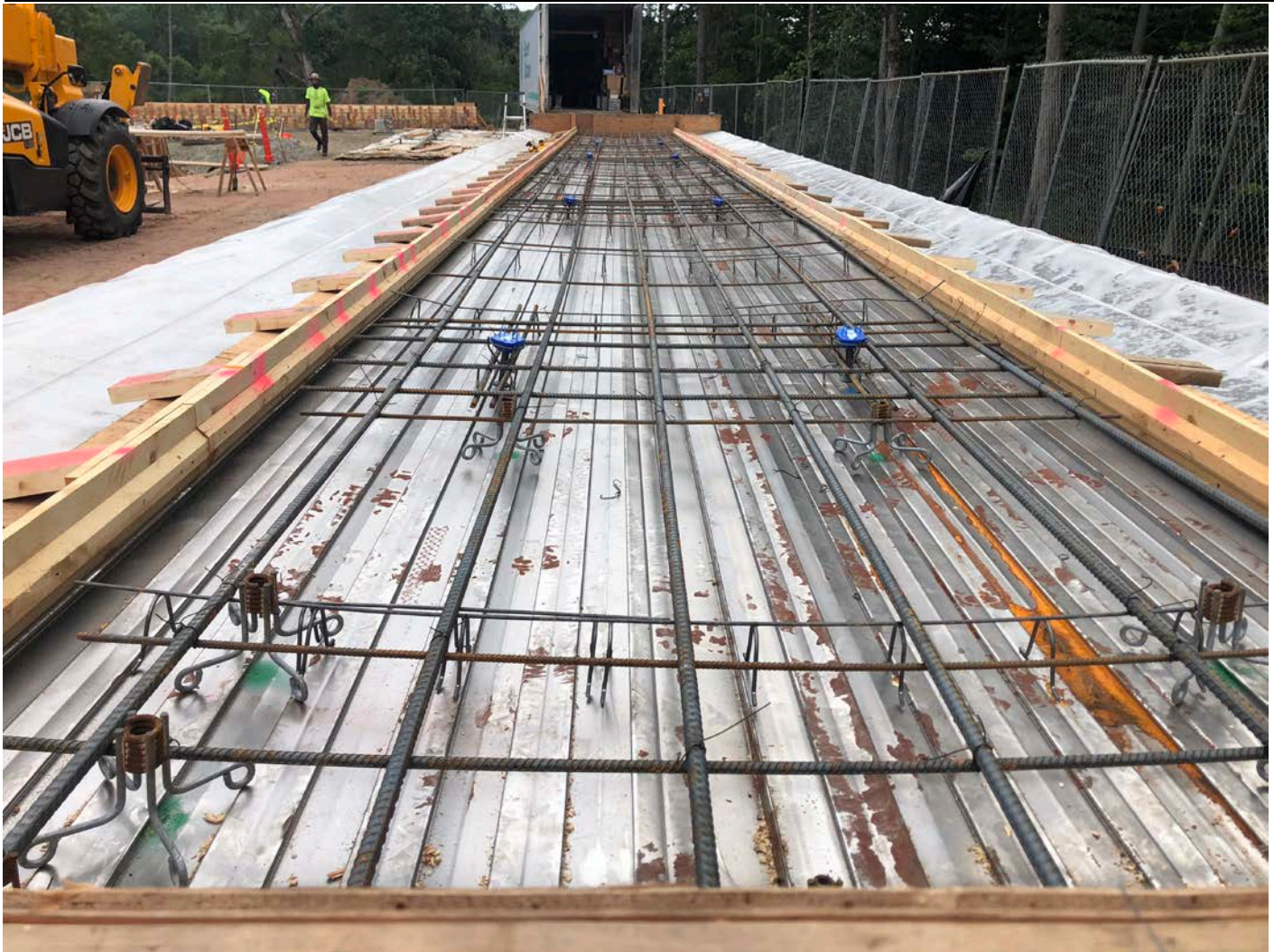
Picture 5: Rebar placed by Northeastern Steel on the concrete form for the narrow side panels of water tank. East of the Shared Access Driveway, Middletown. View to the east.
