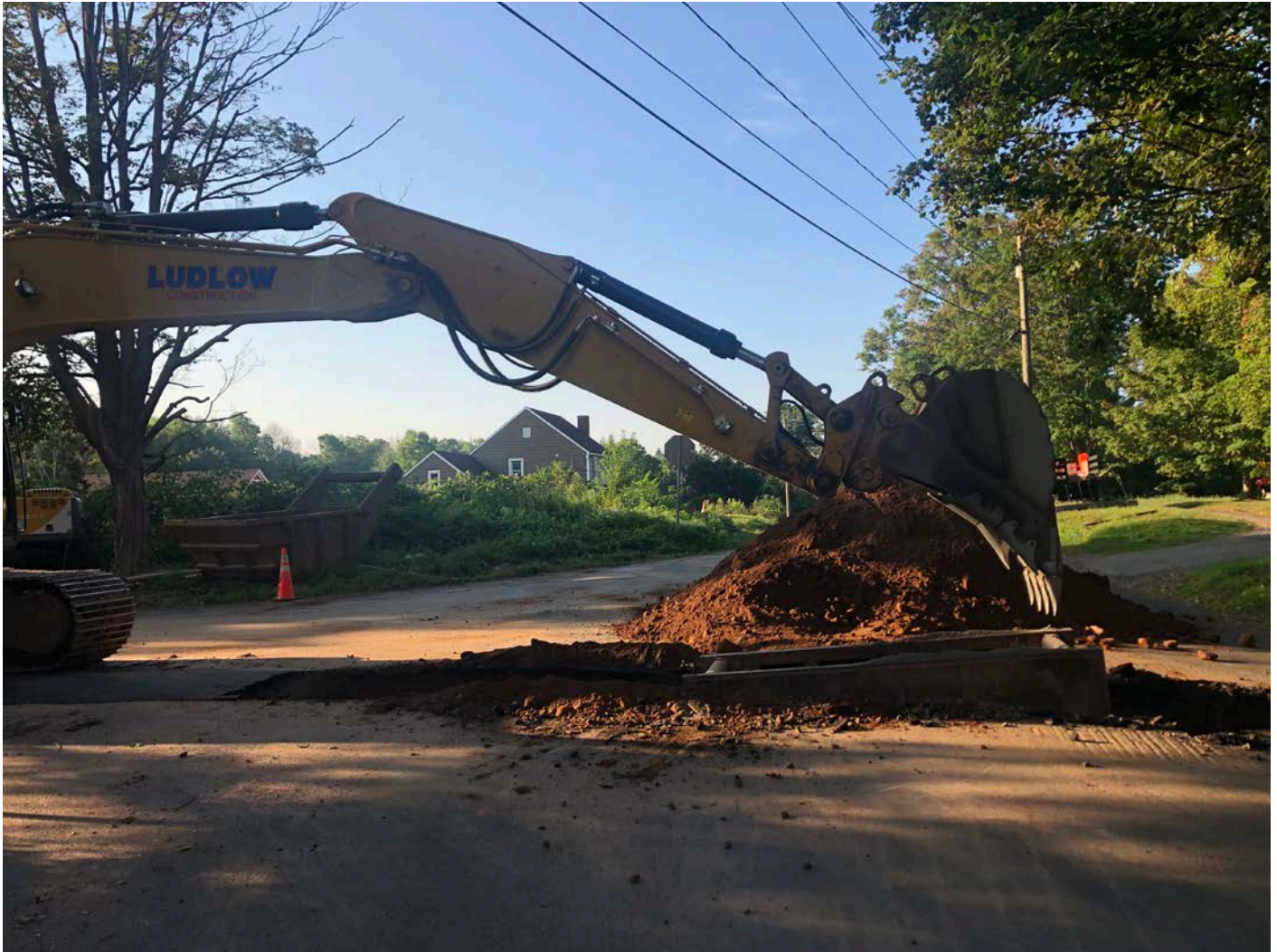
Picture 2: Ludlow excavating at the intersection of Talcott Lane and Maple Avenue, Durham for the installation of three 8" gate valves and gate boxes at Station 940+52. View to the south.
