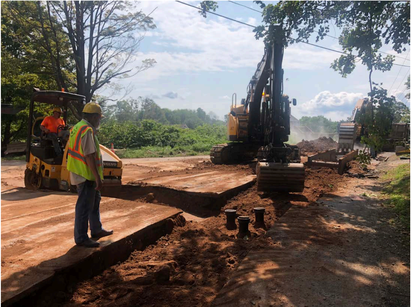
Picture 6: View of placement of 8" DIP on Maple Avenue, Durham at Station 940+52. View to the south.
