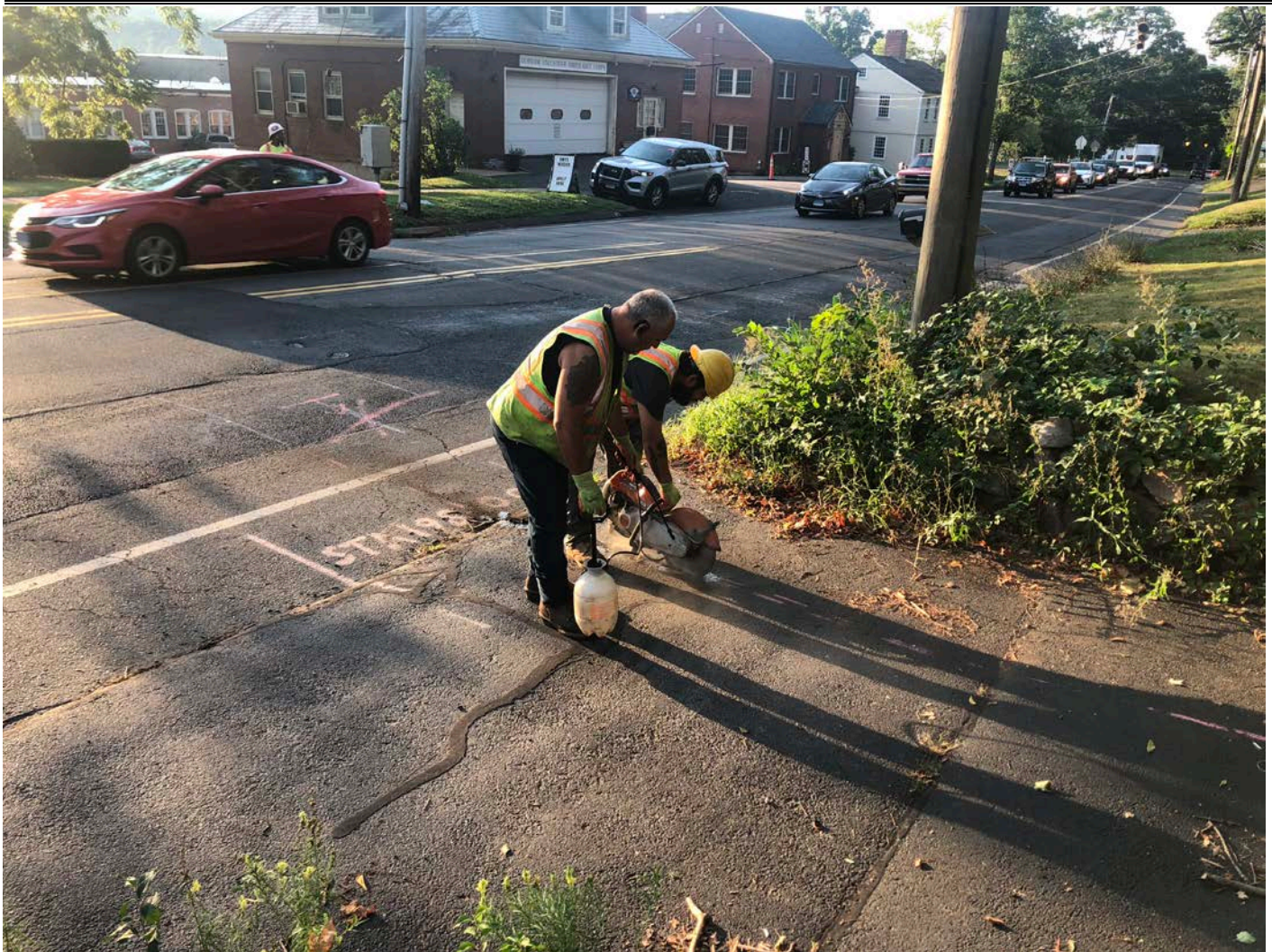
Picture 1: Ludlow saw cutting pavement at 208 Main Street, Durham, for the installation of a curb stop. Station 197+95. View to the southeast.
