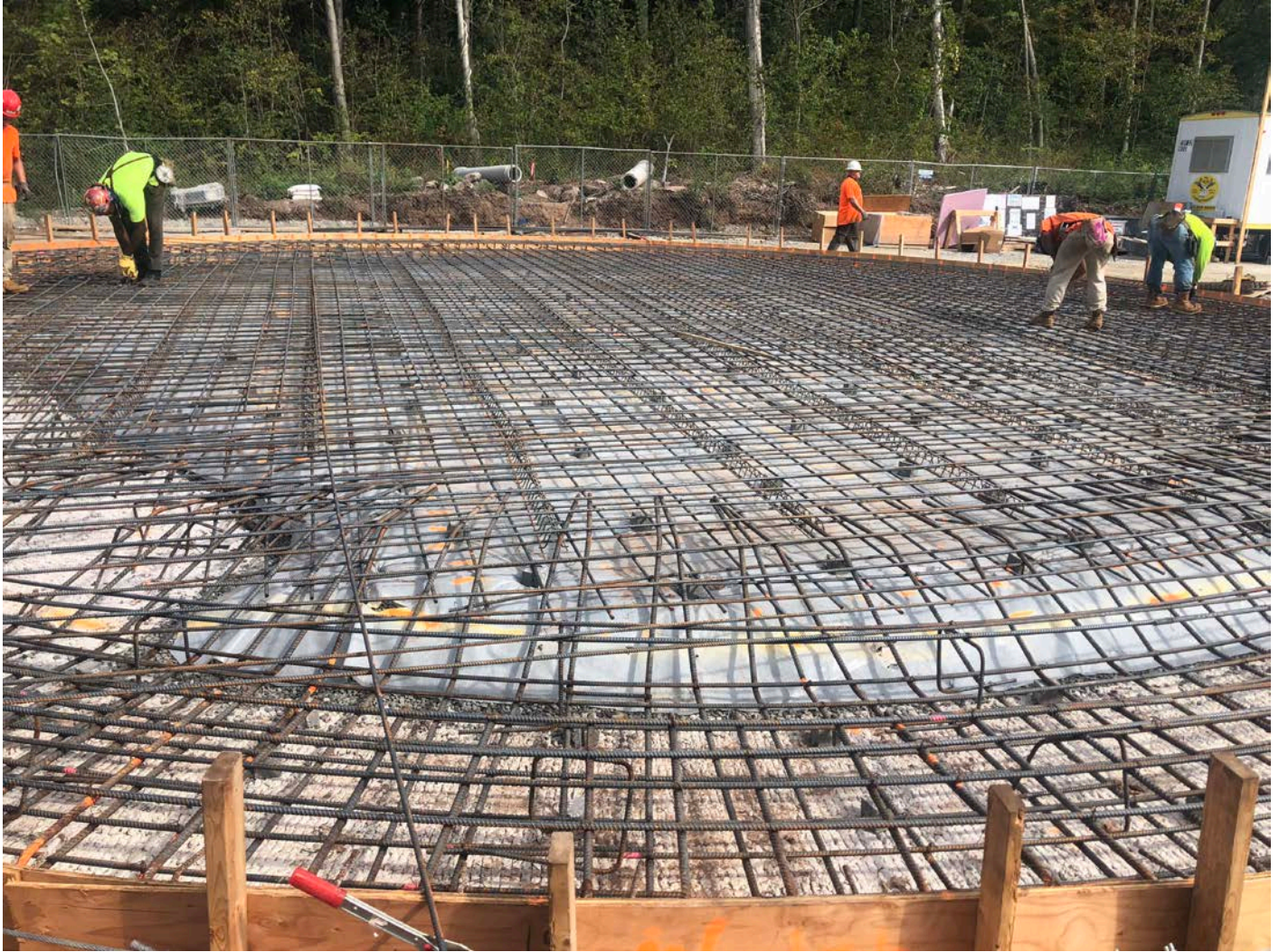
Picture 5: Rebar placement by Northeastern Steel at the water tank pad located to the east of the Shared Access Driveway, Middletown. View to the south.
