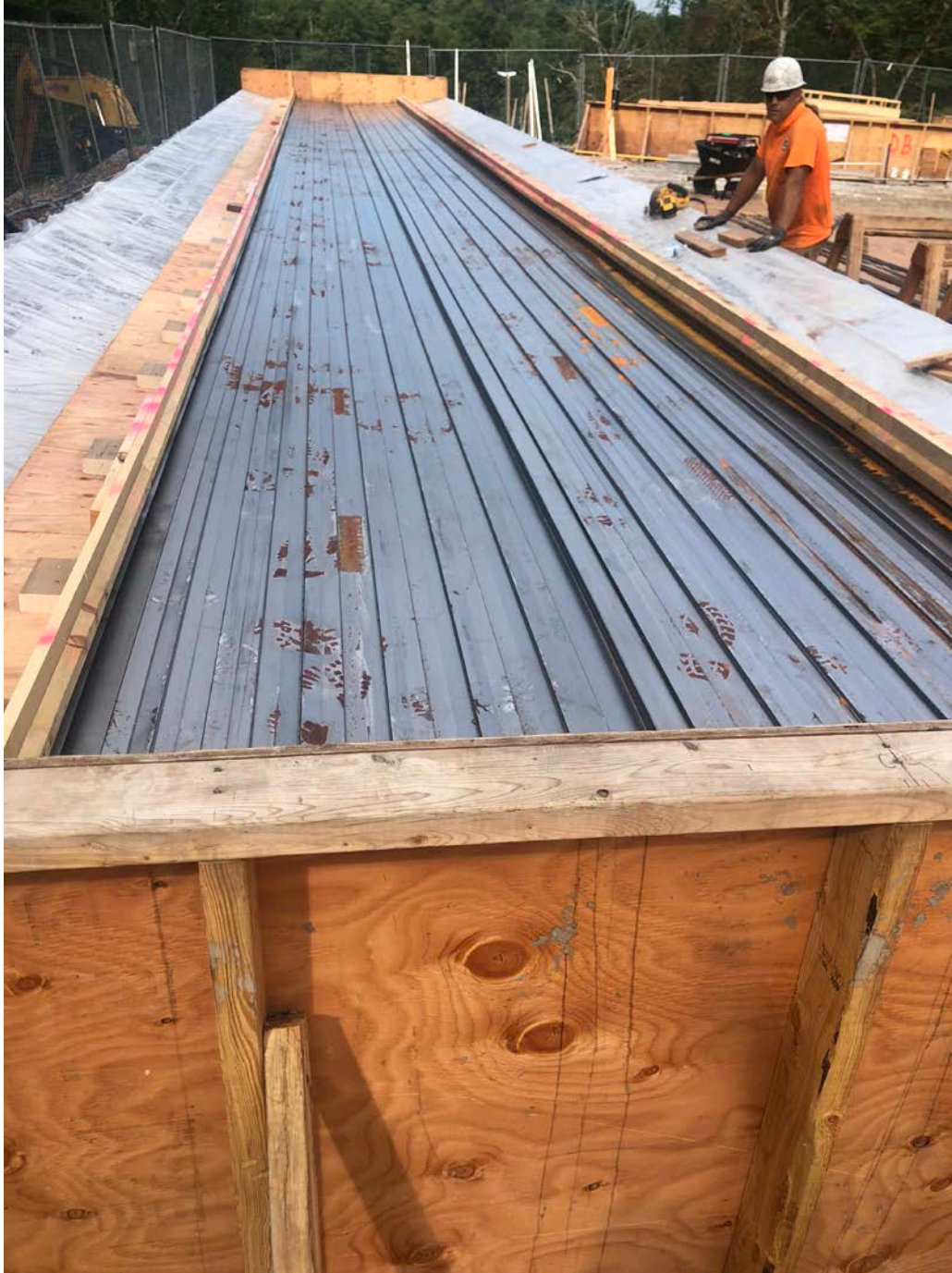
Picture 7: DN Tanks building a more narrow concrete form for two water tank side panels at the water tank pad located to the east of the Shared Access Driveway, Middletown. View to the west.
