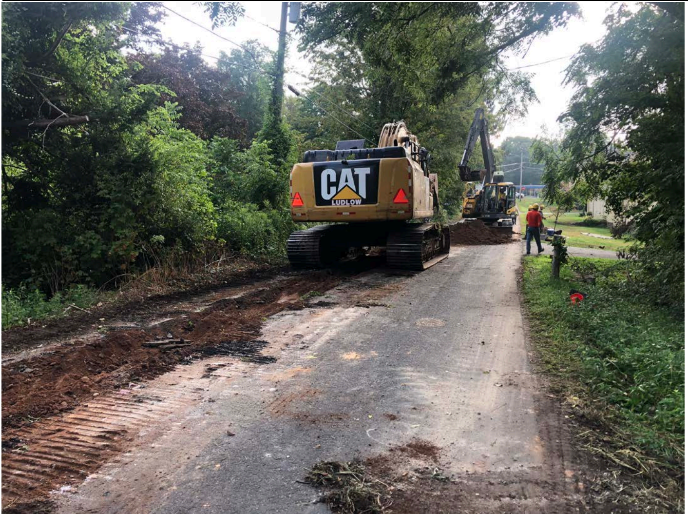
Picture 1: Ludlow installing 8" DIP on Talcott Lane, Durham, starting at Station 302+94. View to the west.
