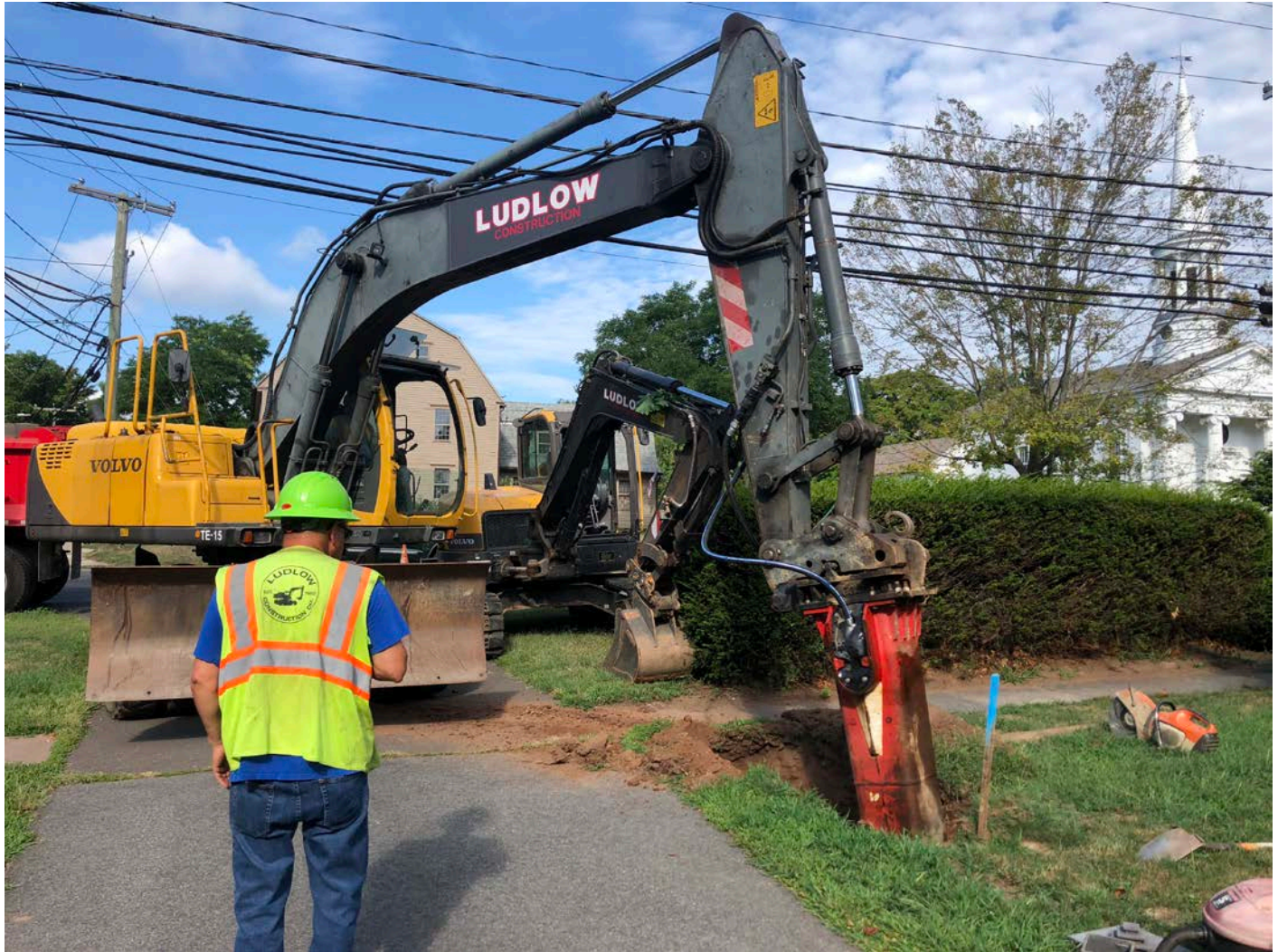
Picture 4: Ludlow hammering rock at Station 194+78 (227 Main Street, Durham) during the installation of a curb stop. View to the northeast.
