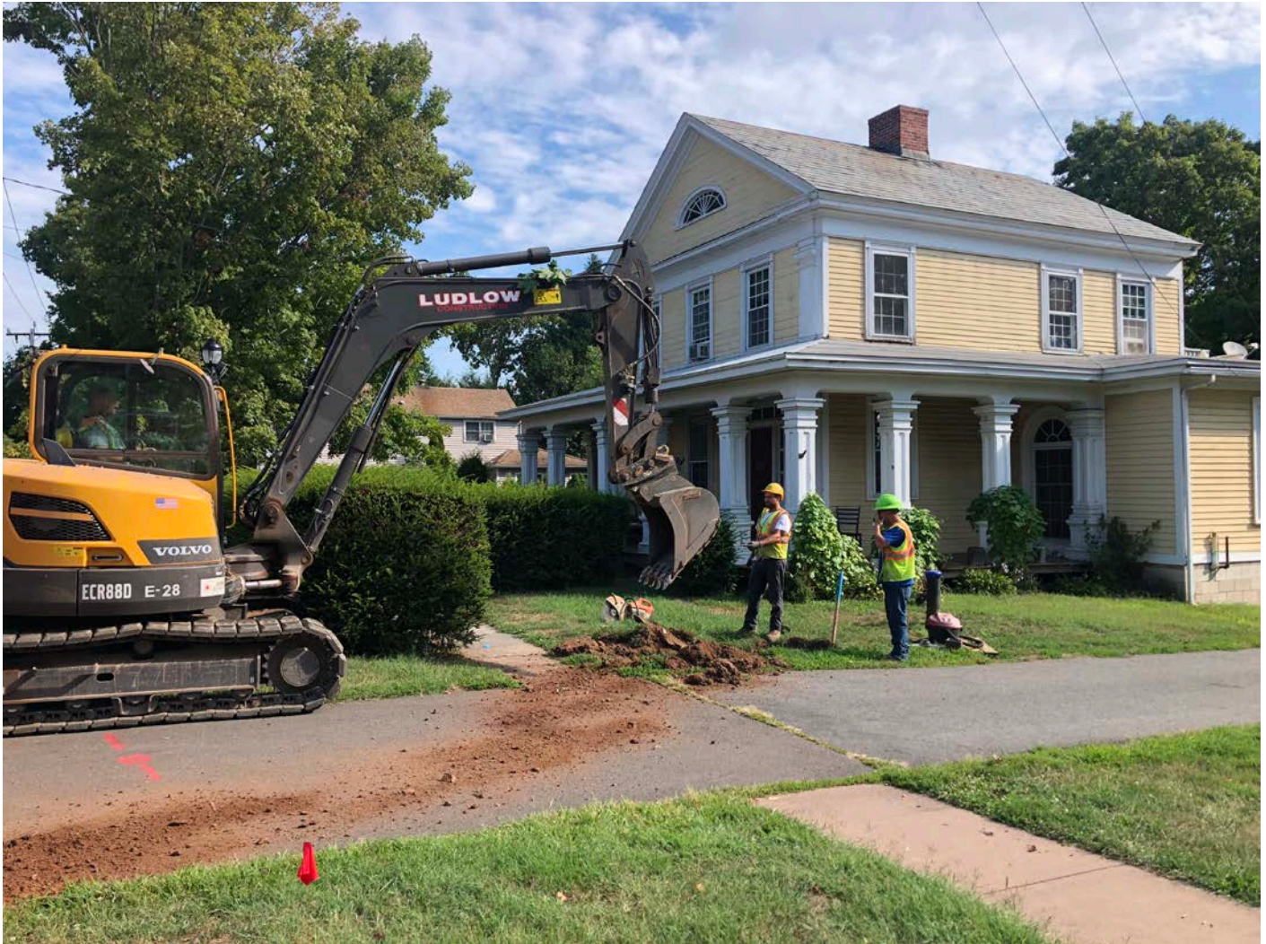
Picture 3: Ludlow trenching at Station 194+78 (227 Main Street, Durham) for the installation of a curb stop. View to the south.
