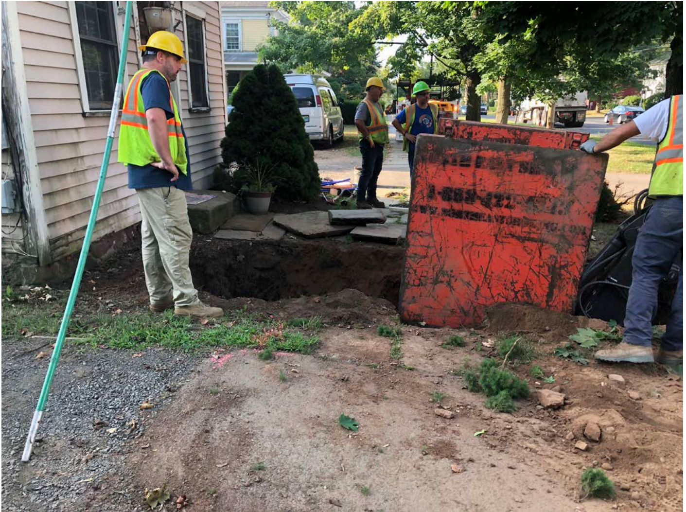
Picture 2: Ludlow trenching at Station 193+31 (233 Main Street, Durham) for the installation of a curb stop. View to the south.
