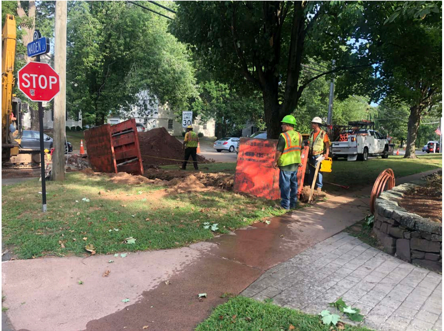
Picture 5: Ludlow placing curb stop at Station 191+30 (243 Main Street), Durham. View to the northwest.
