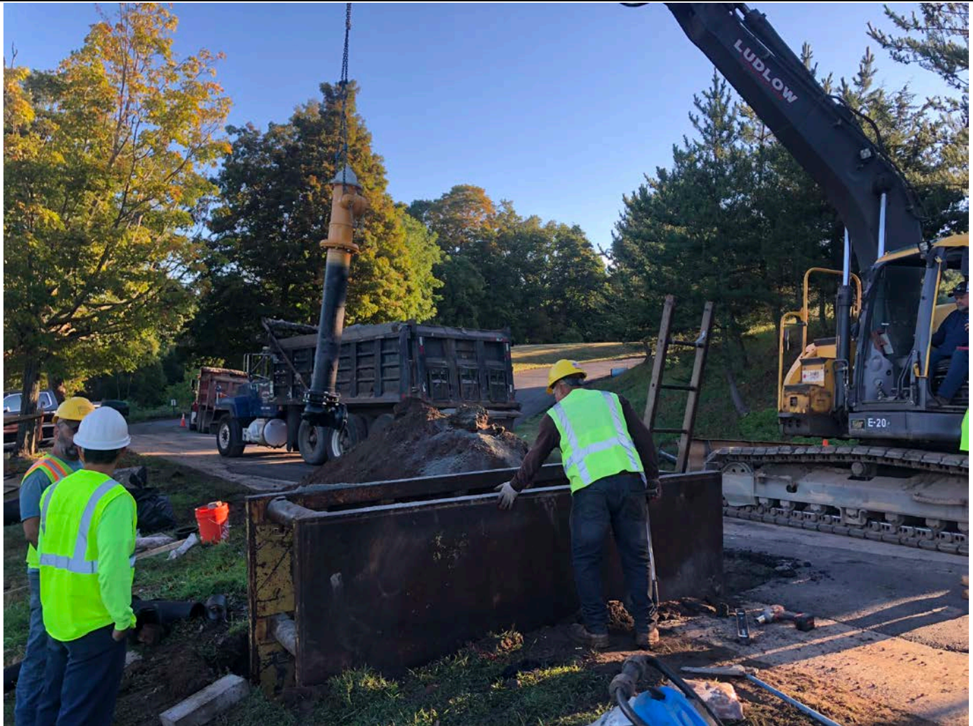
Picture 1: Ludlow installing a hydrant at Station 900+87.5. Maple Avenue, Durham. View to the north.
