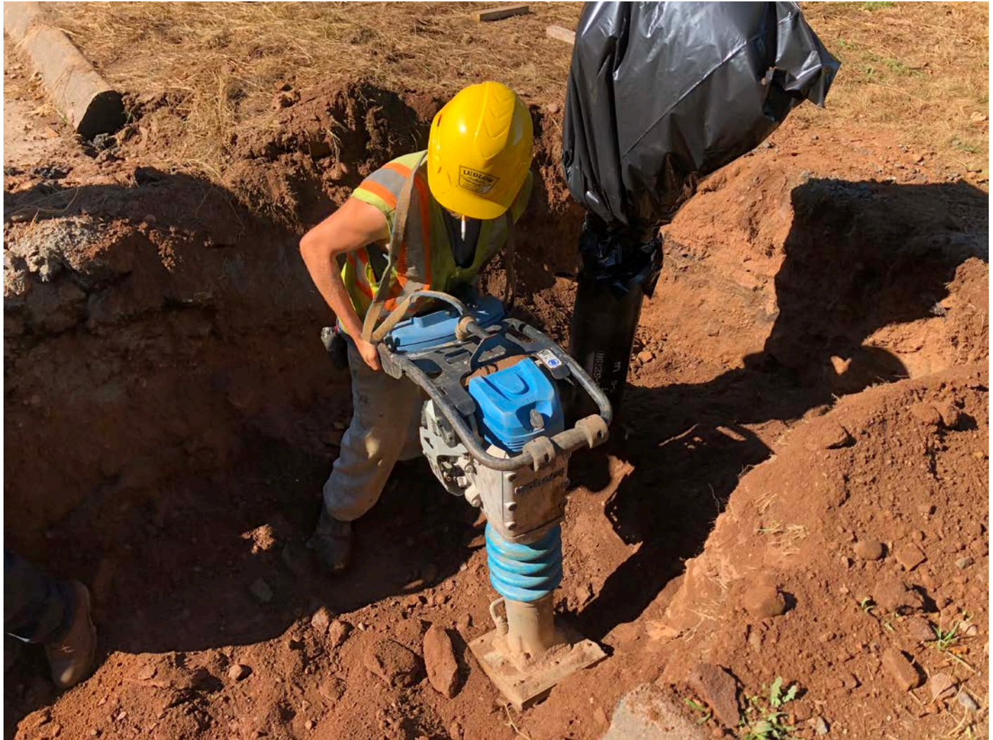
Picture 6: Ludlow compacting soil around a hydrant that they are in the process of installing at Station 906+90. Maple Avenue, Durham.
