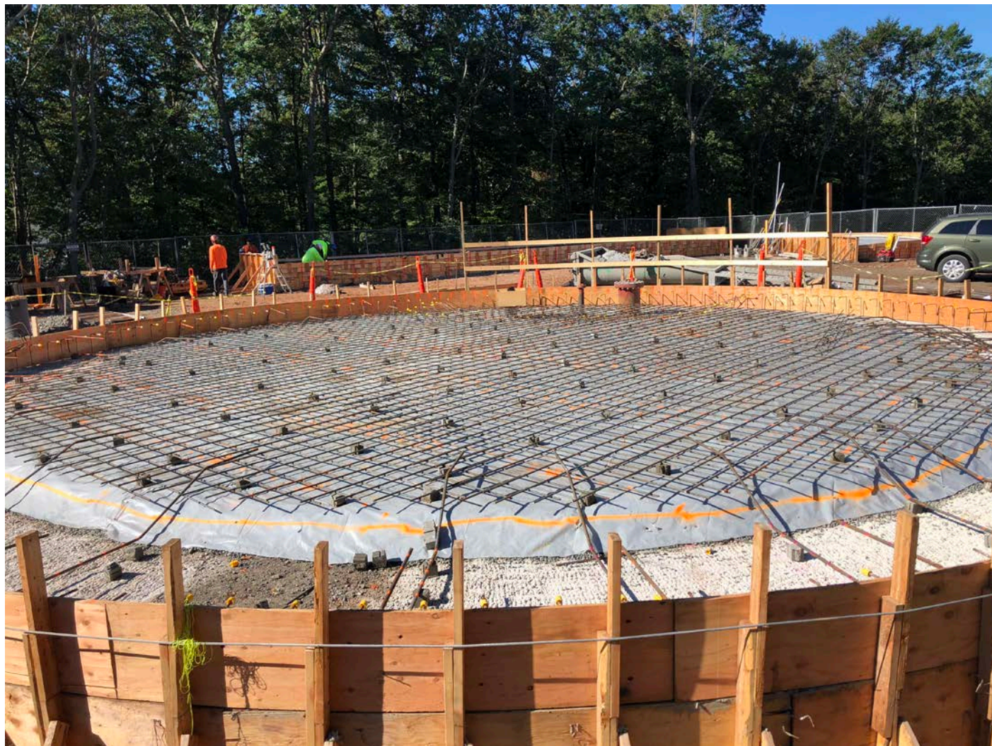
Picture 5: The footprint of the water tank with additional rebar placed since yesterday. Water tank work zone, east of the Shared Access Driveway, Middletown. View to the south.
