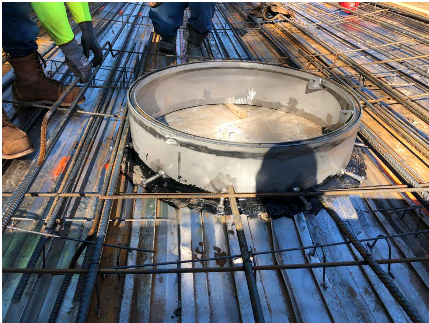
Picture 4: Rebar placed and fastened on one of the side panel concrete forms, with a 37" diameter manway also secured onto the form. Water tank work zone, east of the Shared Access Driveway, Middletown. View to the west.
