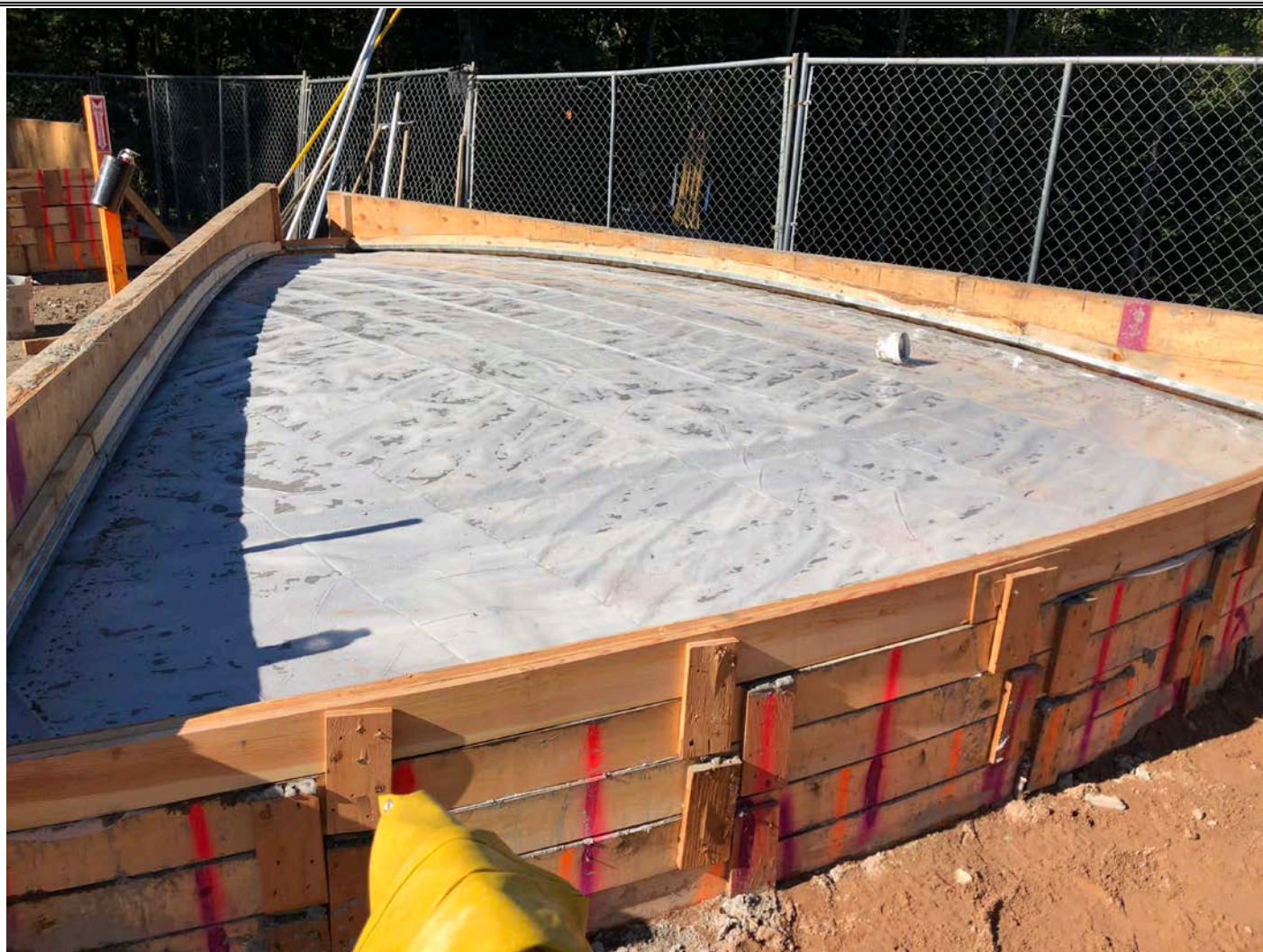
Picture 3: One of the two concrete forms for the water tank's top, where poly sheeting was placed over setting concrete. Water tank work zone, east of the Shared Access Driveway, Middletown.
