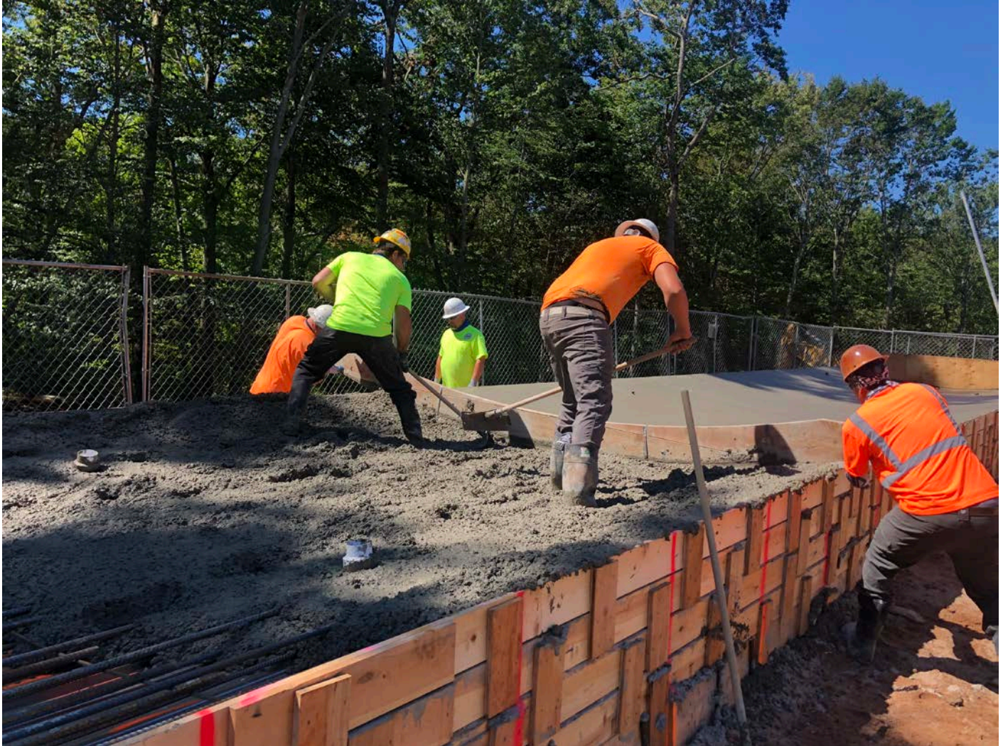
Picture 7: DN Tanks placing 4000 PSI concrete on the first of two concrete forms for the side panels of the water tank. East of the Shared Access Driveway, Middletown. View to the west.
