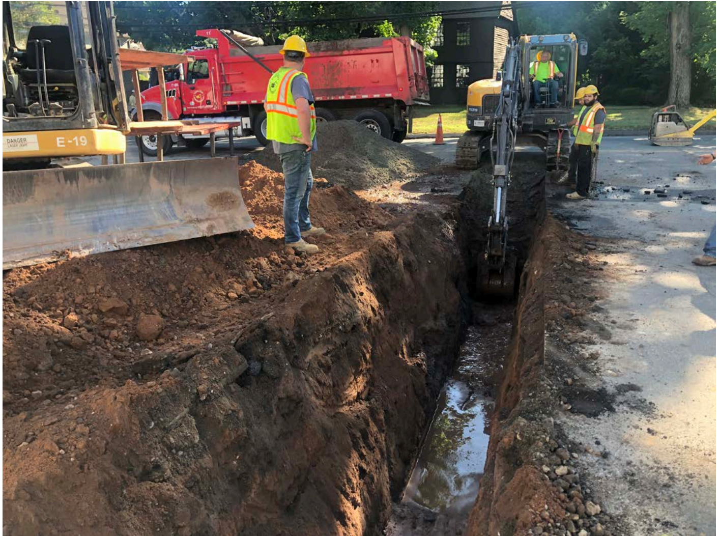
Picture 2: Ludlow trenching at Station 193+18 (238 Main Street, Durham) for the installation of a curb stop. View to the east.
