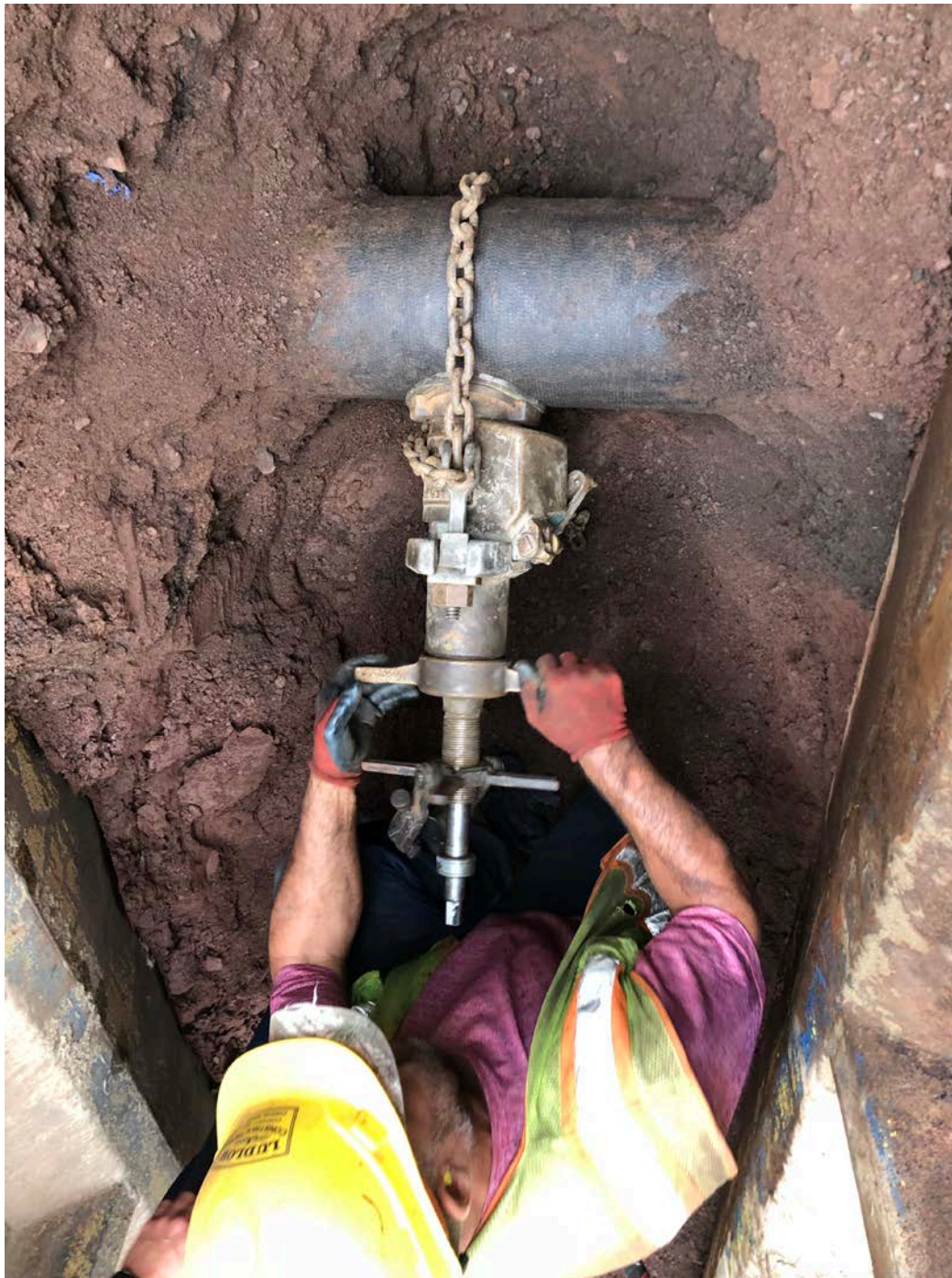
Picture 7: Ludlow tapping existing 8" water line at 13 Maple Avenue, Durham in order to install a corporation stop.
