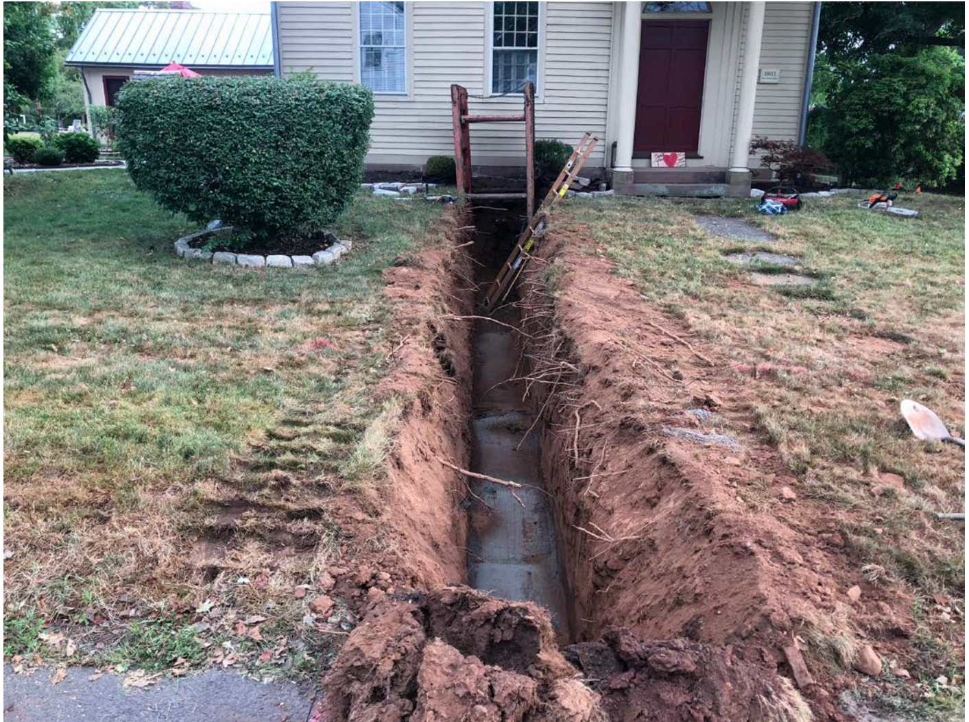
Picture 6: Trench that Ludlow has excavated for the installation of a curb stop and 1" copper service line at the residence at 13 Maple Avenue, Durham. View to the north.
