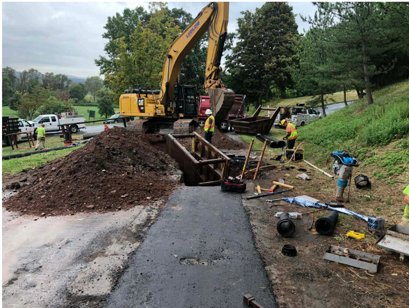
Picture 9: Ludlow connecting to the existing 8" DIP water line to the 12" DIP that they previously installed south of the Maple Avenue stream crossing. View to the north.
