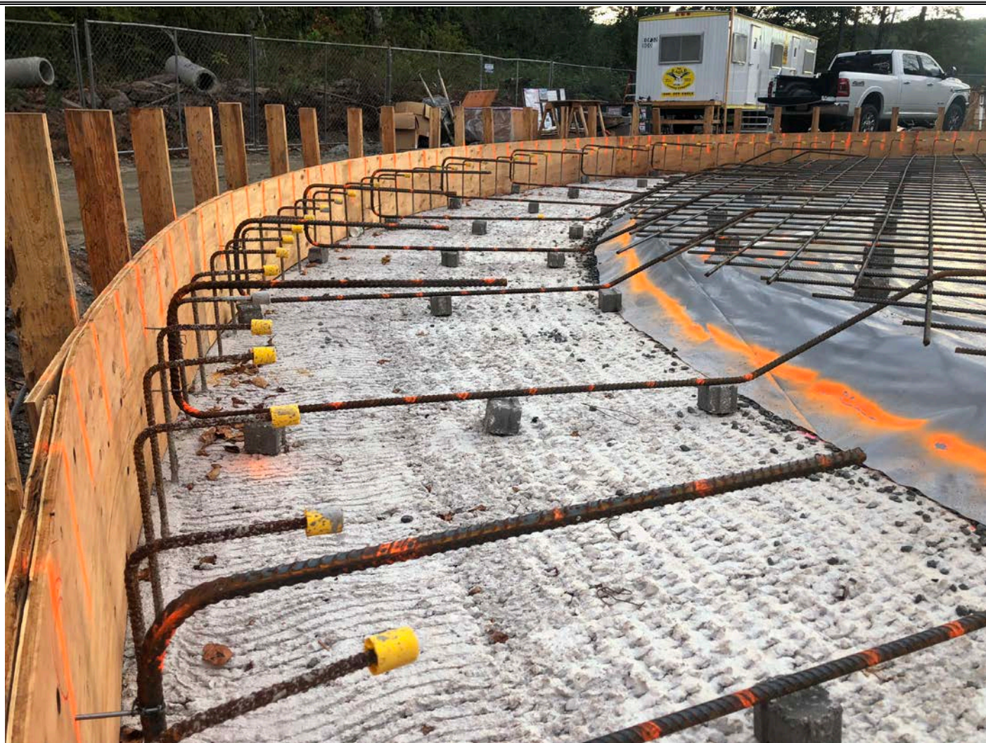
Picture 1: Rebar placed on frost wall of the water tank footprint by Northeastern Steel. Water tank work zone, east of the Shared Access Driveway, Middletown. View to the west.
