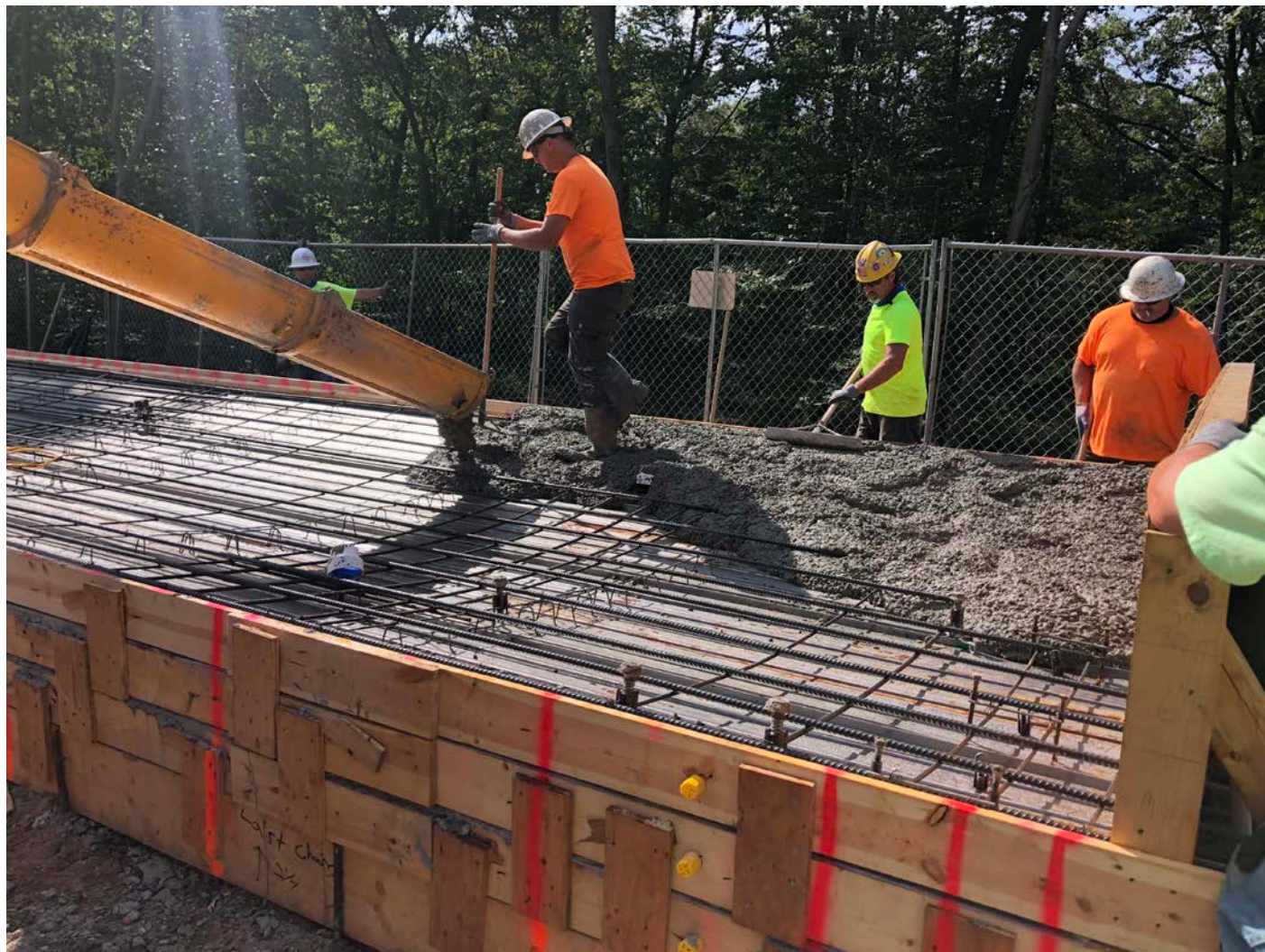
Picture 2: DN Tanks placing 4000 PSI concrete on the first of two concrete forms for the side panels of the water tank. East of the Shared Access Driveway, Middletown. View to the south.
