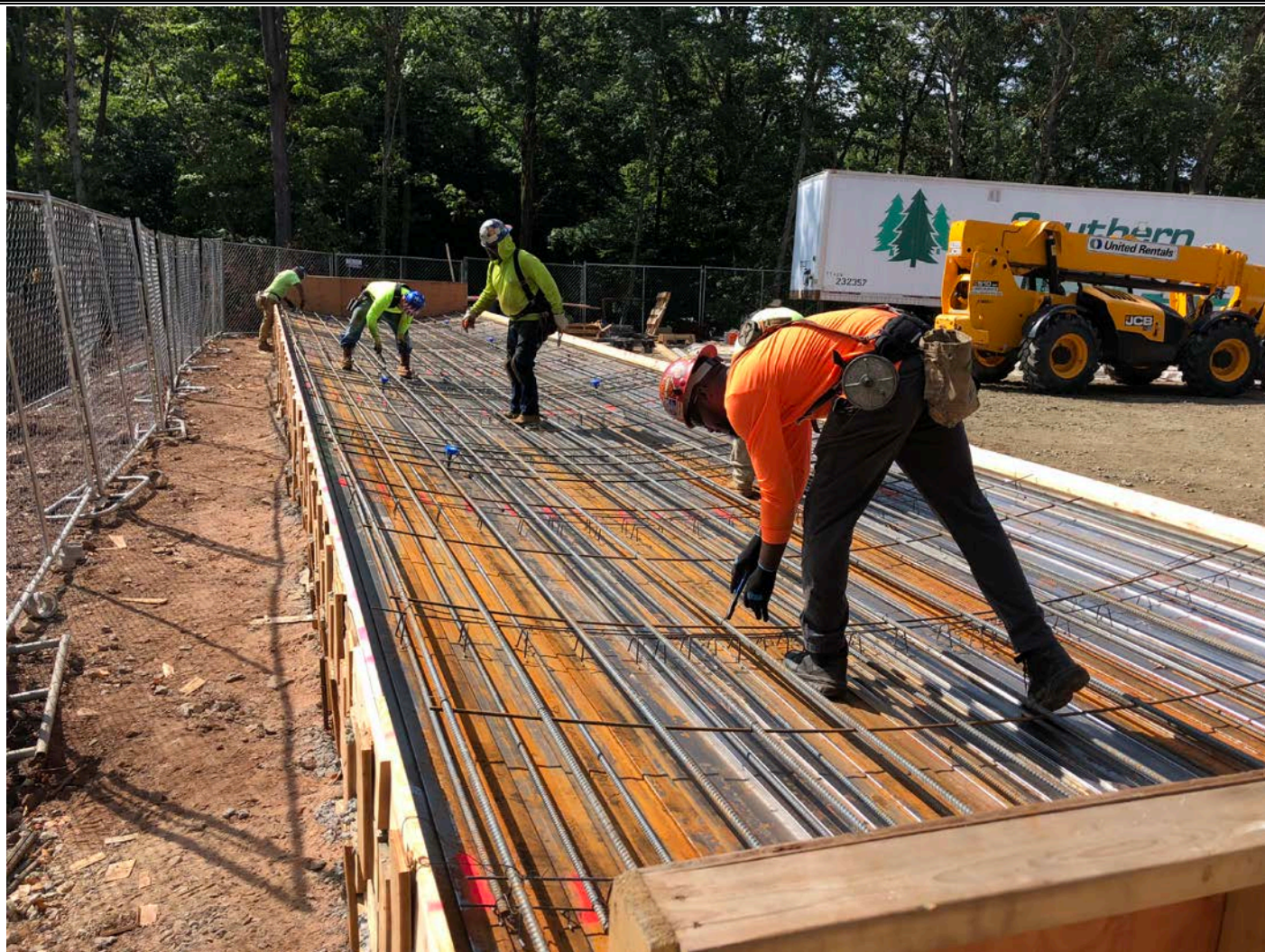
Picture 3: Northeastern Steel fastening rebar with wire ties on top of chairs on one of the two water tank side panel concrete forms. Water tank work zone, east of the Shared Access Driveway, Middletown.
