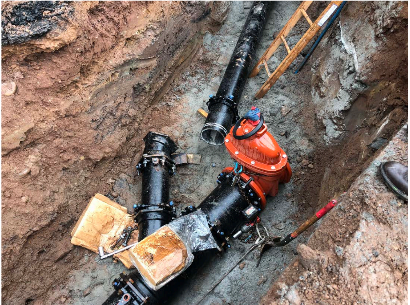
Picture 10: Ludlow preparing to connect 8" DIP to WYE fitting coming off of the 12" DIP on Maple Avenue, Durham.
