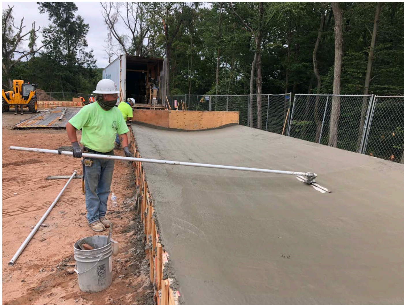
Picture 4: DN Tanks finishing the surface of concrete placed on one of the two water tank side panel concrete forms. Water tank work zone, east of the Shared Access Driveway, Middletown. View to the east.
