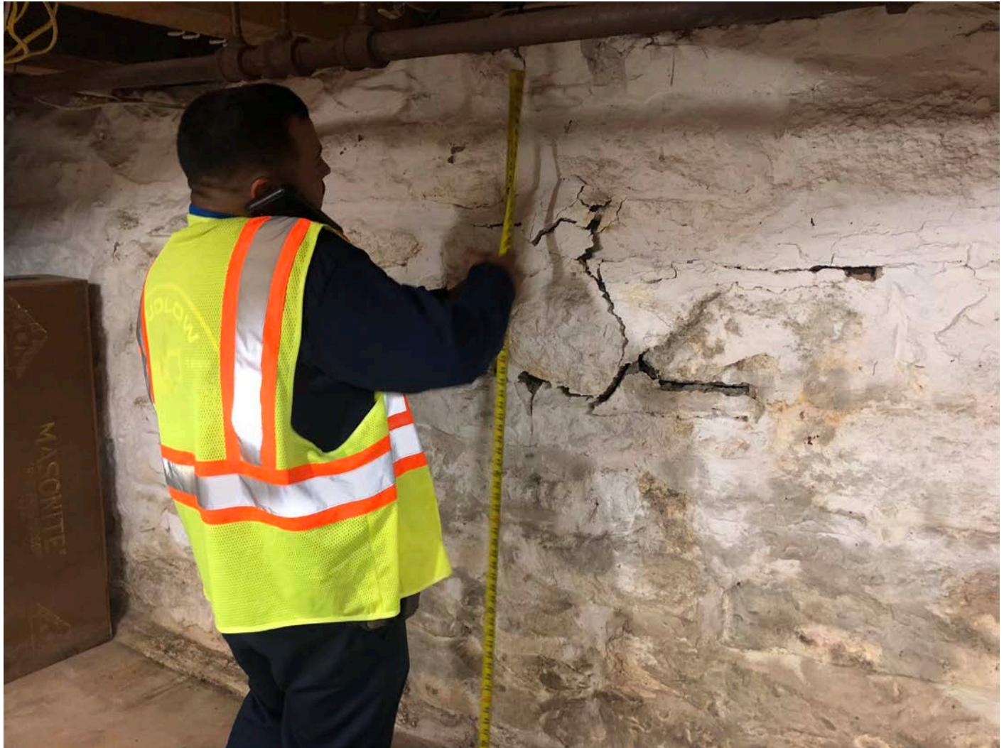
Picture 5: Ludlow preparing to penetrate the basement wall of the residence at 13 Maple Avenue, Durham in order to bring a 1" copper service line into the house.
