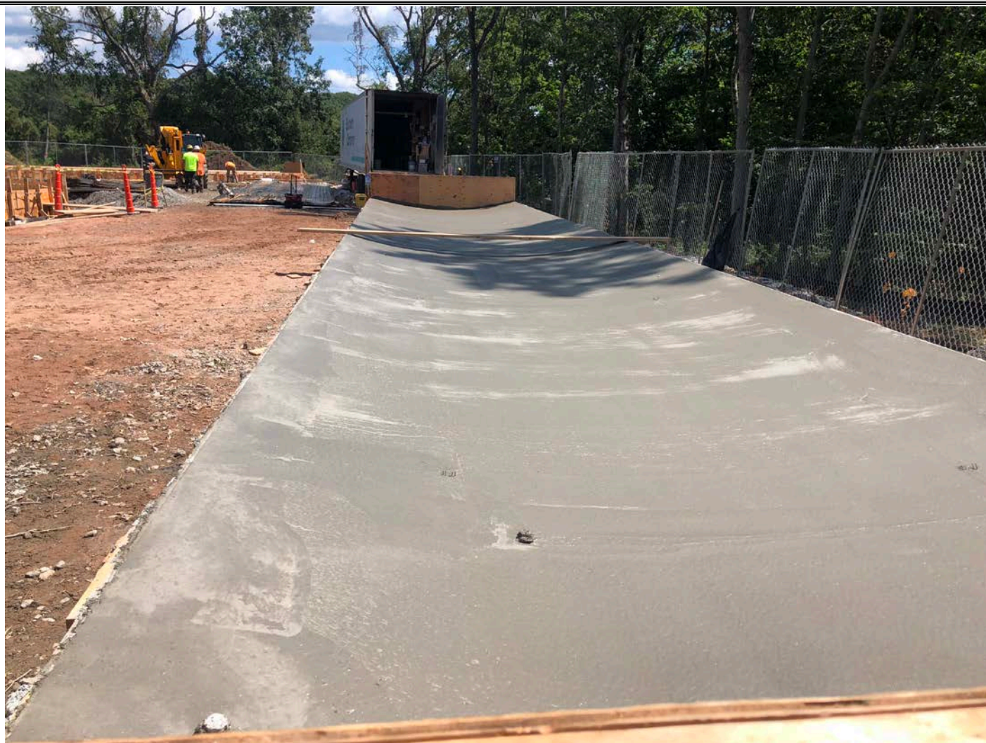
Picture 7: The first of two concrete forms with 4000 PSI concrete curing after being placed today. Water tank work zone, east of the Shared Access Road, Middletown. View to the east.
