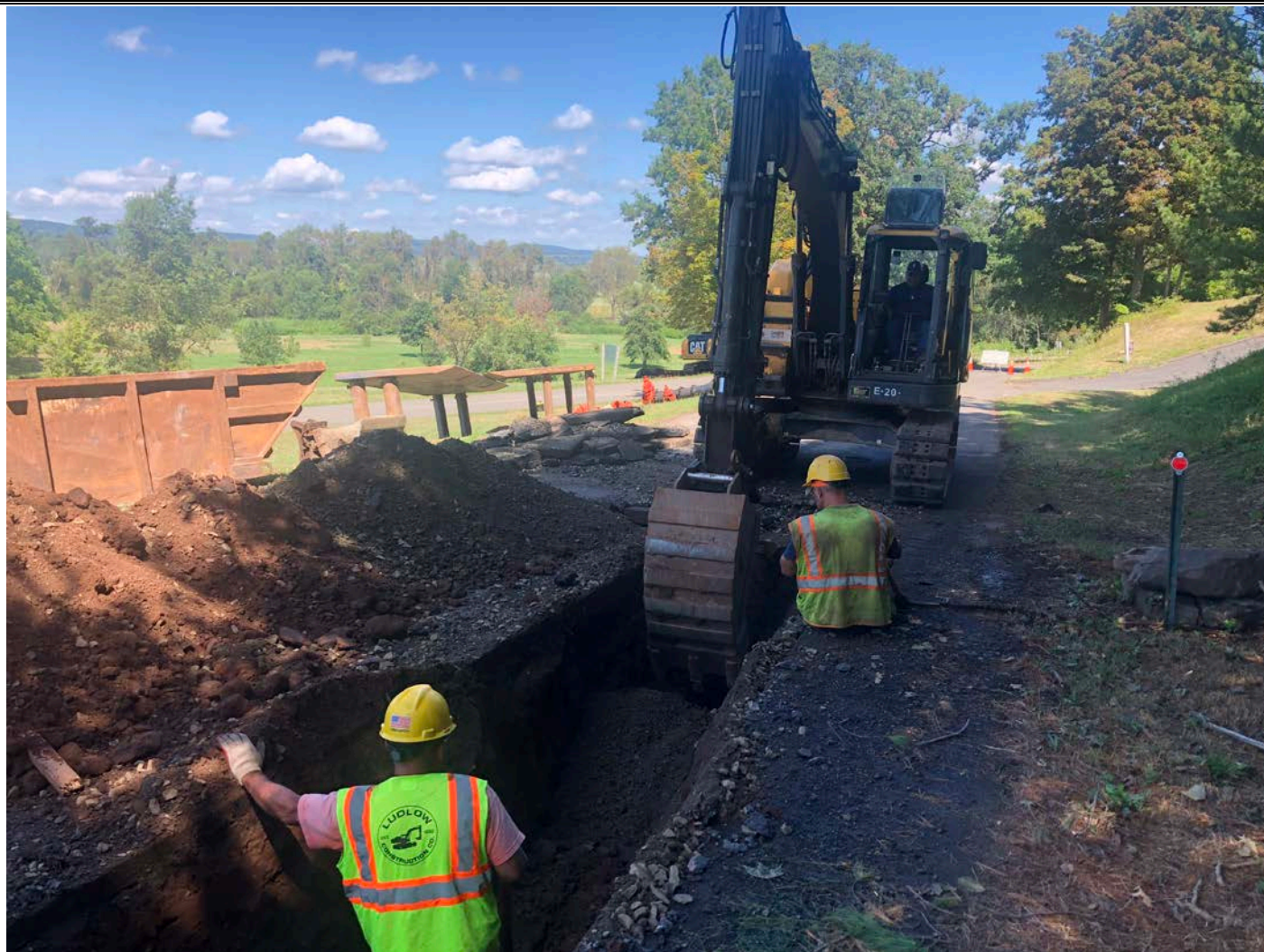
Picture 8: Ludlow excavating on Maple Avenue (just south of Station 900+00) to daylight the northern end of the line in order to assess what they will need for hardware in order to connect the existing line to the 12" DIP they will soon install south of Station 900+00 on Maple Avenue. View to the north.
