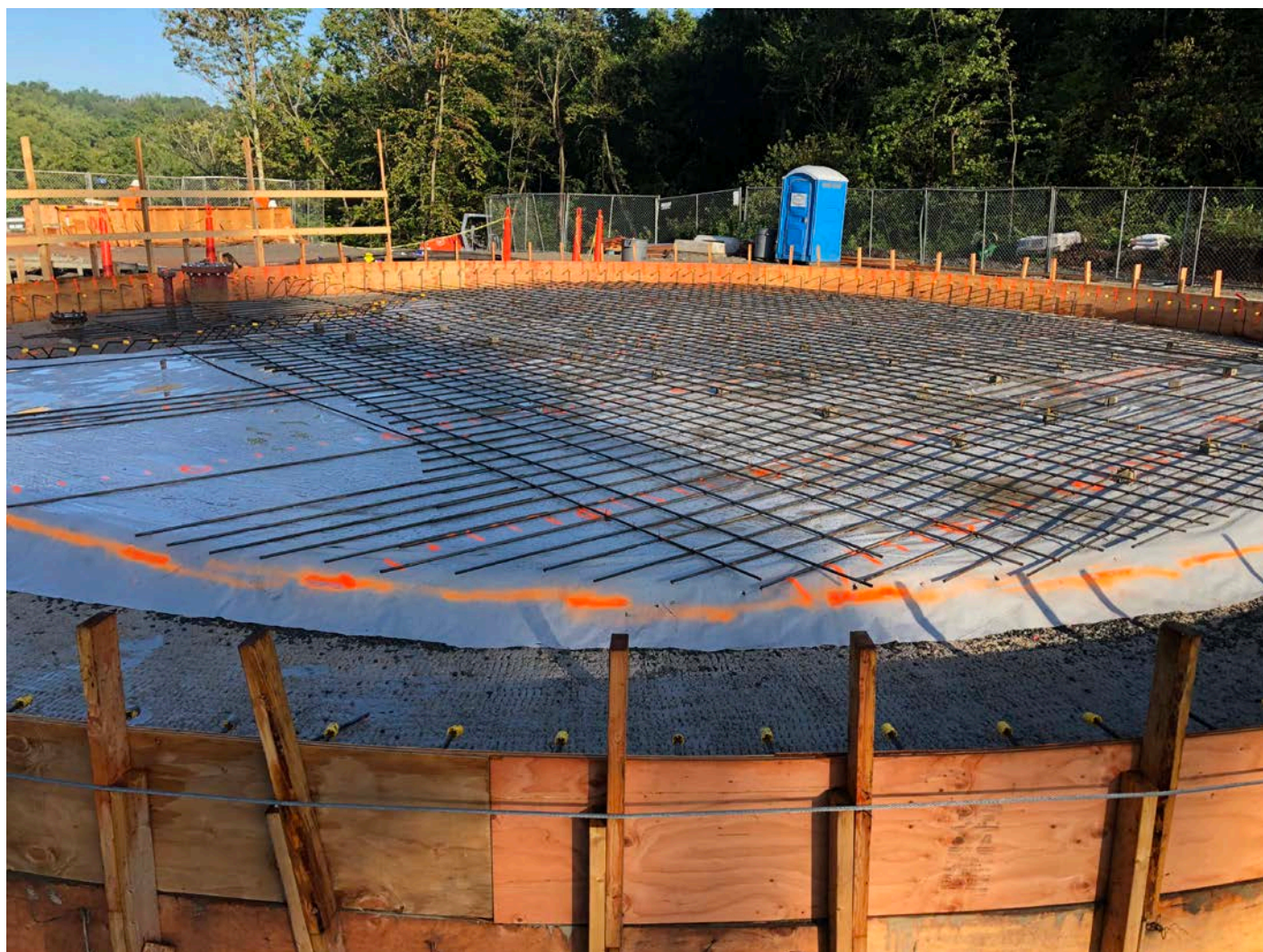
Picture 1: Rebar placed on water tank footprint by Northeastern Street. Water tank work zone, east of the Shared Access Driveway, Middletown. View to the northwest.
