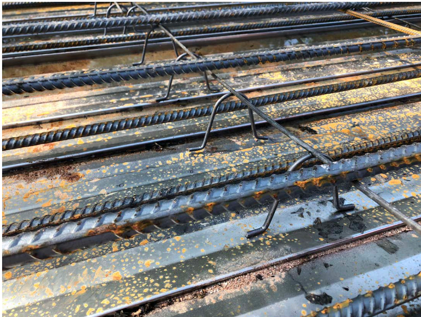
Picture 2: Rebar placed on top of chairs on one of the two water tank side panel concrete forms. Water tank work zone, east of the Shared Access Driveway, Middletown.
