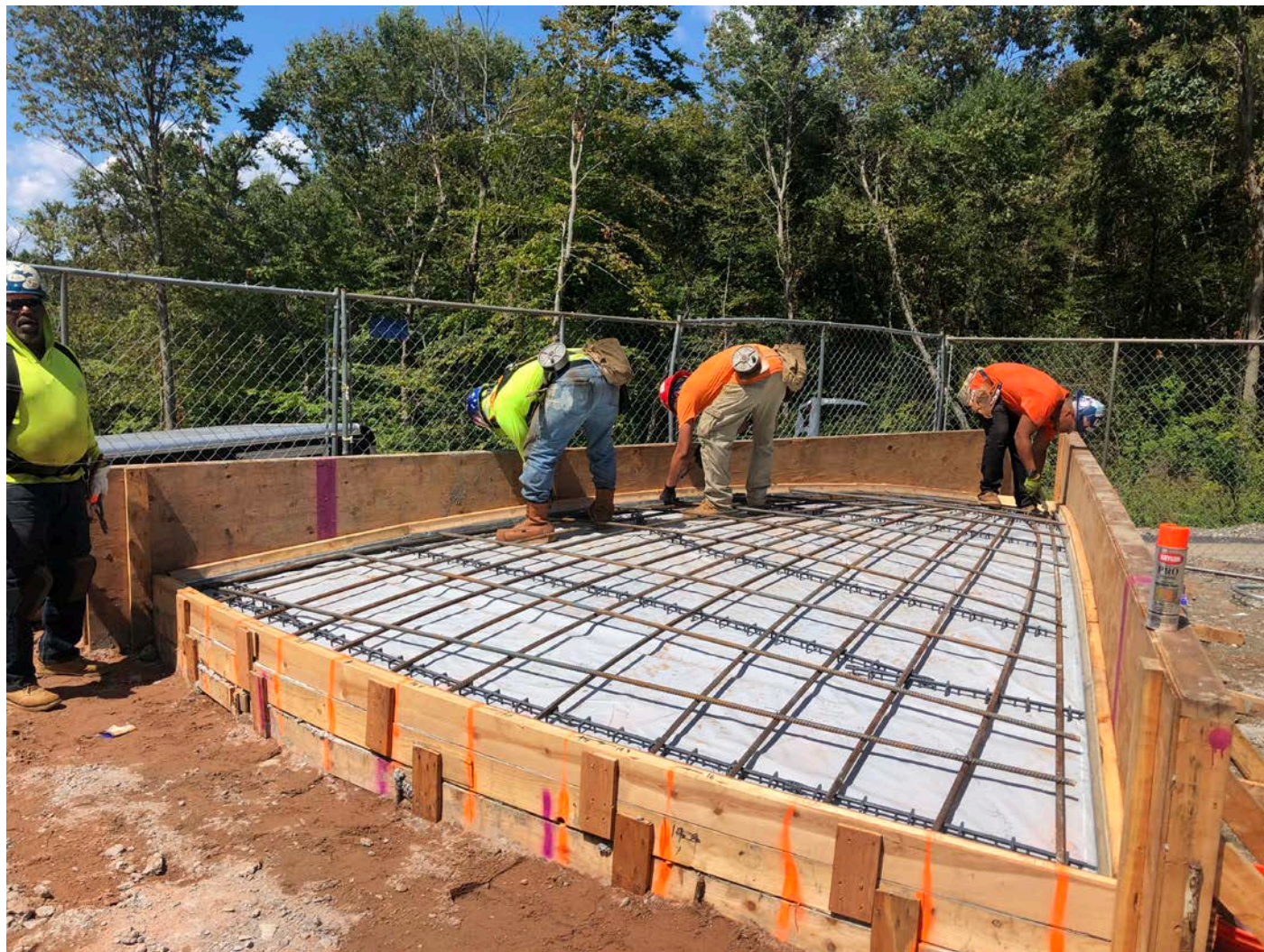
Picture 5: Northeastern Steel placing rebar on top of chairs on one of the two water dome panel concrete forms. Water tank work zone, east of the Shared Access Driveway, Middletown. View to the northwest.
