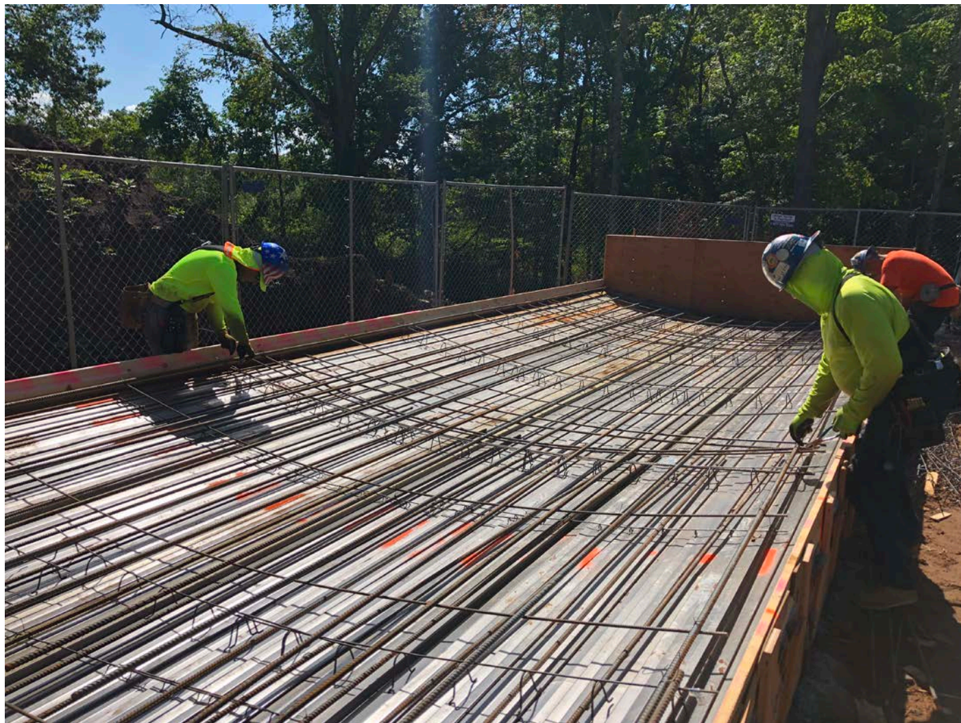
Picture 4: Northeastern Steel placing rebar on top of chairs on one of the two water tank side panel concrete forms. Water tank work zone, east of the Shared Access Driveway, Middletown. View to the west.
