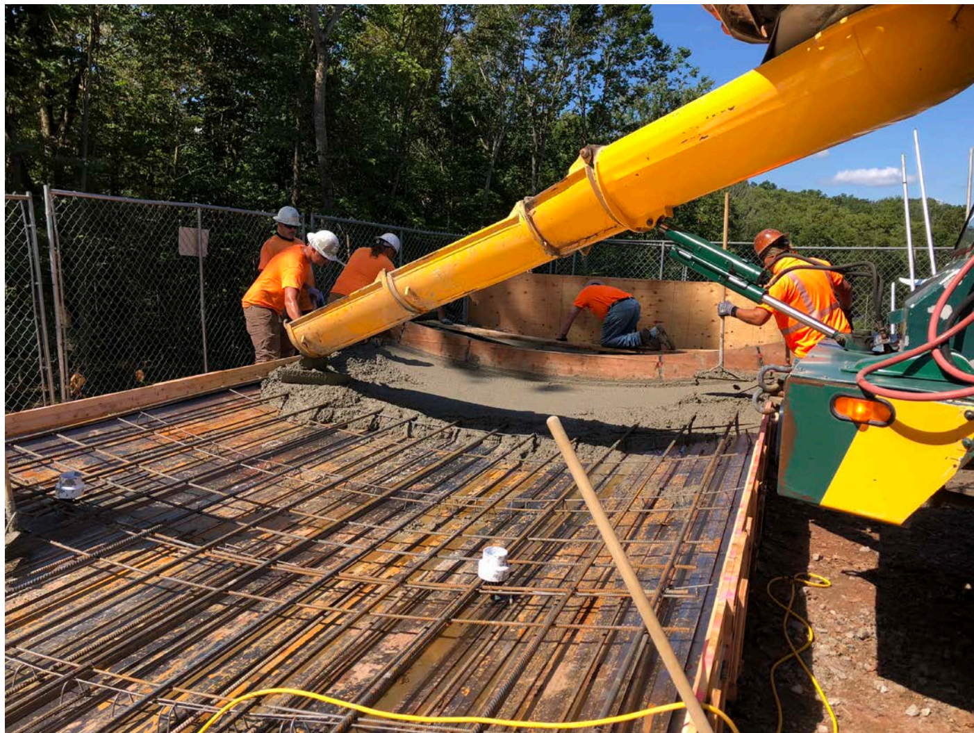
Picture 6: DN Tanks placing 4000 PSI concrete on the first of two concrete forms for the side panels of the water tank. East of the Shared Access Driveway, Middletown. View to the east.
