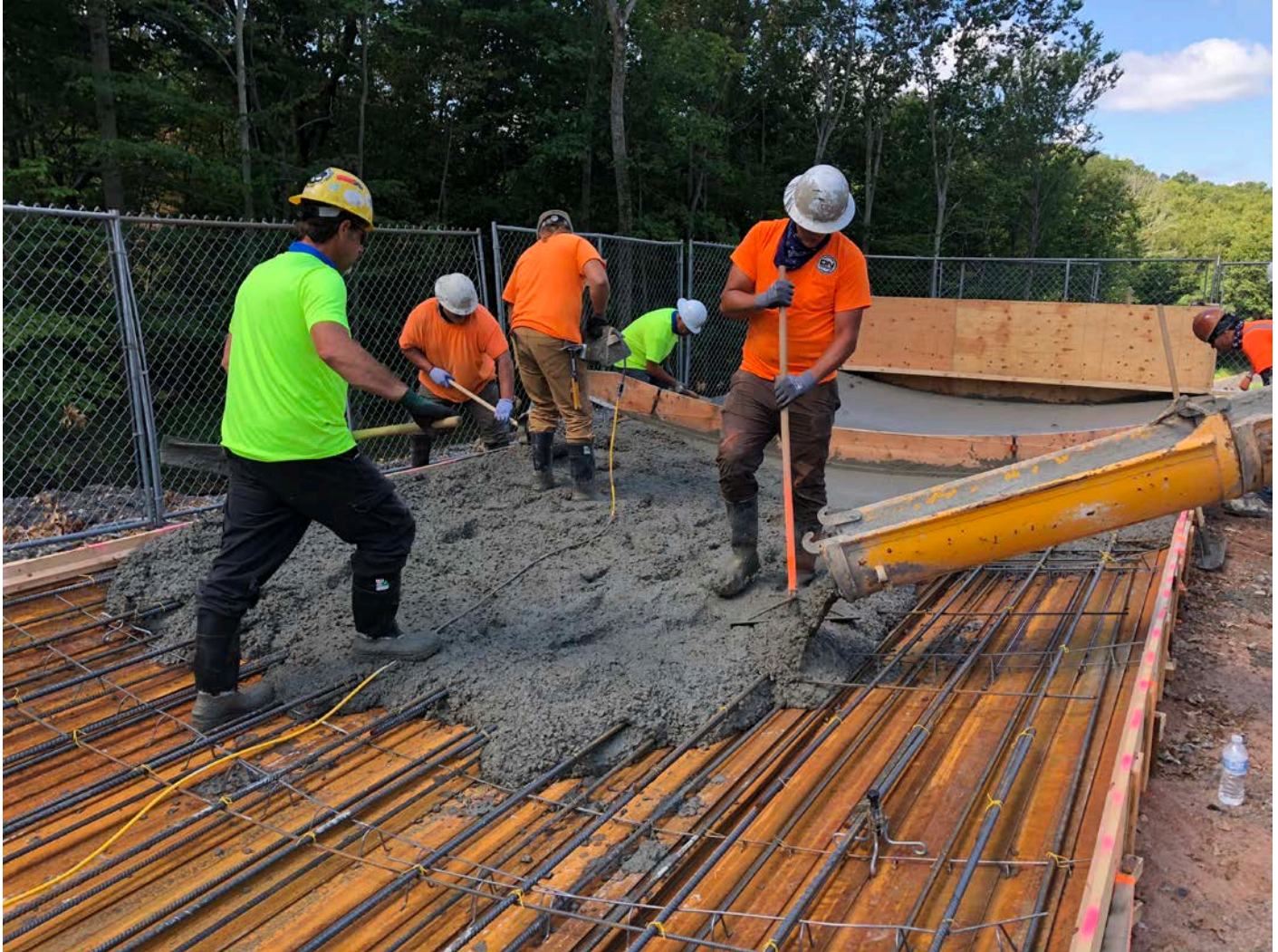
Picture 5: DN Tanks placing 4000 PSI concrete on the first of two water tank side panel concrete forms. Two DN Tank Laborers can be seen in the background leveling the concrete. East of the Shared Access Driveway, Middletown. View to the west.
