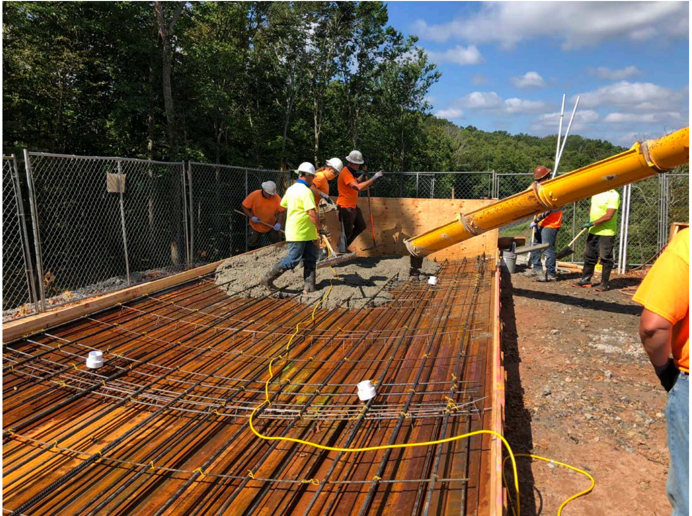
Picture 4: DN Tanks placing 4000 PSI concrete on the first of two water tank side panel concrete forms. East of the Shared Access Driveway, Middletown. View to the west.
