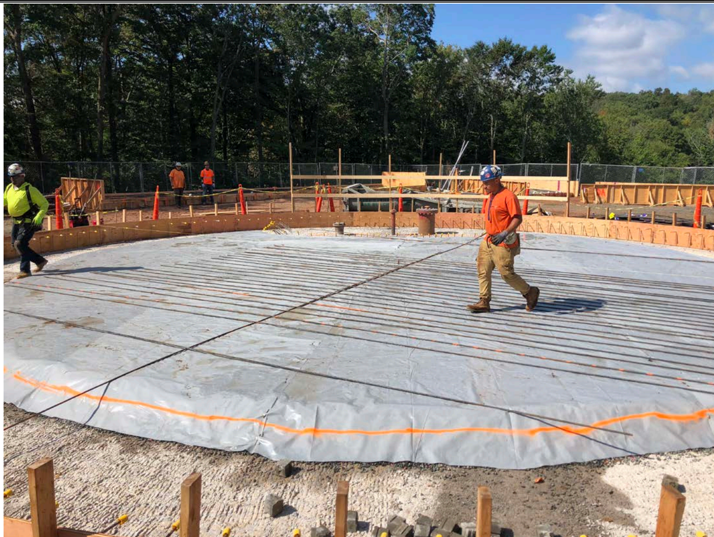
Picture 3: Northeastern Steel placing and fastening rebar on the water tank footprint. Water tank work zone, east of the Shared Access Driveway, Middletown. View to the southwest.
