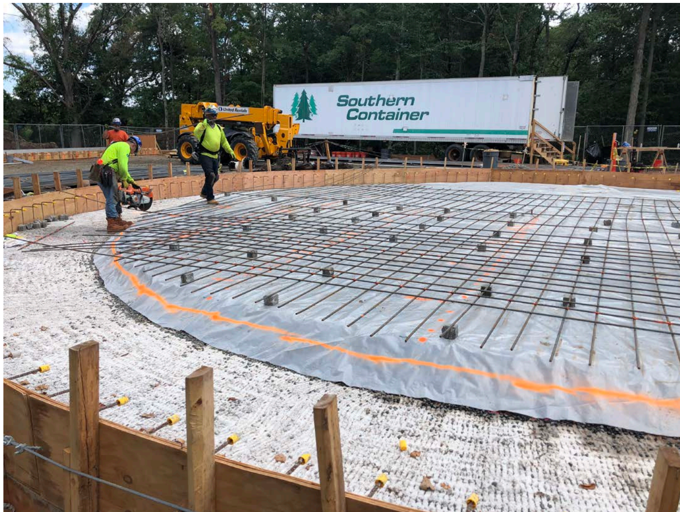
Picture 7: Northeastern Steel having progressed further in placing and fastening rebar on the water tank footprint. Water tank work zone, east of the Shared Access Driveway, Middletown. View to the southwest
