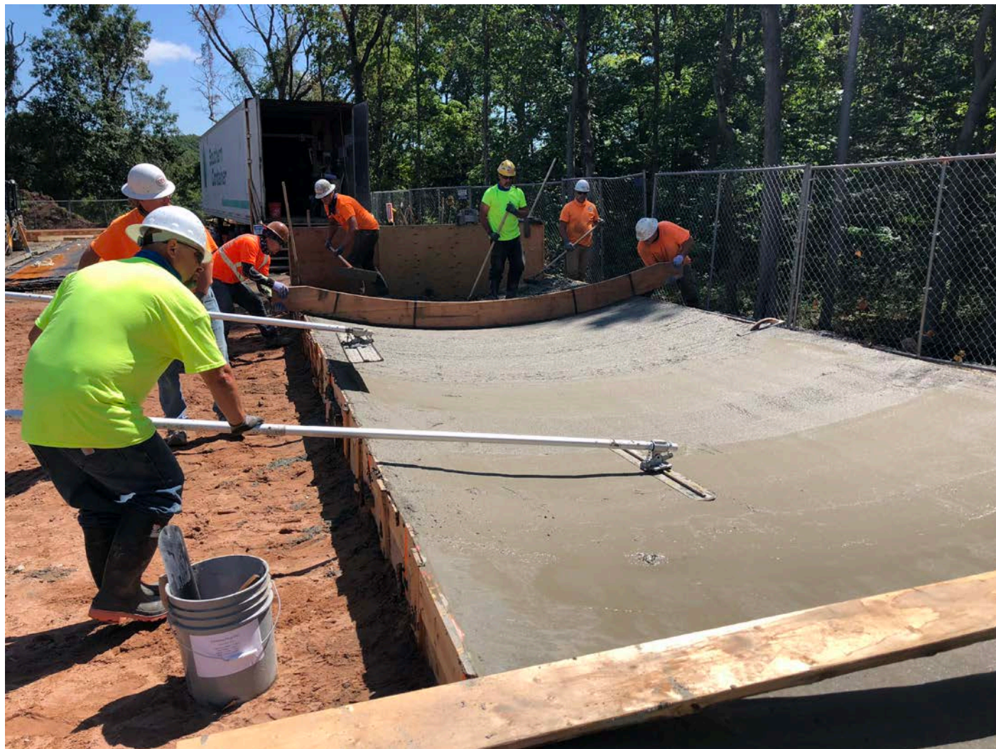
Picture 6: DN Tanks leveling placed concrete on the first of two concrete forms for the side panels of the water tank. East of the Shared Access Road, Middletown. View to the east.
