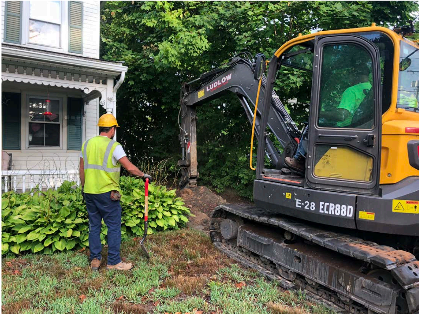
Picture 8: Ludlow trenching on the 312 Main Street, Durham property for the installation of a 1" curb stop at Station 177+54. View to the northwest.
