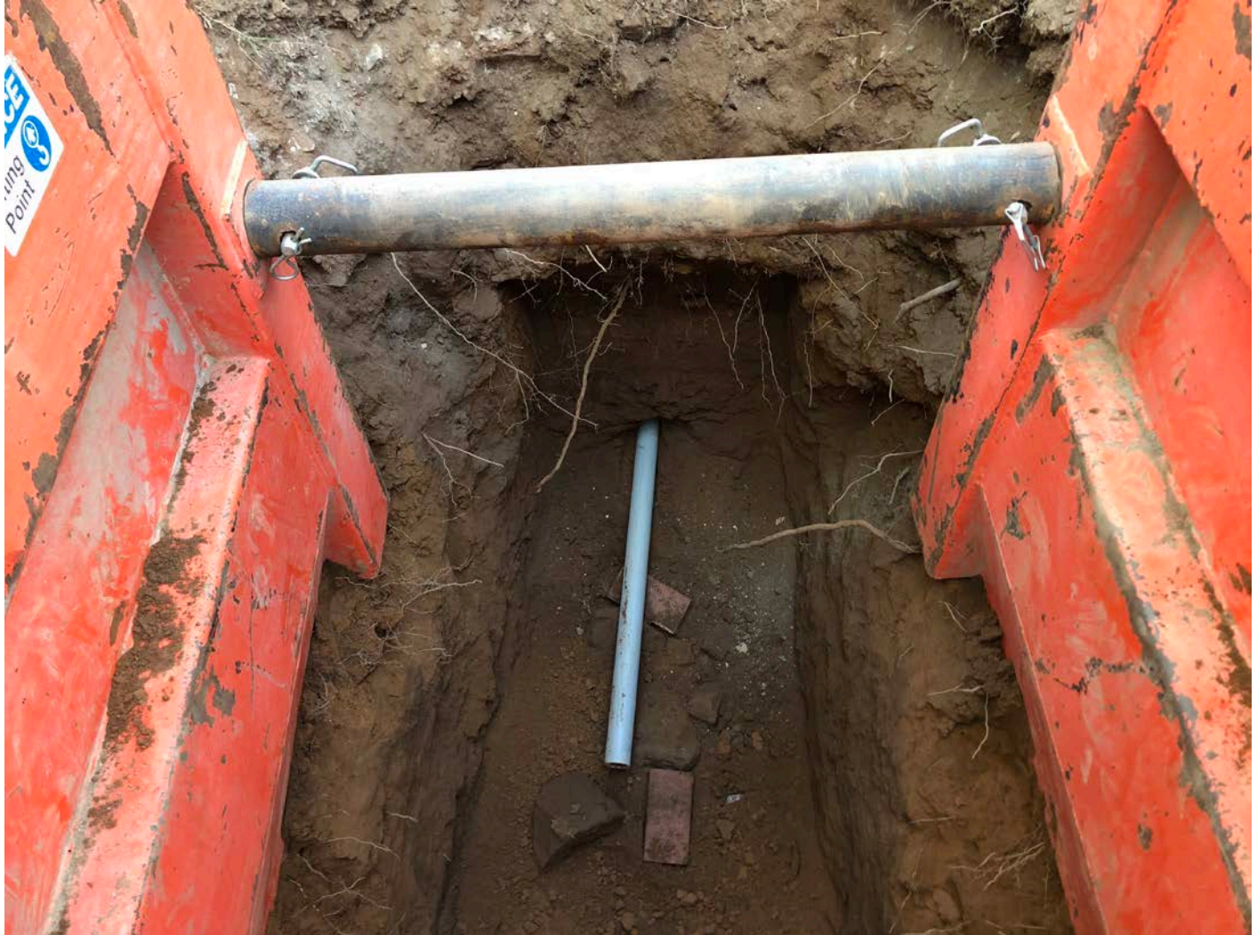
Picture 4: PVC conduit Ludlow placed to run 1" copper service line for the curb stop that was installed under the sidewalk in front of the 275 Main Street residence. Station 184+88. View to the west.
