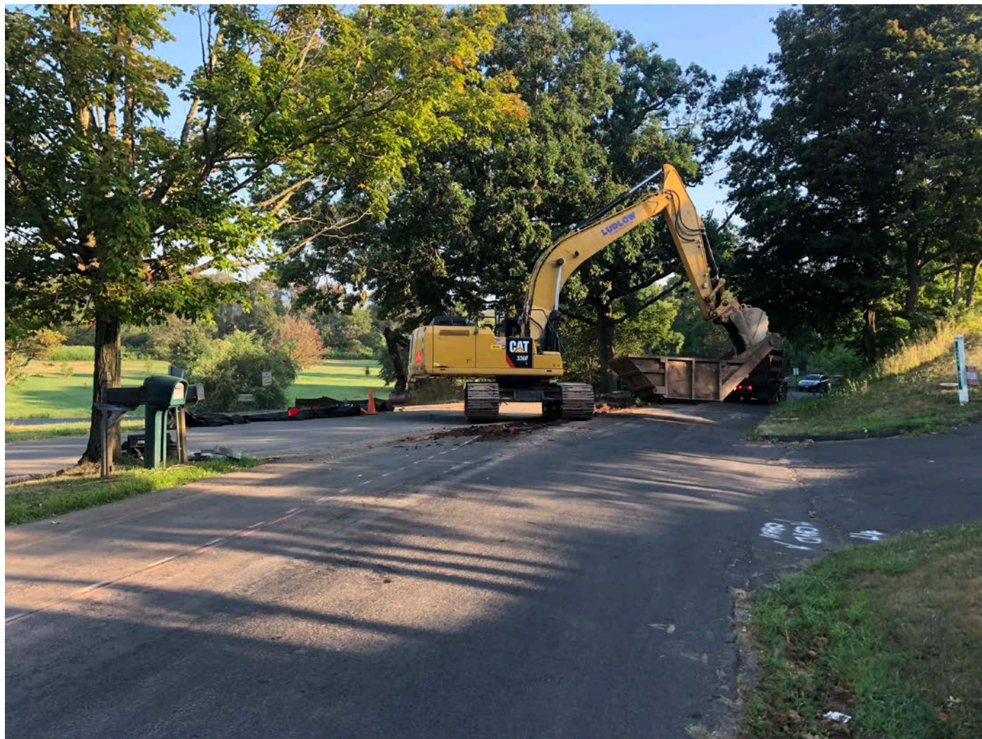
Picture 1: Ludlow excavating on Maple Avenue, Durham, at Station 901+50 for the installation of 12" DIP. View to the north.
