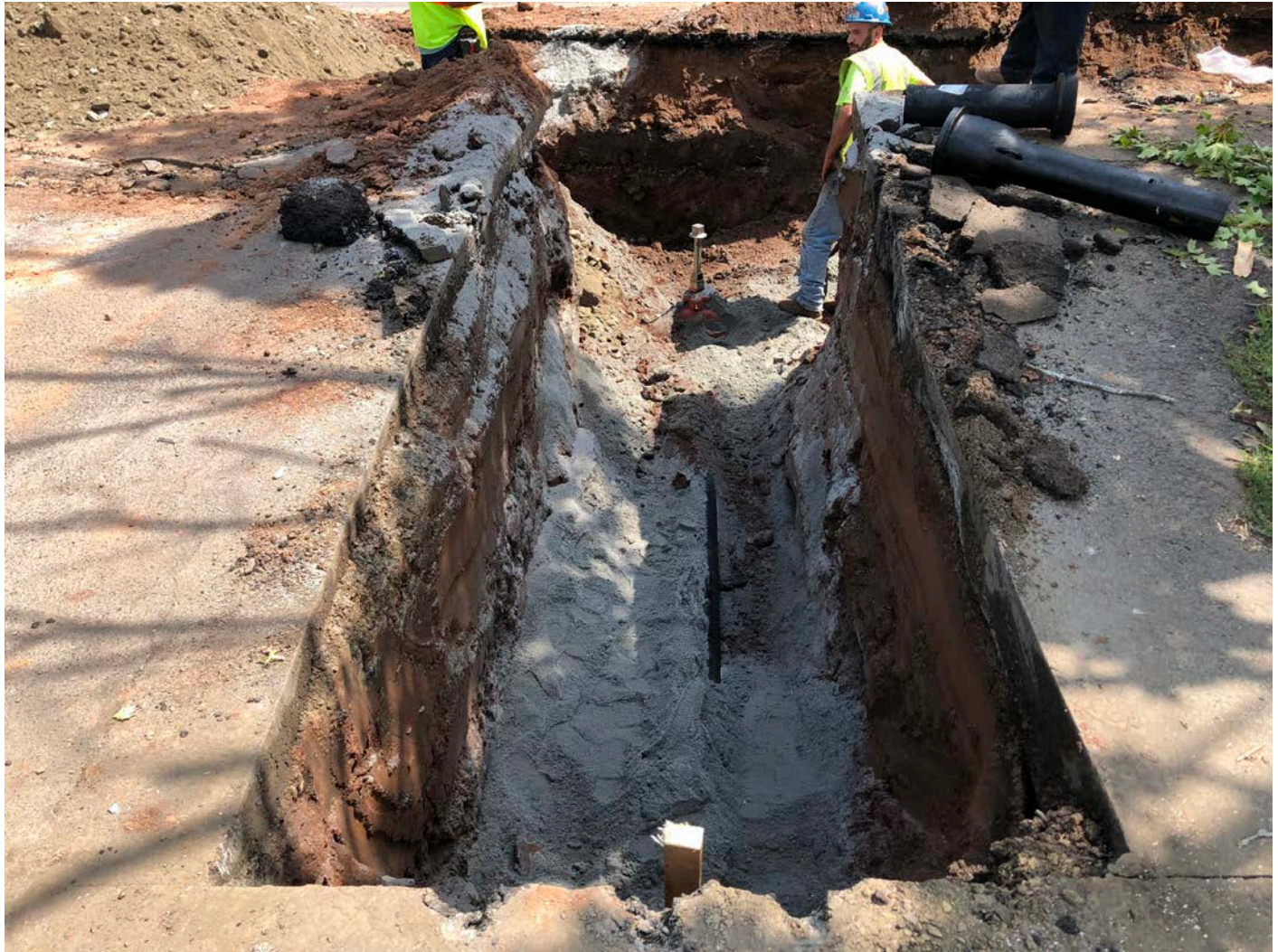
Picture 7: Ludlow installing a 14.5' section of 8" DIP at Station 900+90, placed west of Maple Avenue into the Durham fairgrounds entrance. View to the east.
