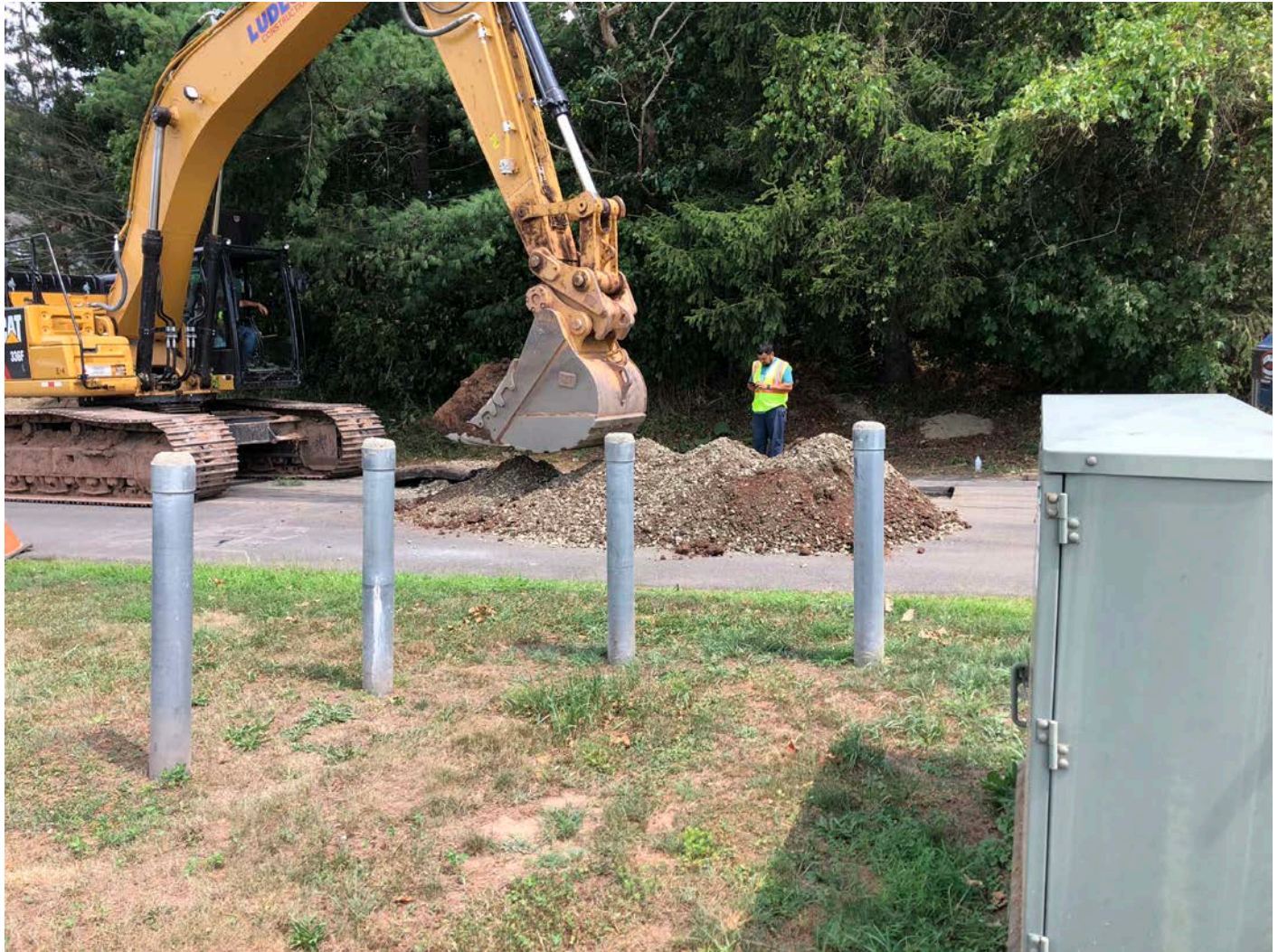
Picture 8: Ludlow excavating a test pit to the south of Station 900+00 in order to daylight the existing water line. Maple Avenue, Durham. View to the east.
