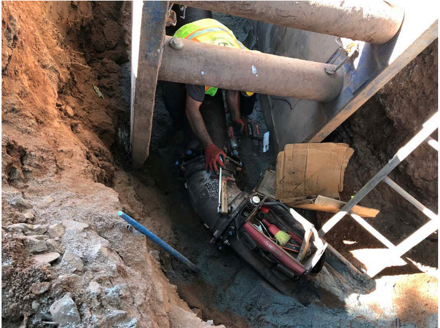
Picture 6: Ludlow attaching a 14' section of 12" DIP to the 45° bend they just installed at Station 901+65. Maple Avenue, Durham. View to the south.
