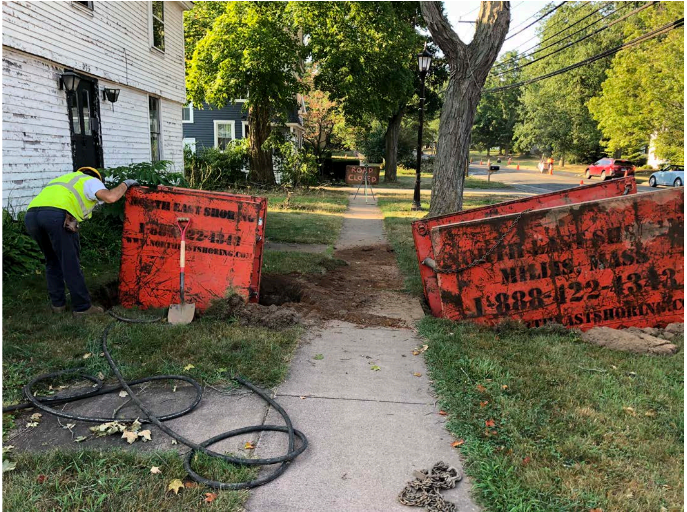
Picture 2: Ludlow installing 1" curb stop at the 275 Main Street, Durham residence at Station 184+88. View to the south.
