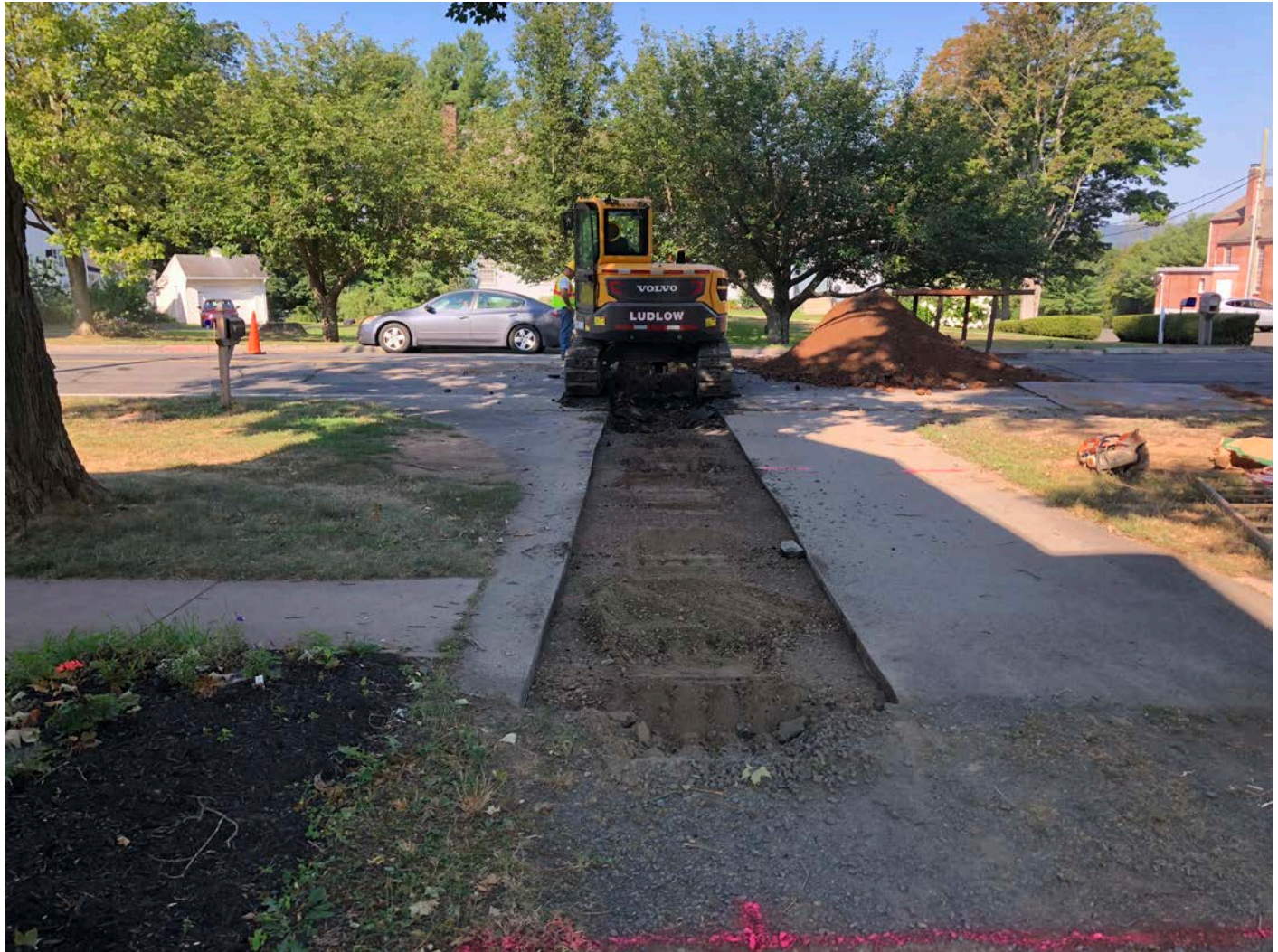
Picture 5: Ludlow working on the installation of a 1" curb stop for the residence at 271 Main Street residence. Station 185+72. View to the west.
