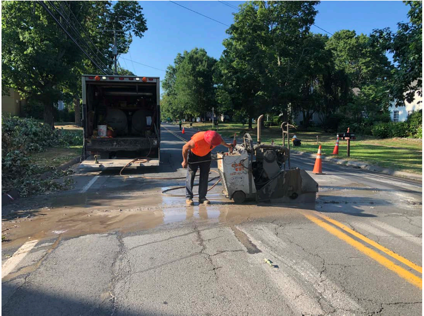
Picture 3: Ludlow saw cutting pavement in front of 265 Main Street for the installation of a curb stop. View to the south.
