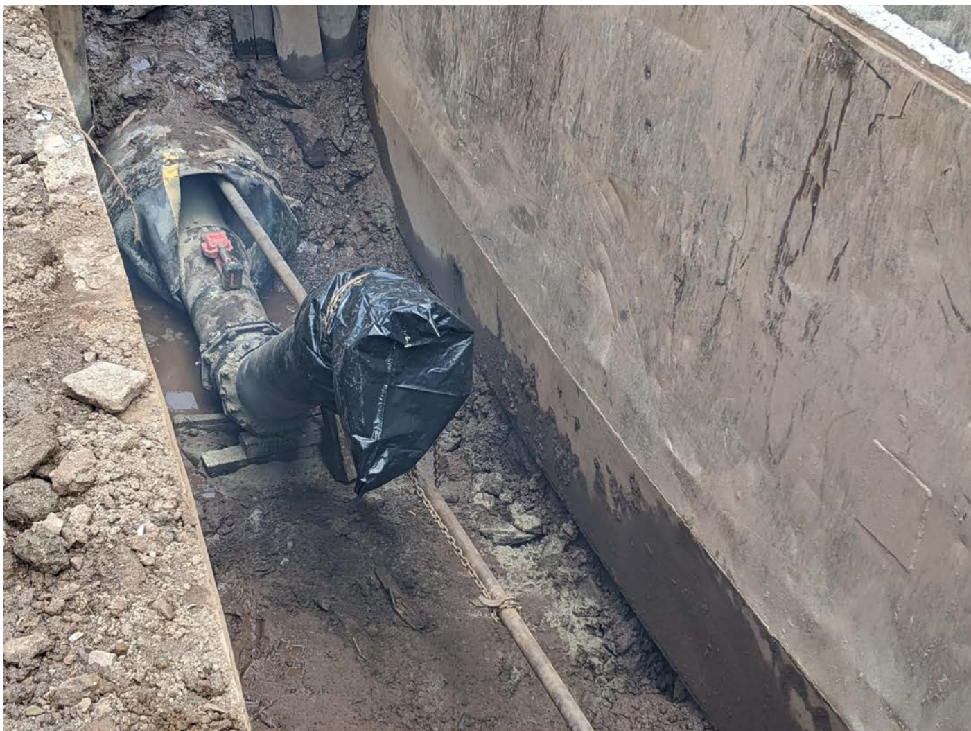
Picture 11: Pipe blowing sand into the annular space between the steel casing and DIP, Station 905 + 00. View to the north.
