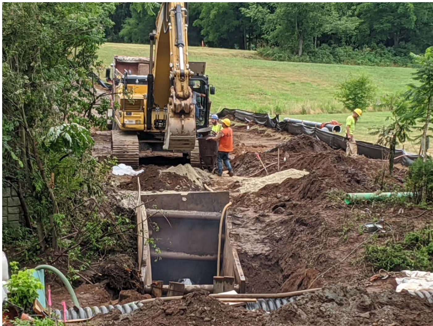
Picture 1: Ludlow Construction beginning to blow sand into the steel casing, Station 905 + 00. View to the south.
