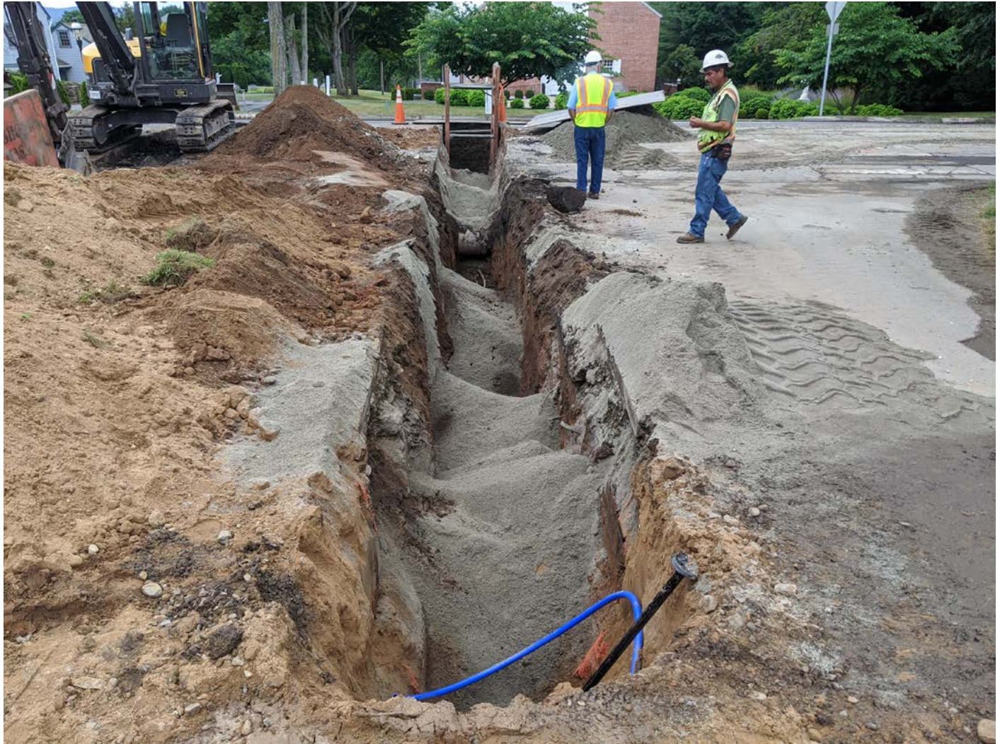
Picture 8: Curb stop installed at Station 184+00 location across from the church, Main Street, Station 184+00. View to the west.
