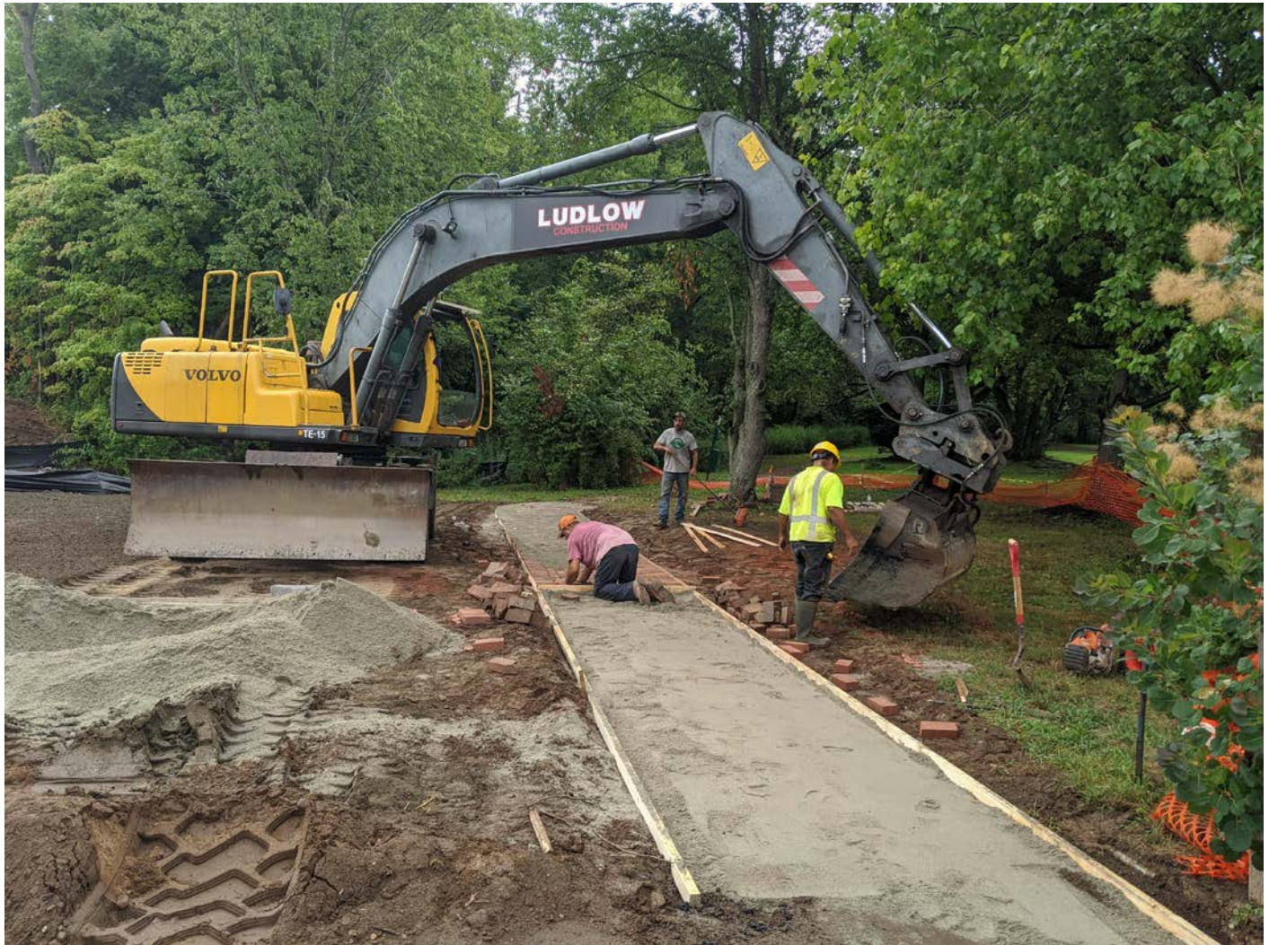
Picture 2: Ludlow Construction restoring a brick sidewalk on Pickett Lane, Pickett Lane, Station 512 + 25. View to the north.
