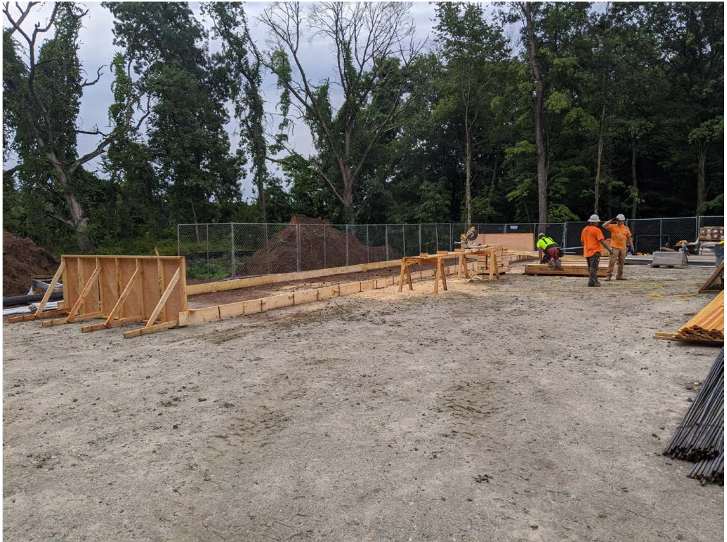
Picture 5: DN tanks working on the concrete forms for the water tank, Shared Access Driveway. View to the northeast.
