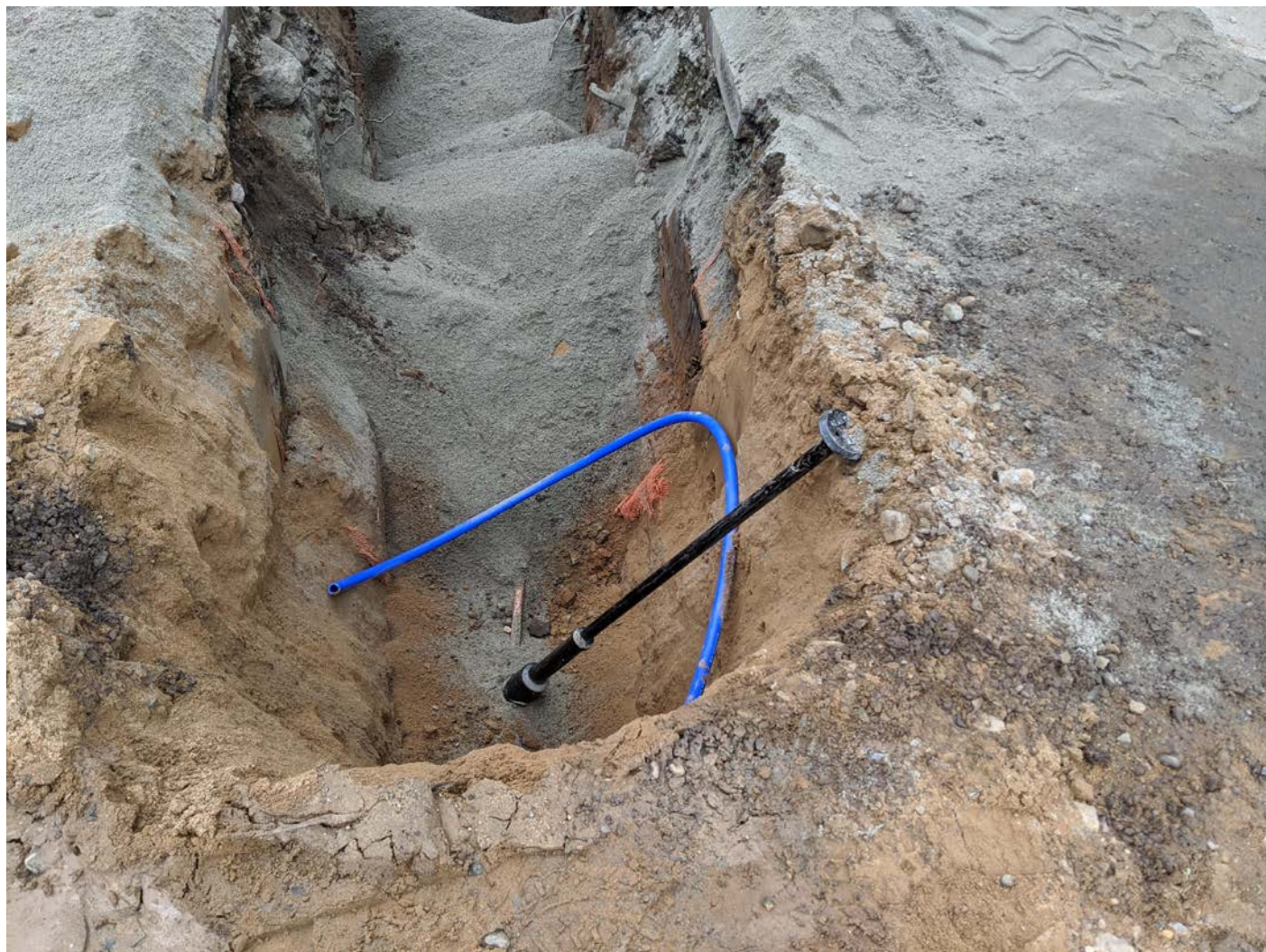
Picture 9: Curb stop installed at the station 184+00 location across from the church, Main Street, Station 184+00. View to the west.
