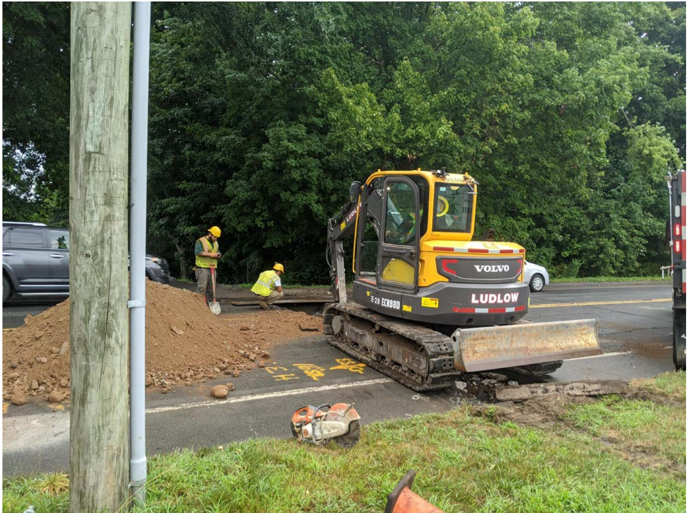
Picture 4: Ludlow Construction working on exposing the water main between 183+00 and 183+50 on Main Street, Main Street, Stations 183+00 and 183+50. View to the west.
