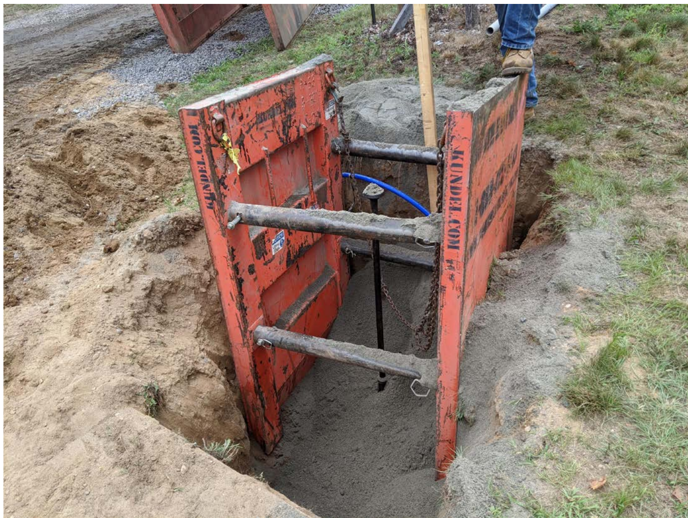
Picture 13: Curb stop installed at station 184+50 on Main Street, Main Street, Station 184+50. View to the west.
