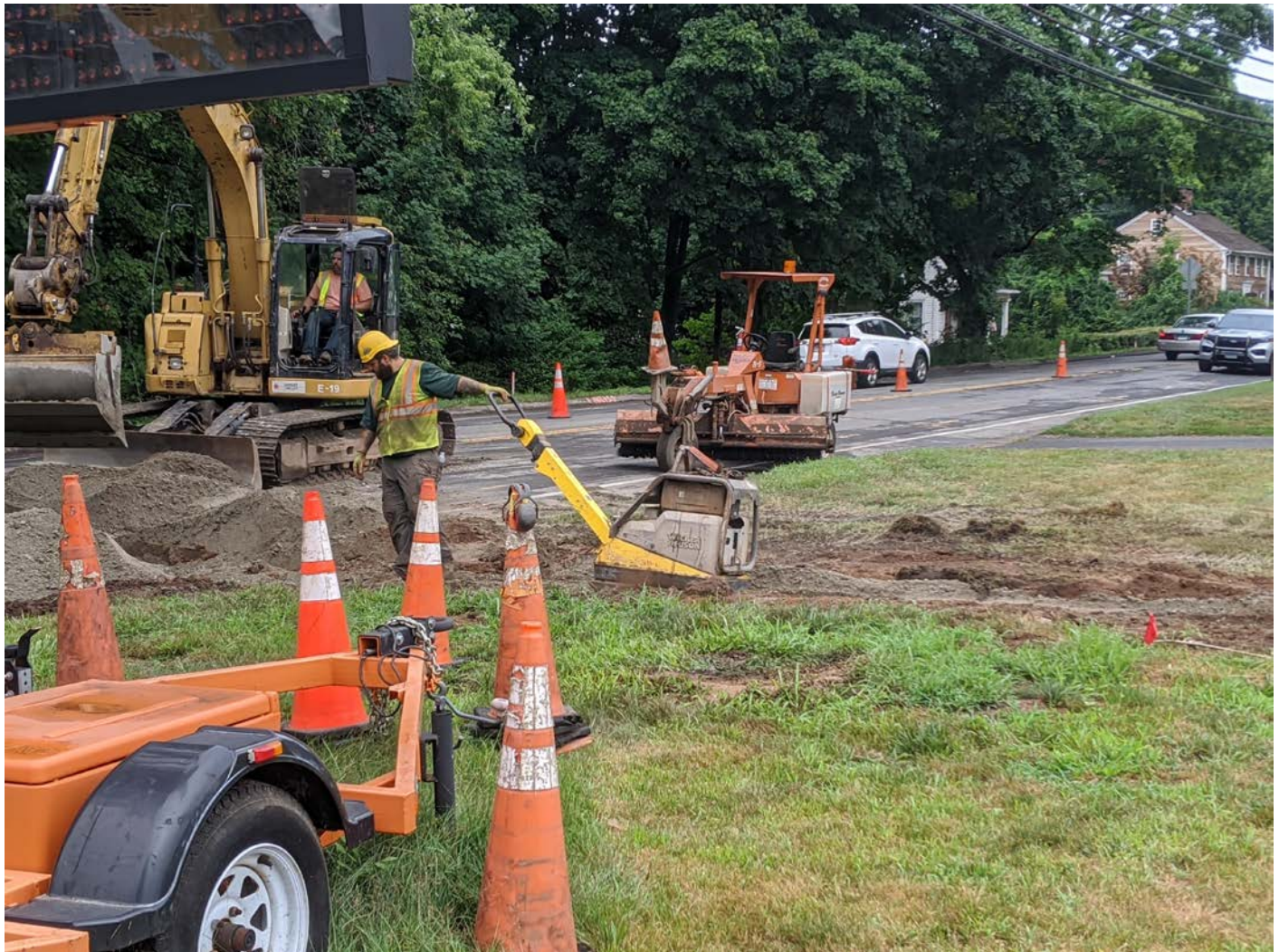
Picture 7: Ludlow Construction compacting the trench line between stations 183+00 and 183+50 on Main Street, Main Street, Station 183+00 and 183+50. View to the northwest.
