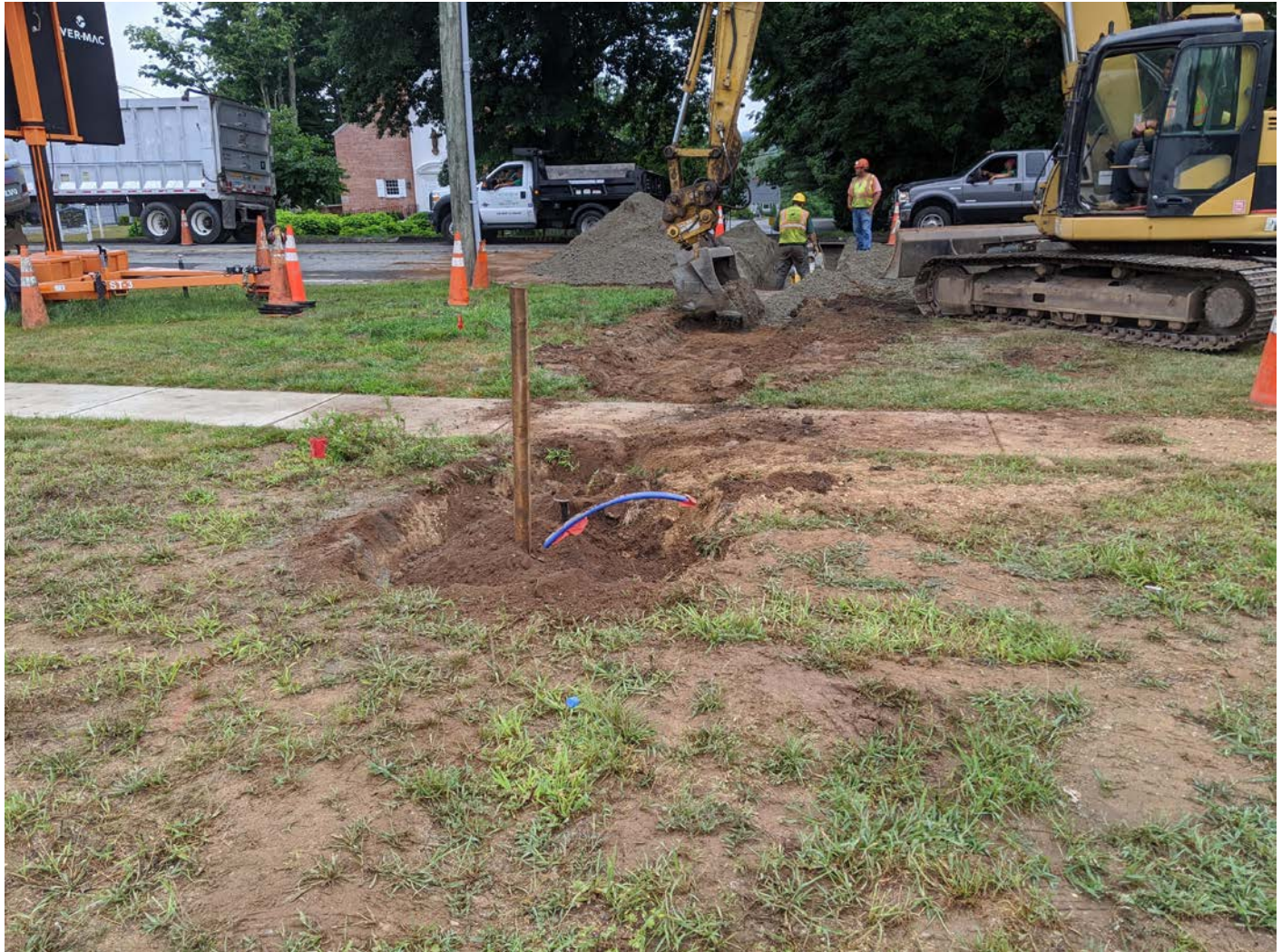
Picture 6: Curb stop installed between stations 183+00 and 183+50 on Main Street, Main Street, Stations 183+00 and 183+50. View to the west.
