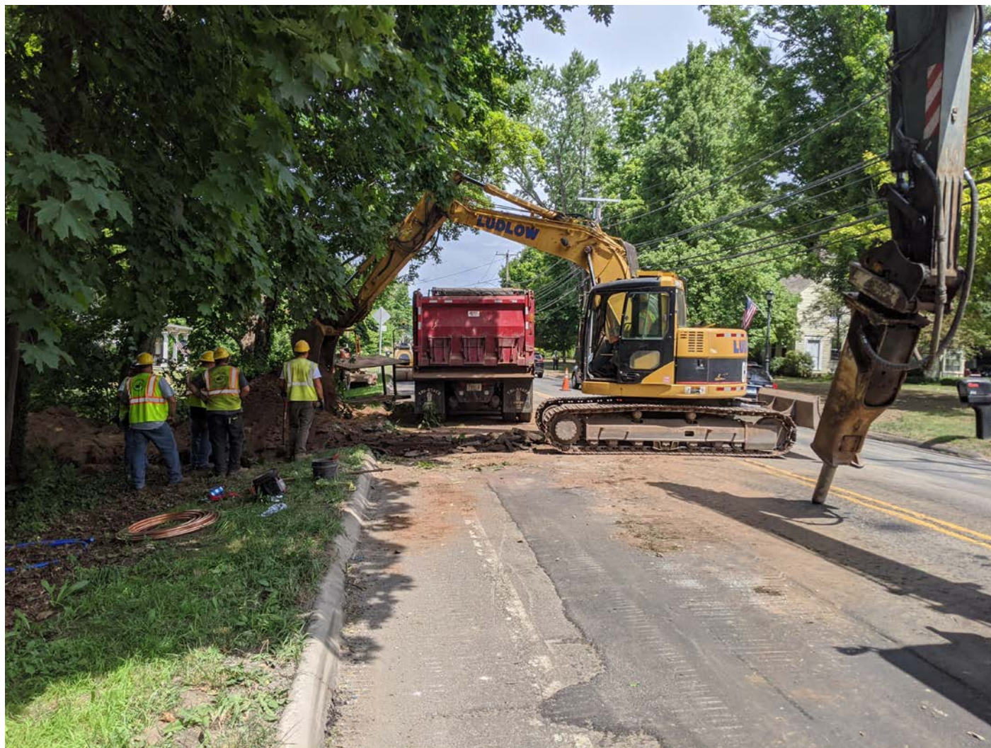
Picture 7: Ludlow Construction digging trench for the curb stop installation at Station 182+00, Main Street, Durham. View to the north.
