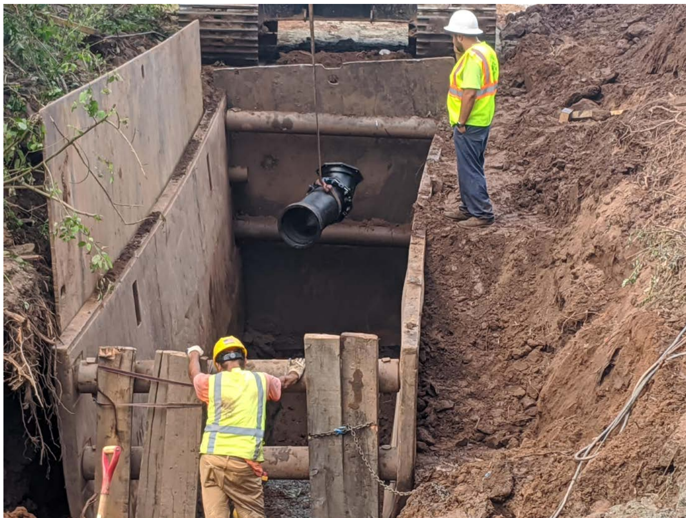
Picture 2: Ludlow Construction installing a vertical bend to the 12" DIP piping in the trench, Maple Avenue, Station 905 + 00. View to the south.
