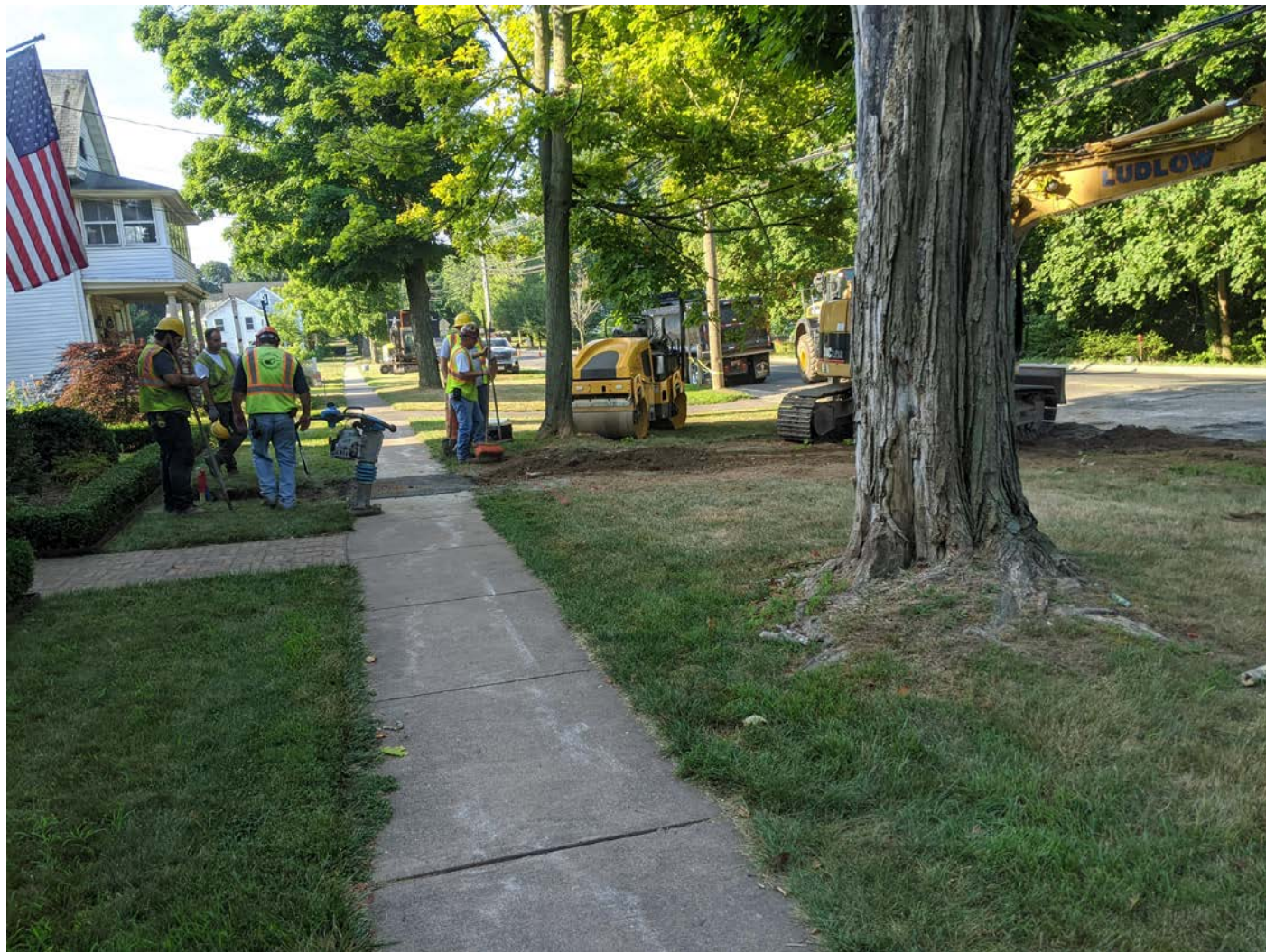
Picture 3: Ludlow Construction compacting trench to 293 Main Street, Main Street, Station 182+00. View to the south.
