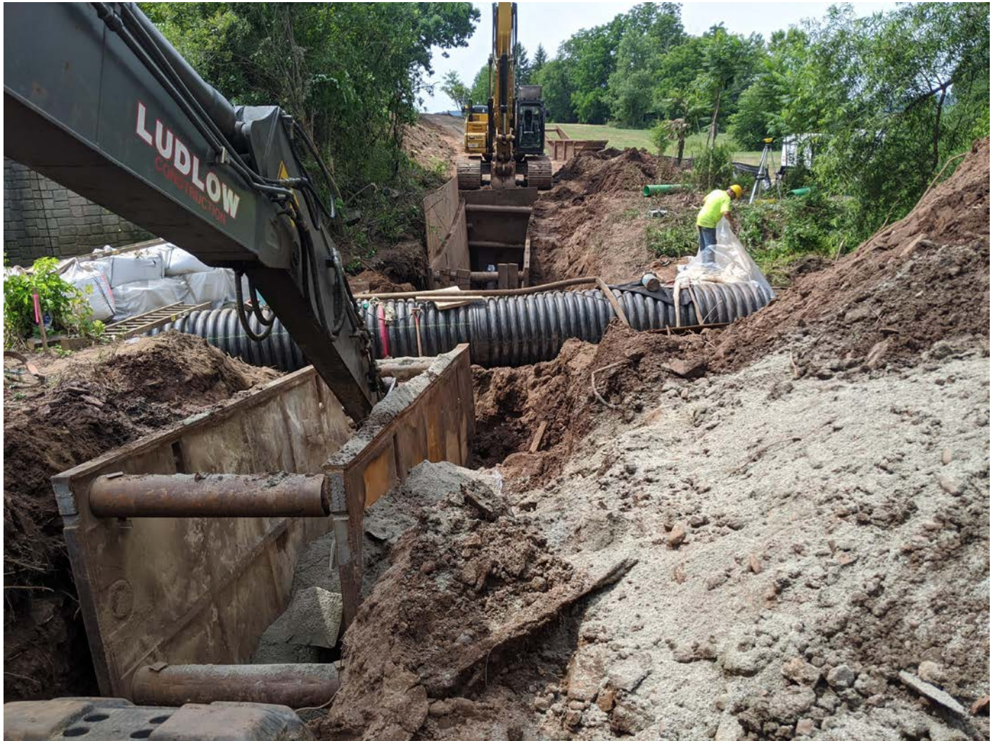
Picture 9: Ludlow Construction backfilling excavation with bedding, Maple Avenue, Station 905+00. View to the south.
