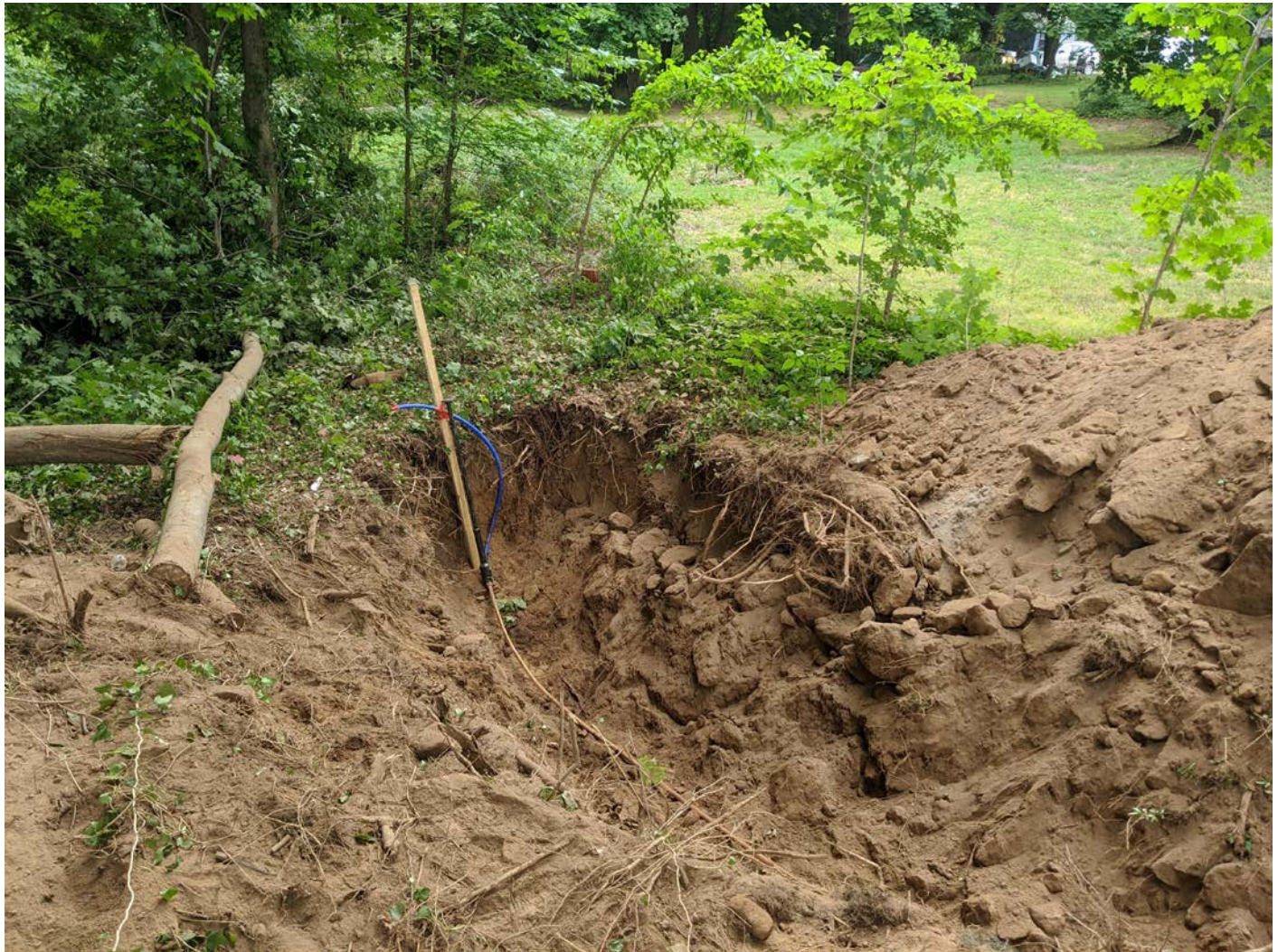
Picture 8: Curb stop partially installed at the Station 182+00 location, Main Street, Durham. View to the west.
