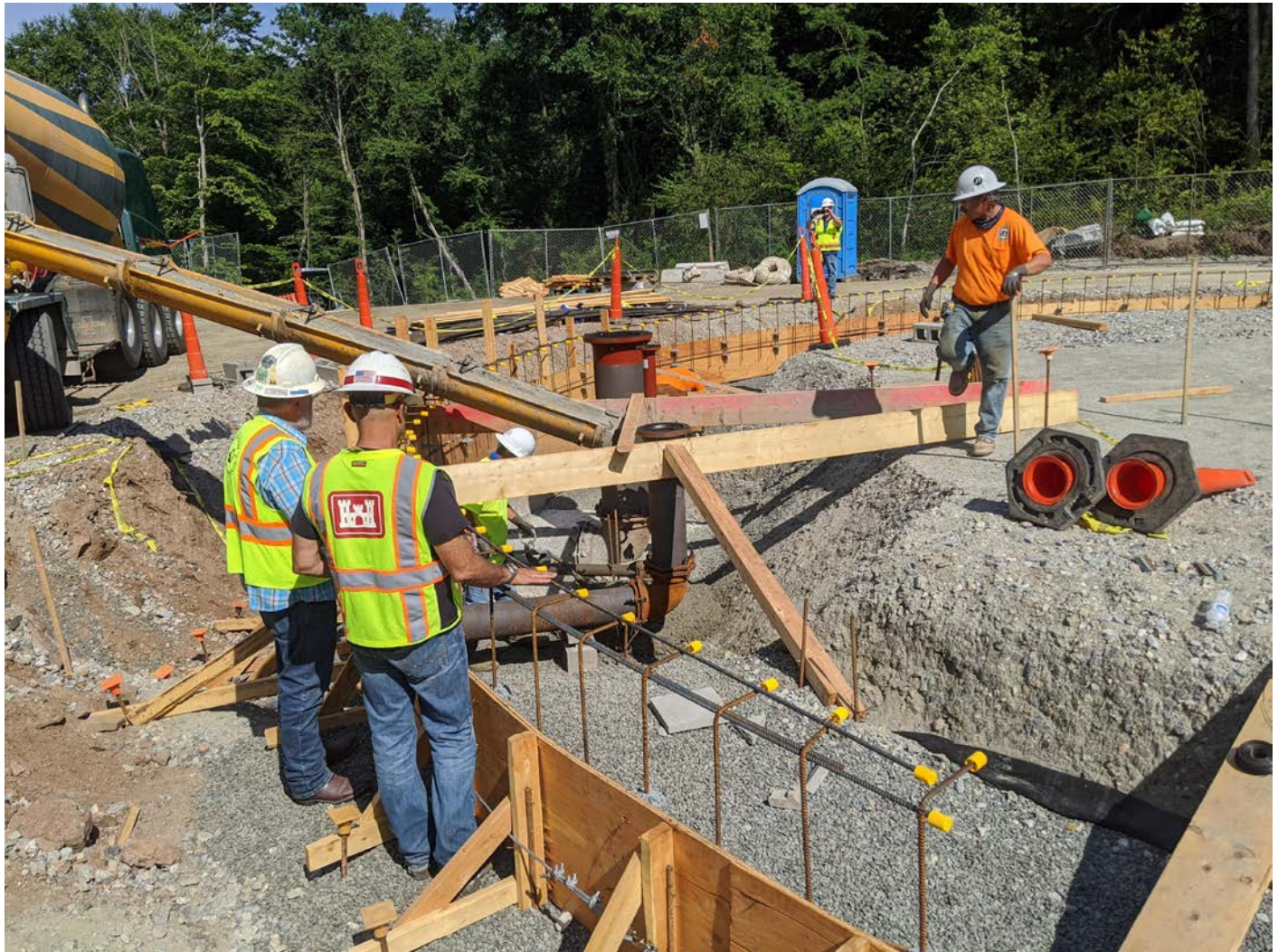
Picture 4: Concrete being placed around the pipes for the water tank, Shared Access Driveway. View to the north.
