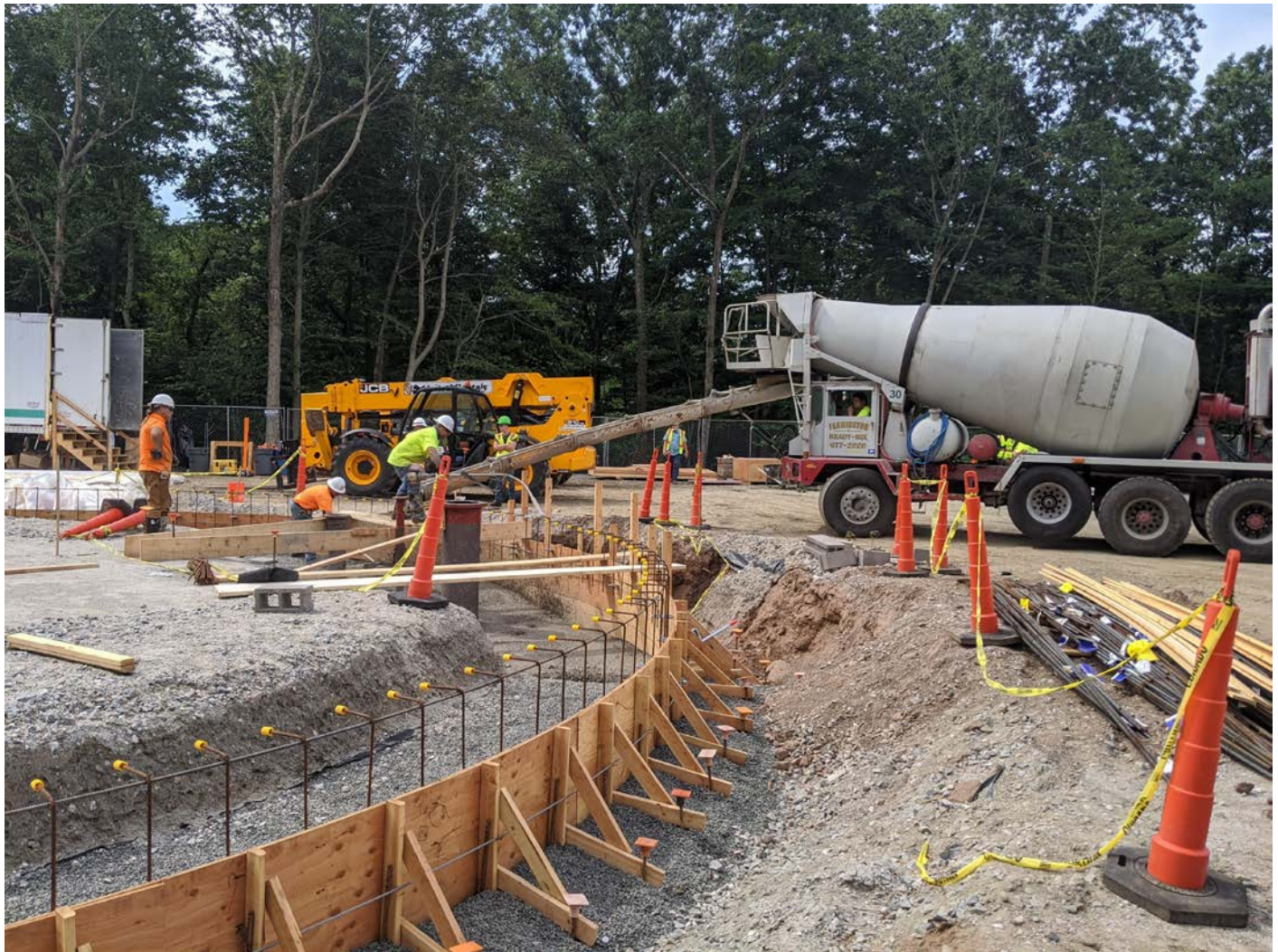
Picture 5: Concrete being placed around the pipes for the water tank, Shared Access Driveway. View to the south.
