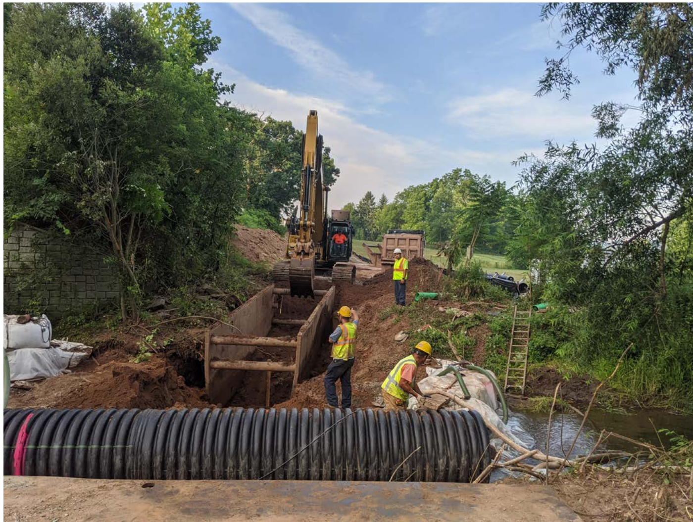
Picture 1: Ludlow Construction moving trench box after installing a 20' section of 12" DIP, Maple Avenue, Station 905 + 00. View to the south.
