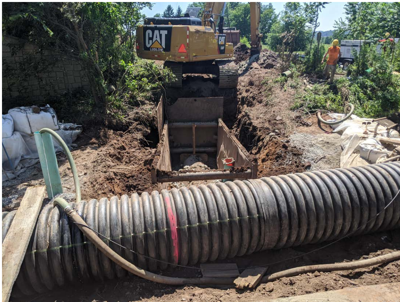
Picture 7: Ludlow construction backfilling stream bed excavation with soil and gravel, Maple Avenue, Station 905+00. View to the south.
