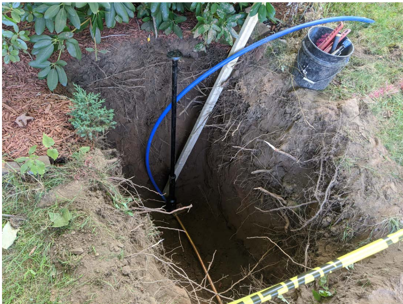
Picture 5: Curb stop installed by Ludlow construction at 297 Main Street, Main Street, Station 180+50. View to the east.
