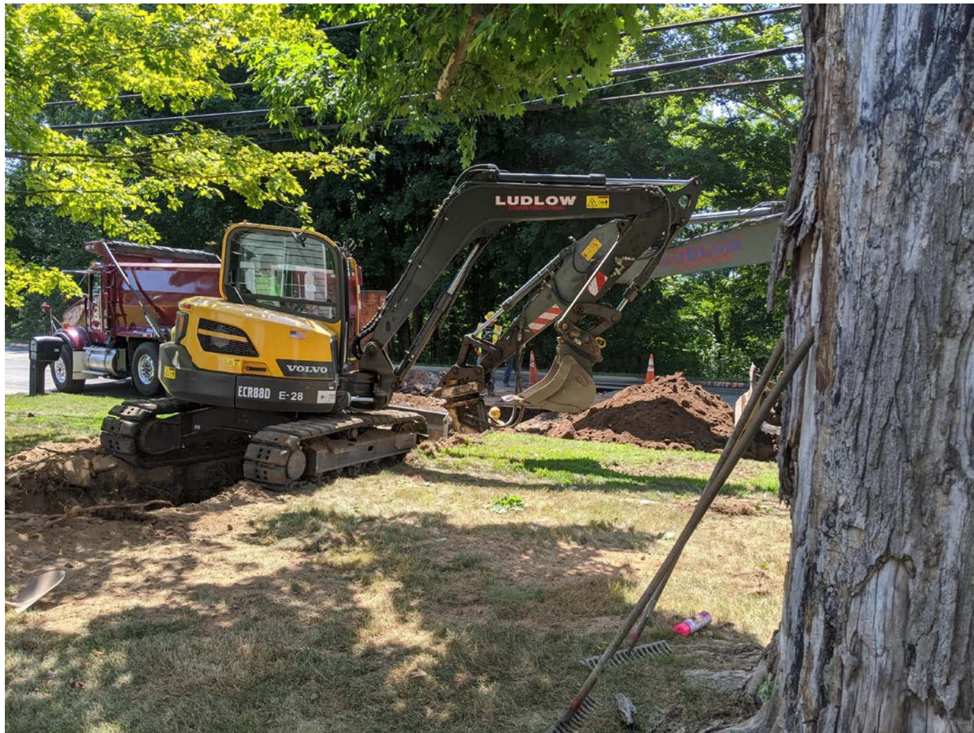
Picture 8: Ludlow construction rock hammering in a trench line at 293 Main Street due to shallow bedrock, Main Street, Station 182 + 00. View to the west.
