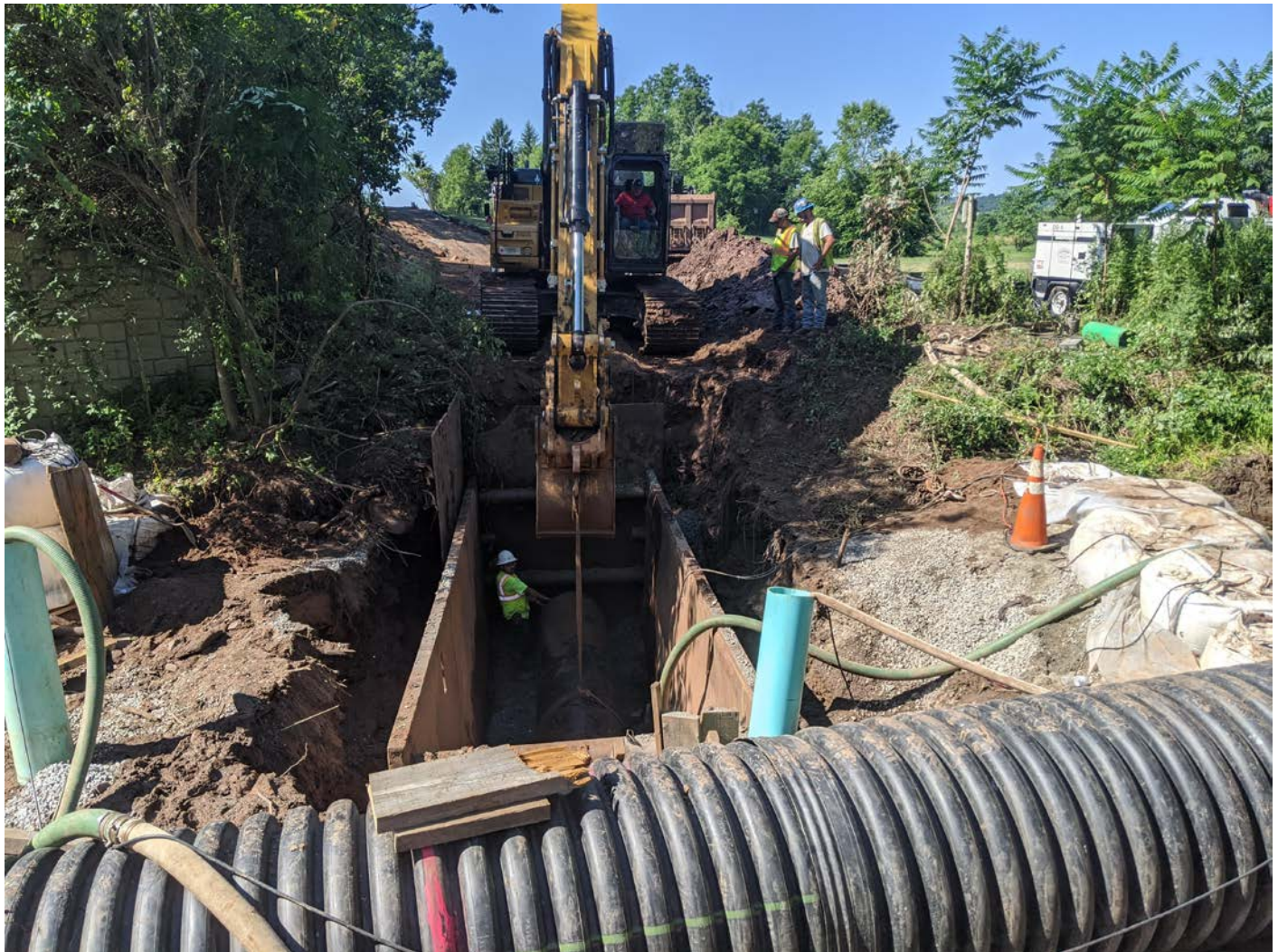
Picture 3: Ludlow construction installing 36" diameter steel casing into the stream bed excavation, Maple Avenue, Station 905+00. View to the south.
