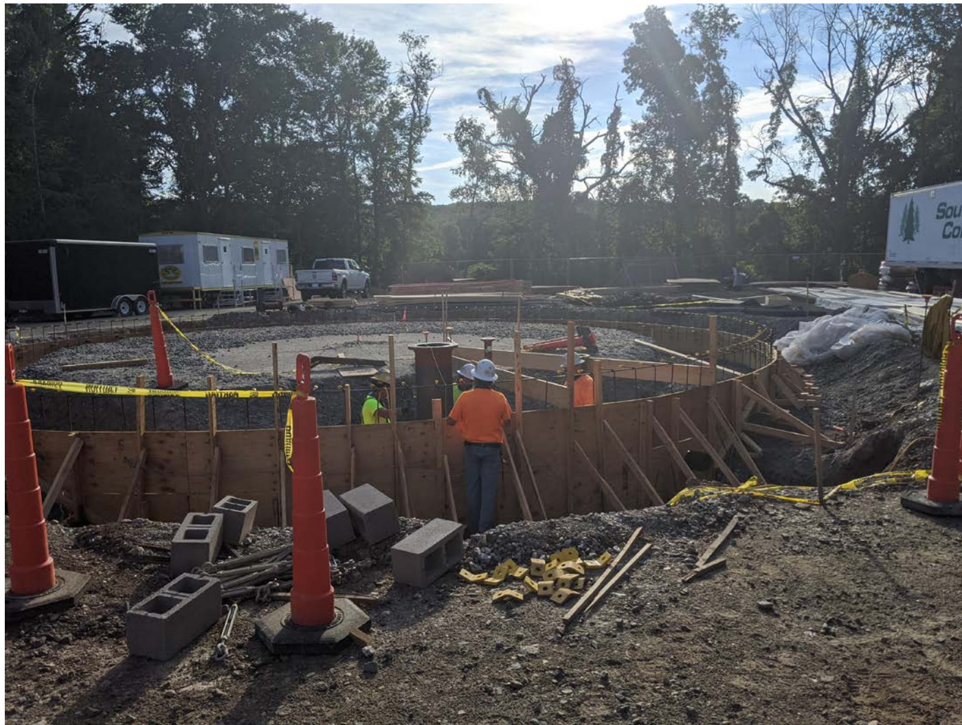
Picture 6: DN Tanks checking levels of newly installed tank piping, Shared access driveway. View to the north.
