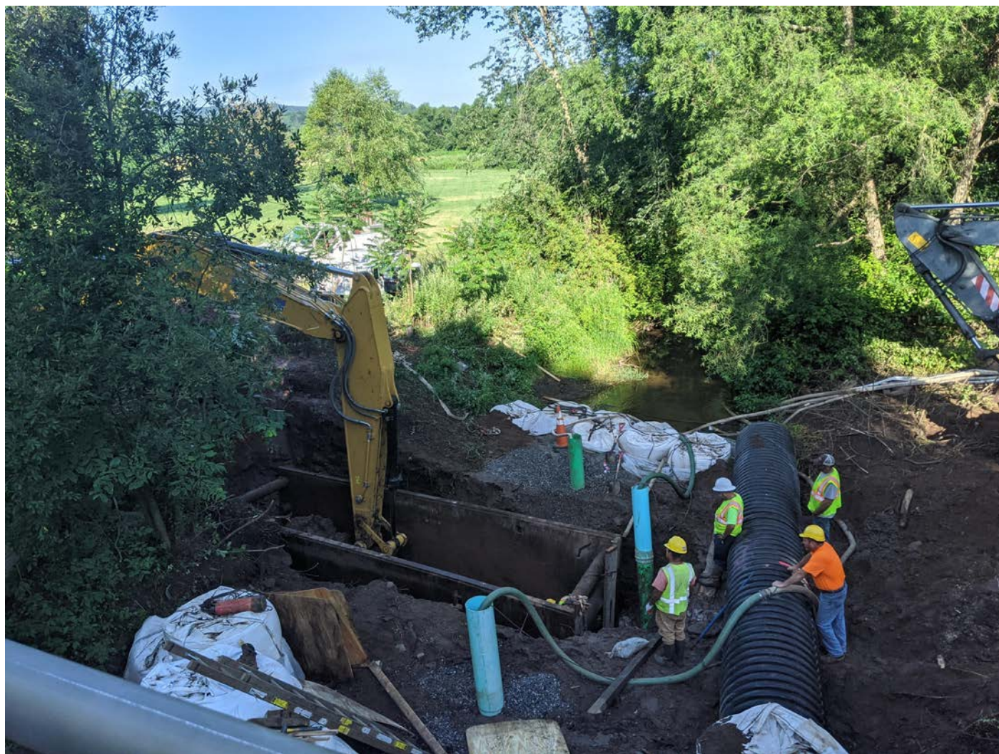
Picture 2: Ludlow construction installing a trench box in the new excavation area, Maple Avenue, Station 905 + 00. View to the southwest.
