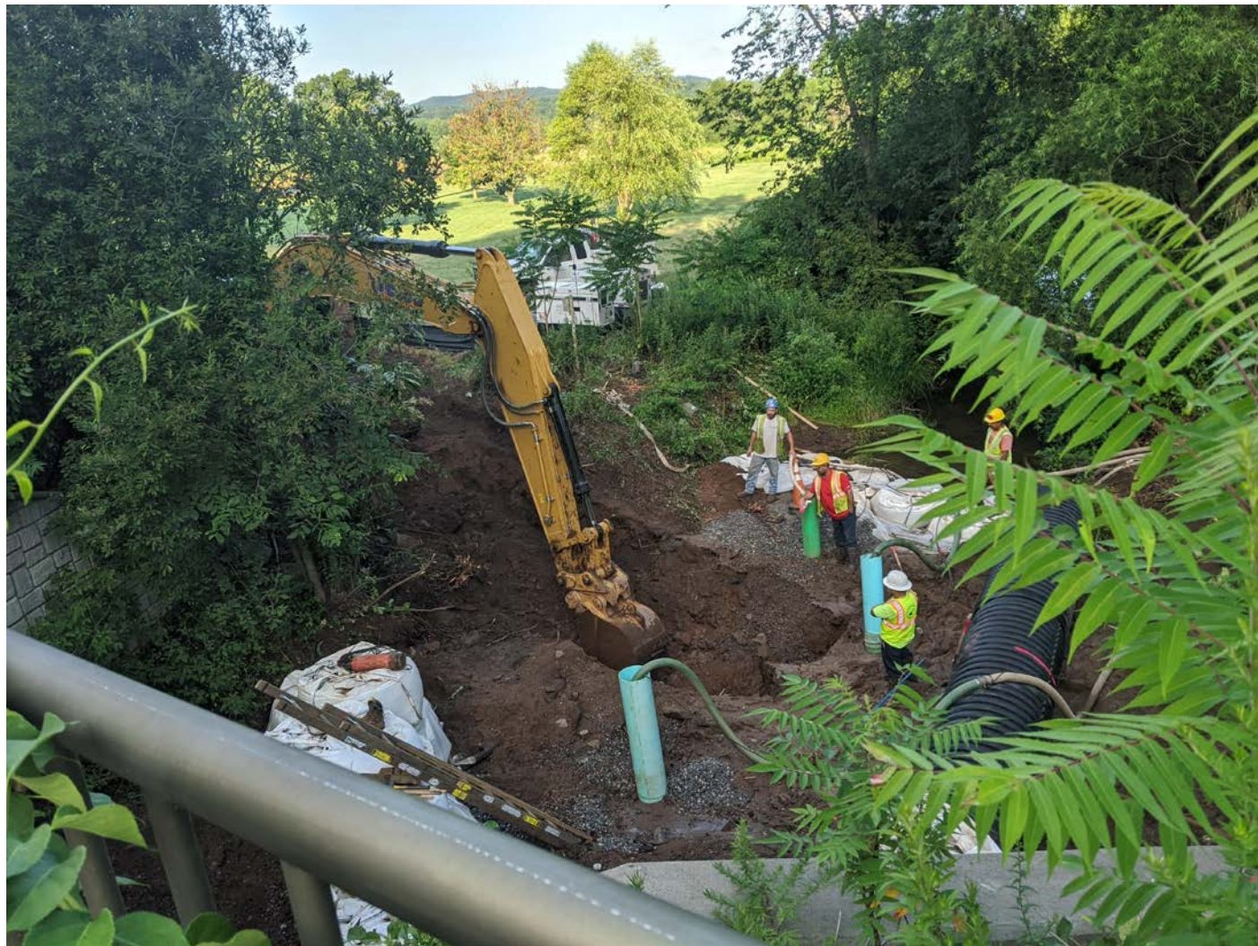
Picture 1: Ludlow construction digging new trench for 36" steel casing, Maple Avenue, Station 905 + 00. View to the southwest.
