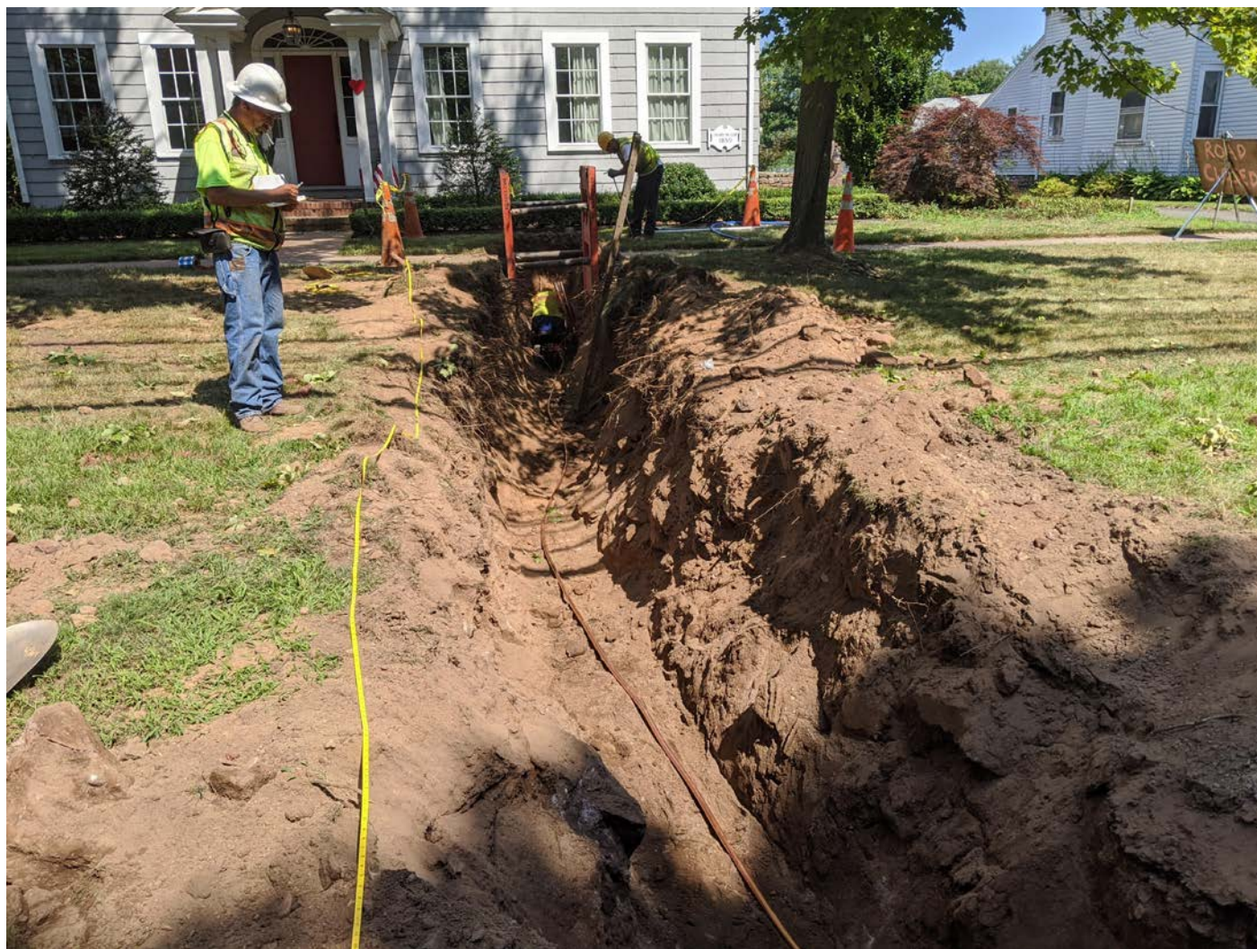
Picture 10: Ludlow construction installing curb stop at 293 Main Street, Main Street, Station 182+00. View to the east.
