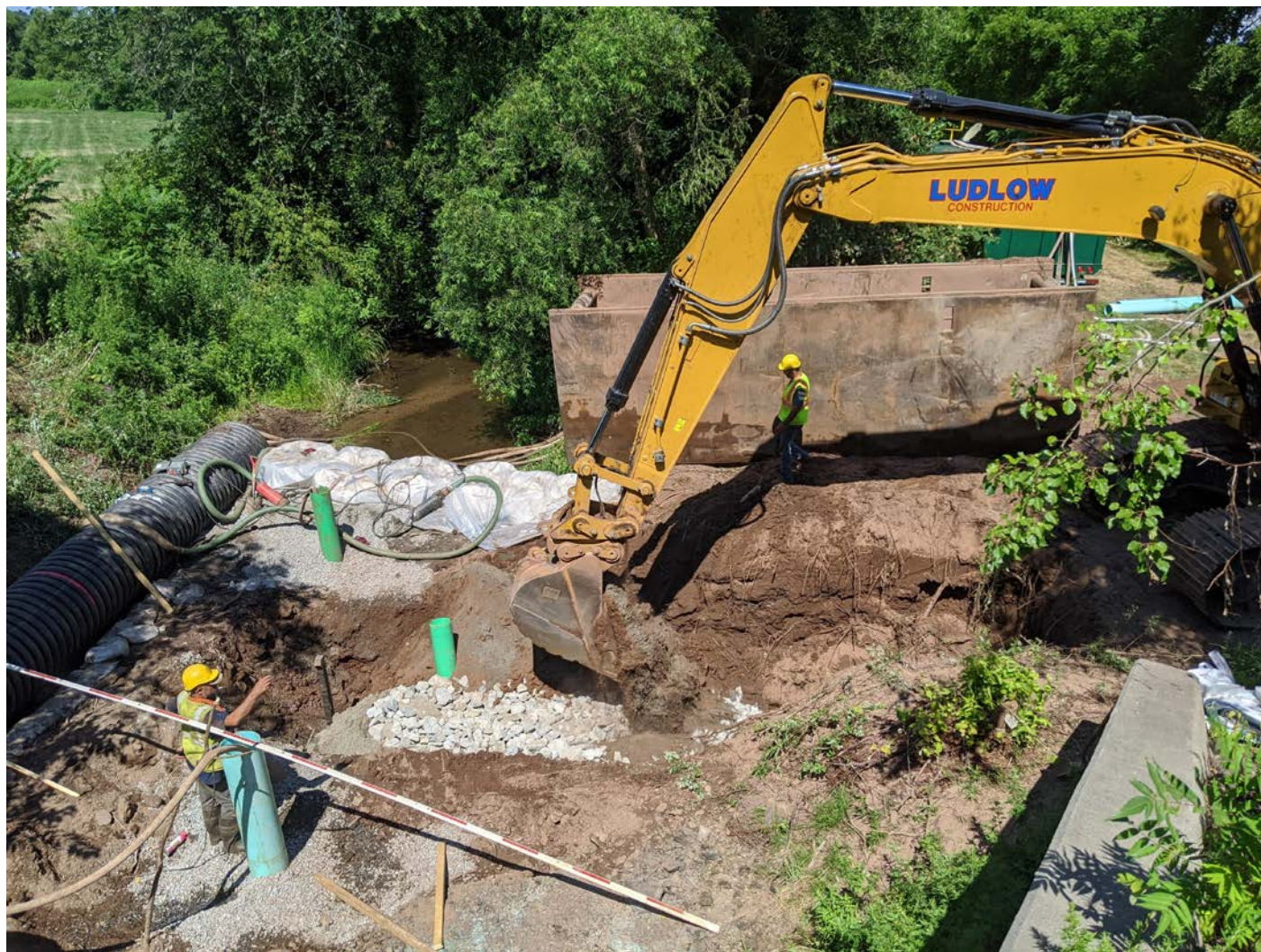
Picture 10: Ludlow Construction backfilling the stream bed excavation with soil and rip rap, Maple Avenue, Station 905. View to the west.
