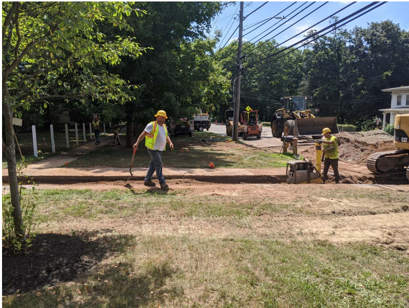
Picture 9: Ludlow Construction compacting the trench line to 303 Main Street, Main Street, Station 179+50. View to the south.
