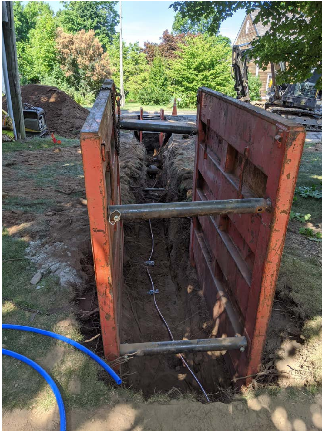
Picture 8: Trench showing service line running towards 305R Main Street, Shared access road. View to the west.
