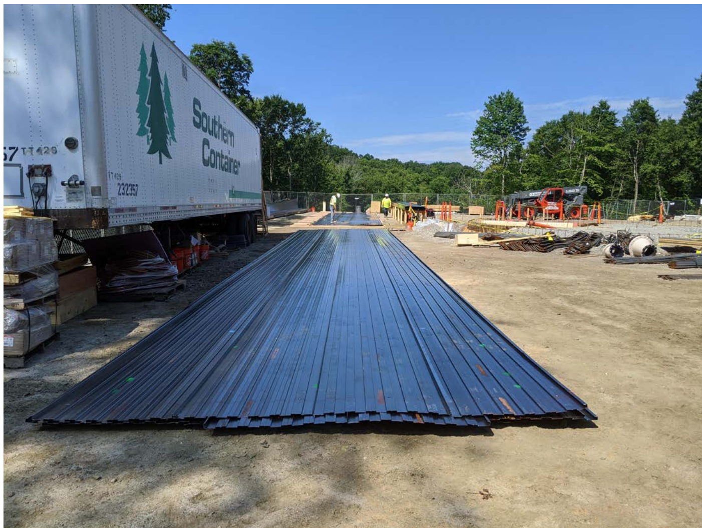
Picture 7: Stack of sheet metal for the water tank side panels, Shared access driveway. View to the south.
