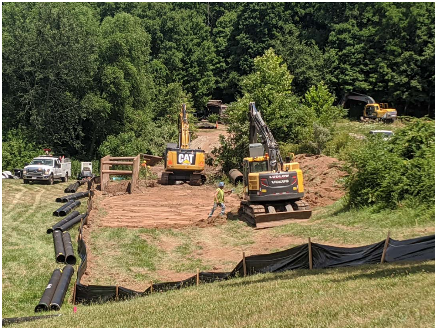
Picture 12: Ludlow construction removing topsoil in preparation for a piping run on the south side of Allyn Brook, Maple Avenue. View to the North.
