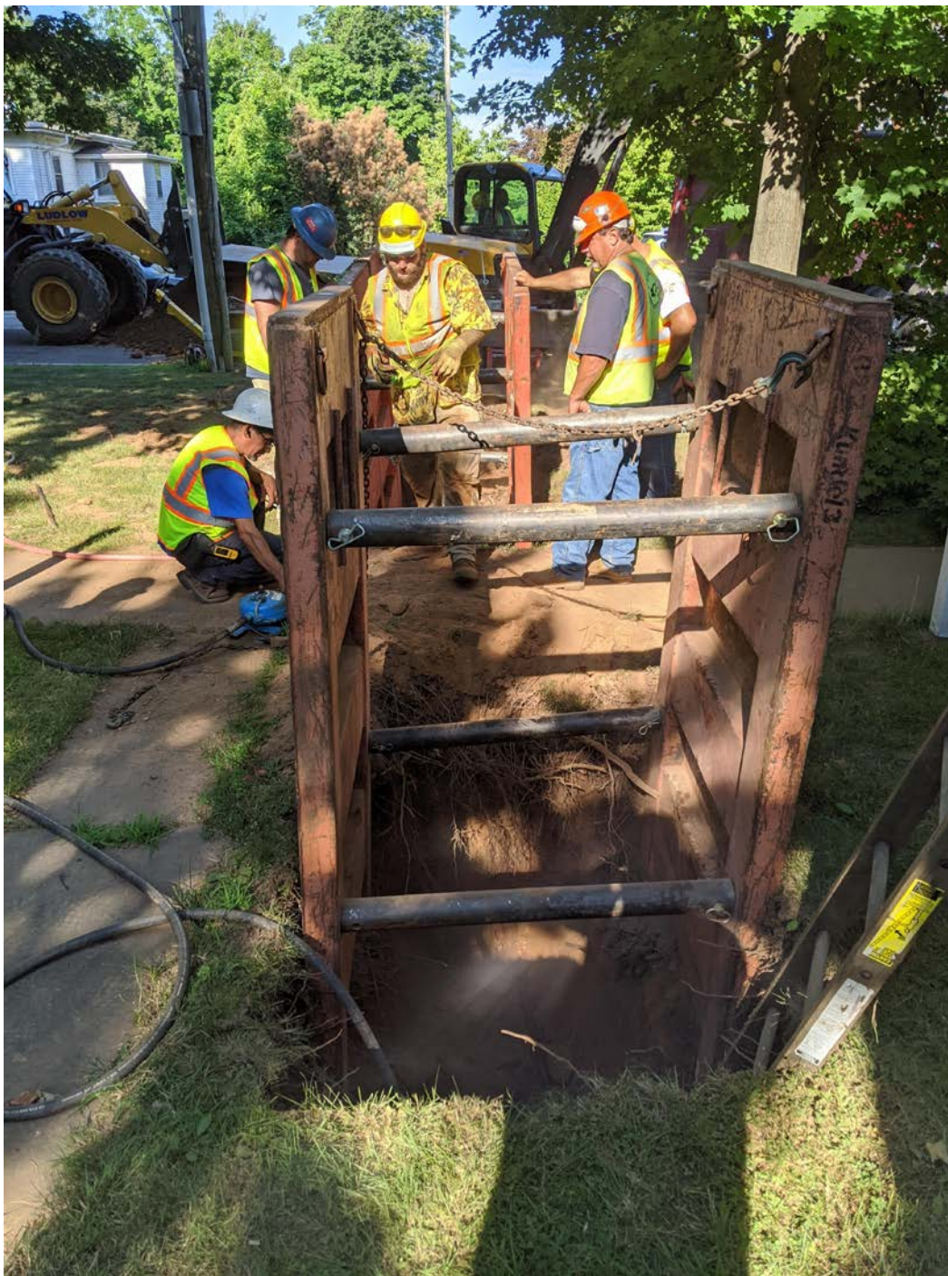
Picture 5: Ludlow construction using a pneumatic horizontal drill to install the service line for 303 Main Street, Main Street, Station 179+50. View to the west.
