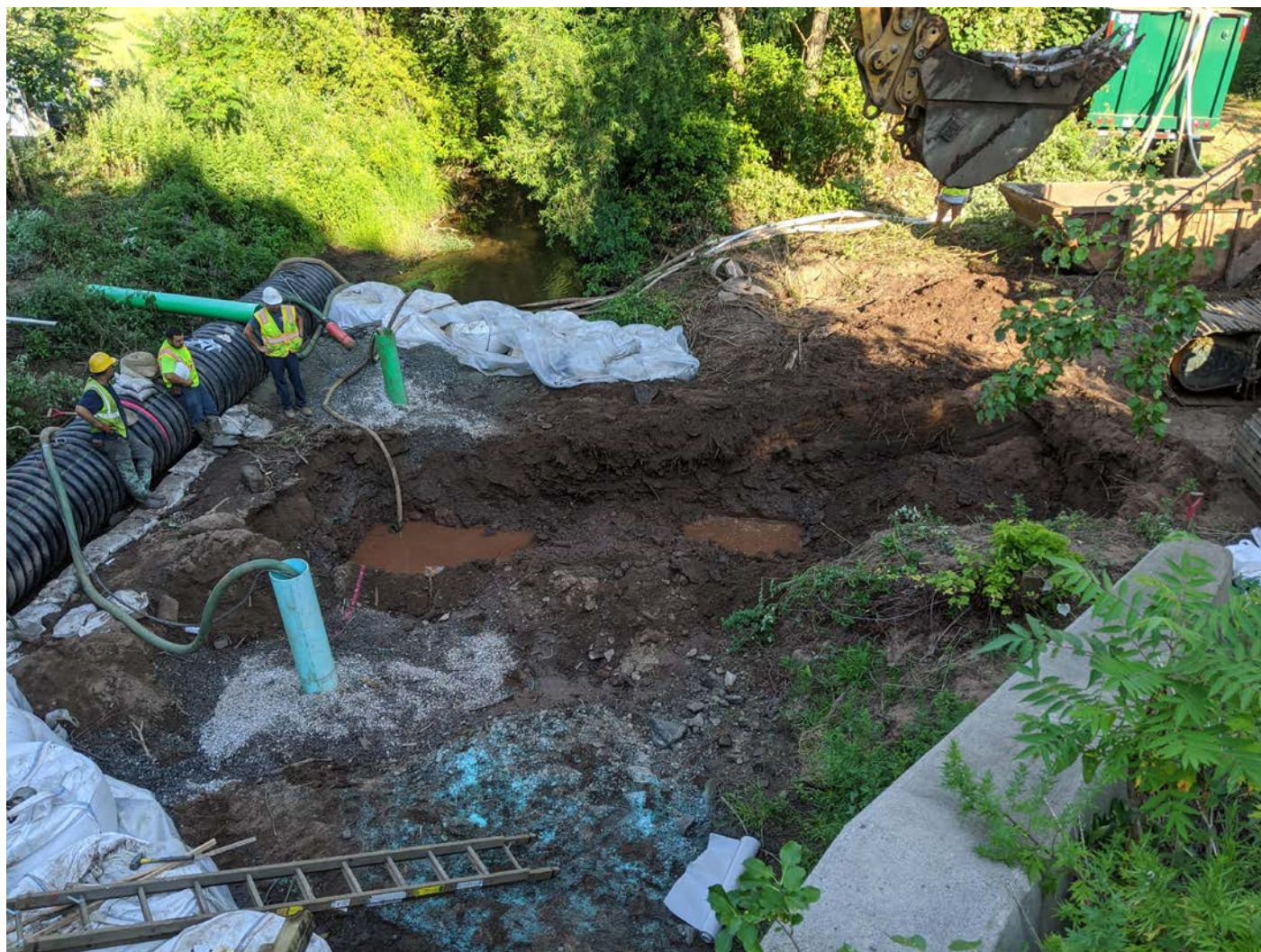
Picture 2: Ludlow construction pumping groundwater from the stream bed excavation, Maple Avenue, Station 905+00. View to the west.
