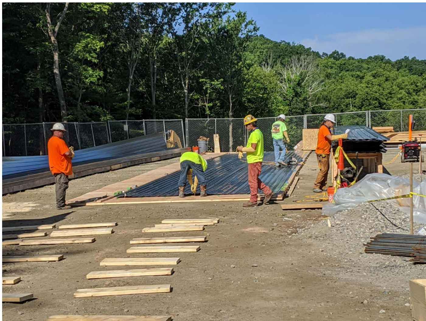
Picture 6: DN Tanks seaming together the sheet metal for the tank side panels, Shared access driveway. View to the south.
