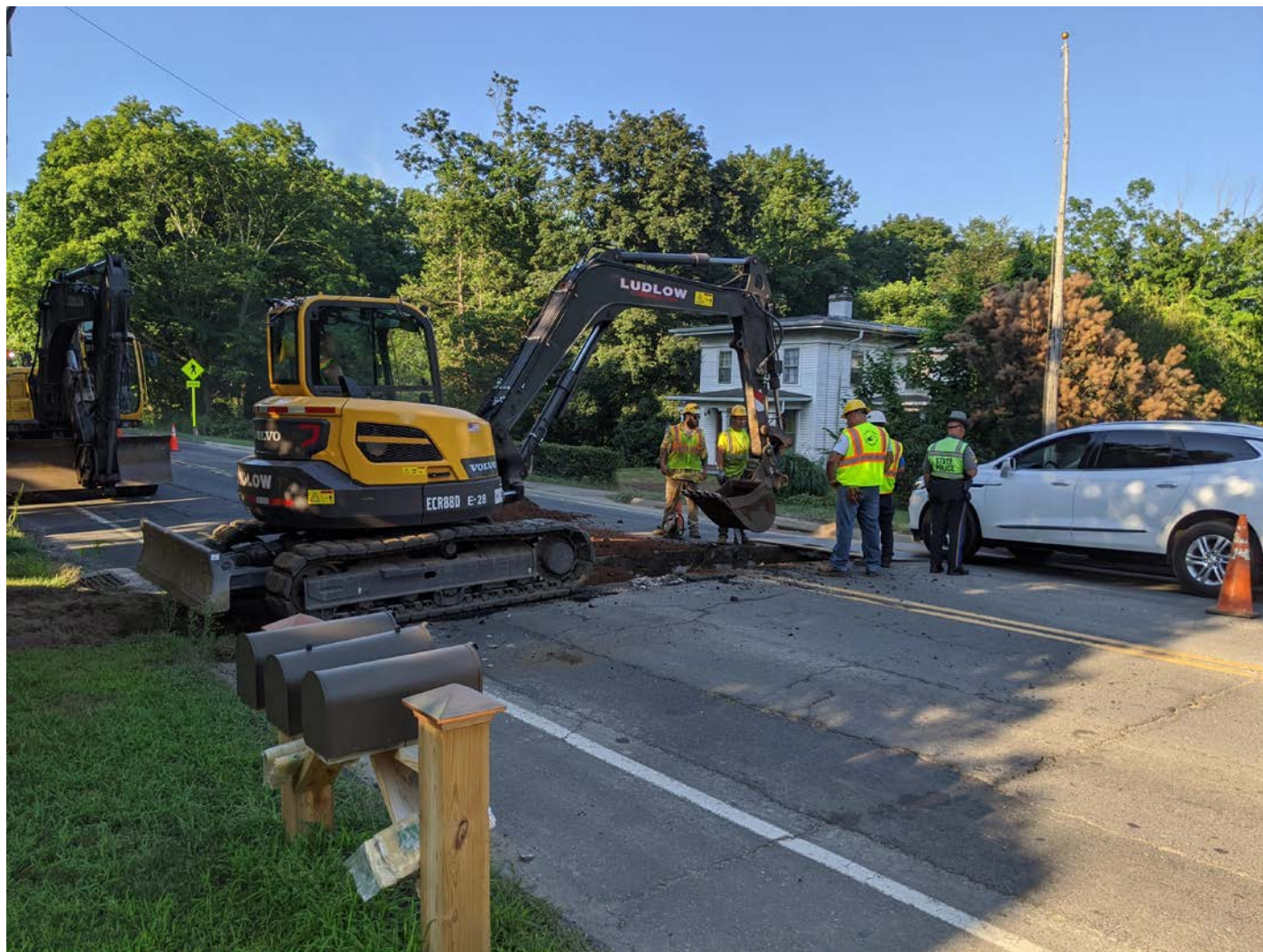
Picture 4: Ludlow construction digging a water service trench on Main Street, Main Street, Station 179+50. View to the southwest.
