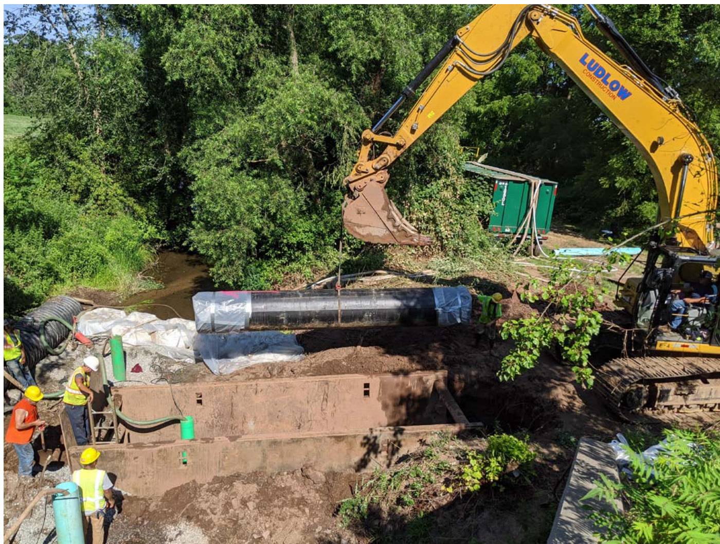
Picture 3: Ludlow construction installing 20' long 36" diameter casing into the stream bed excavation, Maple Avenue, Station 905+00. View to the west.
