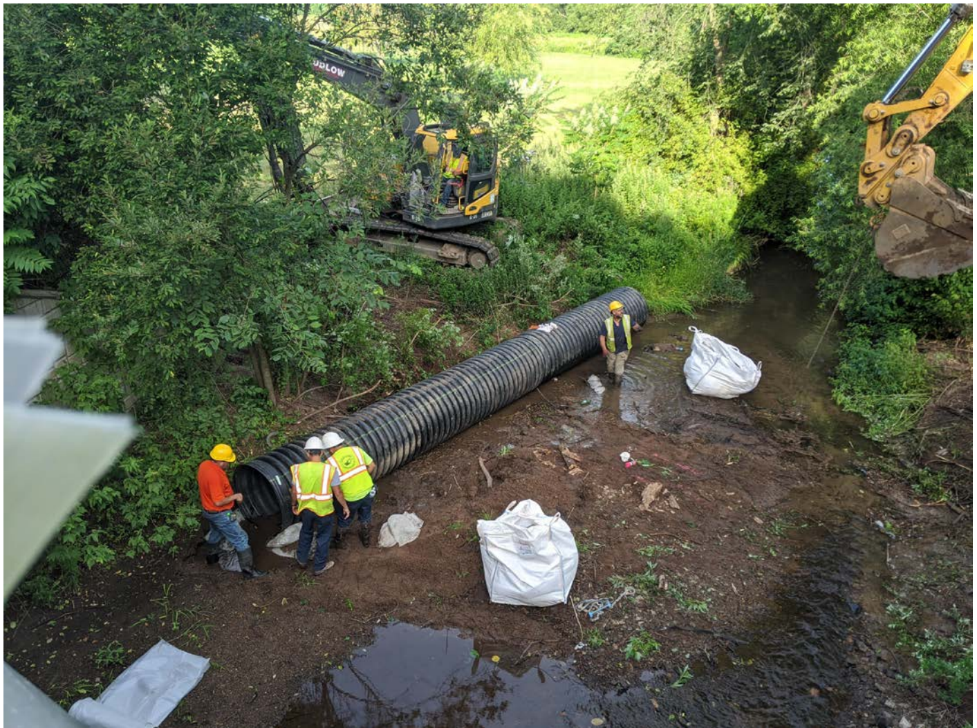
Picture 4: Ludlow construction installing sandbags and corrugated piping in the stream bed, Maple Avenue, Station 905. View to the west.
