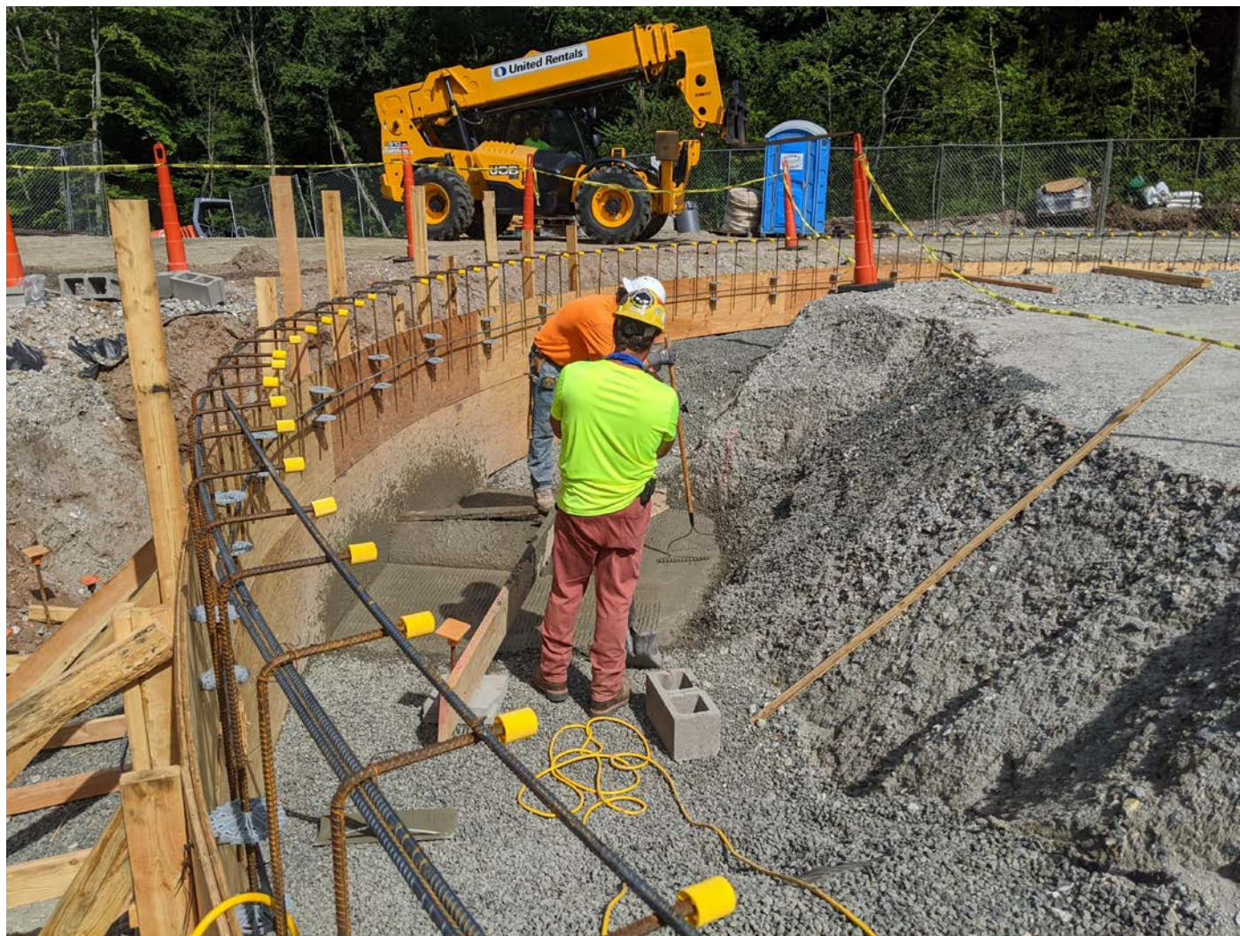
Picture 7: DN Tanks placing concrete around a pipe for the water tank, Shared Access Driveway. View to the west.
