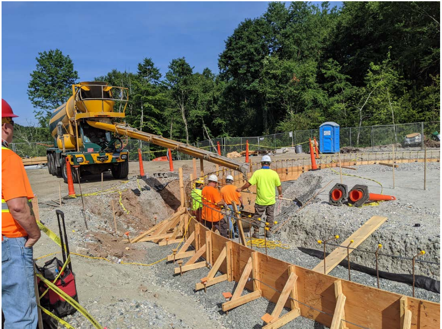
Picture 6: DN Tanks placing concrete around a pipe for the water tank, Shared Access Driveway. View to the west.
