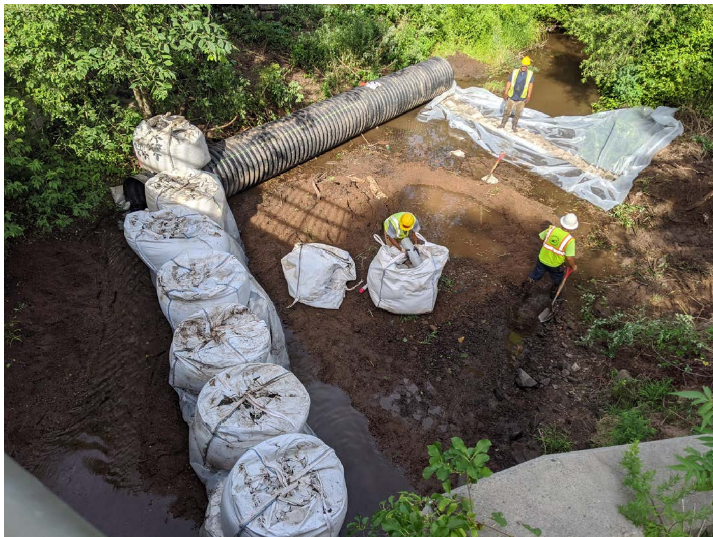
Picture 5: Ludlow construction installing sandbags and corrugated piping in the stream bed, Maple Avenue, Station 905. View to the west.
