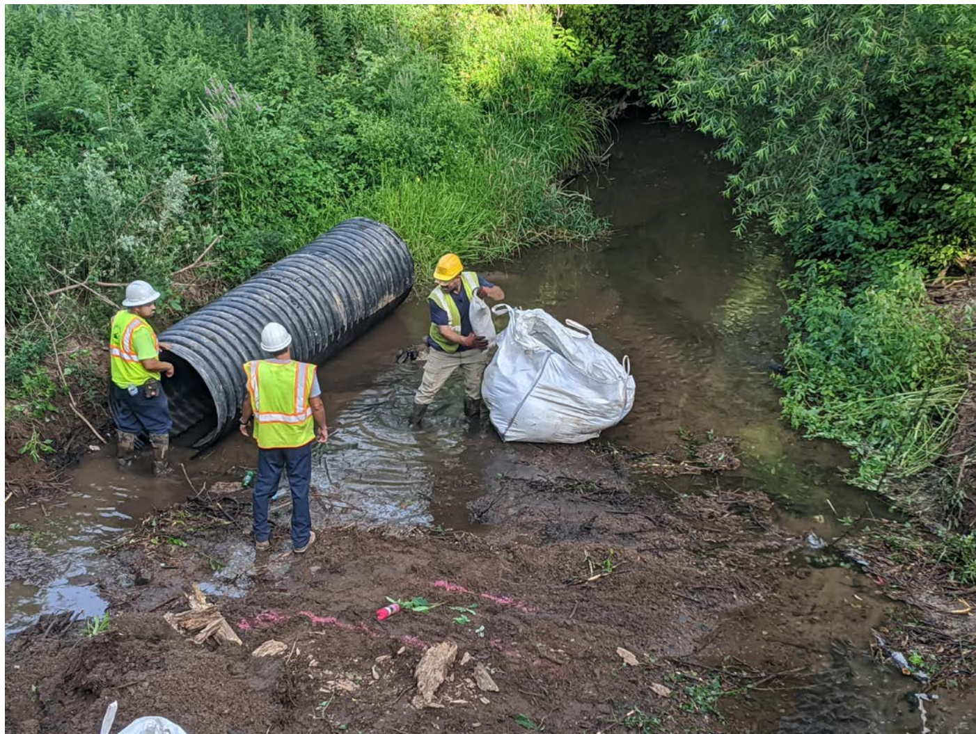
Picture 3: Ludlow construction installing sandbags and corrugated piping in the stream bed, Maple Avenue, Station 905. View to the west.
