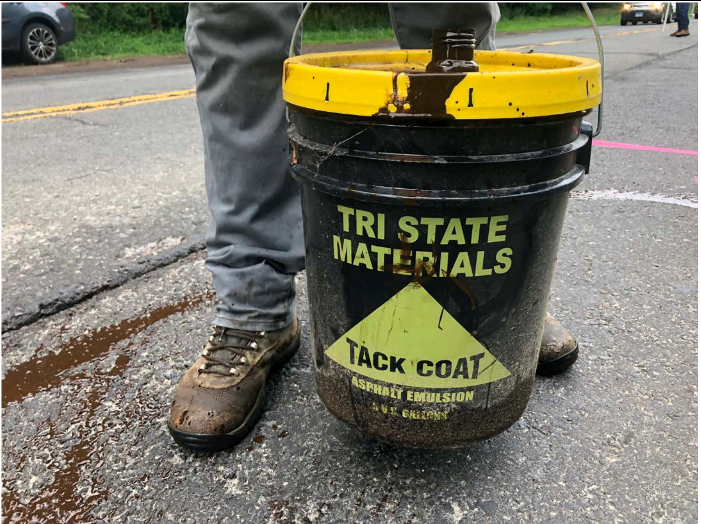
Picture 4: Tack coat applied prior to shim coating.
