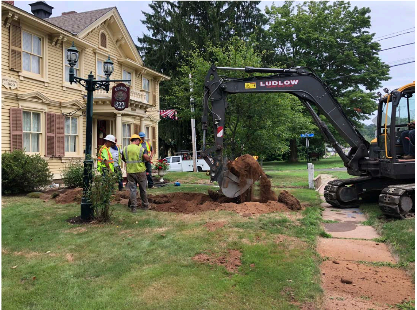
Picture 13: Ludlow installing a curb stop at 322 Main Street; Station 176+00. View to the north.
