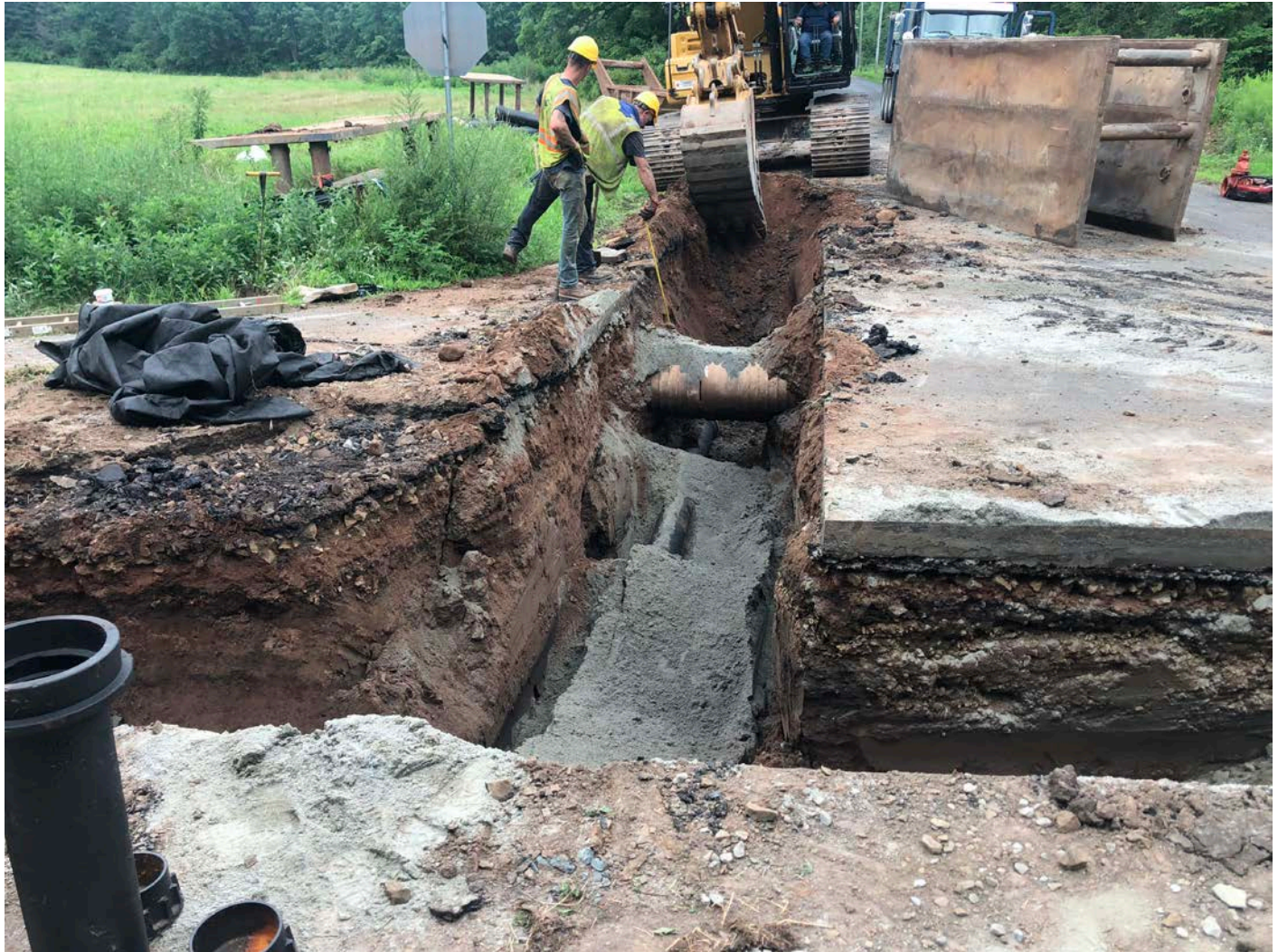
Picture 7: Ludlow installing an 8" water main stub for a hydrant on Brick Lane. View to the north.
