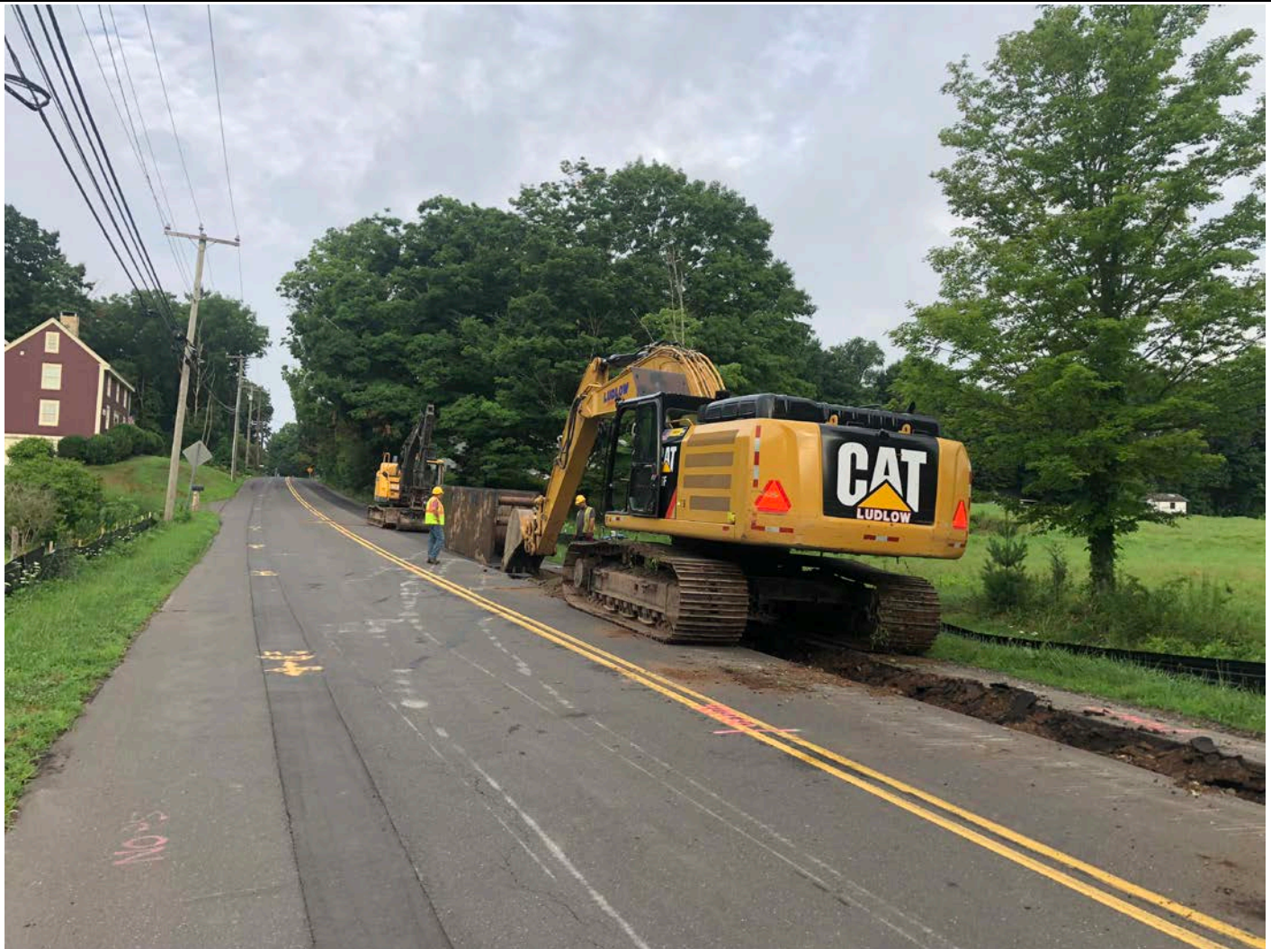
Picture 1: Ludlow beginning to excavate on Maiden Lane to begin installing 12" DIP. View to the west.
