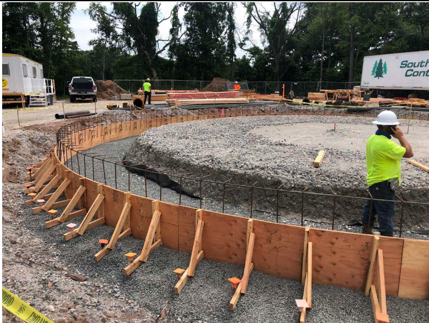
Picture 5: DN Tanks placing rebar on the top of the hook bars on the concrete form surrounding the water tank footprint to the east of the Shared Access Road. View to the east.
