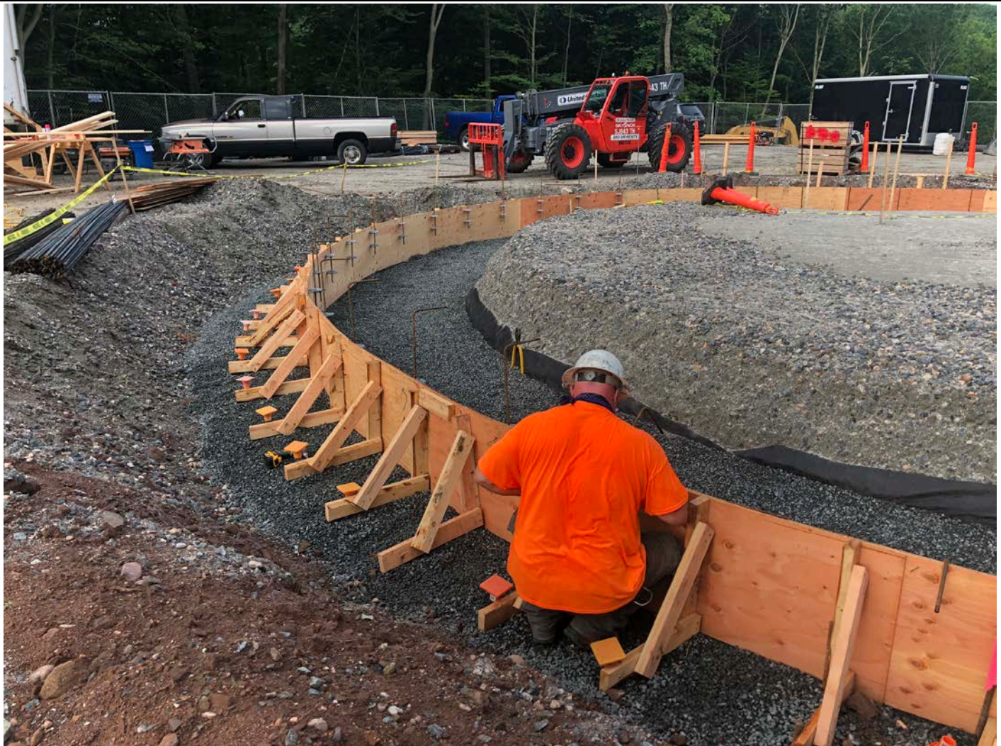
Picture 3: DN Tanks installing hook bars on the concrete form surrounding the water tank footprint to the east of the Shared Access Road. View to the east.
