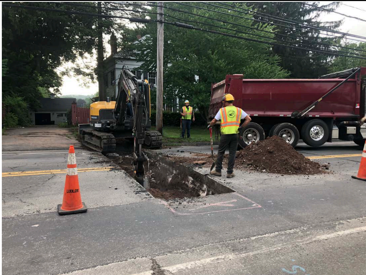
Picture 2: Ludlow excavating on the east side of Main Street at Station 177+10 for the installation of a curb stop at 313 Main Street, Durham. View to the east.
