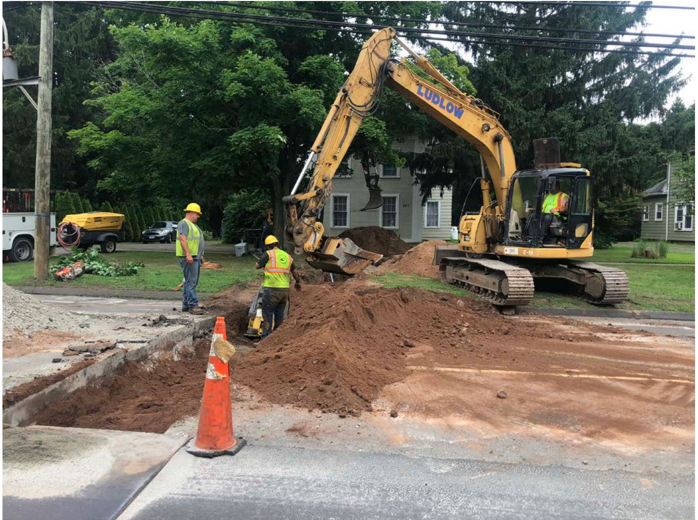
Picture 6: Ludlow excavating for the installation of a curb stop at Station 178+55. Main Street, Durham. View to the east.
