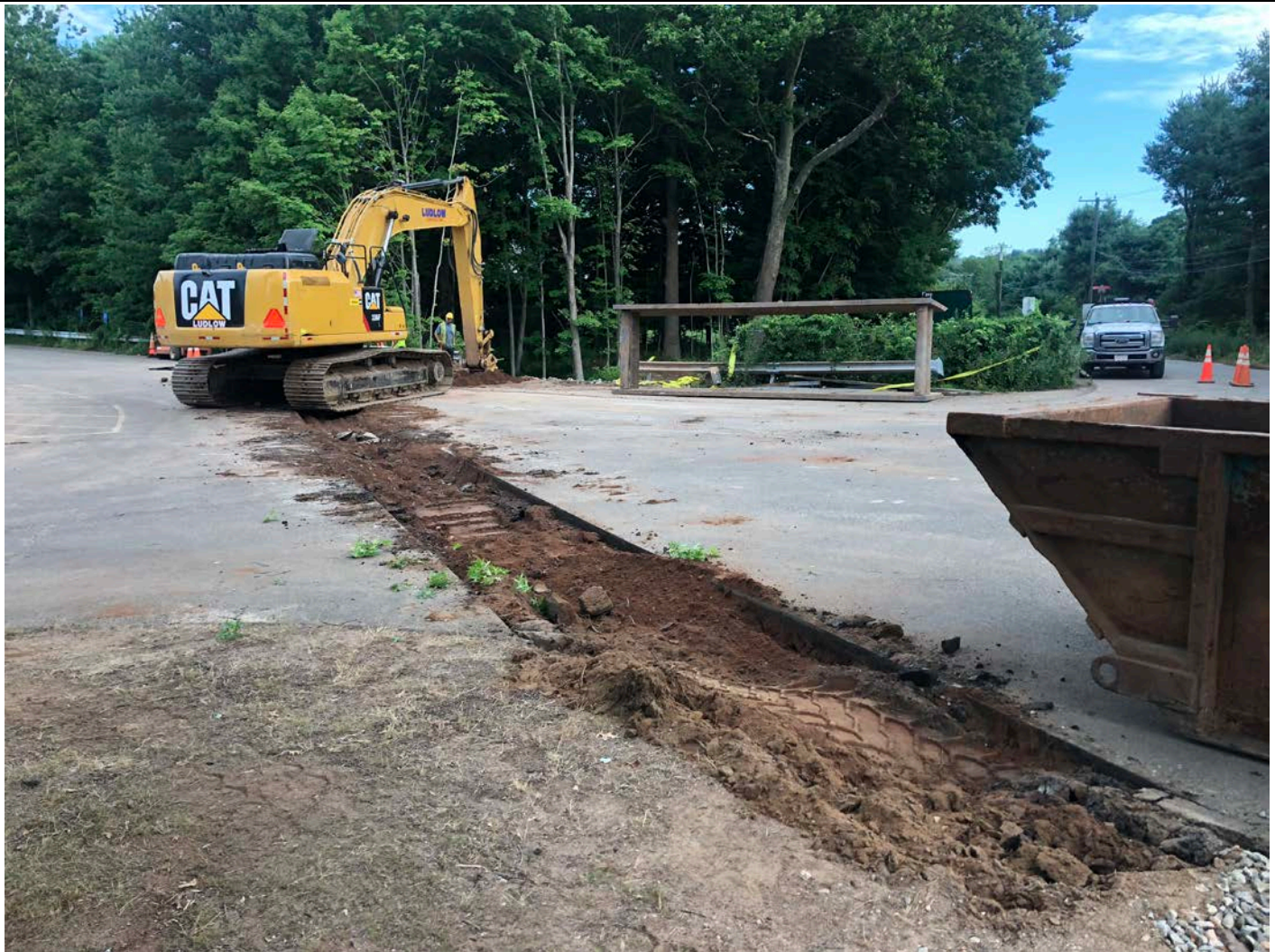
Picture 1: Ludlow peeling back asphalt before excavating trench south of Hersig Brook to install 12" DIP. Pickett Lane, Durham; Station ~531+00.
