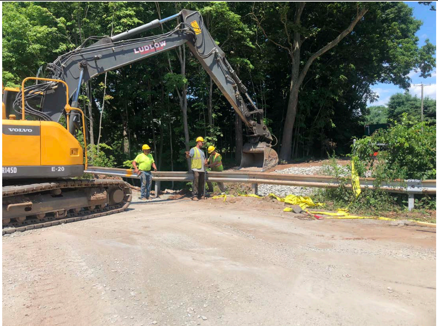
Picture 4: Ludlow replacing guard rail on the south side of the Hersig Brook stream crossing. Pickett Lane, Durham. View to the north.
