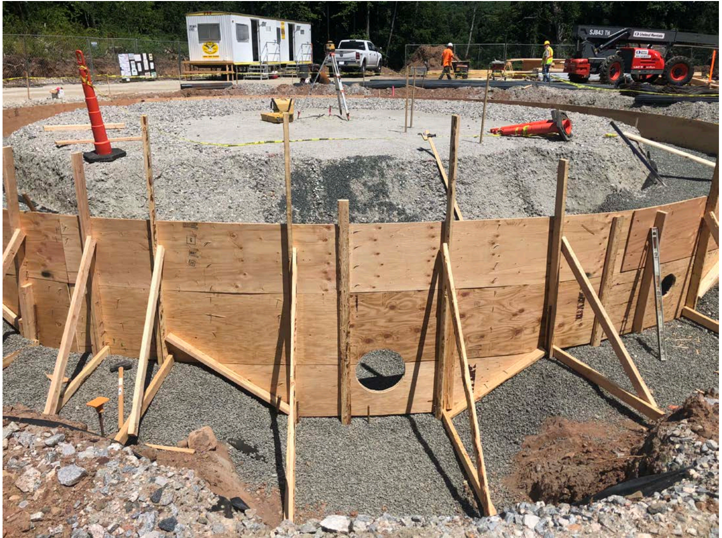
Picture 8: Concrete form being constructed by DN Tanks at the water tank footprint. Shared Access Driveway, Middletown. View to the east.
