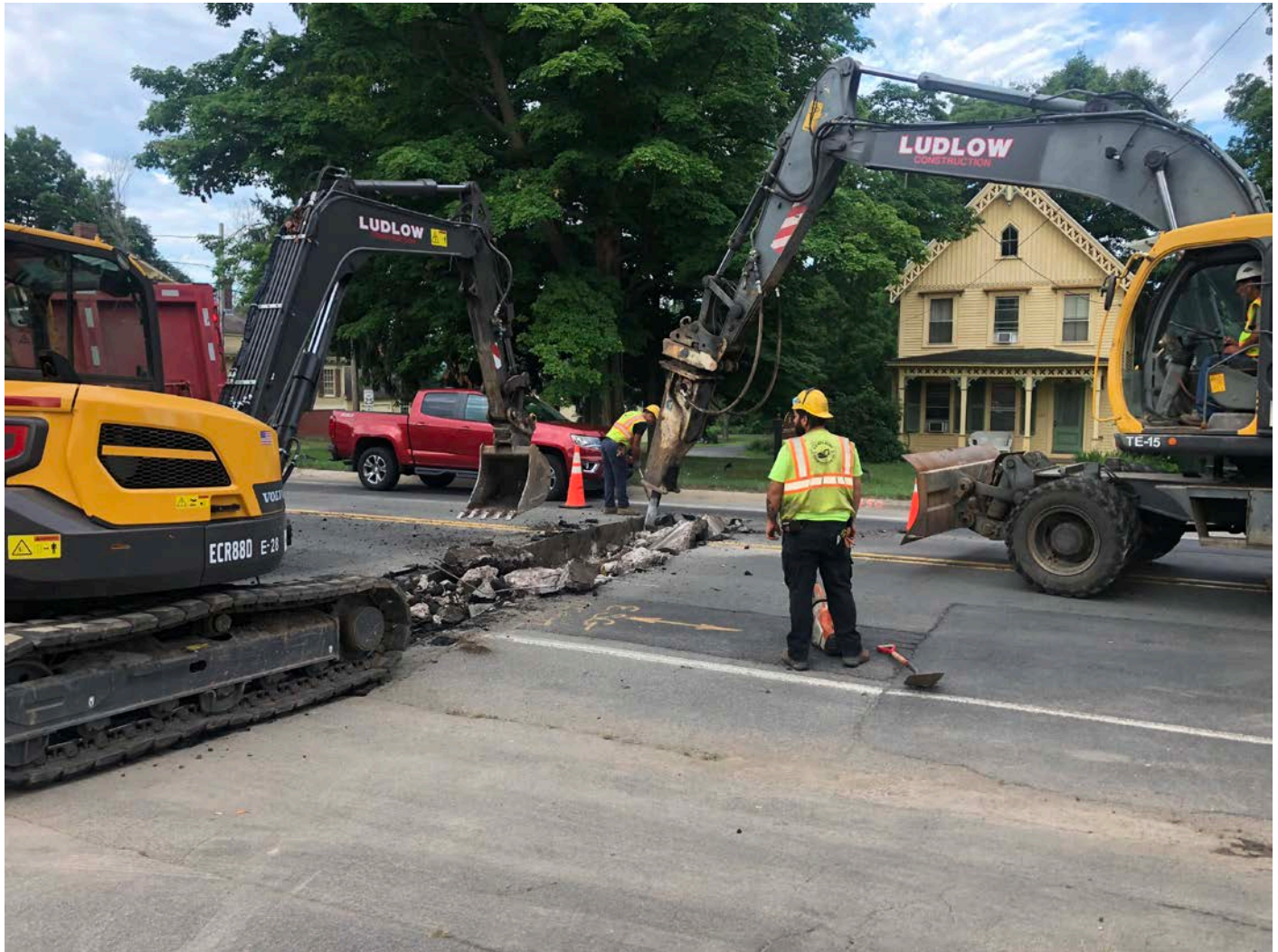
Picture 2: Ludlow beginning to excavate at Station 174+57 in order to install a curb stop for 327 Main Street, Durham. View to the west.
