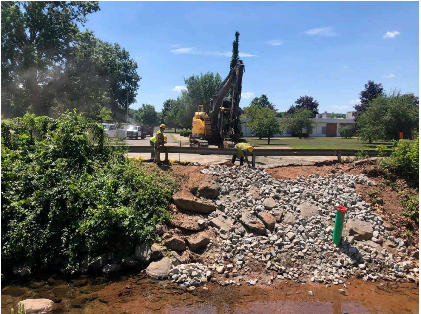
Picture 5: Ludlow replacing guard rail on the south side of the Hersig Brook stream crossing. The south bank of the brook has been backfilled with 6"+ rock. Pickett Lane, Durham. View to the south.
