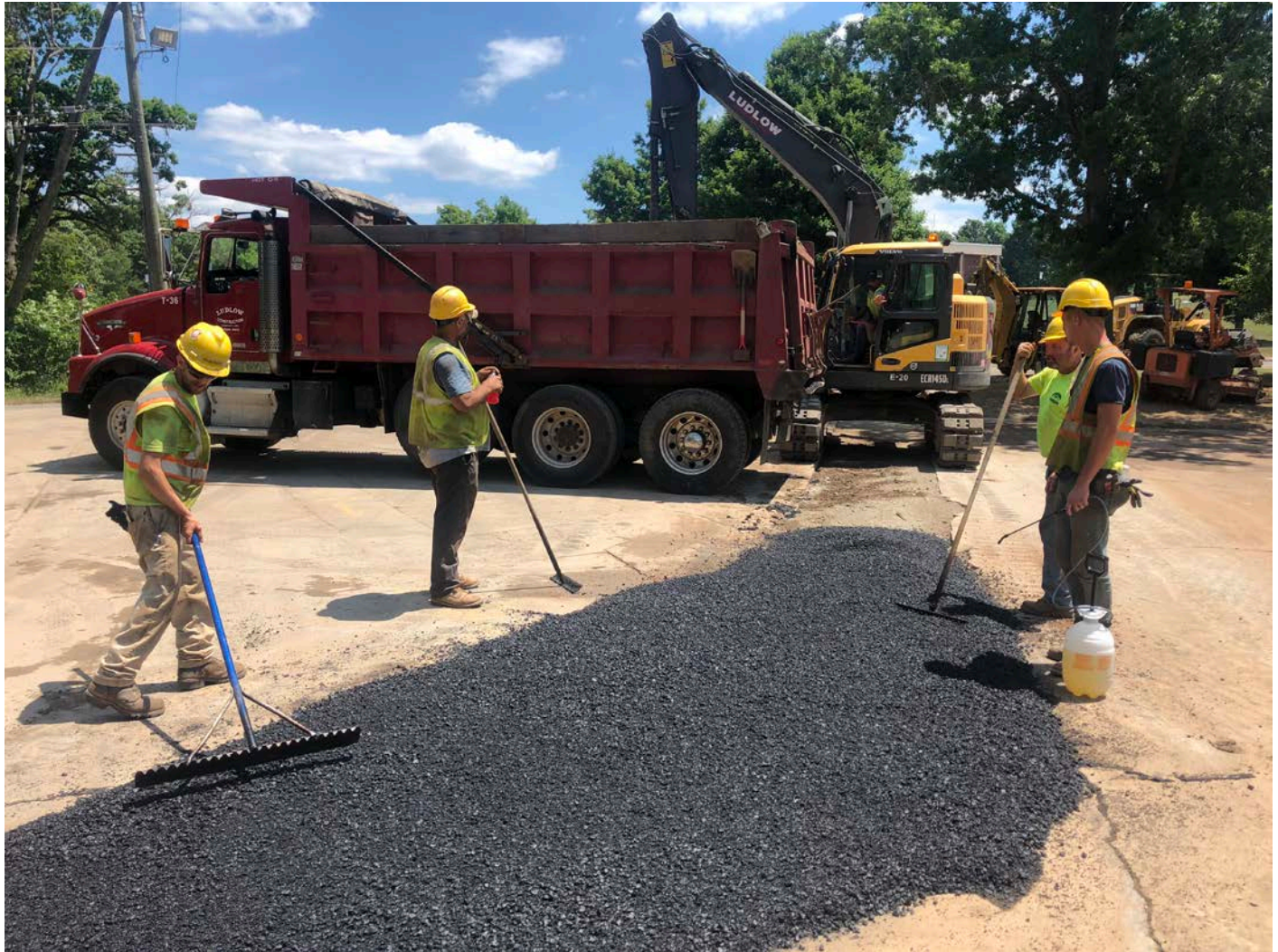
Picture 7: Ludlow placing hot patch over the trench where 12" DIP was placed today to the south of the Hersig Brook stream crossing. Pickett Lane, Durham. View to the southeast.
