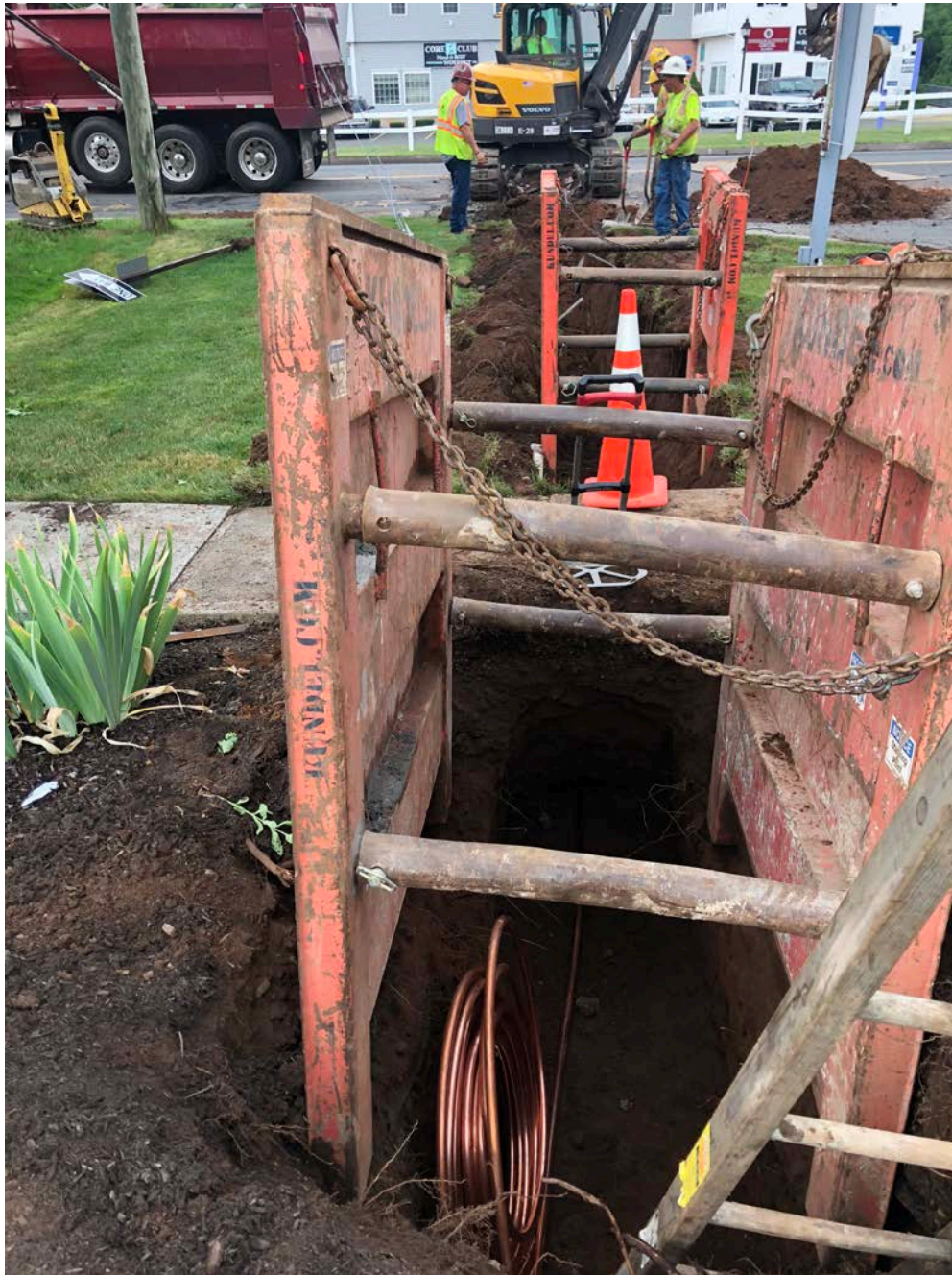
Picture 3: Curb stop installation underway at Station 171+22. Ludlow has 1" copper water line partially installed. View to the west. Main Street, Durham.
