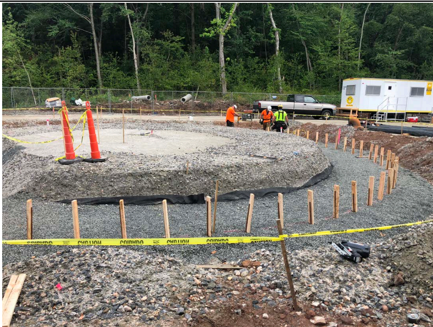
Picture 5: DN Tanks constructing cement form for the water tank frost wall. Shared Access Driveway, Middletown. View to the northeast.
