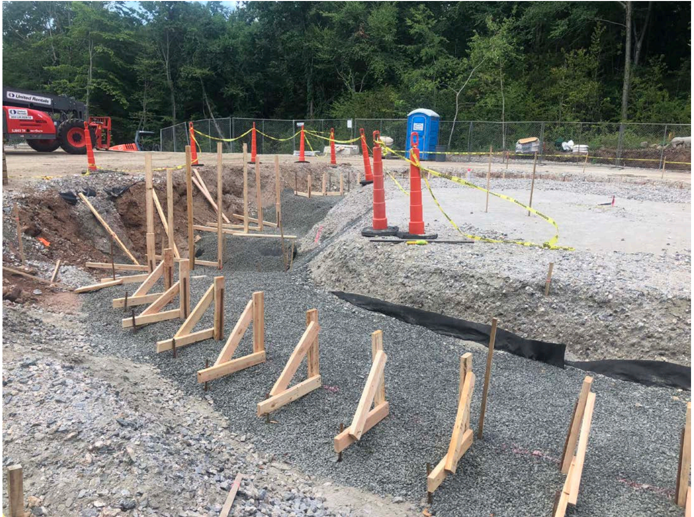
Picture 6: DN Tanks constructing cement form for the water tank frost wall. Shared Access Driveway, Middletown. View to the north.
