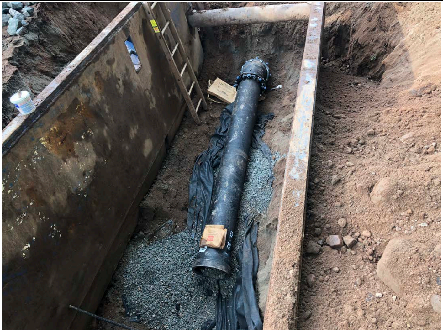
Picture 1: 9' section of 12" DIP and 45° bend that Ludlow installed on the north side of the Hersig Brook stream crossing. Pickett Lane, Durham; Station ~532+00.
