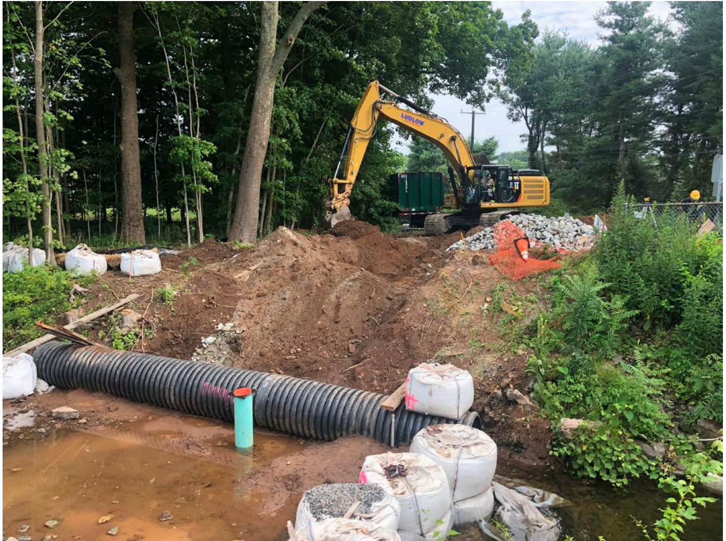
Picture 7: Ludlow backfilling trench on the north bank of Hersig Brook after the installation of 12" DIP. Pickett Lane, Durham; Station ~532+00. View to the northeast.
