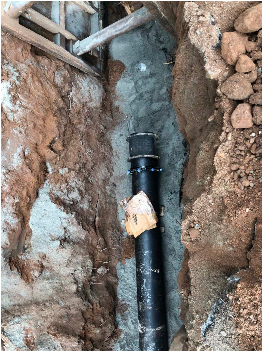
Picture 2: 20' section of 12" DIP and a female-female 12" DIP sleeve that Ludlow installed on the north side of the Hersig Brook stream crossing. Pickett Lane, Durham; Station ~532+00.
