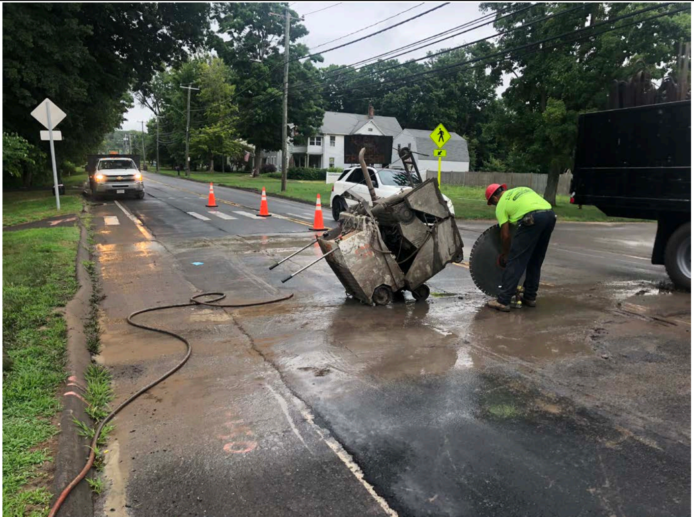
Picture 2: Ludlow preparing to saw cut pavement on Main Street, Durham. View to the north.
