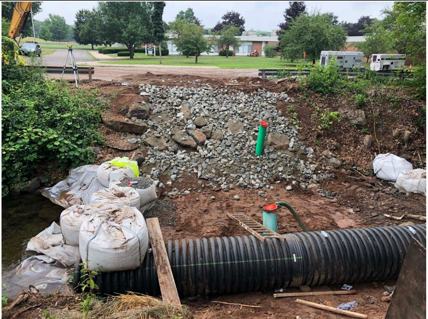
Picture 5: South bank of Hersig Brook after Ludlow placed riprap. View to the south. Station ~532+00, Pickett Lane, Durham.
