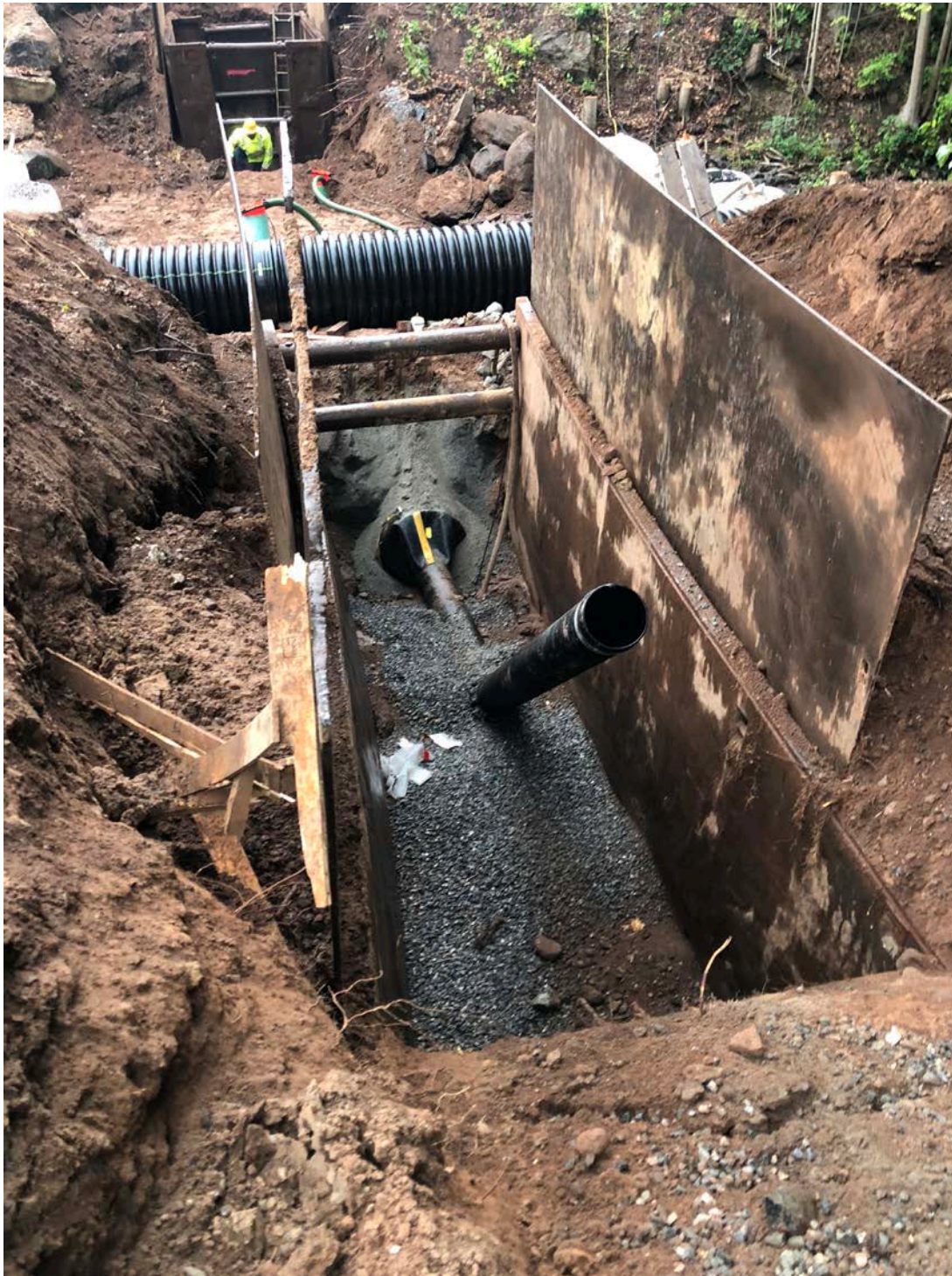
Picture 1: 12" DIP and 45° bend that Ludlow installed on the north side of the Hersig Brook stream crossing yesterday. Pickett Lane, Durham; Station ~532+00. View to the south.
