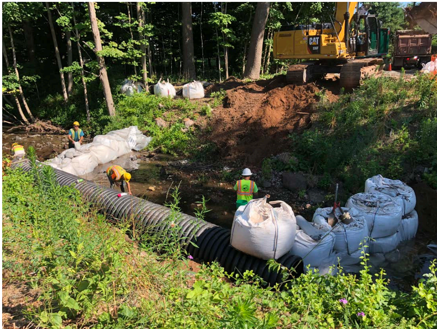
Picture 2: Ludlow placing large and small sandbags downstream of the Hersig Brook stream crossing work zone. Pickett Lane, Durham. Station ~532+00. View to the northwest.
