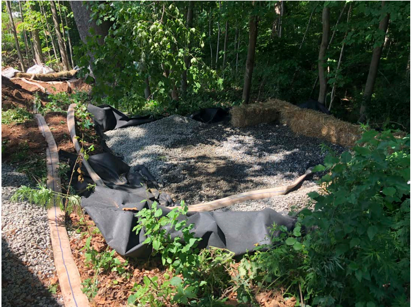
Picture 4: One of two filter beds Ludlow constructed on the north side of Hersig Brook. View is to the west. Pickett Lane, Durham. Station ~532+00.
