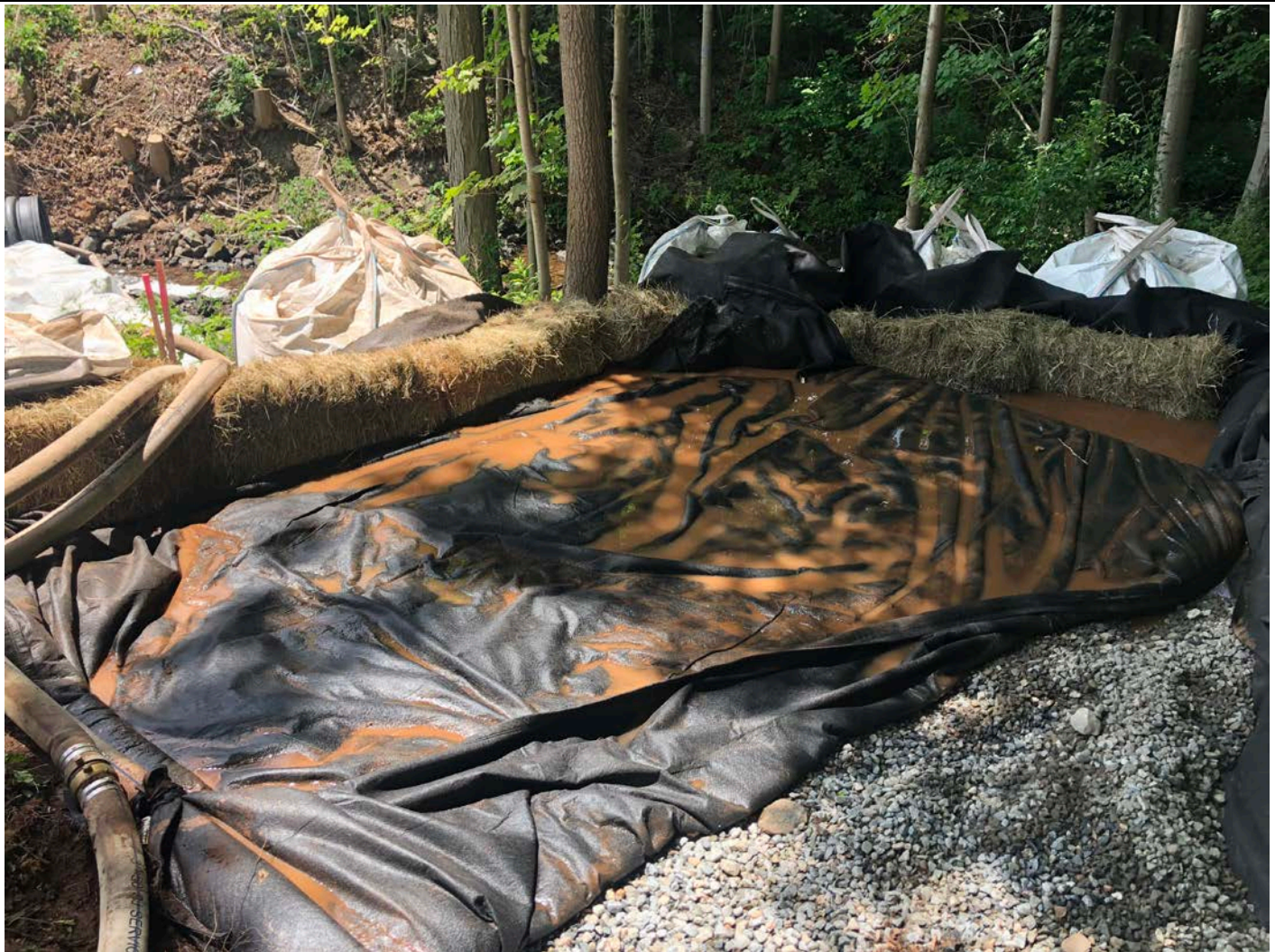
Picture 6: The filter bed Ludlow constructed closest to the stream bank of Hersig Brook. View is to the northwest. Pickett Lane, Durham. Station ~532+00.
