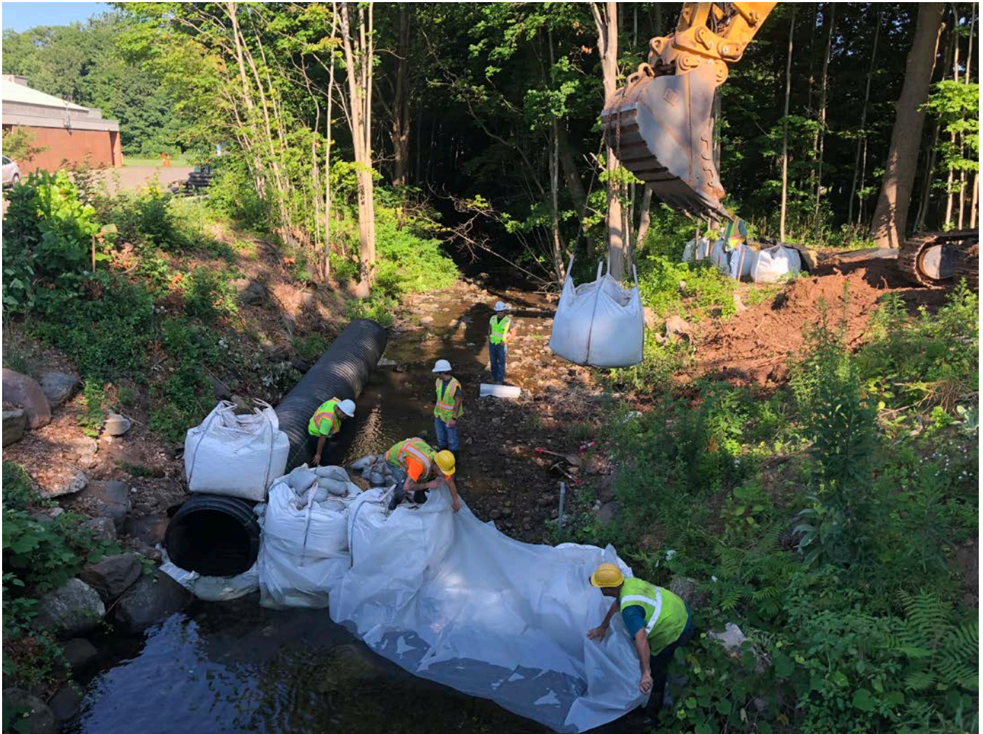
Picture 1: Ludlow placing large and small sandbags upstream of the Hersig Brook stream crossing work zone to direct stream flow into the 40" plastic corrugated flow bypass pipe placed on the south shore of the brook. View is to the west. Pickett Lane, Durham. Station ~532+00.
