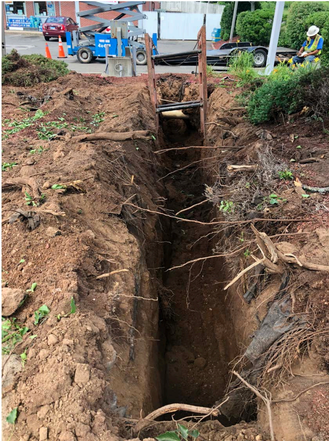
Picture 9: Partially excavated curb stop trench at Station 162+73, 384 Main Street, Durham. View to the west.
