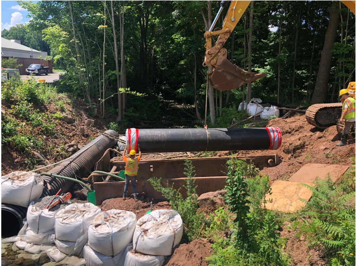
Picture 8: Ludlow placing 36" pipe conduit in the bed of Hersig Brook. View to the west. Pickett Lane, Durham. Station ~532+00.
