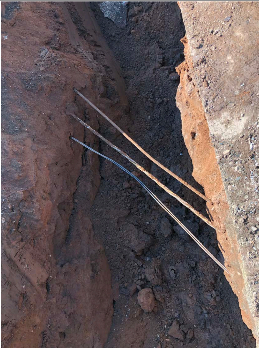
Picture 3: Subsurface utilities daylighted by Ludlow as they excavated near Station 512+00 while installing 12" DIP. Pickett Lane, Durham.
