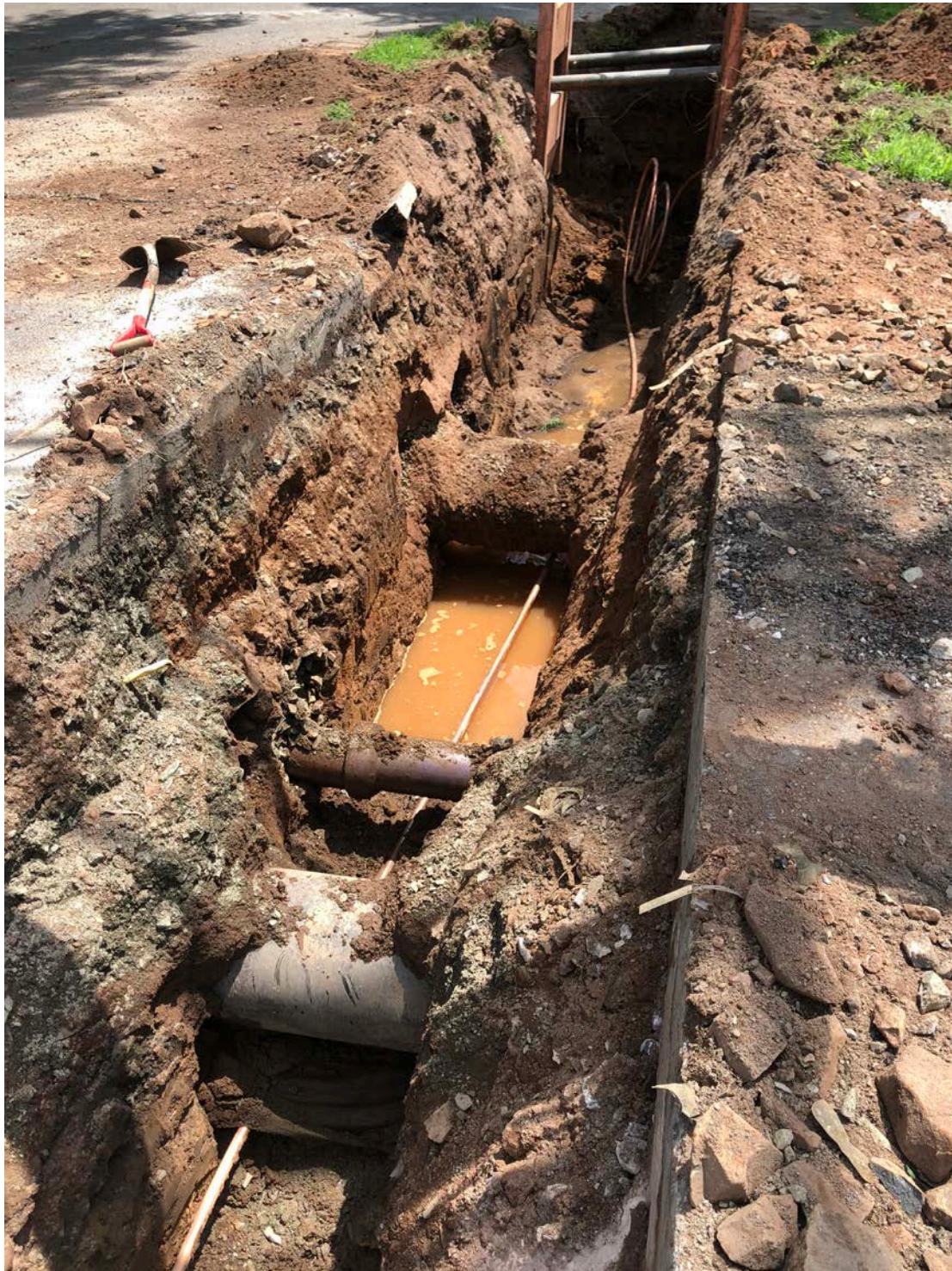
Picture 5: Water observed in trench as Ludlow installed a corporation stop and a curb stop at Station 163+01. Main Street, Durham. View to the east.
