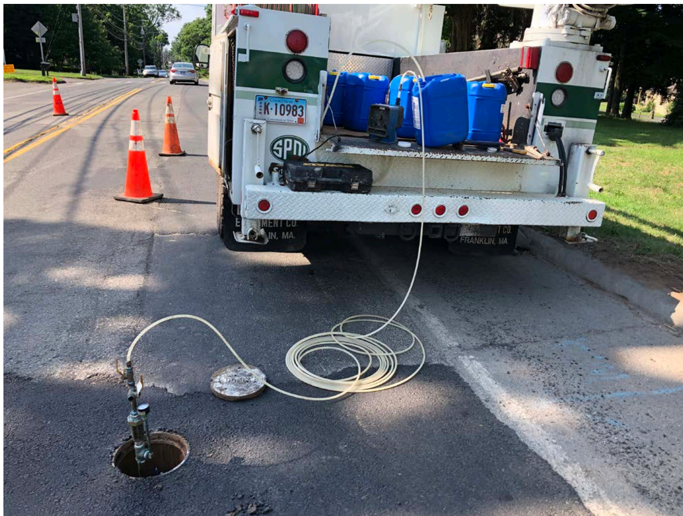
Picture 4: The intersection of Marina Place and Main Street where a 12.5% solution of sodium hypochlorite is introduced into the Main Street water line as part of chlorination activities. View to the south.
