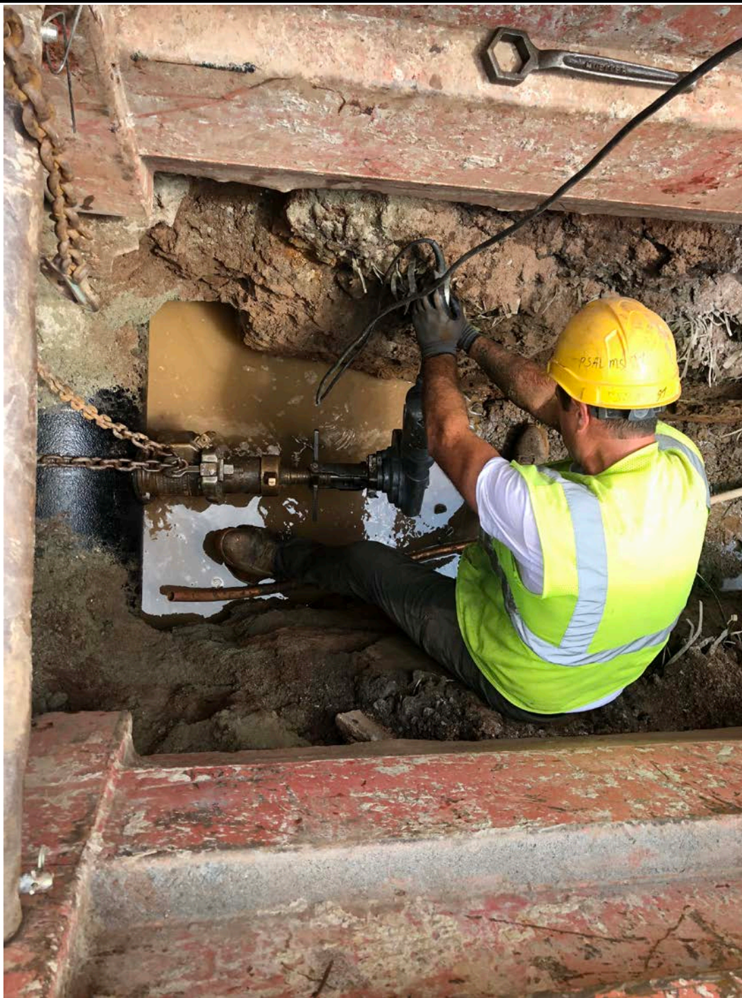
Picture 6: Ludlow tapping the main water line to install a corporation stop at Station 163+01.
