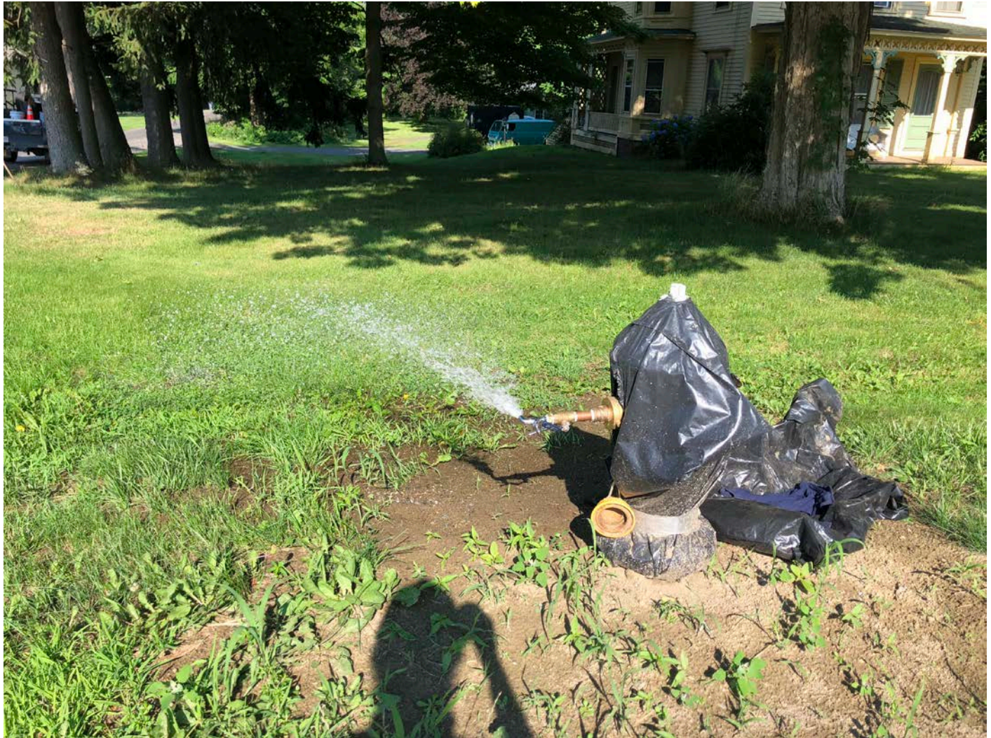
Picture 2: Ludlow venting the hydrant at the intersection of Talcott Lane and Main Street, Durham, as part of water line chlorination activities. View to the northwest.
