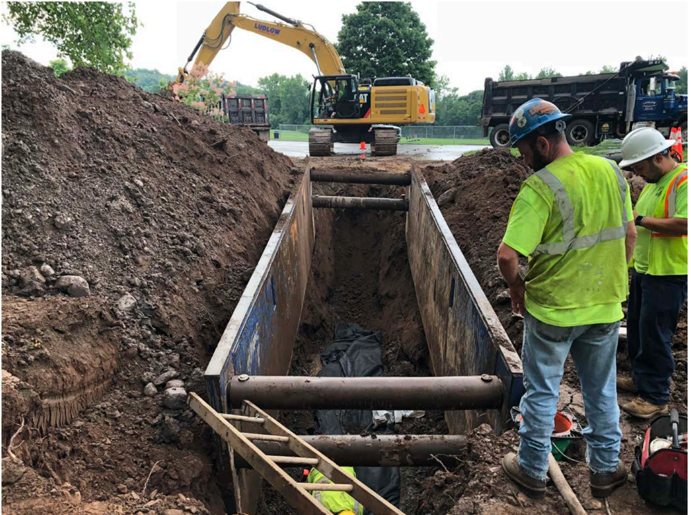
Picture 1: Ludlow installing 12" DIP to the east of Allyn Brook. They are placing the next 20' section in the direction of Pickett Lane, which can be seen in the background. View is to the southeast, looking towards Station 512+00.
