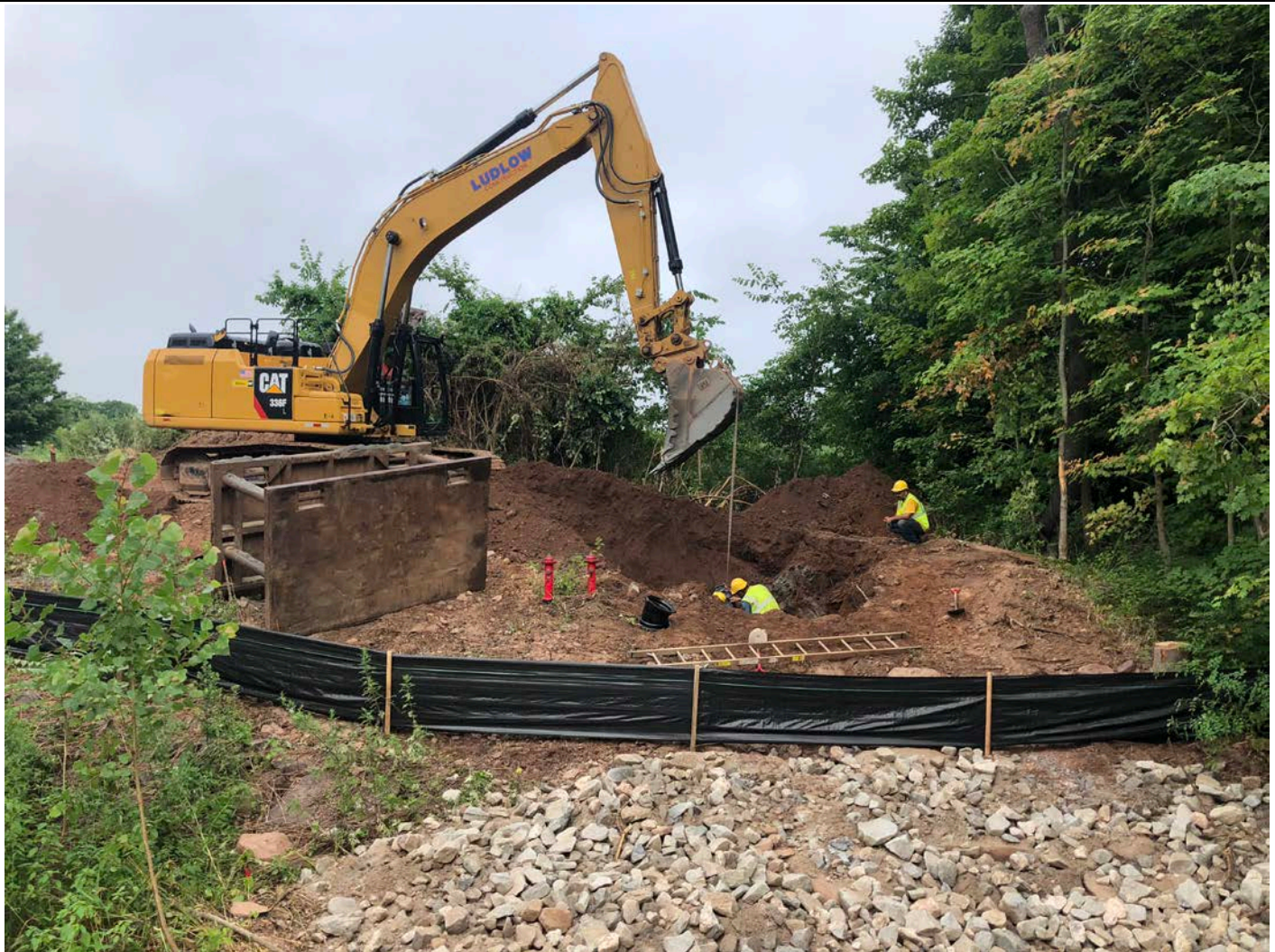
Picture 1: Ludlow installing 12" DIP to the west of Allyn Brook. Pickett Lane, Durham. View to the west.
