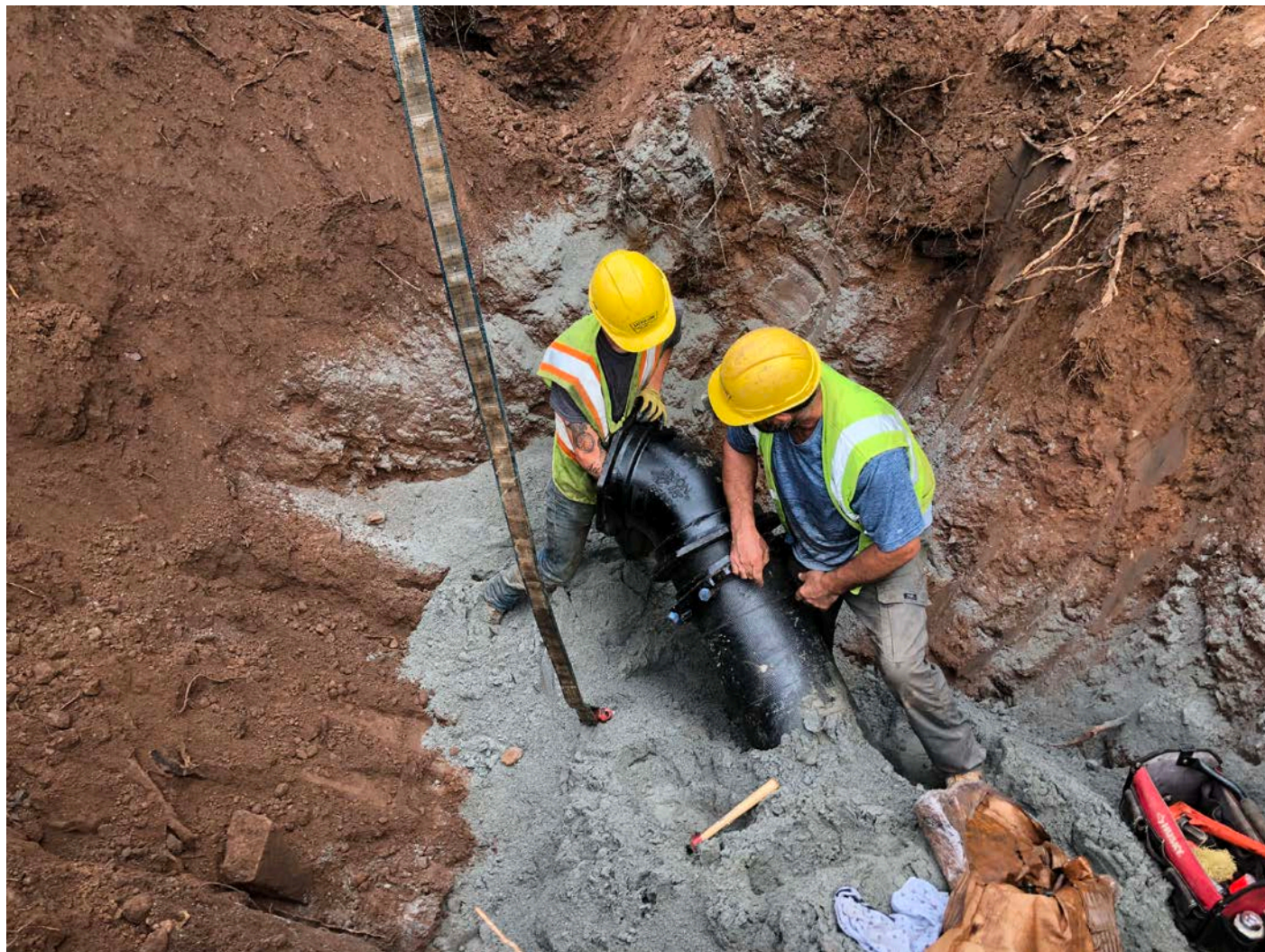
Picture 2: Ludlow installing 12" 45° bend to the west of Allyn Brook. Pickett Lane, Durham. View to the west.
