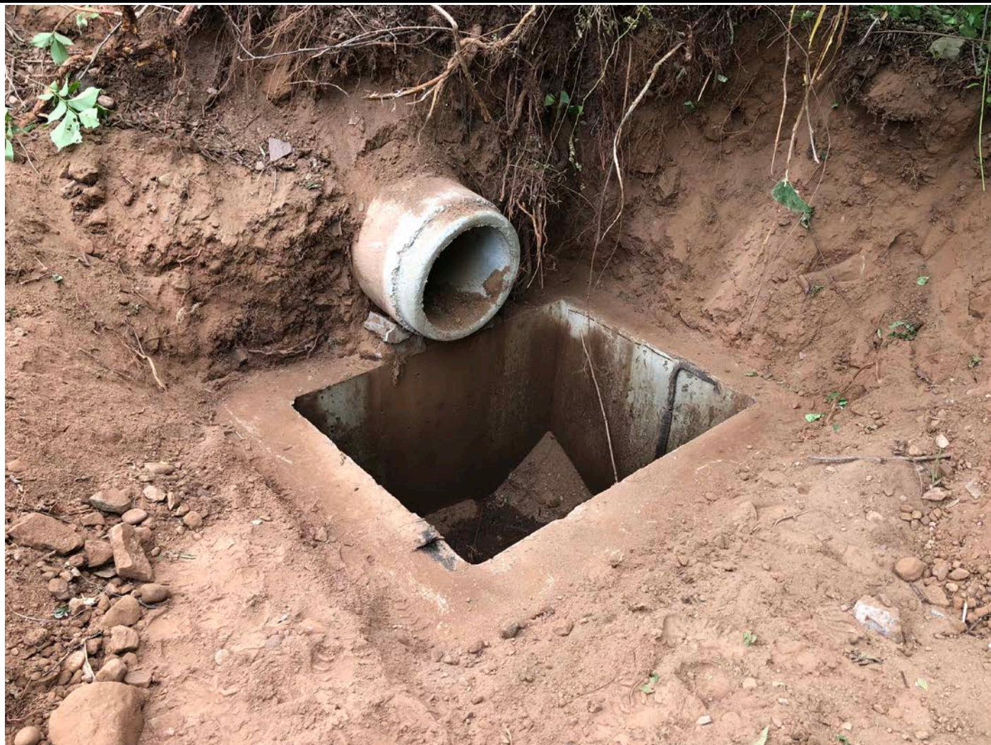
Picture 5: Existing storm drainage structures daylighted by Ludlow while working on the west bank of Allyn Brook. Ludlow accidentally broke the riser that was located here. View to the southwest. Pickett Lane, Durham.
