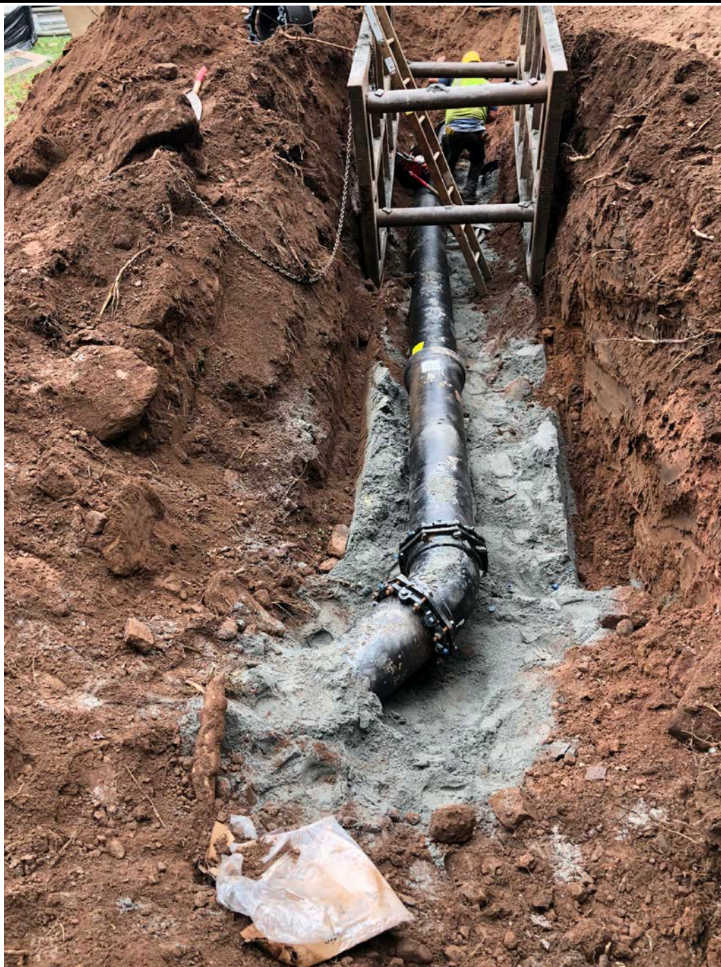
Picture 3: Ludlow installing 12" DIP to the west of Allyn Brook. Pickett Lane, Durham. View to the south.
