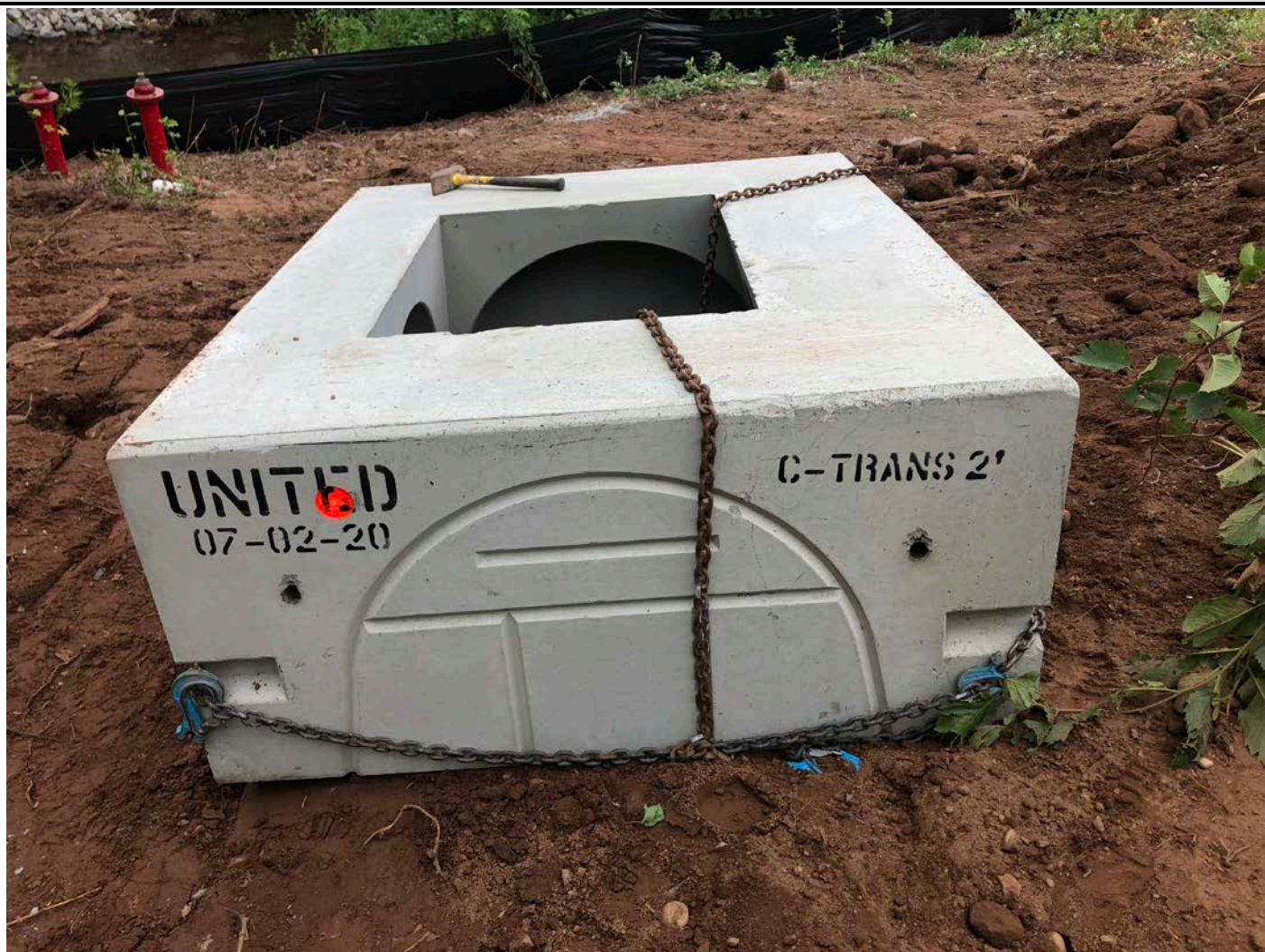
Picture 6: Riser that Ludlow is about to install to replace the one they accidentally broke yesterday on the west side of Allyn Brook.
