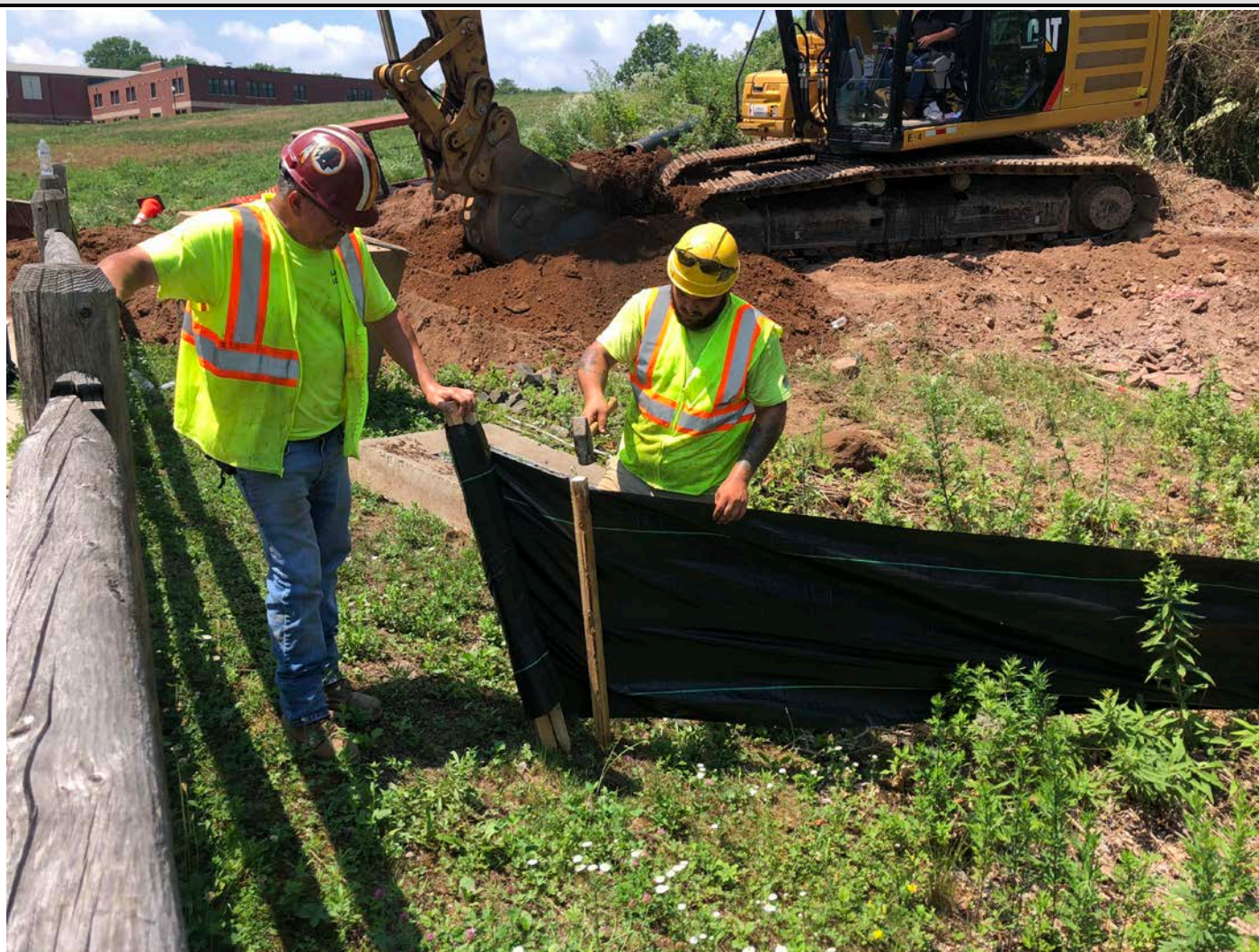
Picture 6: Ludlow installing silt fence on the west side of Allyn Brook. View to the west. Station ~509+50, Pickett Lane, Durham.
