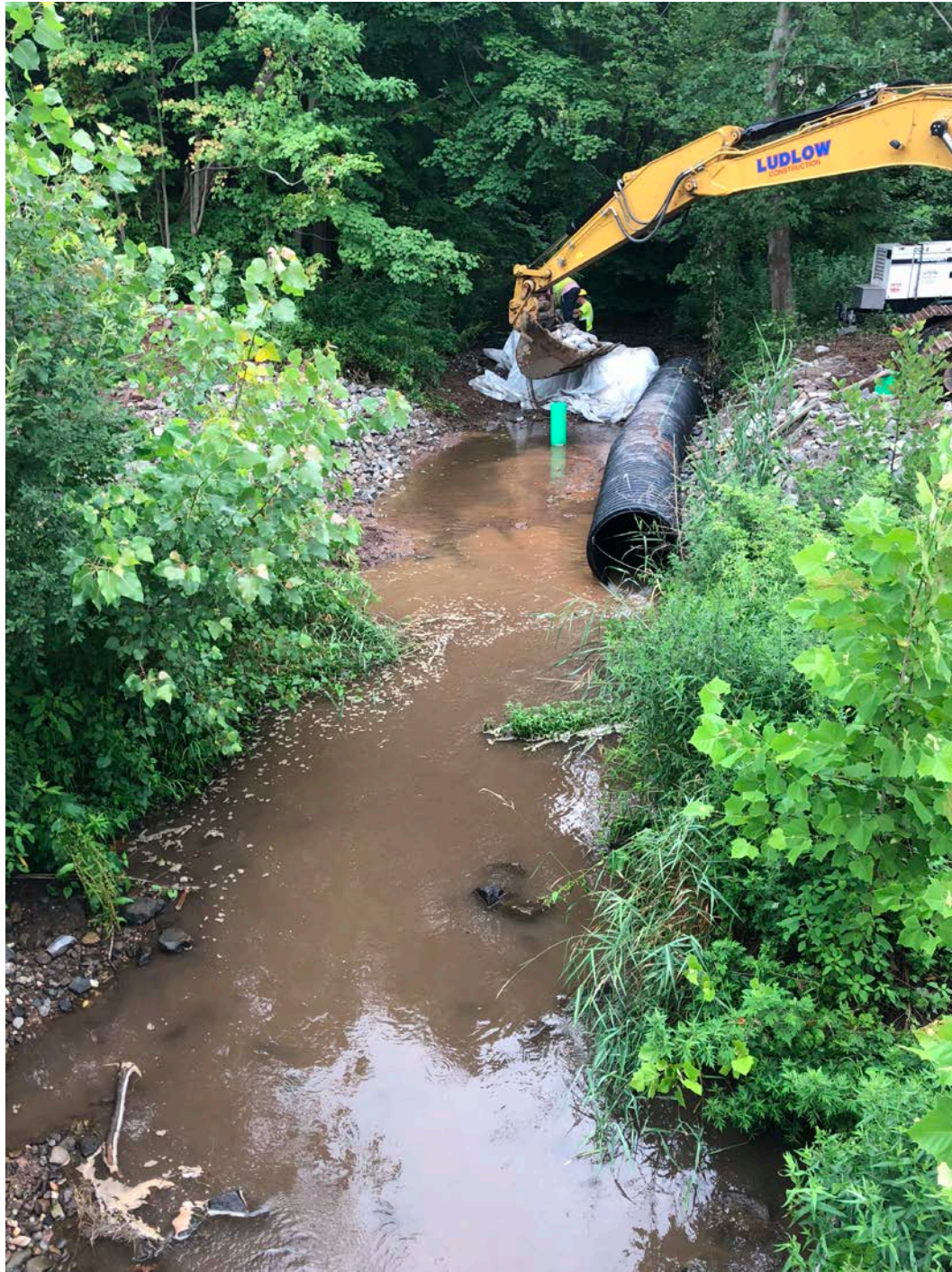
Picture 2: Ludlow removing upstream coffer dam of sandbags. Allyn Brook looking north. Pickett Lane, Durham.
