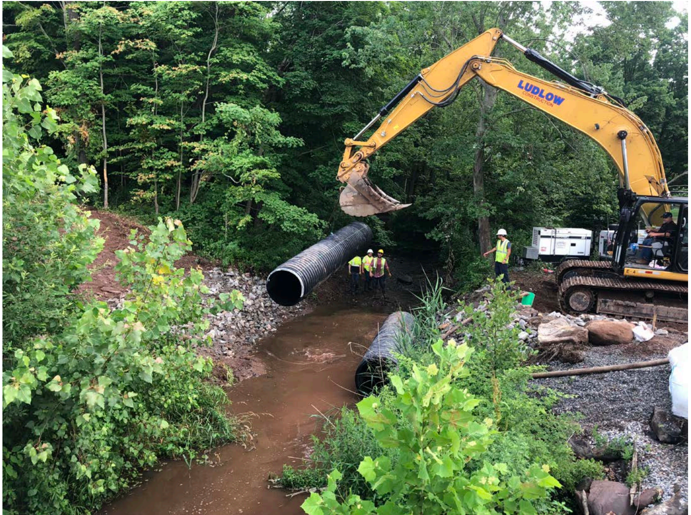
Picture 3: Ludlow removing stream bypass conduit. Allyn Brook, looking north. Station ~511+00, Pickett Lane, Durham.
