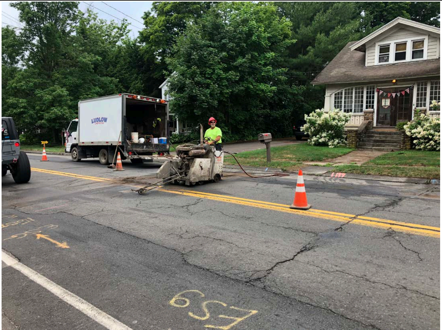
Picture 1: Ludlow saw cutting pavement on the southbound lane of Main Street, Durham. View to the southwest.
