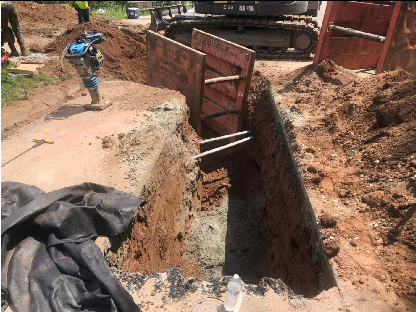
Picture 5: Ludlow about to place 12" DIP and a 45° bend at Station ~509+15. View to the northeast. Pickett Lane, Durham.
