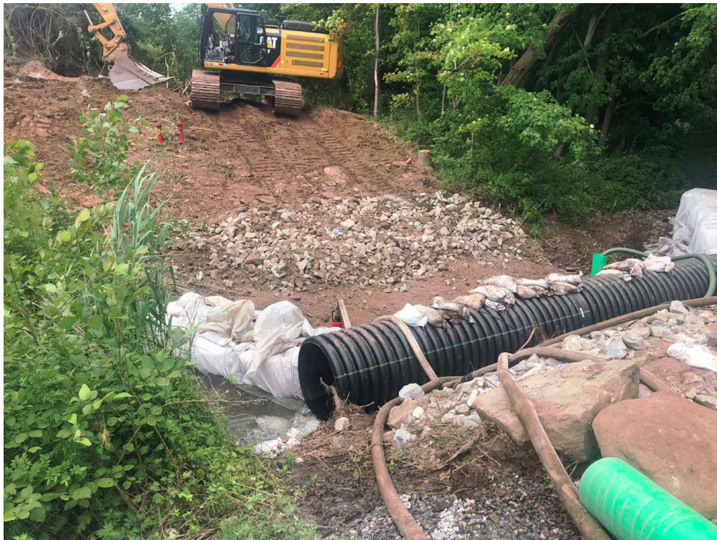
Picture 10: West bank of Allyn Brook after trench on the west slope was backfilled and riprap was placed along the shoreline. Station ~511+00, Pickett Lane, Durham. View to the west.
