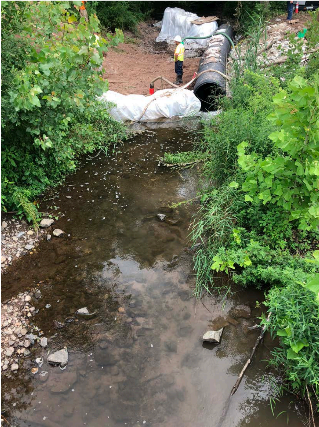
Picture 9: Minor turbidity observed downstream of ongoing stream crossing activities. Station ~511+00, Pickett Lane, Durham. View to the north.
