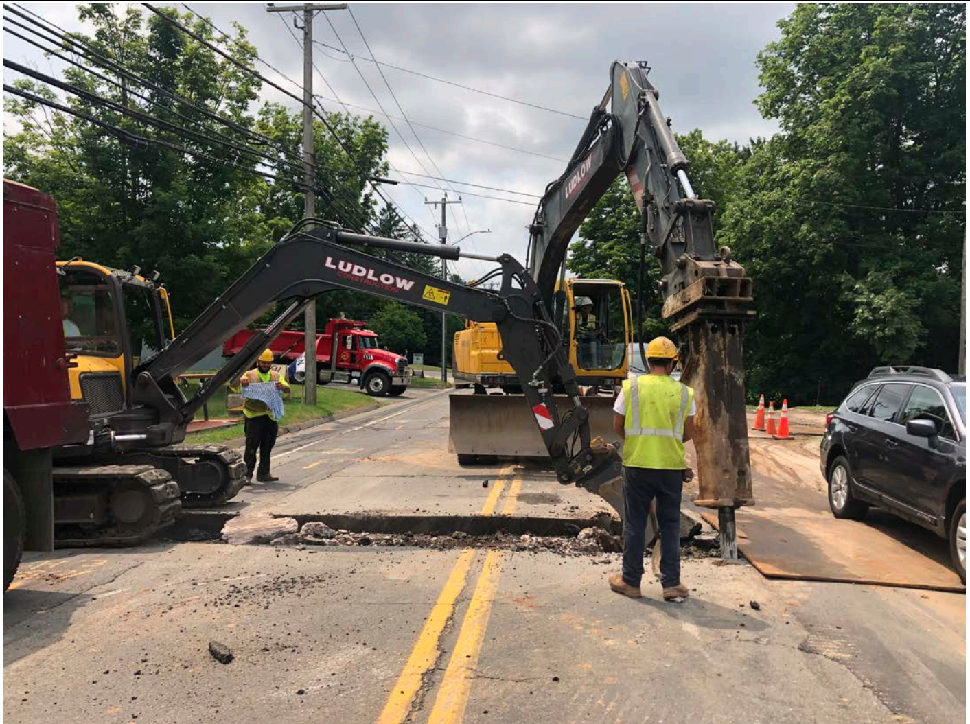
Picture 7: Ludlow beginning to excavate on the northbound lane of Main Street at Station 172+77 for the installation of a curb stop. View to the south.
