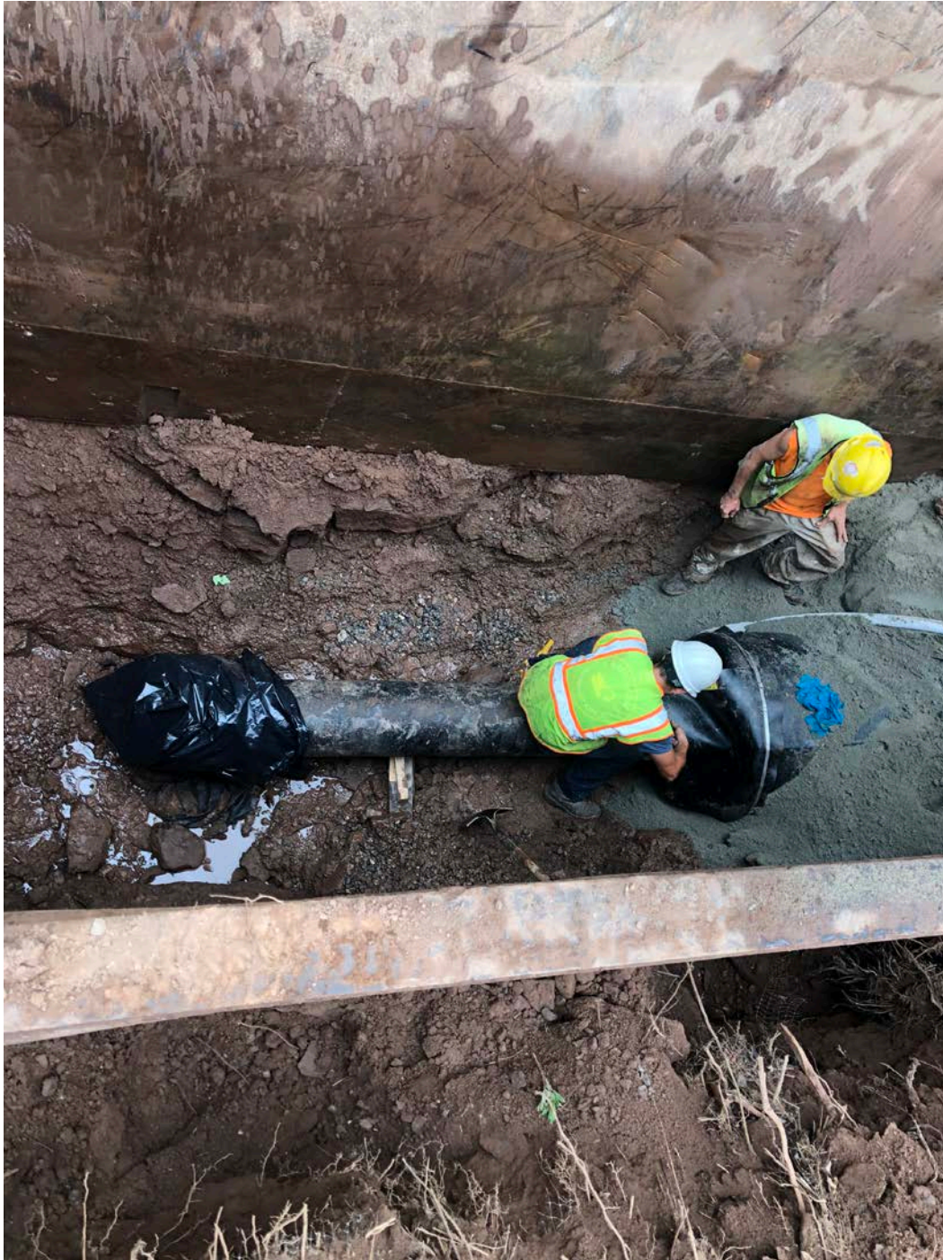
Picture 4: Ludlow placing an end seal of thick rubberized material over the junction between the 12" DIP and the 36" conduit to contain the sand they will blow into the interstitial space between the 12" DIP and the 36" conduit from the east side of Allyn Brook. Station ~511+00, Pickett Lane, Durham.
