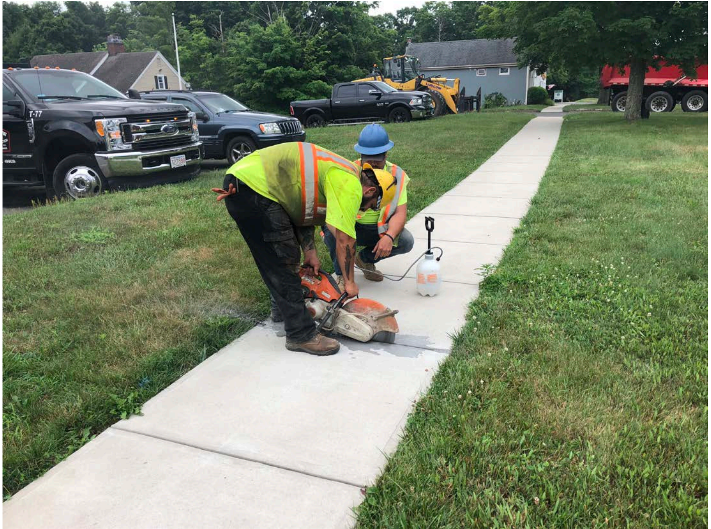
Picture 8: Ludlow saw cutting sidewalk to allow for the installation of a curb stop at Station 172+77. Main Street, Durham. View to the northwest.
