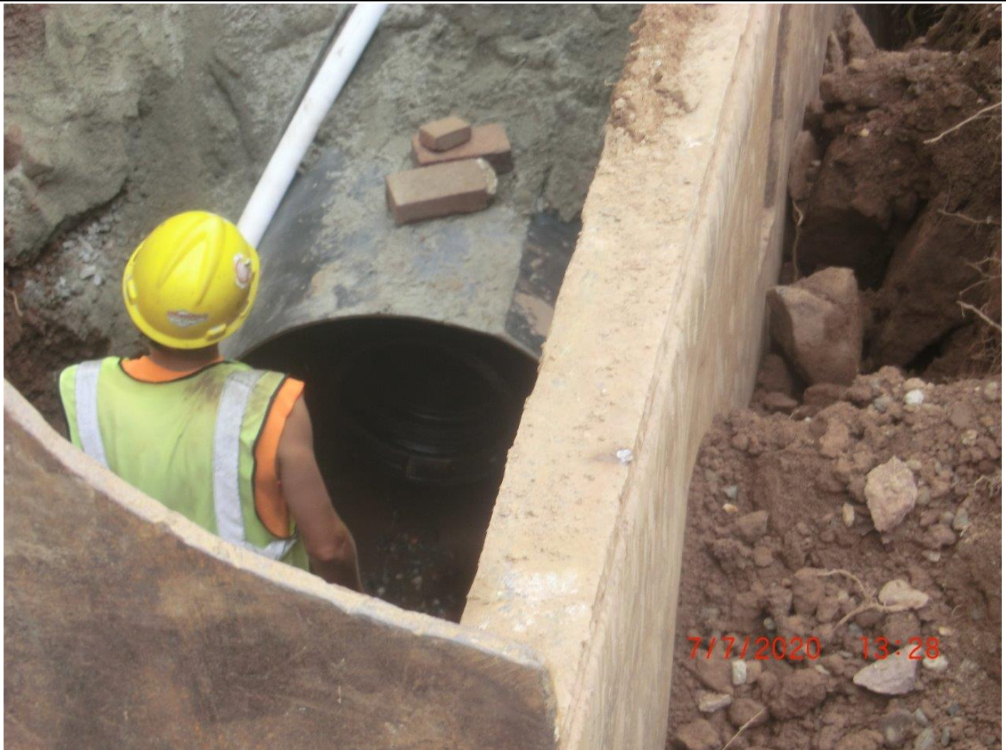
Picture 7: 36" conduit with 12" DIP placed inside of it. Station ~511+00, Pickett Lane, Durham. View to the east.
