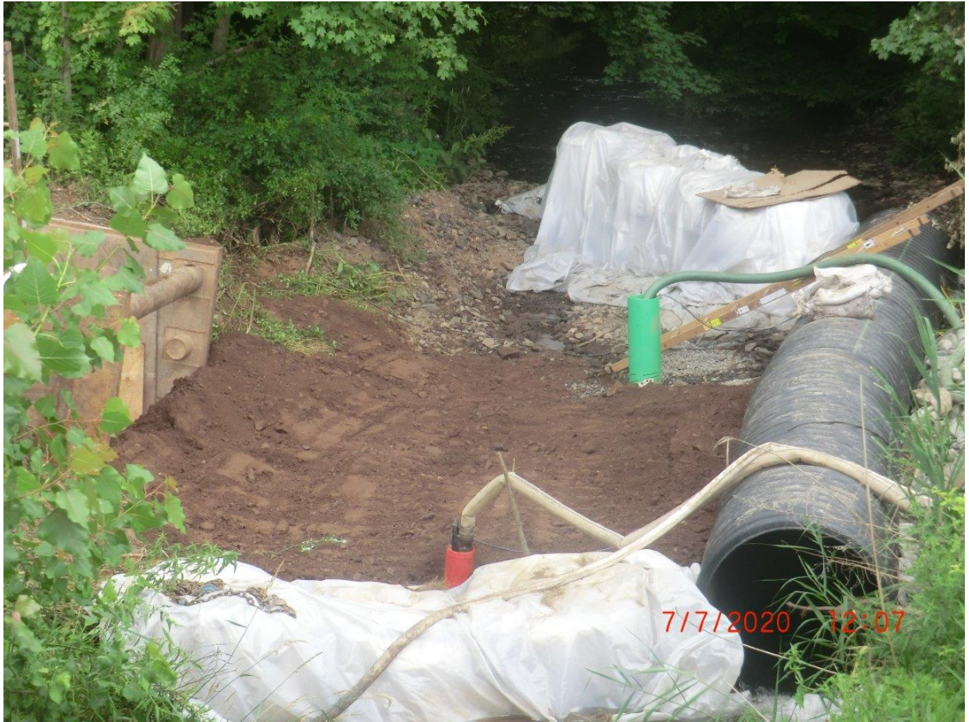
Picture 3: Allyn Brook after the 36" conduit was backfilled with sand. Station ~511+00, Pickett Lane, Durham. View to the north.
