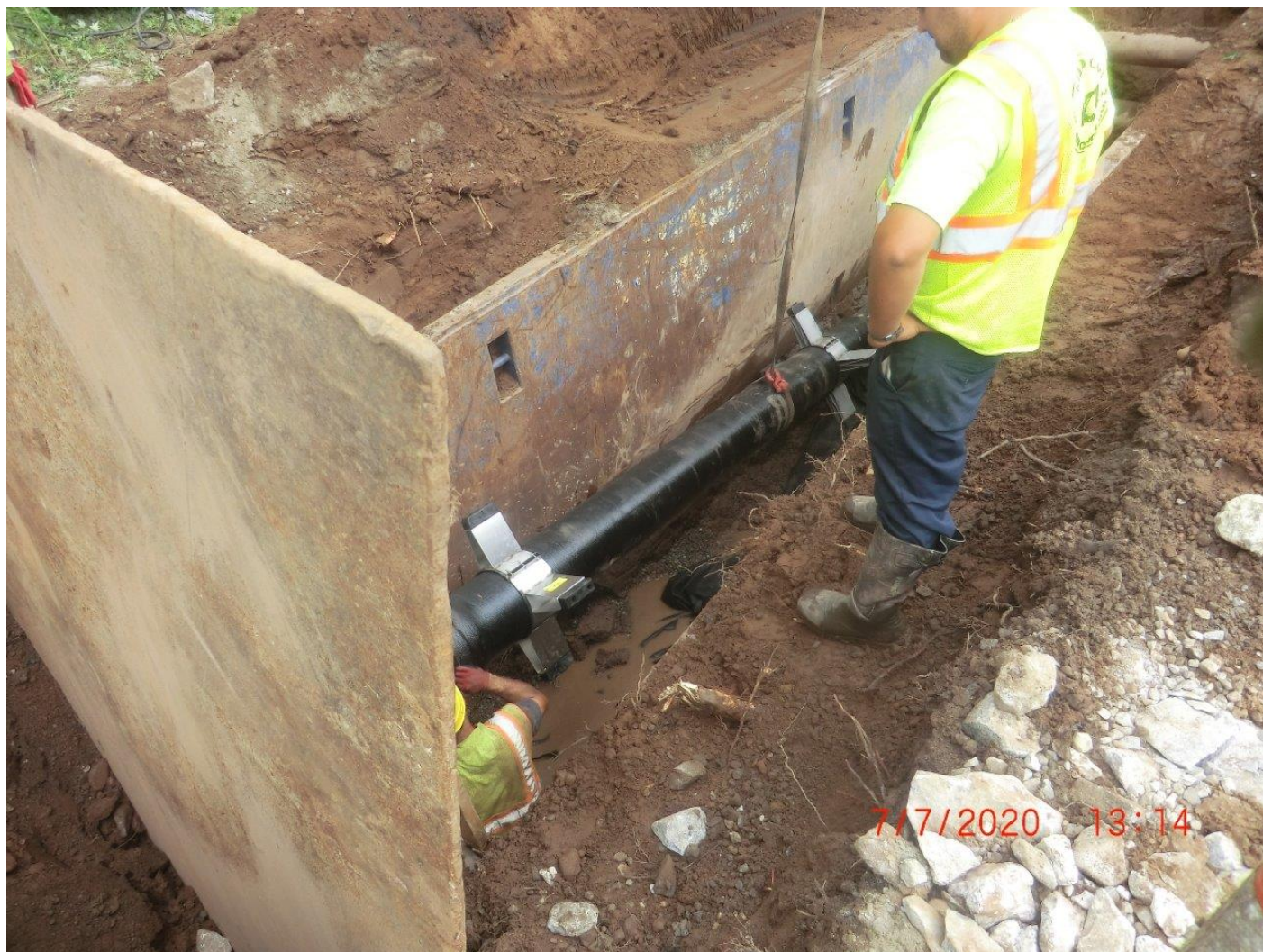
Picture 5: Ludlow preparing to insert 12" DIP with casing spacers into the 36" conduit. Station ~511+00, Pickett Lane, Durham. View to the northeast.
