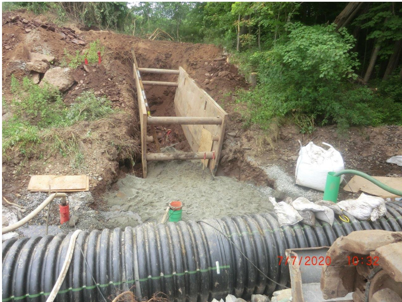
Picture 2: Trench box on the west bank of Allyn Brook during pipe installation activities. The 36" conduit has been backfilled with sand. Station ~511+00, Pickett Lane, Durham. View to the west.
