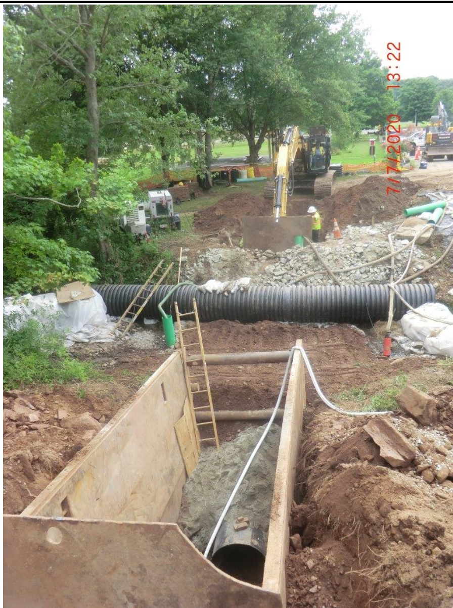
Picture 6: Overview of stream crossing work zone; view to east. 36" conduit is visible in the foreground within the trench box. Station ~511+00, Pickett Lane, Durham. View to the east.
