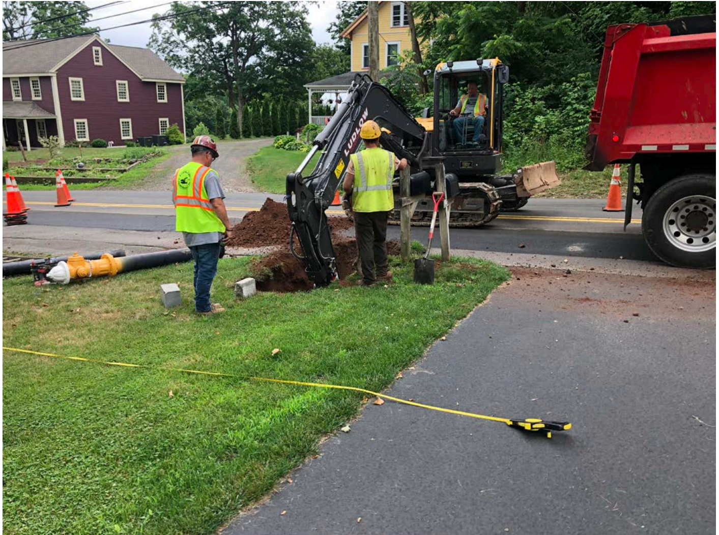
Picture 8: Ludlow installing hydrant at Station 405+40. The tape measure is located at Station 405+31, where the hydrant was originally located on Sheet C-37. View to the southeast from the driveway of 24 Maiden Lane, Durham.
