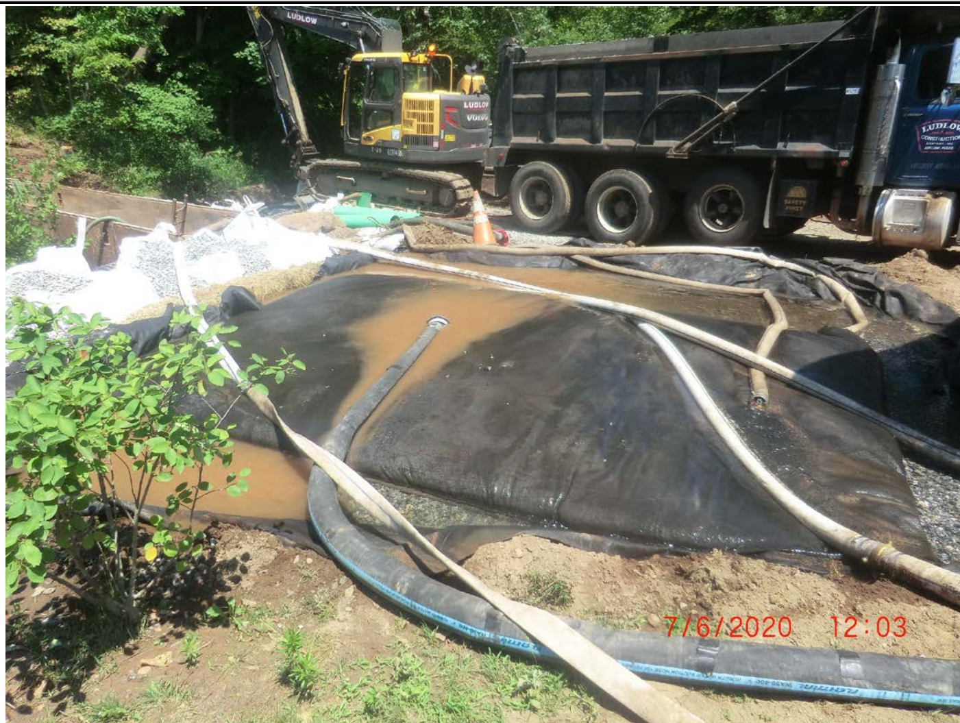
Picture 6: Water being pumped from work zone into filter bed that Ludlow placed on the east bank of Allyn Brook. Station ~511+00, Pickett Lane, Durham. View to the northwest.
