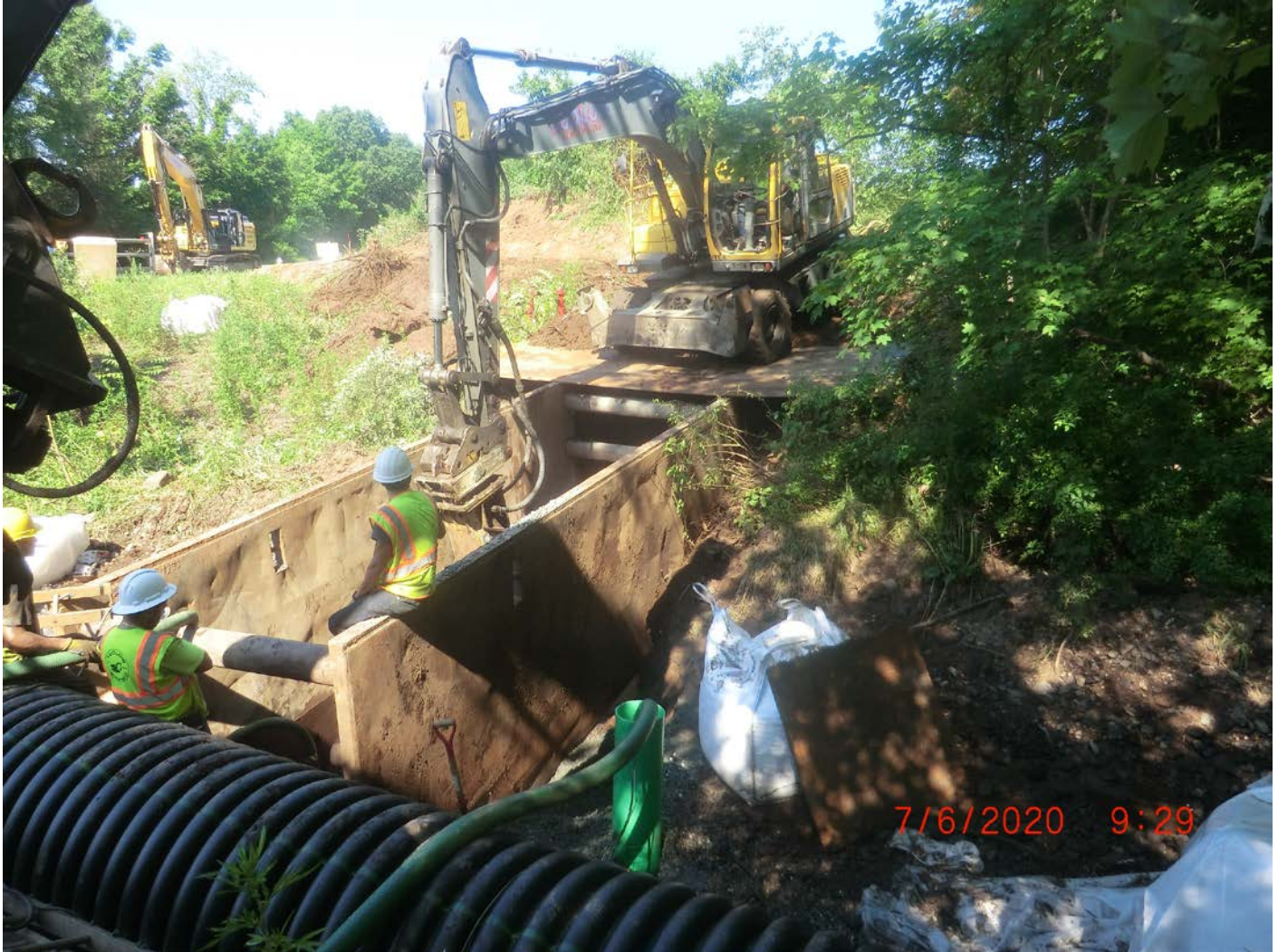
Picture 4: Ludlow staged on the west bank of Allyn Brook as they begin to excavate the bank and stream bed for the placement of 36" conduit. Station ~511+00, Pickett Lane, Durham. View to the west.
