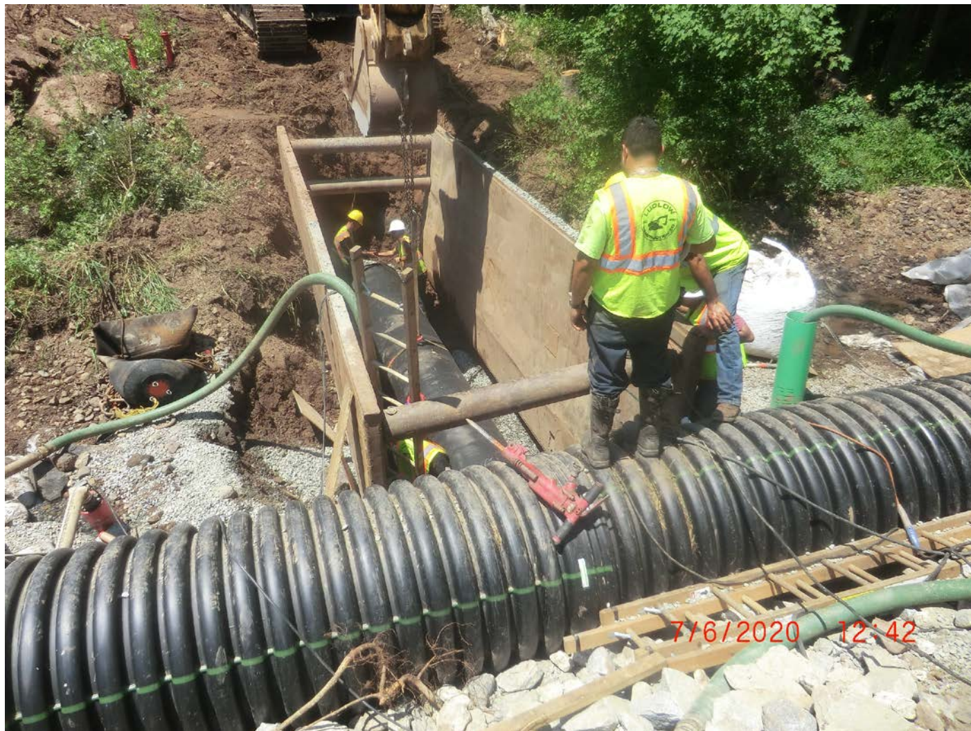
Picture 9: View of 36" conduit being placed across stream bed to meet another piece of 36" conduit that was installed last week. Station ~511+00, Pickett Lane, Durham. View to the east.
