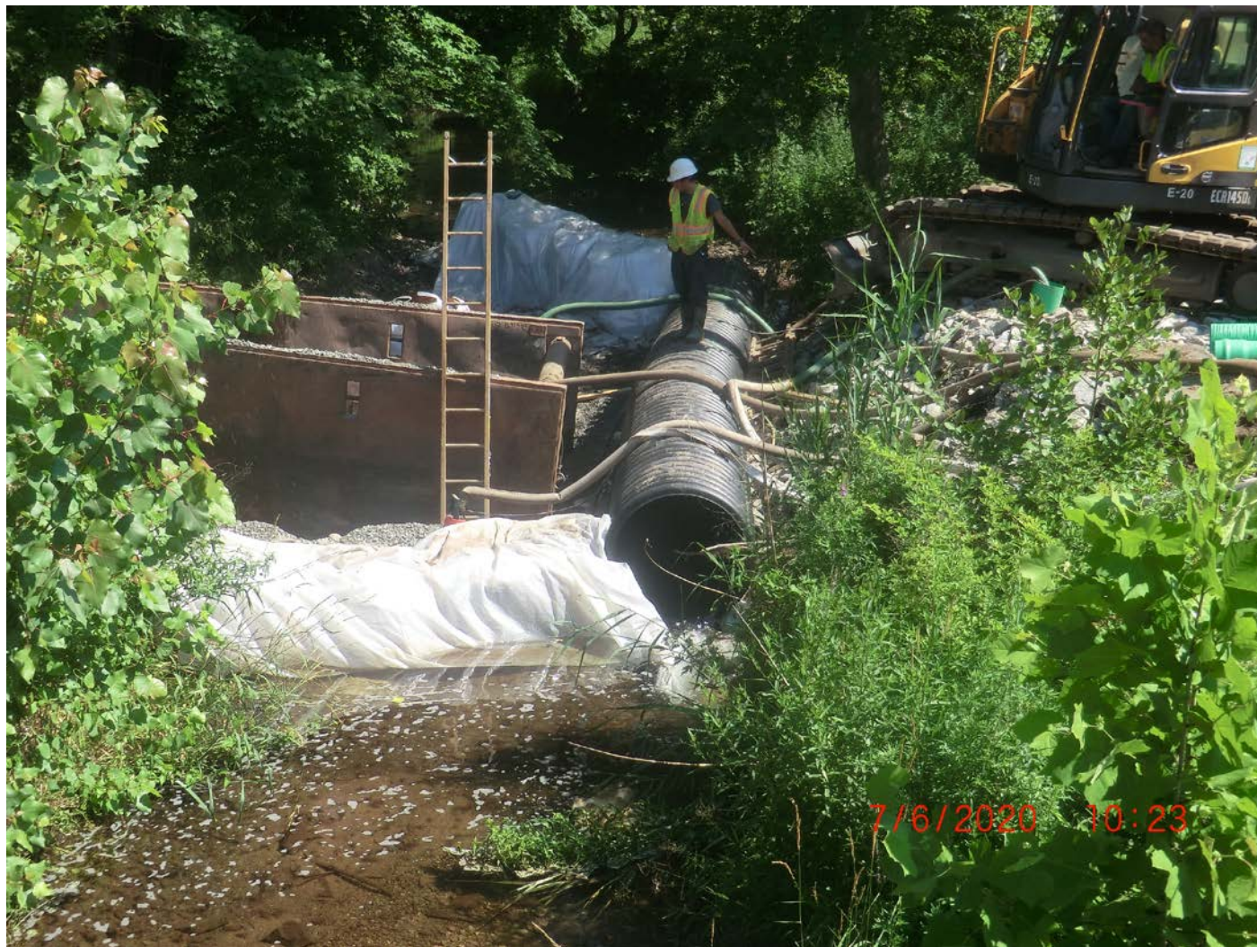
Picture 5: View of trench box installed on the west bank of Allyn Brook for the excavation of the stream bank and stream bed for the placement of 36" conduit. Station ~511+00, Pickett Lane, Durham. View to the north.
