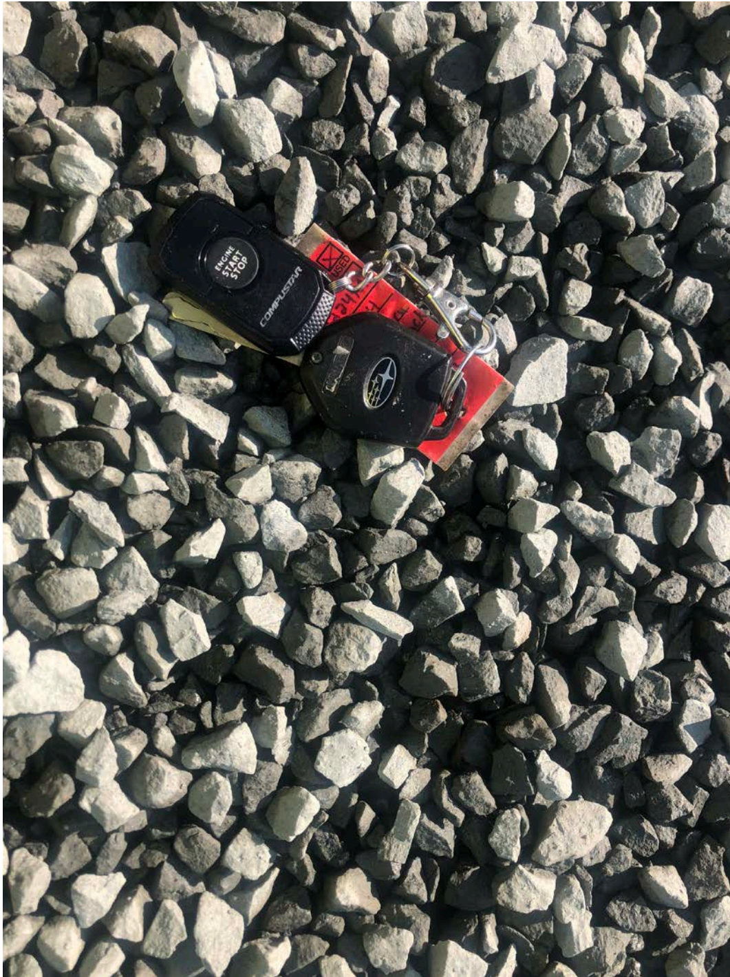
Picture 11: Close-up of No. 67 1/2" gravel being placed in Picture 10. Water tank footprint, Shared Access Driveway, Middletown.
