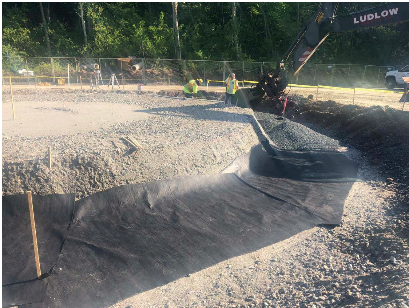
Picture 10: Ludlow placing No.67 ½" gravel on top of filter fabric on the ring of soil at elevation 437 within the water tank footprint. Shared Access Driveway, Middletown. View to the southeast.
