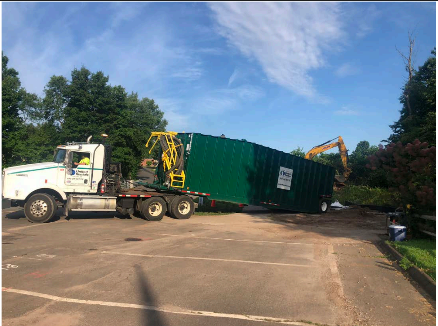
Picture 1: United Rentals placing frac tank at Station ~511+00 as part of ongoing stream crossing activities. Pickett Lane, Durham. View to the northwest.
