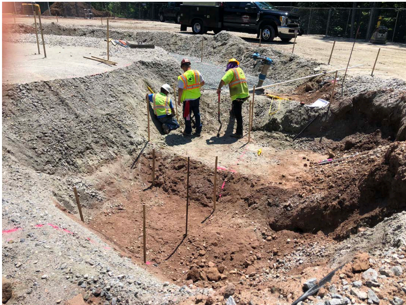
Picture 13: Ludlow refining grades and cuts in fill at the water tank footprint where the tank's supply and feed lines will be placed. Shared Access Driveway, Middletown. View to the southeast.
