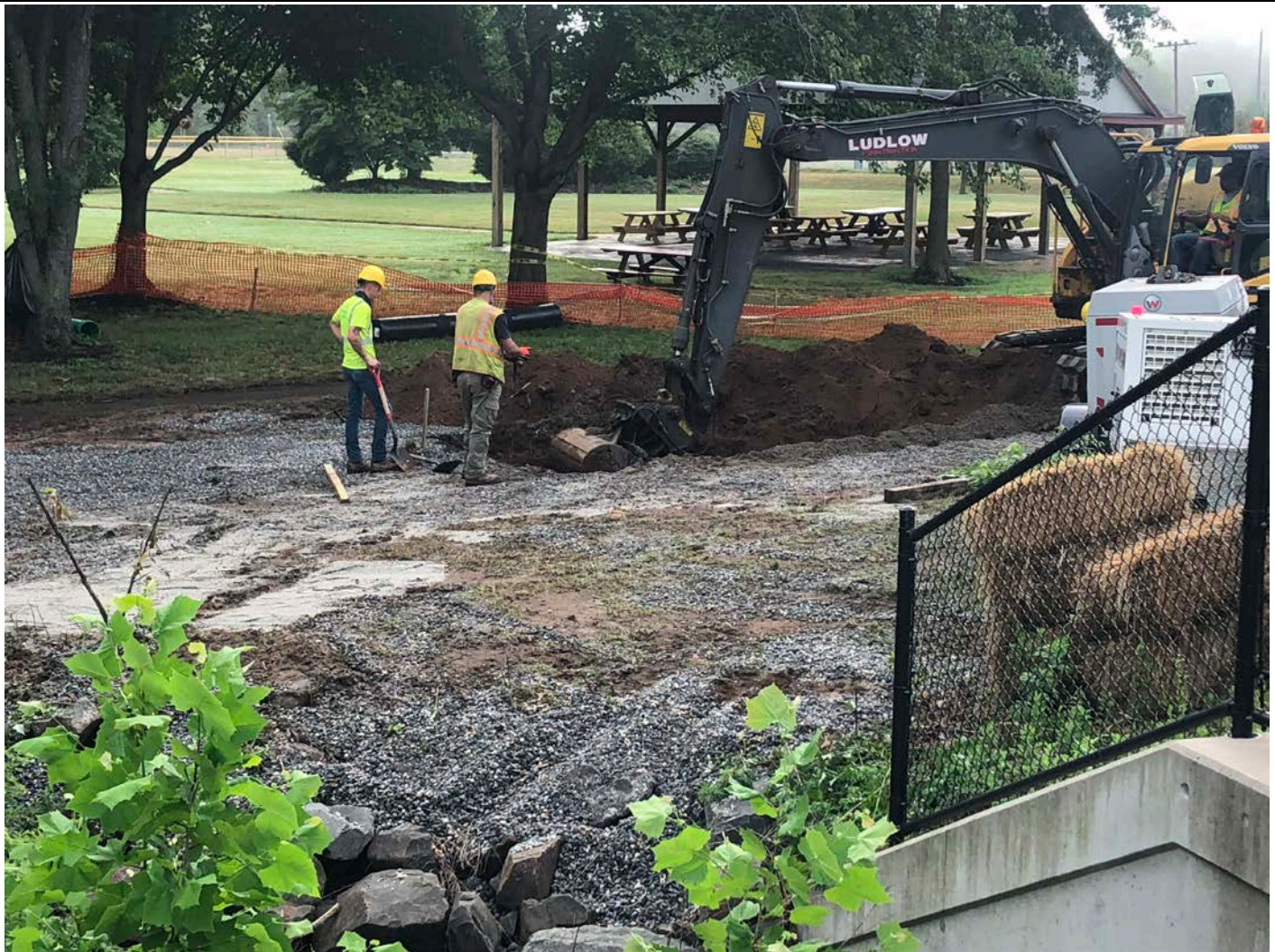
Picture 6: Ludlow excavating test pit to the east of Allyn Brook at Station~511+00. Pickett Lane, Durham.
