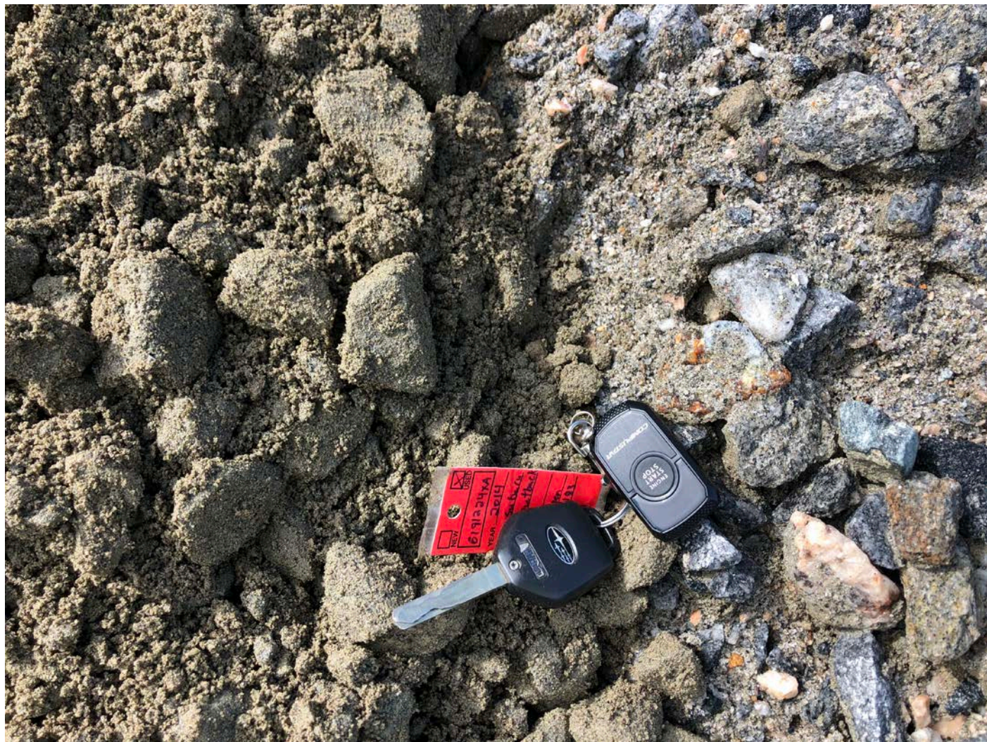
Picture 13: Closeup of the structural fill being placed in the water tank footprint. Shared Access Driveway, Middletown. View to the southeast.
