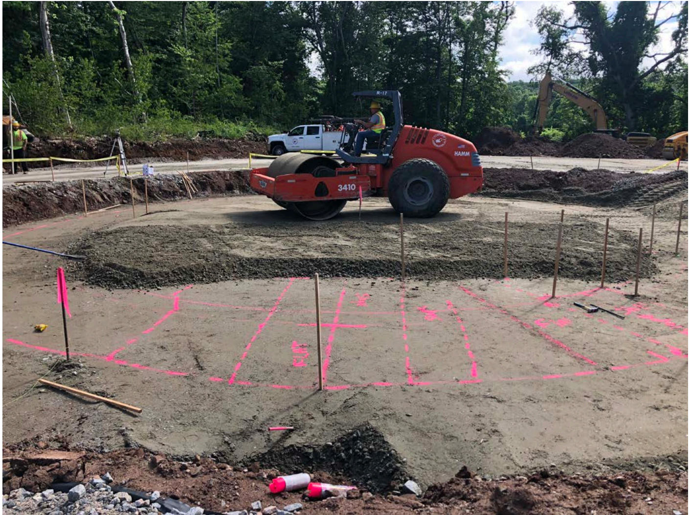
Picture 14: Ludlow compacting structural fill at elevation 437. Shared Access Driveway, Middletown. View to the southeast.
