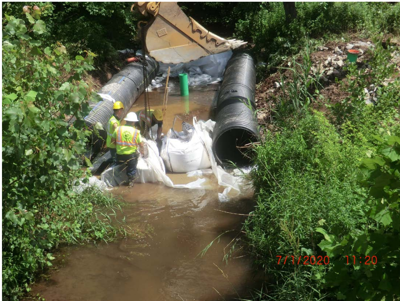
Picture 3: Ludlow in the process of moving sandbags after placing 40" stream flow bypass culvert on the east bank of Allyn Brook. View to the north. Pickett Lane, Durham.
