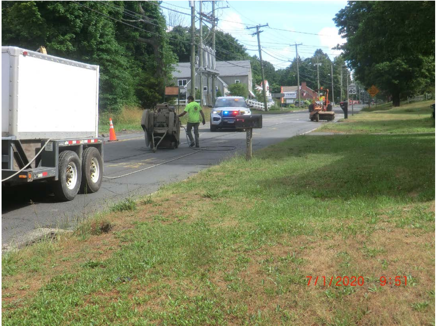
Picture 2: Ludlow subcontractor saw cutting pavement on Main Street in Durham. View to the north.
