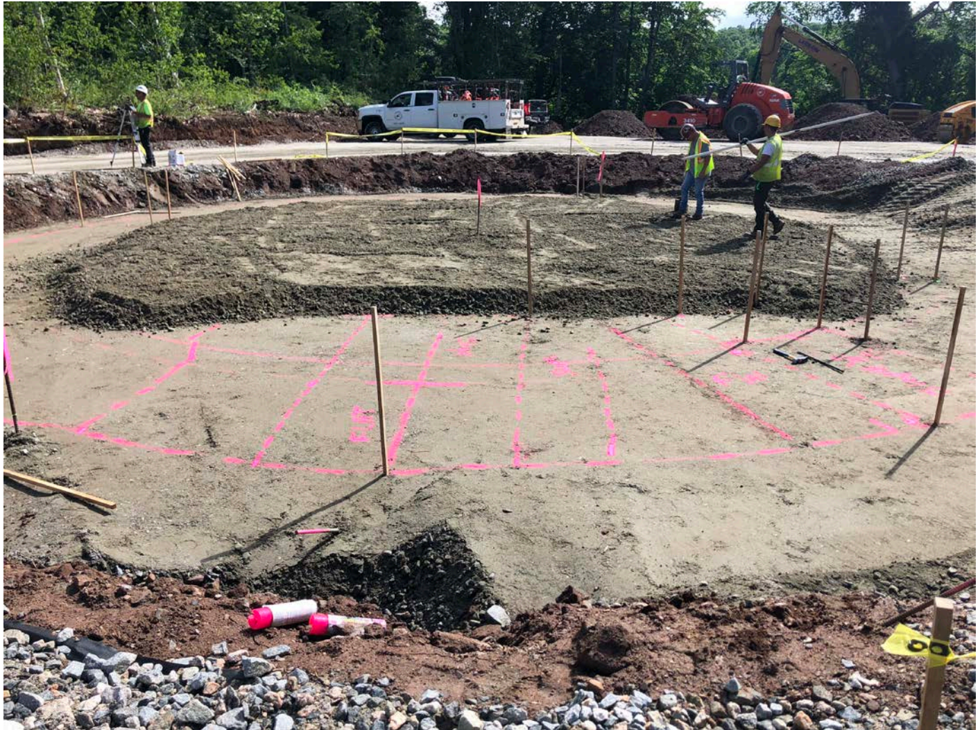
Picture 12: Ludlow continues to place structural fill in an 8" lift at elevation 437. Shared Access Driveway, Middletown. View to the southeast.
