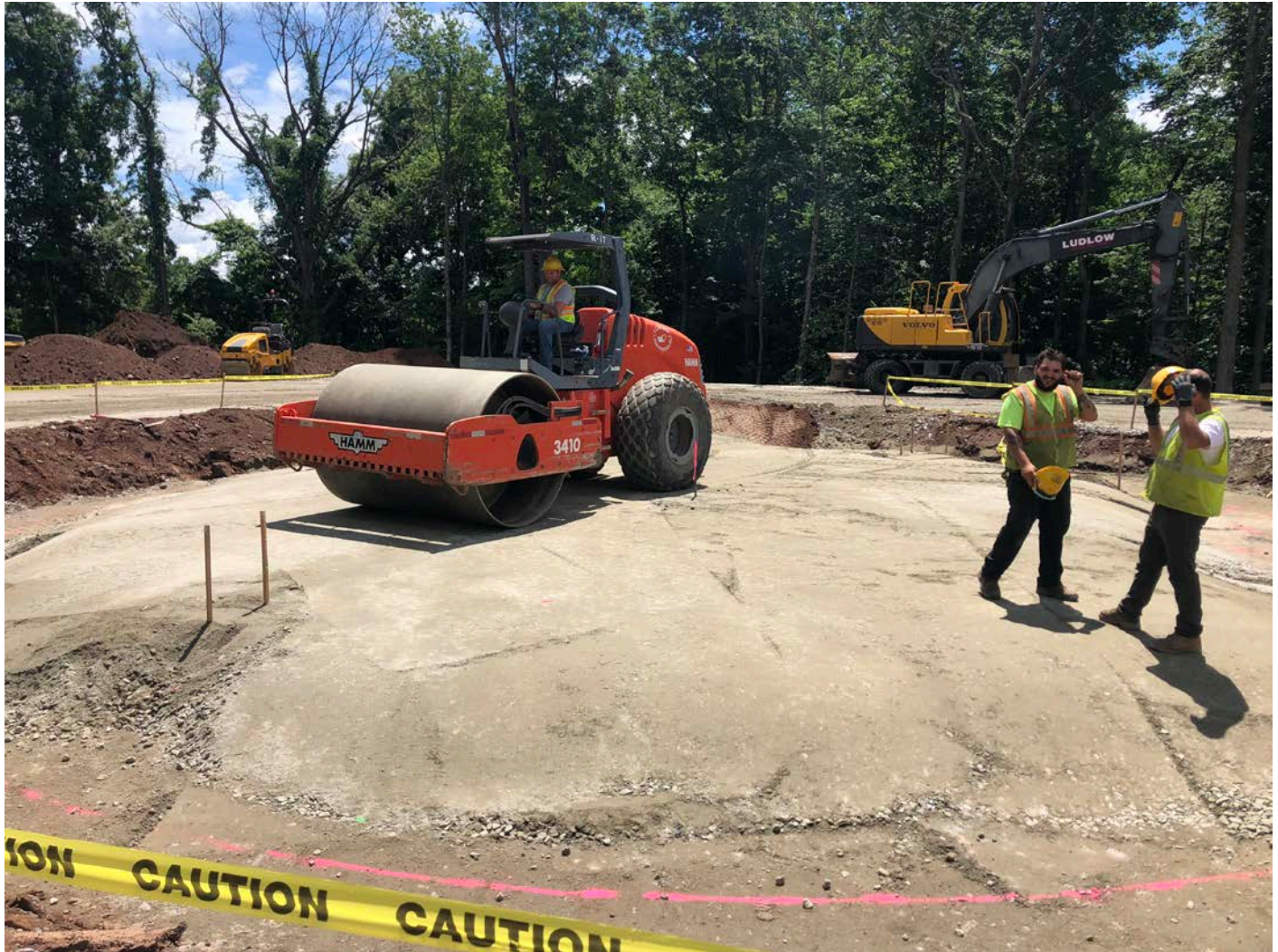
Picture 15: Ludlow compacting structural fill at elevation 438.34. Shared Access Driveway, Middletown. View to the southeast.
