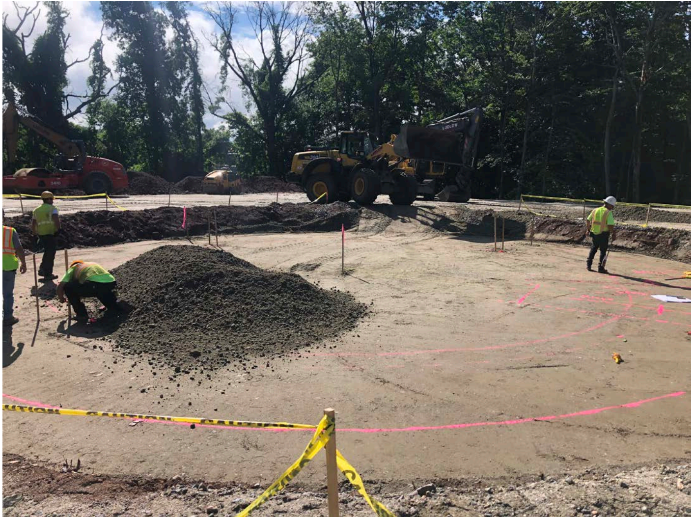
Picture 11: Ludlow begins to place structural fill in an 8" lift at elevation 437. Shared Access Driveway, Middletown. View to the southeast.
