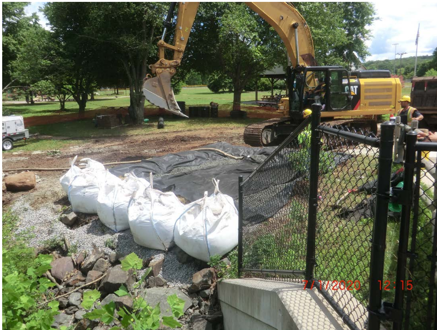
Picture 4: Ludlow building a silt retention basin on the east side of Allyn Brook at Station ~511+00. Pickett Lane, Durham. View to the northeast.
