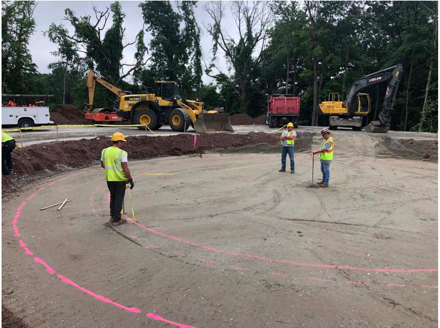
Picture 10: Ludlow setting up grade stakes on the water tank footprint at elevation 437. Shared Access Road, Middletown. View to the southeast.
