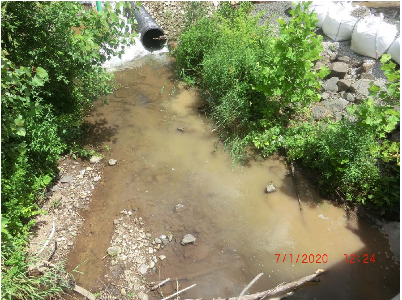
Picture 5: Elevated silt load entering Allyn Brook at Station ~511+00 from silt retention basin. Pickett Lane, Durham. View to the north.
