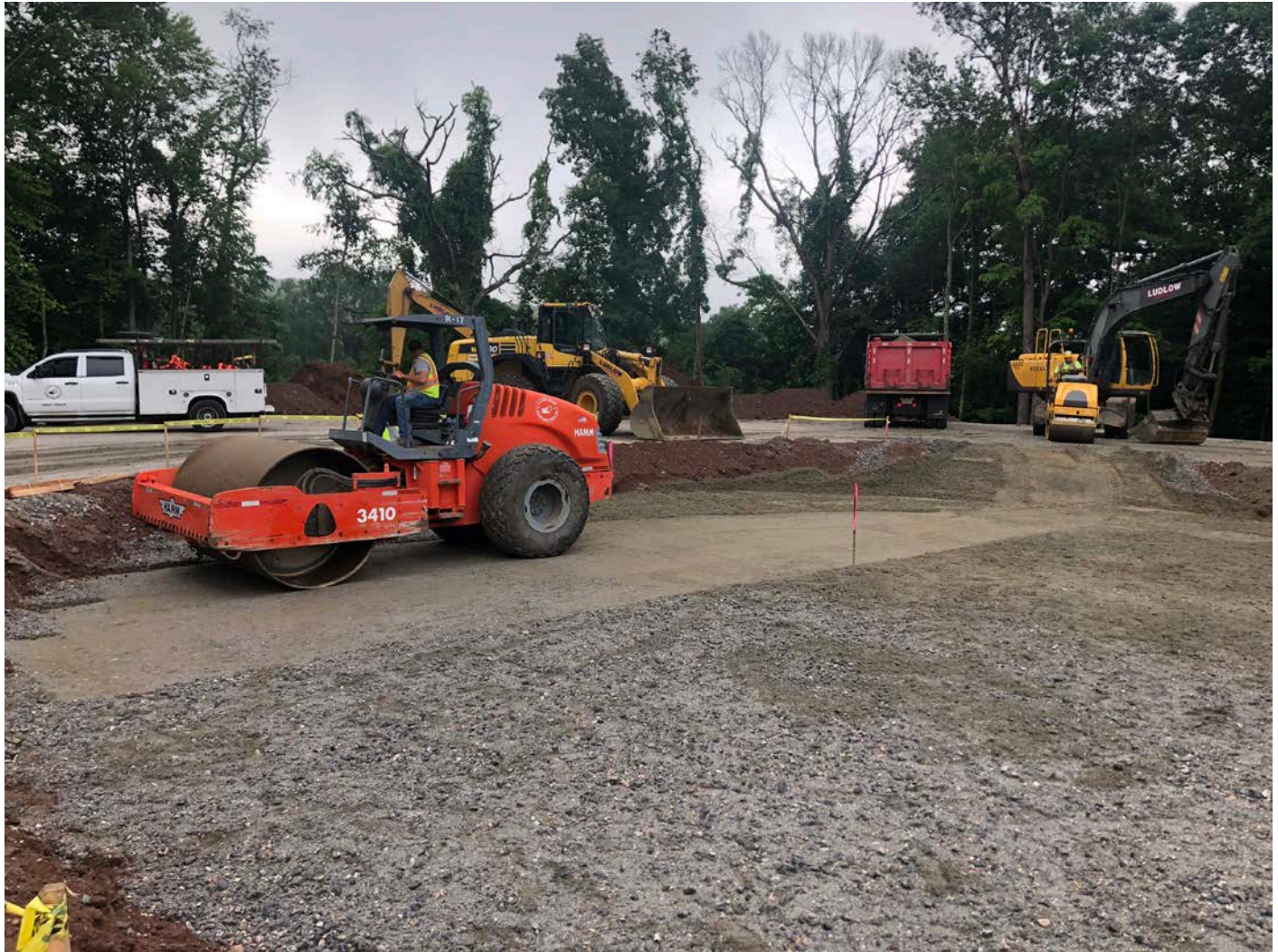
Picture 7: Ludlow compacting 4" lift of structural fill that brought the elevation within the water tank footprint up to 437. Shared Access Driveway, Middletown. View to the southeast.
