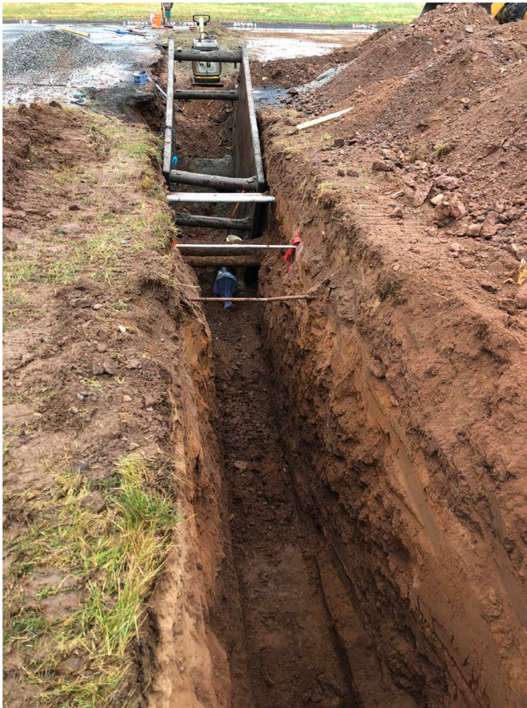
Picture 9: Trench at Station 529+56 after having daylighted a number of utilities. View to the east. Pickett Lane, Durham.
