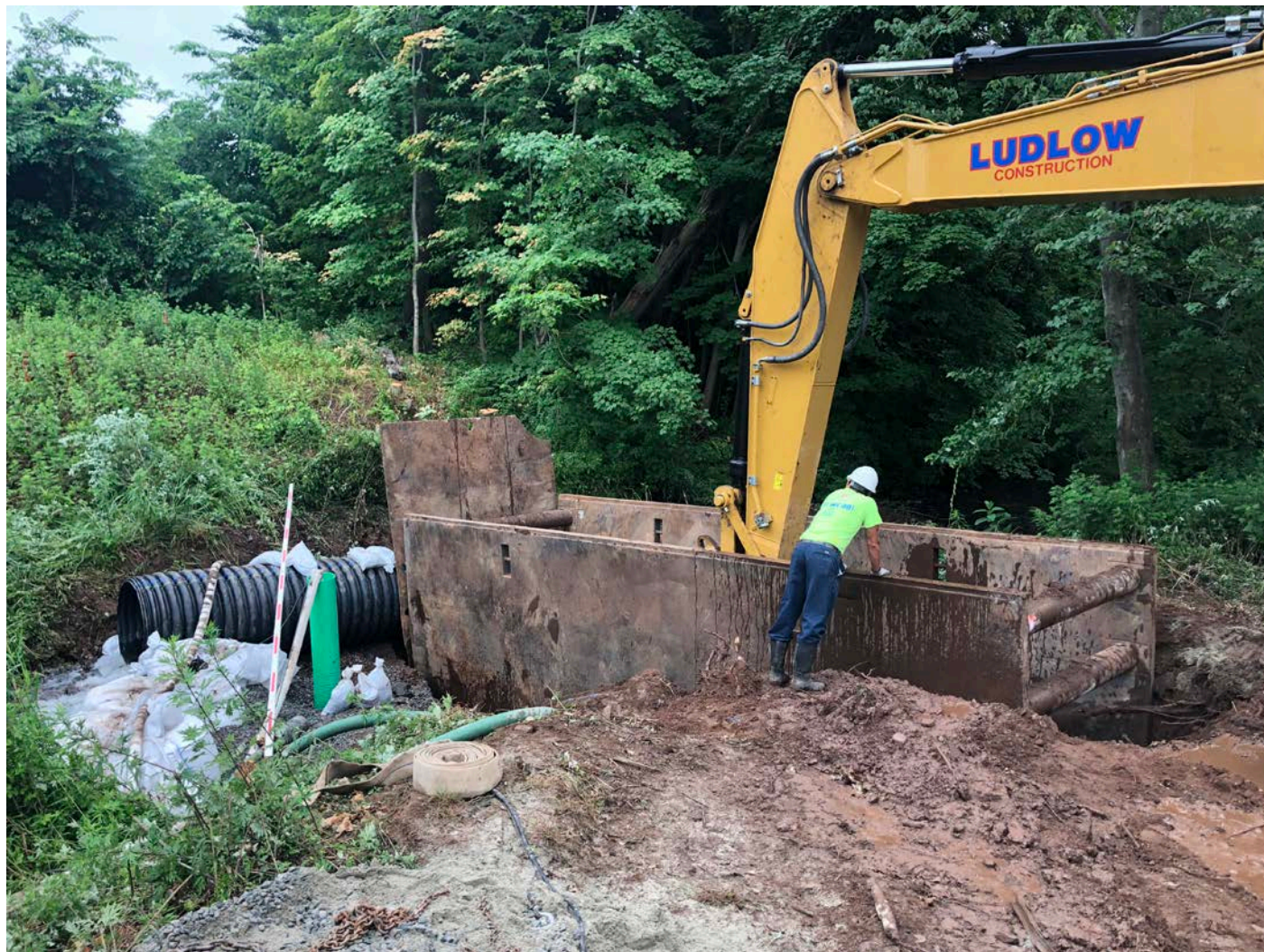
Picture 4: Ludlow excavating within trench box placed at the stream crossing located at Station ~511+00. Pickett Lane, Durham. View to the northwest.
