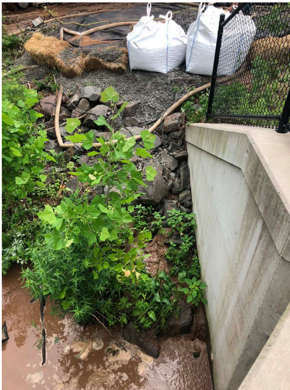
Picture 7: Ludlow employed 3 silt bags to filter water pumped from the stream crossing work zone while placing 30" conduit. The bags (visible at the top of the picture) were not able to keep up with the water flow and silt load and failed, resulting in high turbidity downstream of the work zone. Station ~511+00, Pickett Lane, Durham. View to the northeast.
