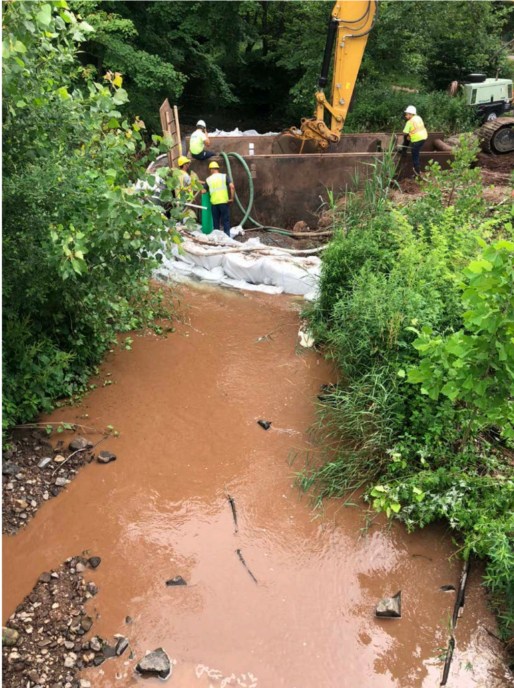
Picture 6: High turbidity observed downstream of the work zone at the stream crossing located at Station ~511+00. View is upstream and to the north. Pickett Lane, Durham.
