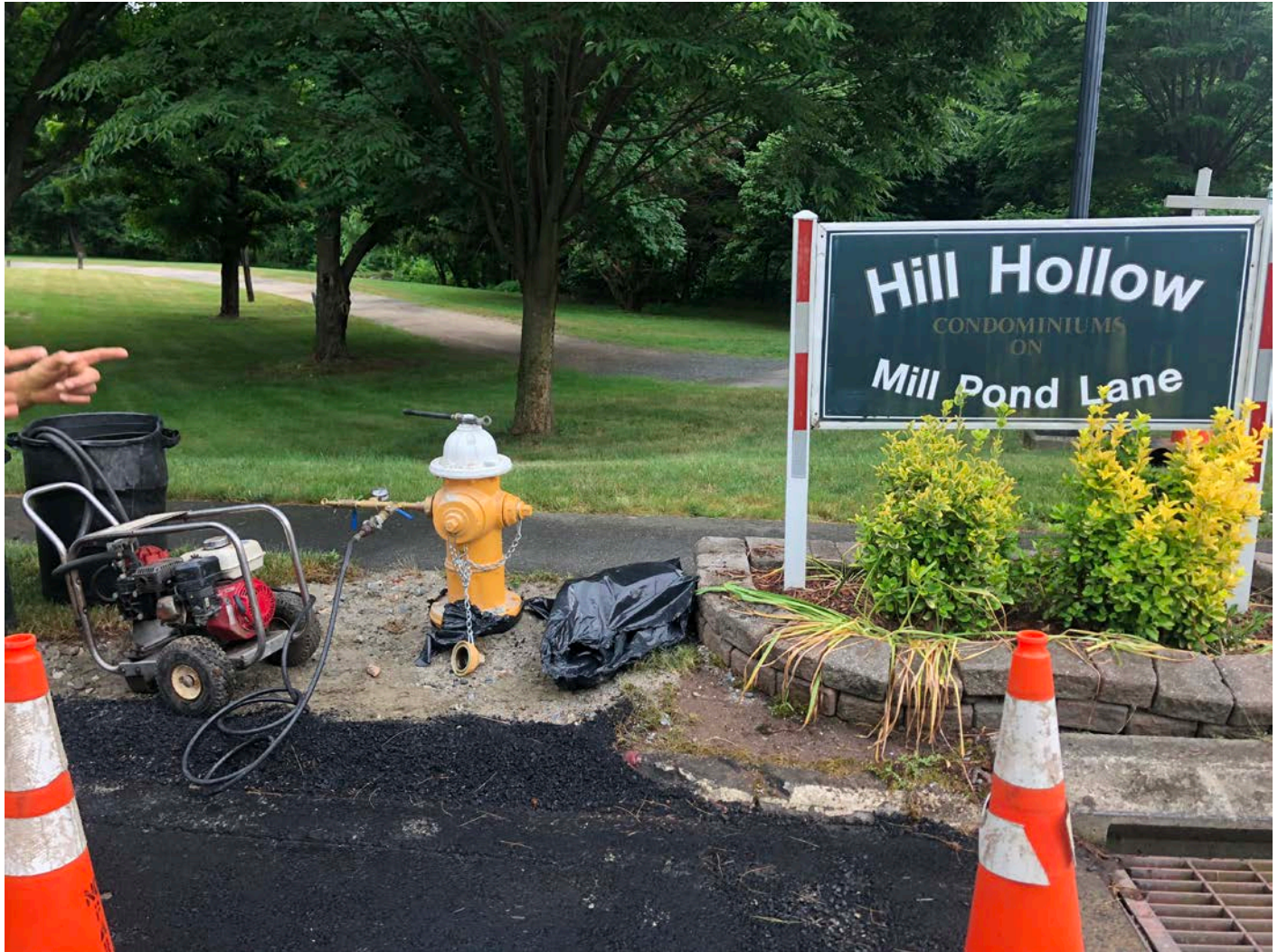
Picture 3: Pressure test set up on the hydrant installed on Mill Pond Lane on June 26, 2020. View to the south.
