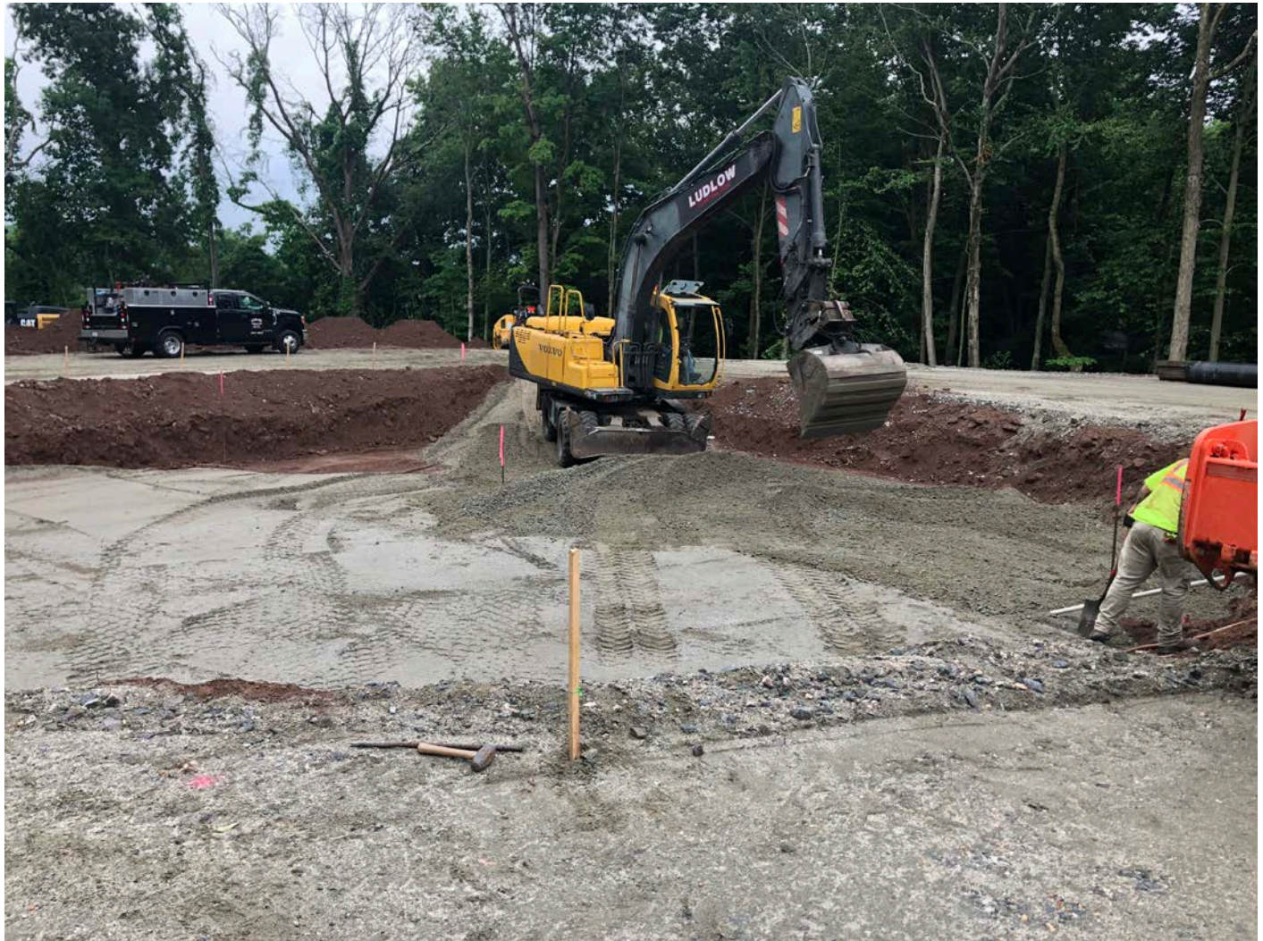
Picture 1: Ludlow placing structural fill at the water tank footprint, bringing the elevation from 435 to 436. Shared Access Road, Middletown. View to the southeast.
