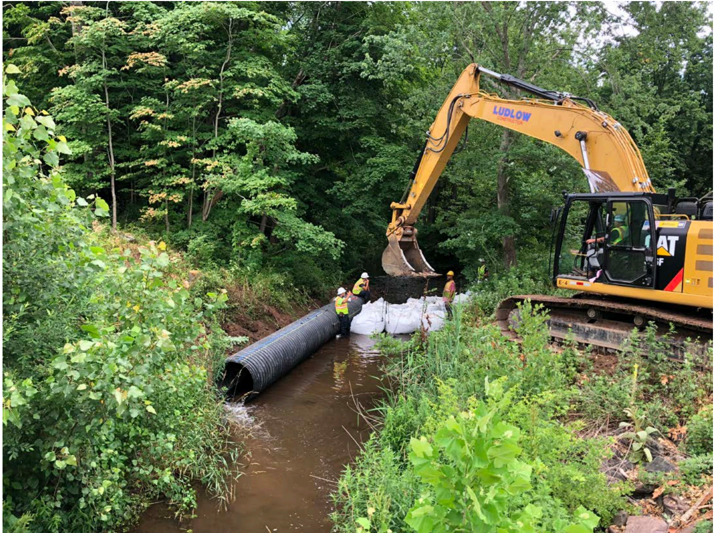
Picture 5: Ludlow installing 40" plastic culvert as a stream flow bypass for the stream crossing at Station ~511+00. Pickett Lane, Durham. View to the north.
