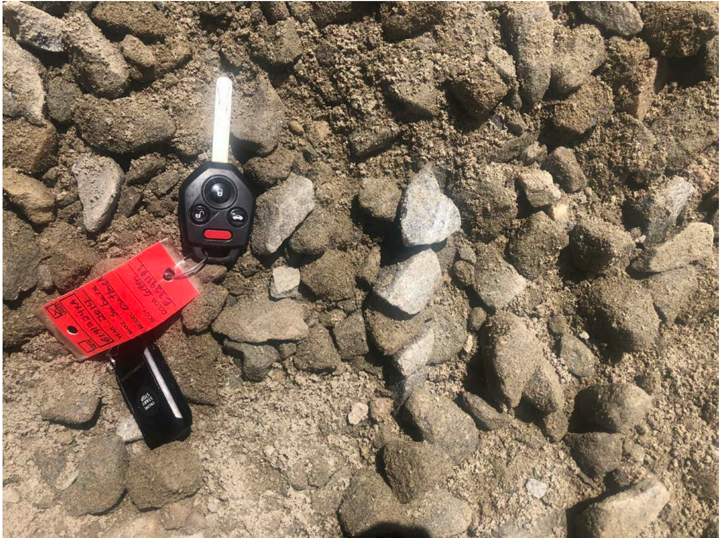
Picture 16: Closeup of structural fill placed on the water tank footprint with keys to provide scale. Shared Access Road, Middletown. View to the southeast.
