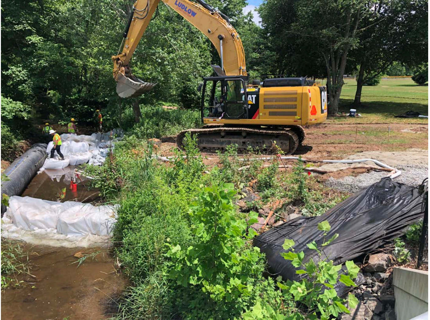
Picture 11: Allyn Brook looking upstream from Pickett Lane. Ludlow has bracketed the work zone for the stream crossing at Station ~511+00 with sand bags and has two pumps moving water from the zone and into the silt bag that is visible on the right hand side of the photo. View is upstream and to the north. Pickett Lane, Durham.
