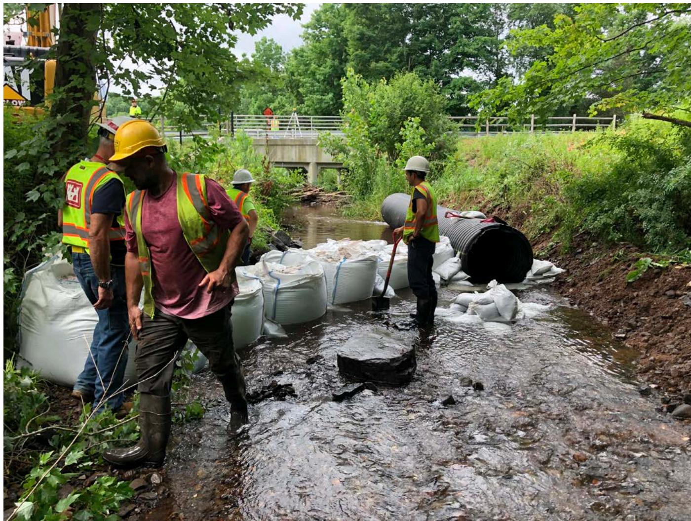
Picture 6: View of the 40" plastic culvert at Station ~511+00 with large and small sand bags placed to divert flow into pipe. View is downstream and to the south. Pickett Lane, Durham.
