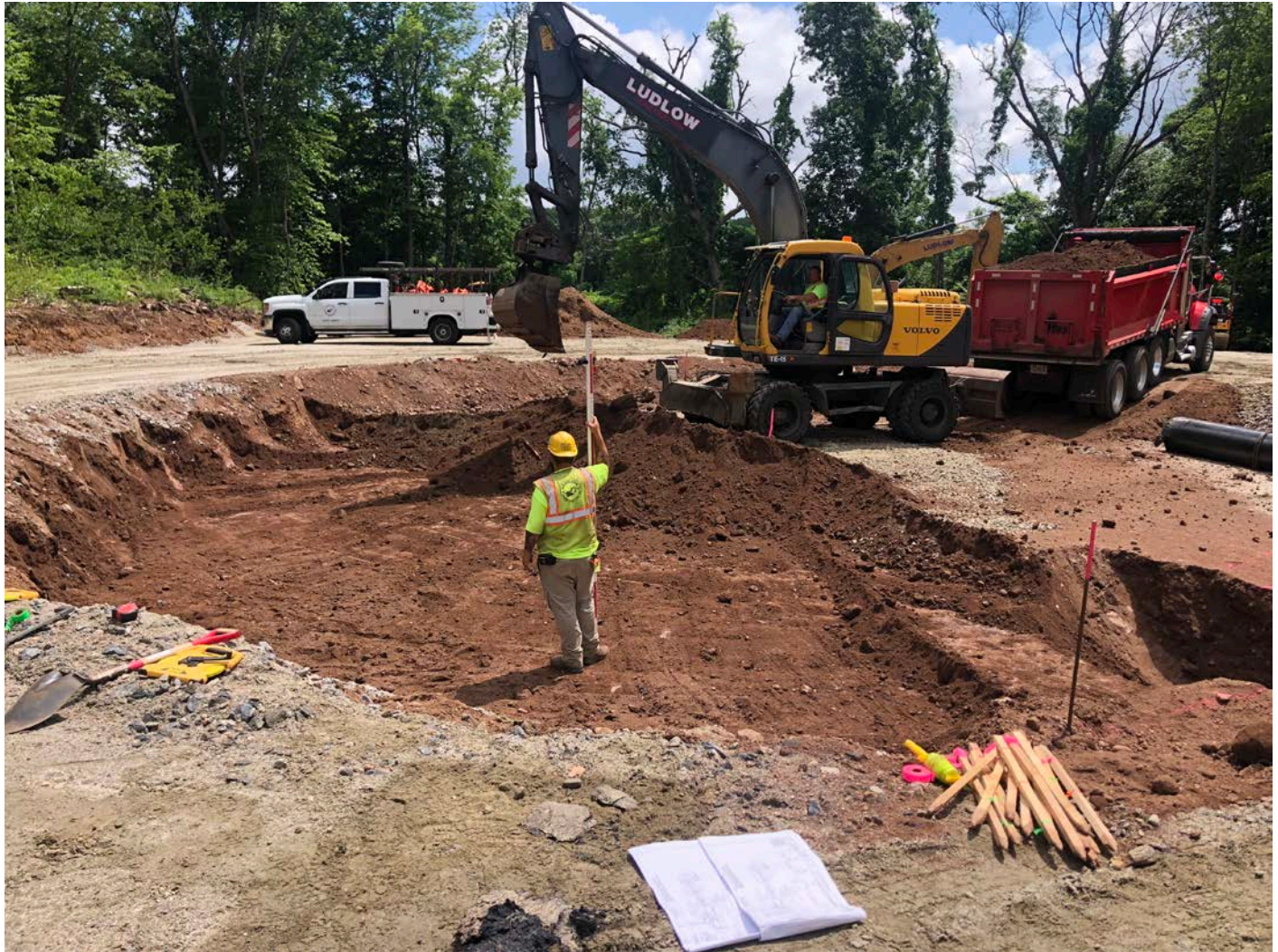
Picture 10: Water tank footprint as Ludlow removes fill down to elevation 435 today upon the advice of DN Tanks. Shared Access Driveway, Middletown. View to the southeast.
