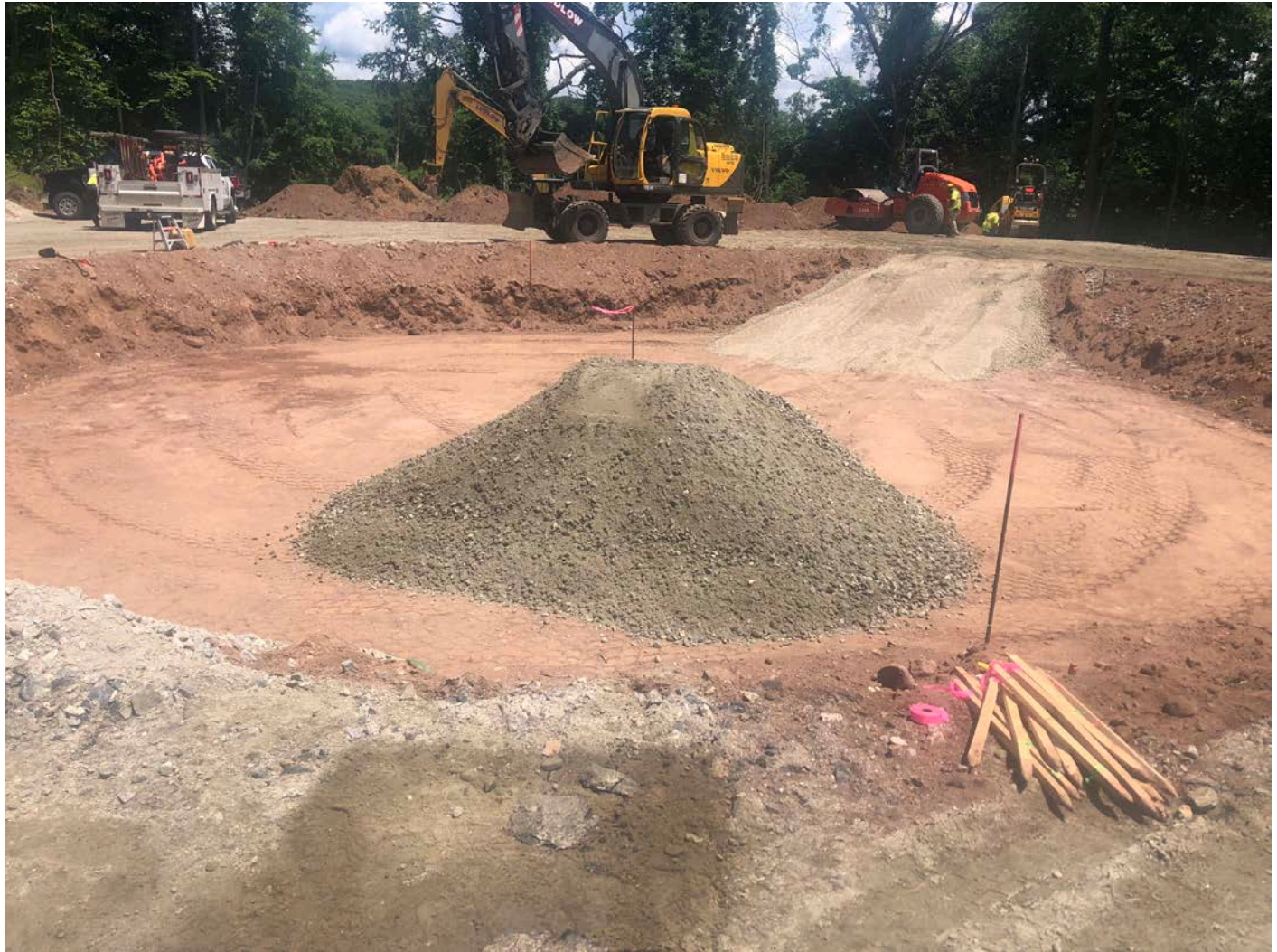
Picture 15: Ludlow placing structural fill on the water tank footprint. Shared Access Driveway, Middletown. View to the southeast.
