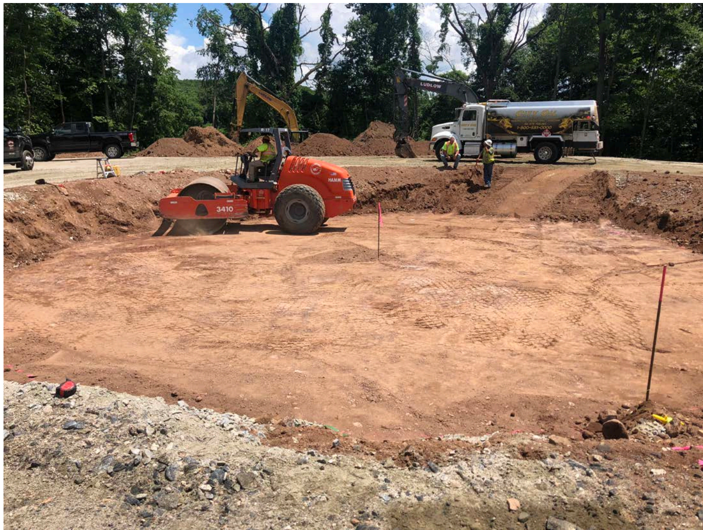
Picture 14: Ludlow compacting fill at elevation 435 at the water tank footprint. Shared Access Driveway, Middletown. View to the southeast.
