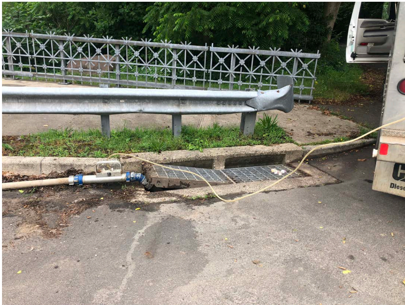
Picture 2: Ludlow dechlorinating the Main Street water line with calcium thiosulfate at the intersection of Main Street and Old Cemetery Road. View to the south.
