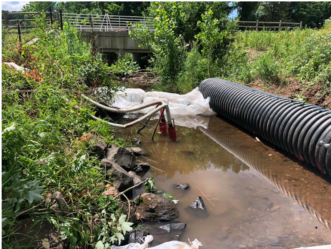
Picture 13: Allyn Brook looking downstream towards Pickett Lane. Ludlow has placed sand bags on the upstream and downstream sides of the stream crossing work zone and stream flow is diverted into the 40" plastic culvert visible on the right. Station ~511+00, Pickett Lane, Durham.
