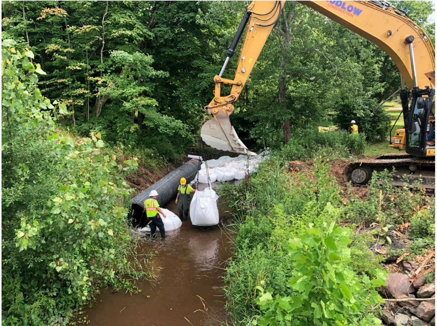
Picture 9: Ludlow placing large sand bag next to work zone for the stream crossing at Station ~511+00. View is upstream and to the north. Pickett Lane, Durham.
