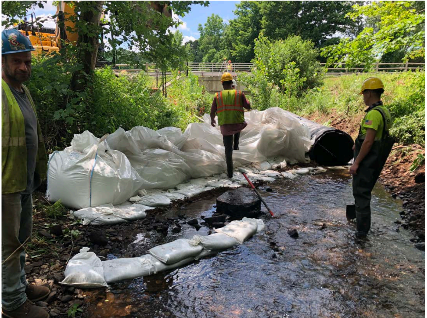
Picture 12: Allyn Brook looking downstream towards Pickett Lane. Ludlow has placed sand bags to divert stream flow into the 40" plastic culvert. Pickett Lane, Durham.
