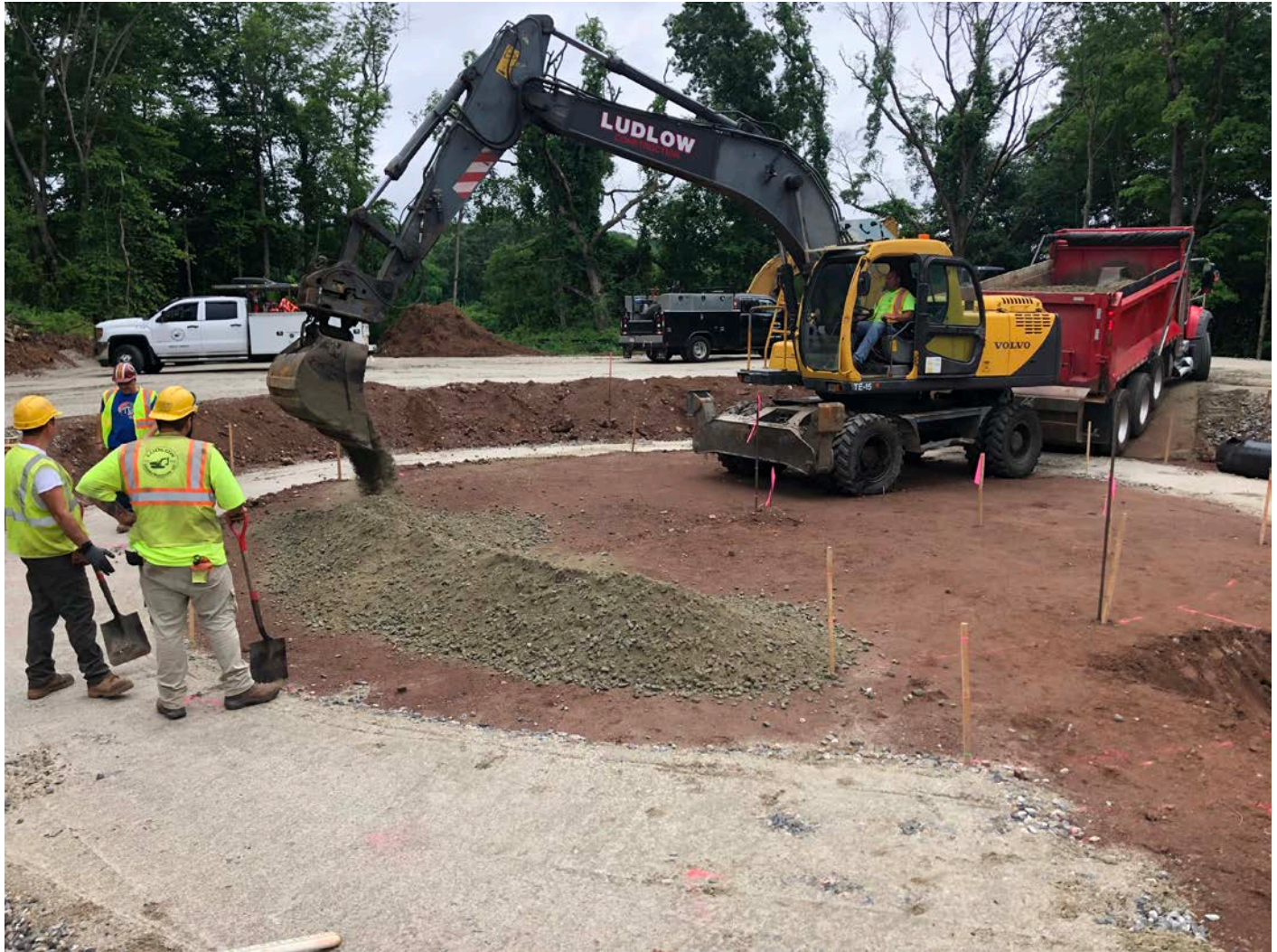
Picture 4: Ludlow placing 1.5" gravel at the water tank footprint. Shared Access Driveway, Middletown. View to the southeast.
