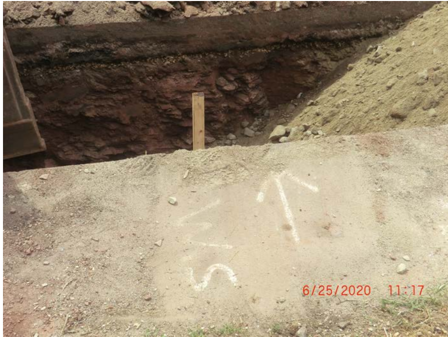
Picture 9: One of two curb stops installed on Maiden Lane, marked by 2x3 stake. View to the south.
