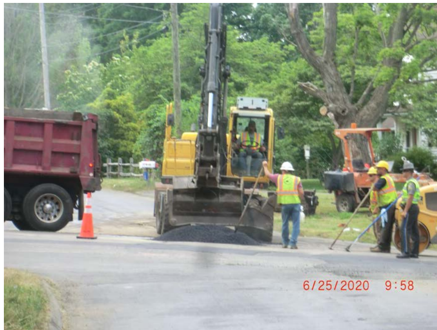
Picture 4: Starting hot patch at Maple Ave. and Wallingford Road (Route 68). View to the south.
