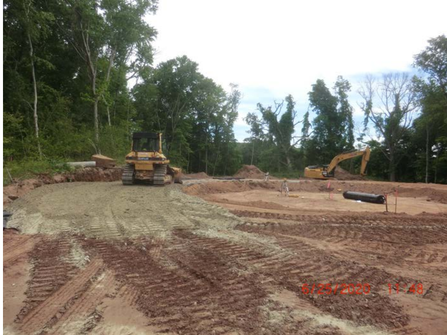
Picture 13: Facing east. Filling on top of matting gravel base for road around tank.
