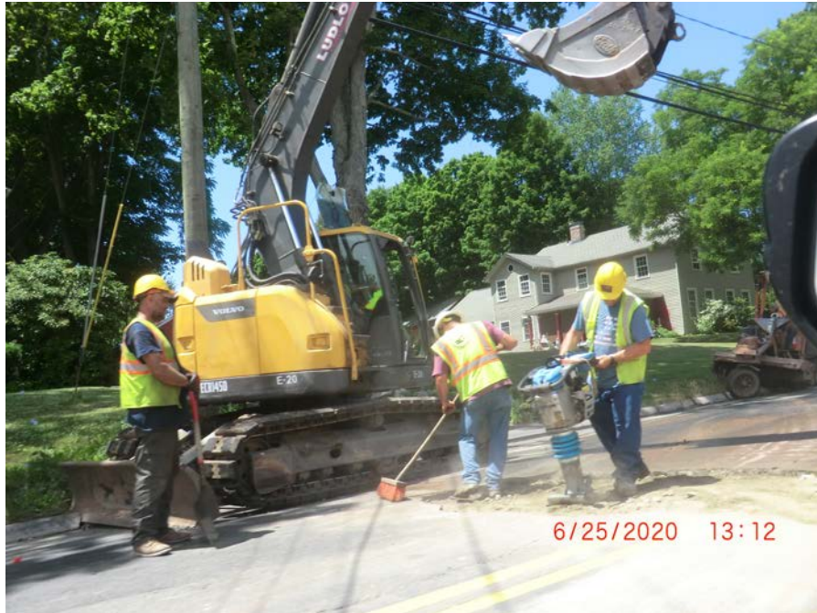
Picture 11: Ludlow finishing up road closing on Route 17, Main Street, across from Durham Manufacturing. Due to amount of bedrock encountered, Ludlow decided to only go halfway across today. View is to northwest.
