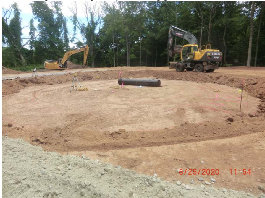
Picture 13: Facing east. Filling on top of matting gravel base for road around tank.
