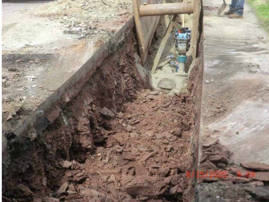
Picture 7: Shallow ledge at roughly 403+70 feet on Maiden Lane. This was the shallowest ledge section in today's trenching. It required hammering before removal. View is to the west.
