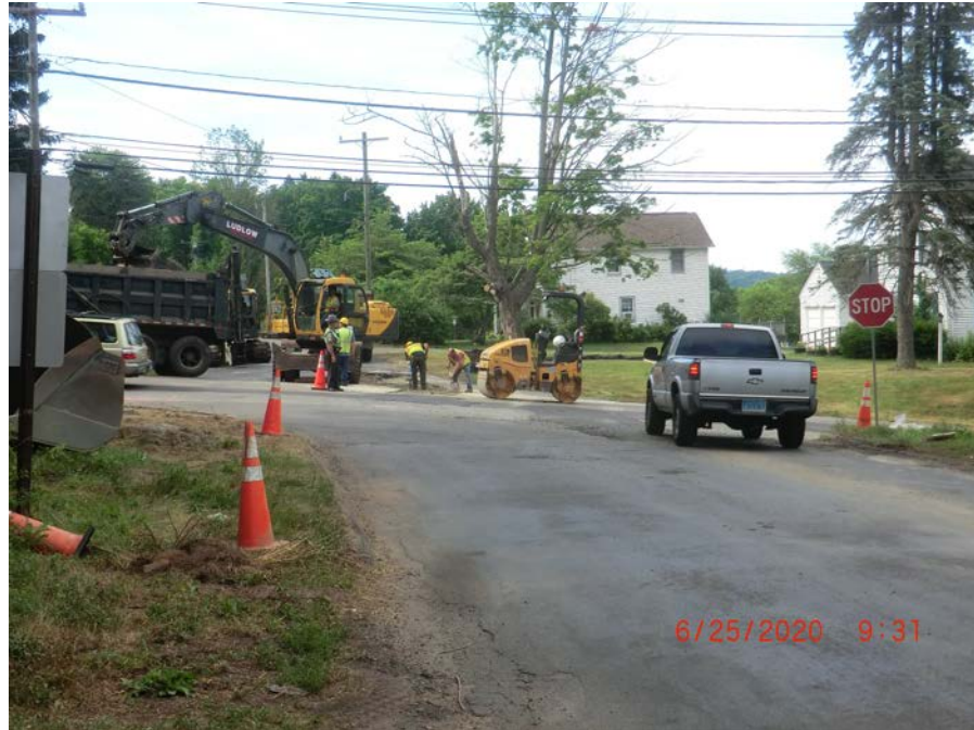
Picture 3: Ludlow completing backfill and compaction at Maple Ave. and Wallingford Road (Route 68). View to the south.
