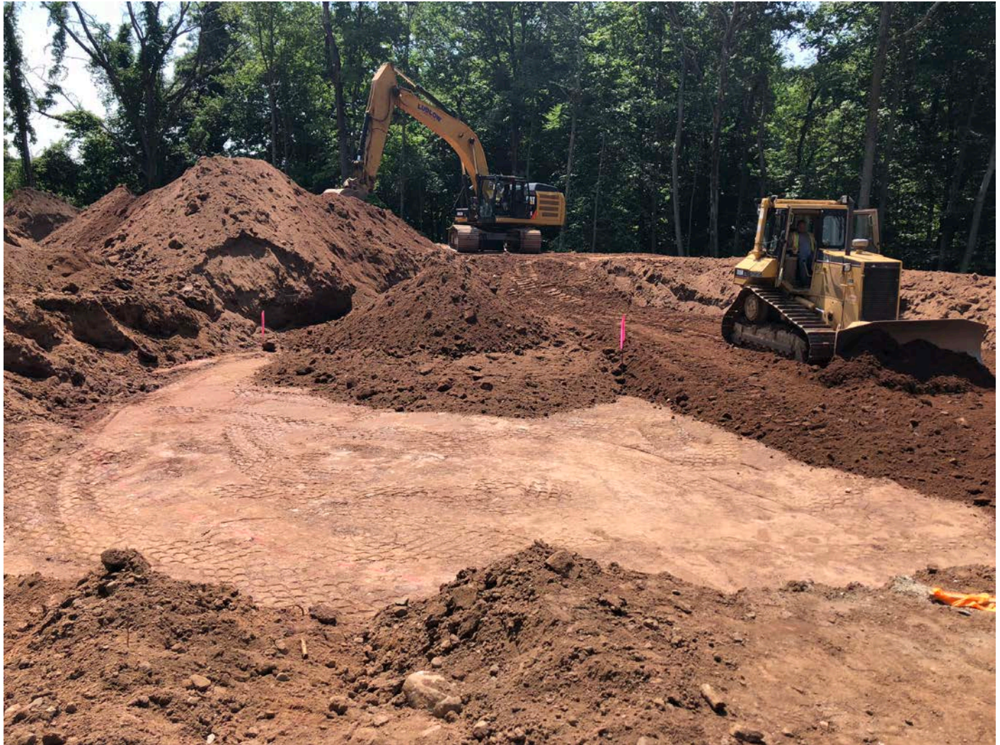
Picture 7: Ludlow placing fill in lifts between compacting at the footprint of the water tank pad. Shared Access Road; view to the southeast.
