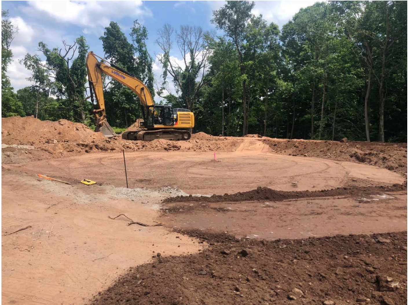
Picture 8: The footprint of the water tank pad after 2' of fill was placed and compacted to make a subbase for the tank pad. Shared Access Driveway; view to the southeast.
