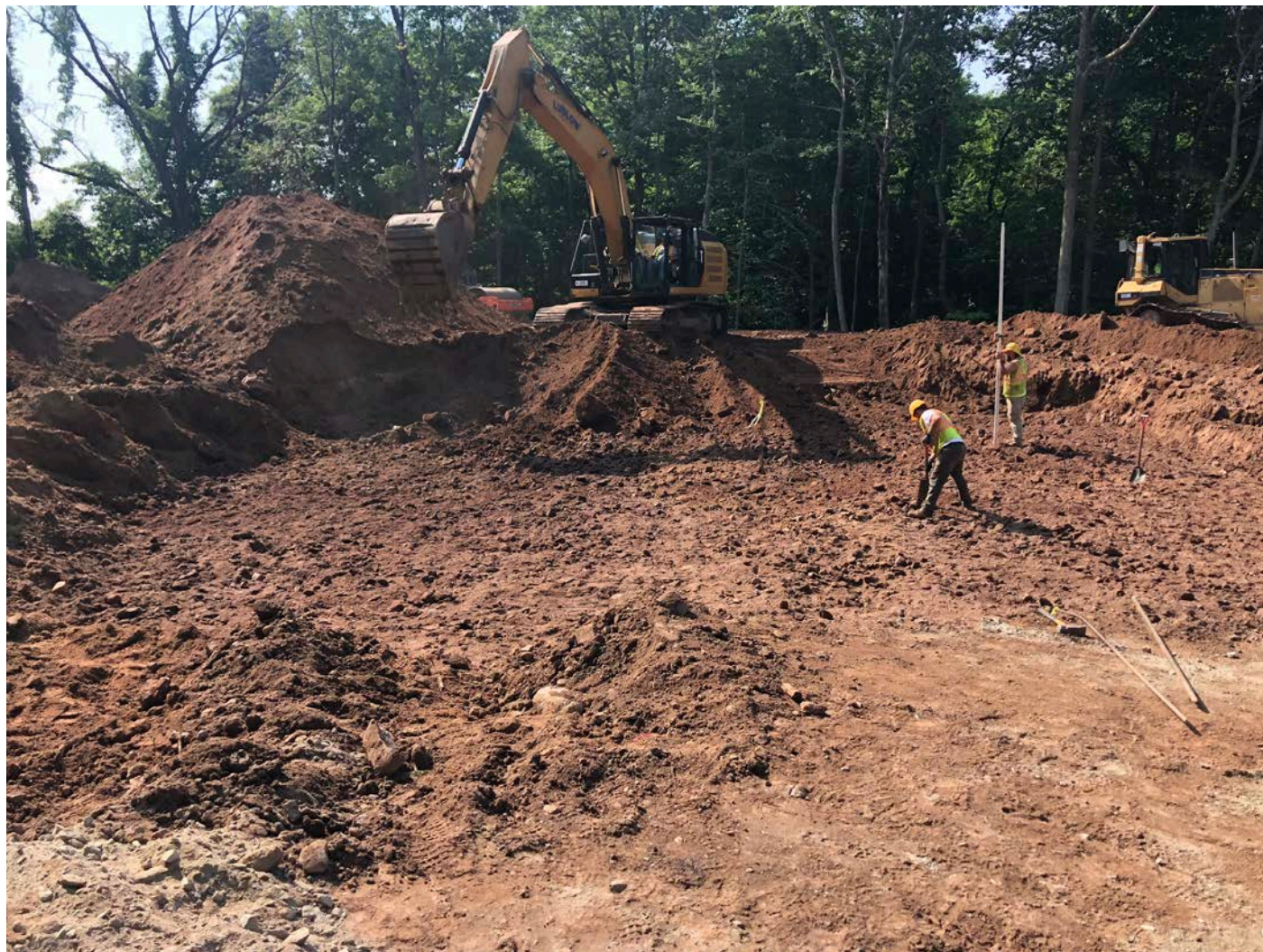
Picture 6: Ludlow excavating soil from the footprint of the water tank pad. Shared Access Driveway; view to the southeast.
