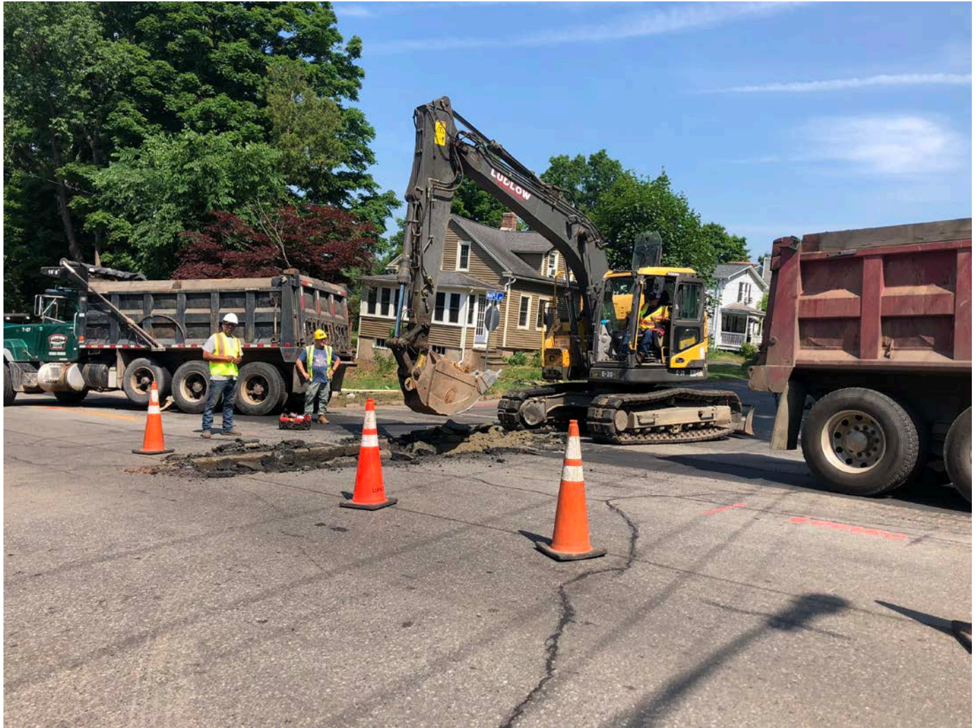
Picture 4: Ludlow excavating at the intersection of Maple Avenue and Route 68 to place 12" DIP at Station 920+65
