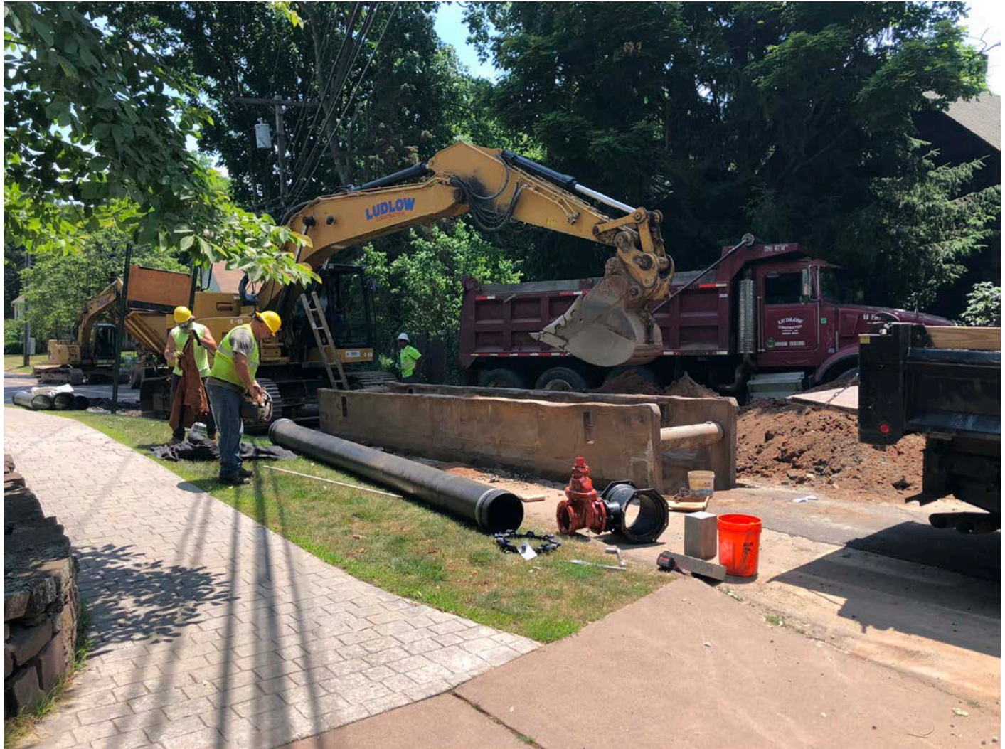
Picture 5: Ludlow installing 12" DIP at Station 400+74. Maiden Lane, Durham. View to the southeast
