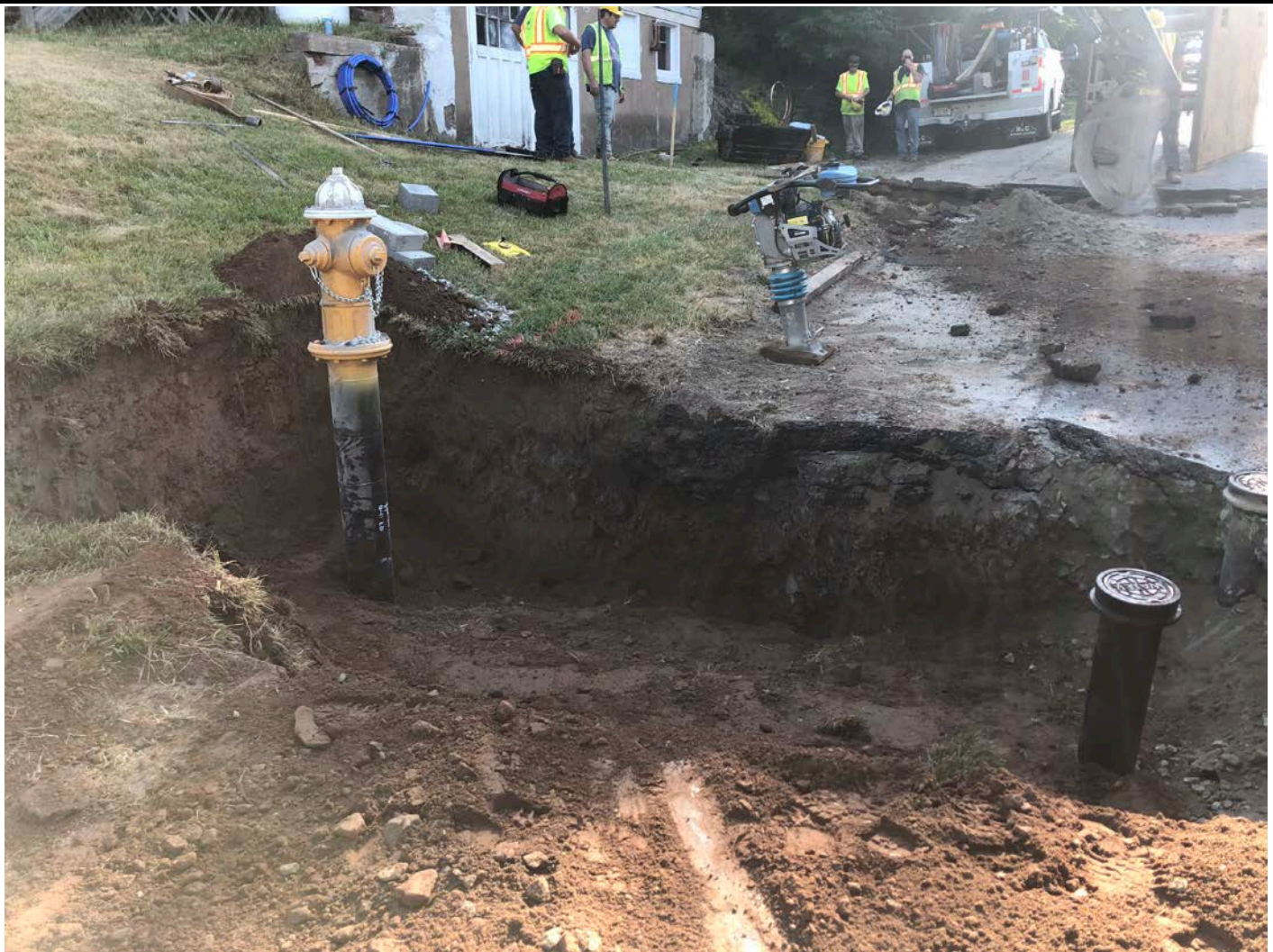
Picture 1: Ludlow installing hydrant at Station 609+46. Route 68; View to the east. Durham.
