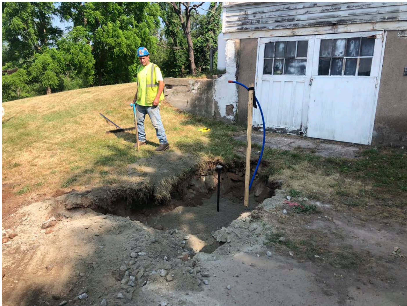
Picture 2: Ludlow installing a curb stop at Station 609+26 to service 47 Wallingford Road (Route 68). View to the north.
