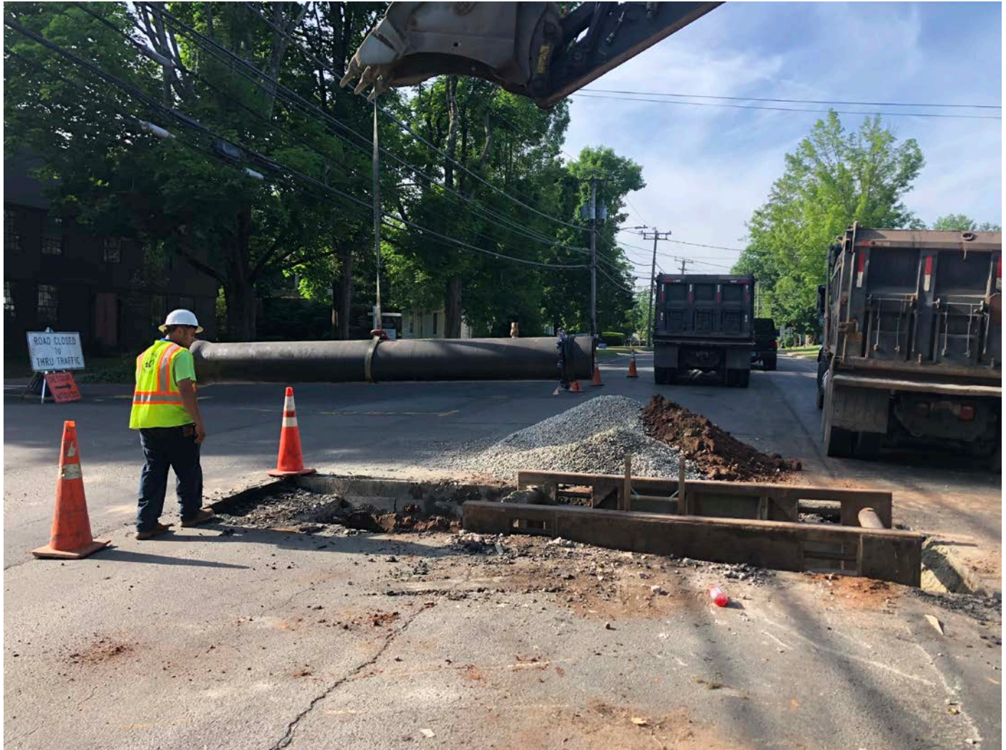
Picture 3: Ludlow installing 12" DIP across Main Street towards Maiden Lane to the east. Durham, view to the south.
