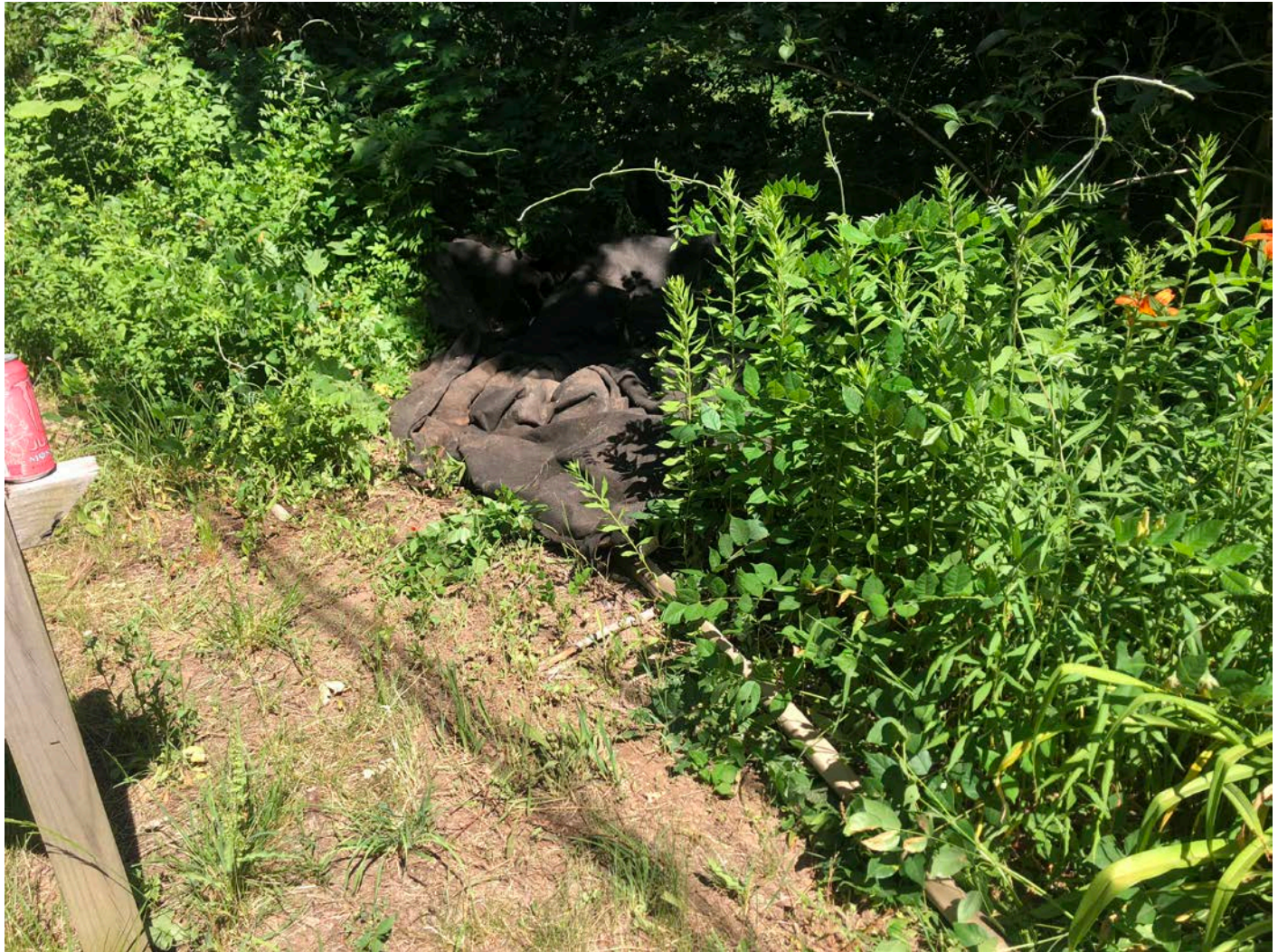
Picture 5: Ludlow discharging water pumped from the trench on Maiden Lane at ~Station 413+50 into a silt bag. View to the northwest.
