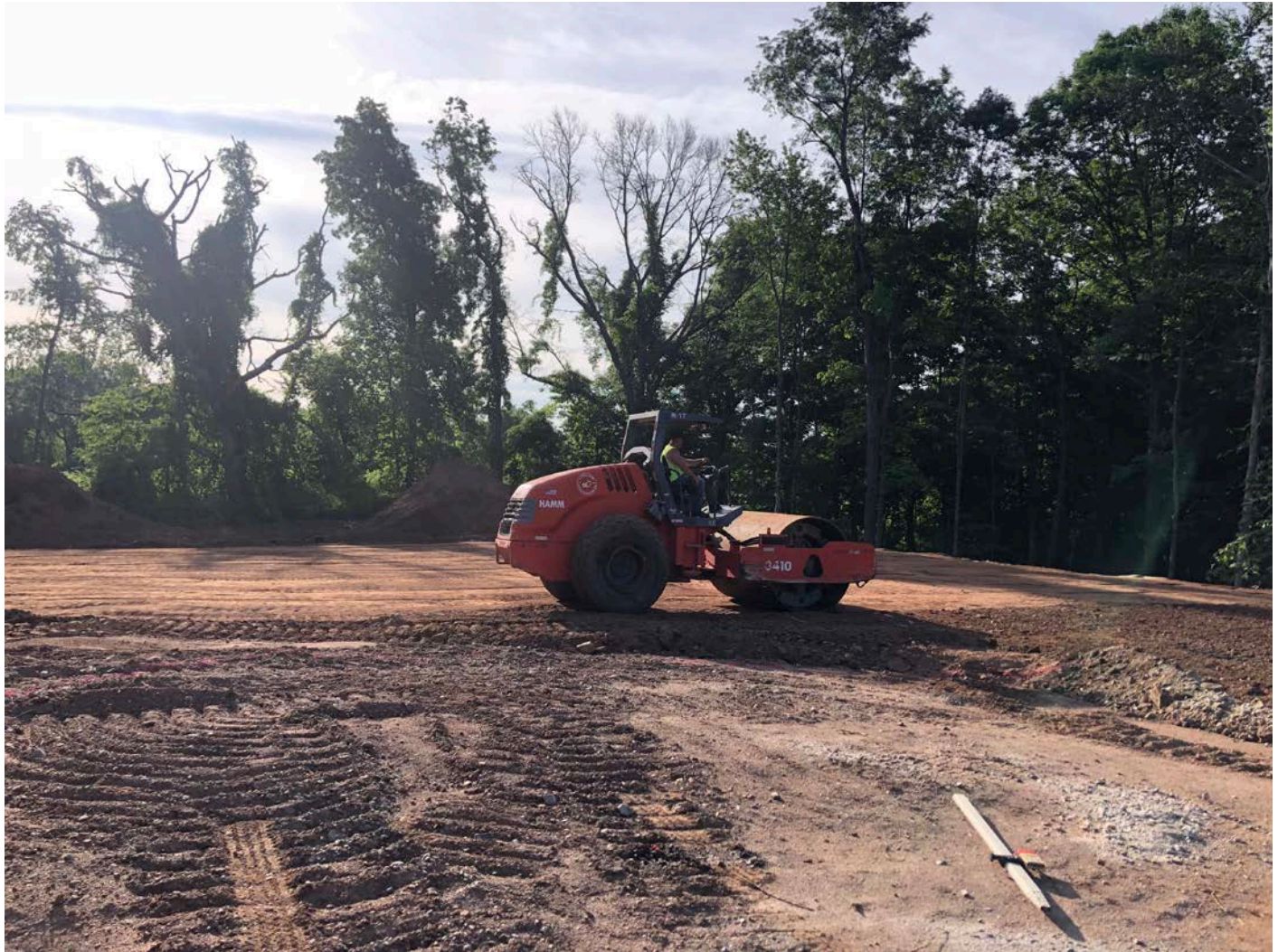
Picture 2: Ludlow compacting fill to the east of the water tank pad. Shared Access Driveway, Middletown. View to the southeast.
