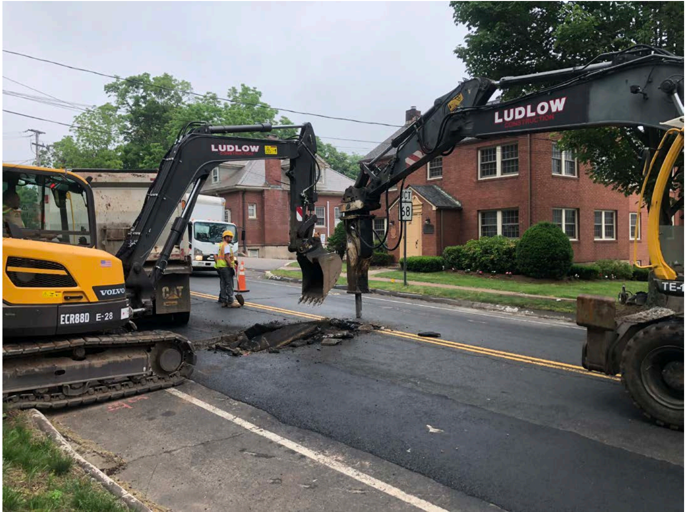
Picture 2: Ludlow beginning to excavate for the installation of a hydrant at Station 200+01; Main Street, Durham. View to the northeast.
