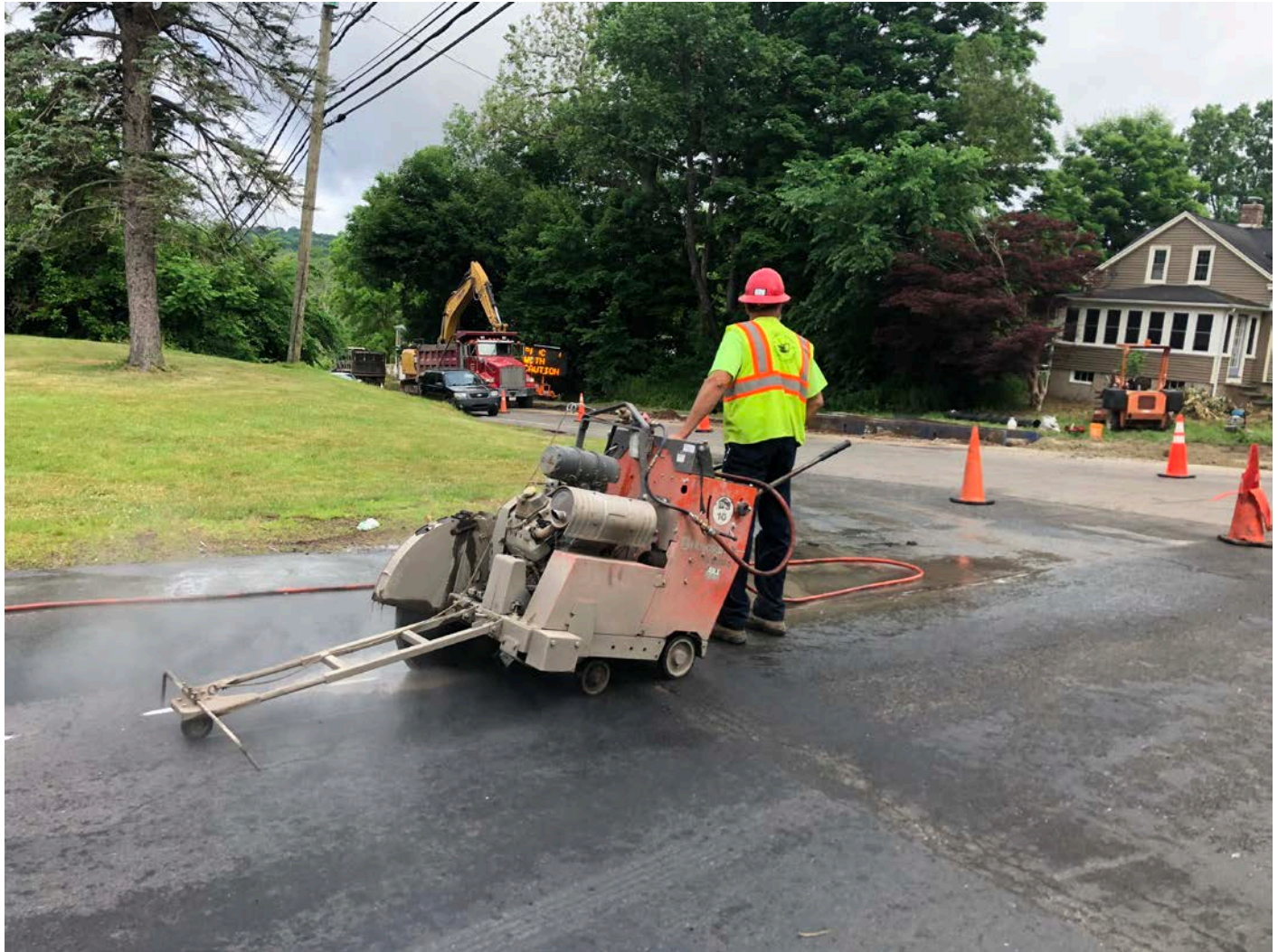
Picture 4: Ludlow saw cutting pavement at Station 920+00, on Maple Avenue, Durham. View to the northwest.
