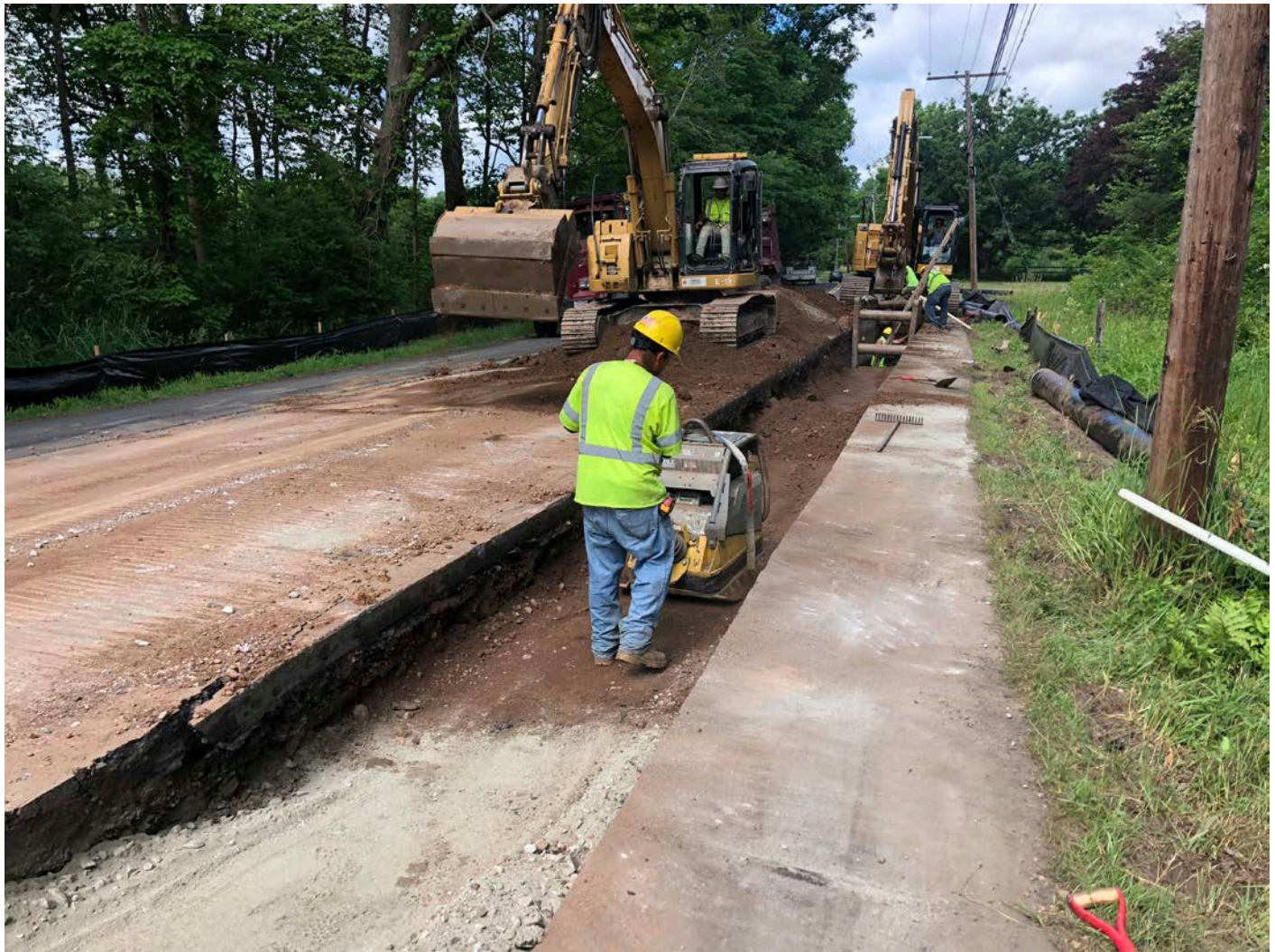
Picture 6: Ludlow compacting fill on Pickett Lane, Durham. View to the west.
