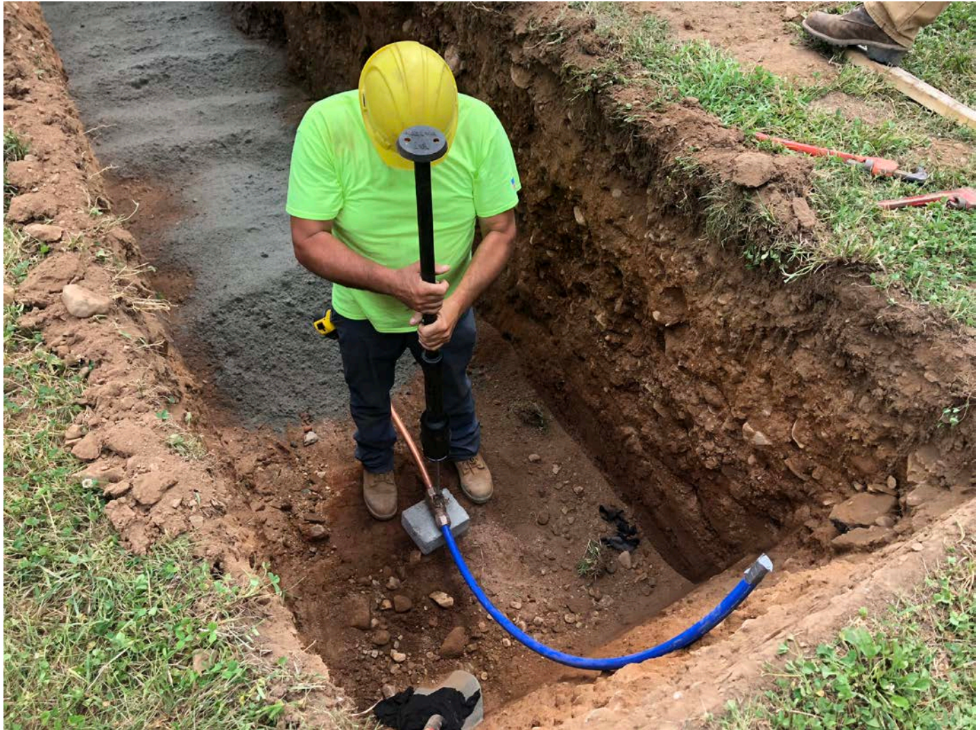
Picture 7: Ludlow installing 1" curb stop at Station 148+02. Main Street, Durham; view to the southeast.
