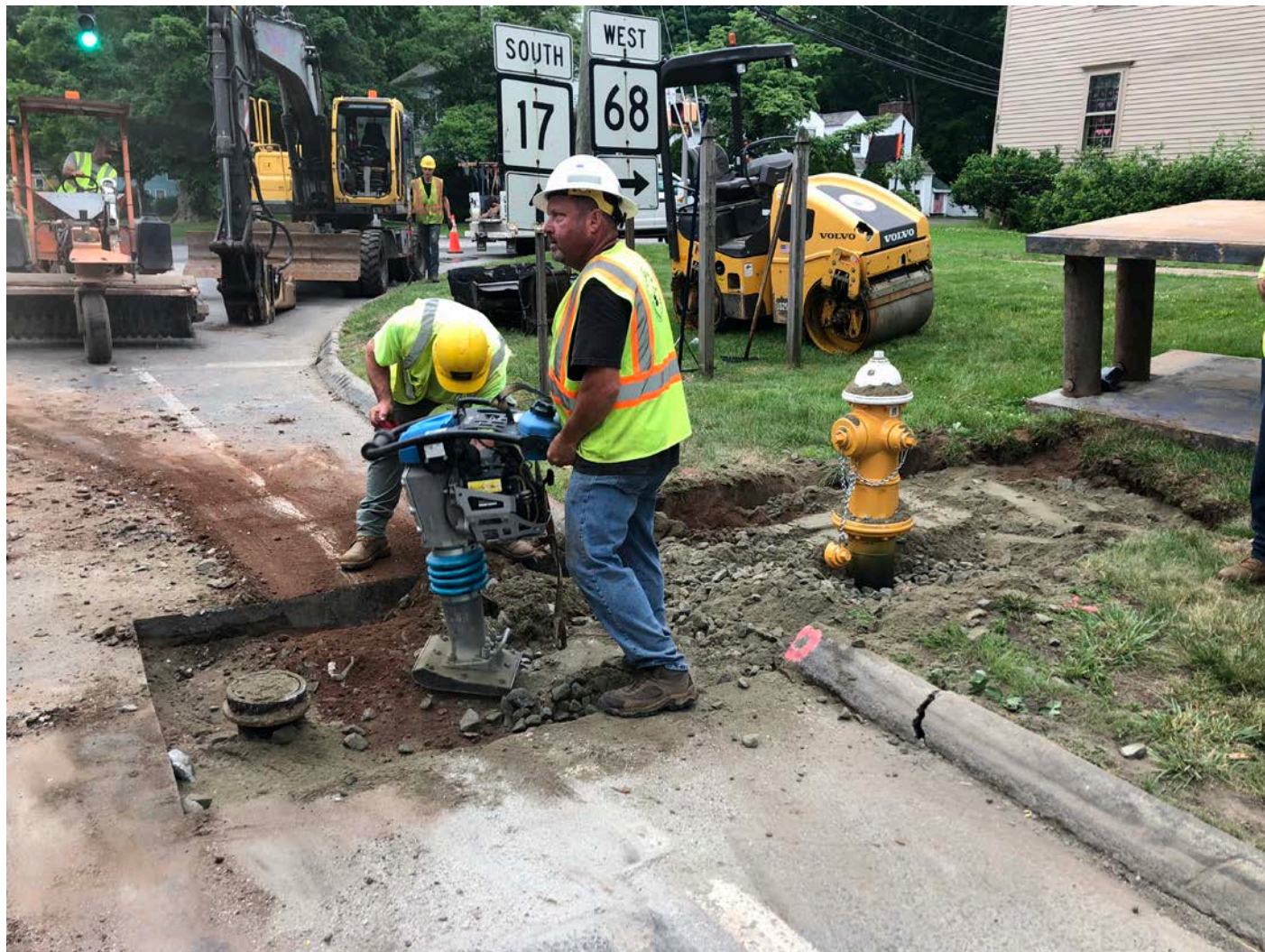
Picture 2: Ludlow compacting fill around newly installed hydrant at Station 194+50. View to the south, Main Street, Durham.
