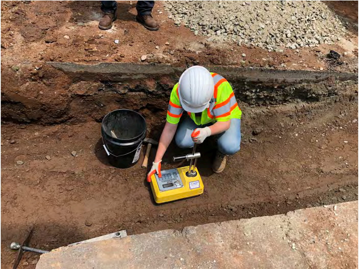
Picture 4: JTC performing soil compaction test at Station 143+22, Main Street, Durham.
