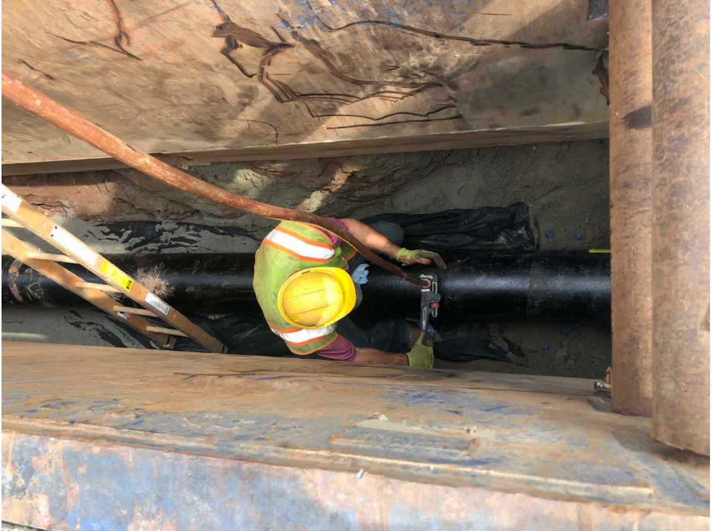
Picture 2: Ludlow installing a 1" copper chlorination inlet at Station 600+02, Route 68, Durham.
