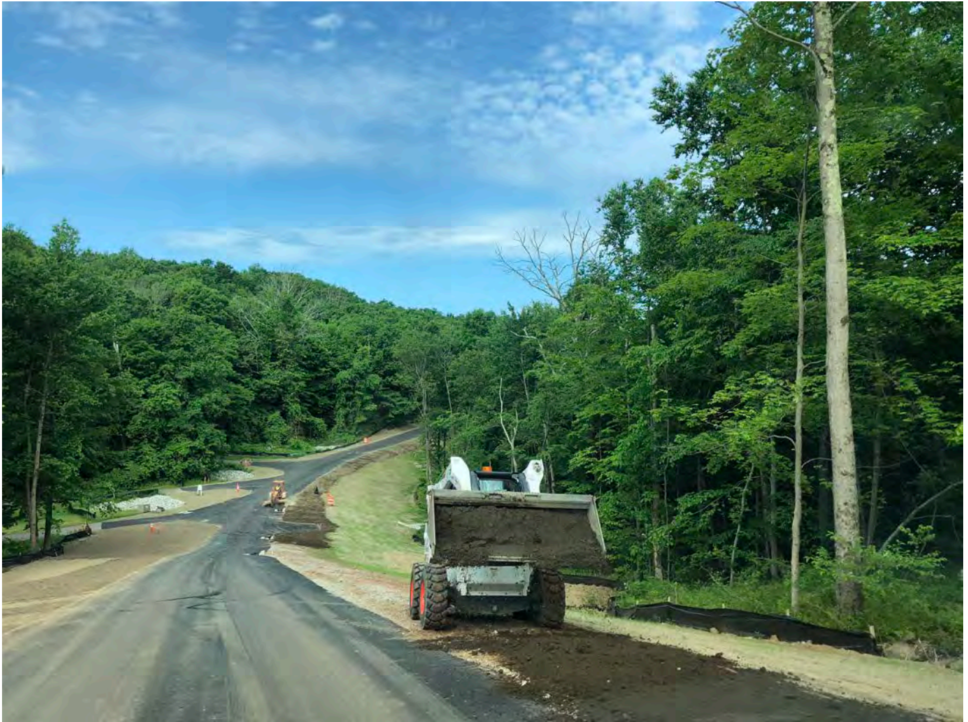
Picture 4: Ludlow placing loam on the north side of the Shared Access Road. View to the west. Middletown, CT.
