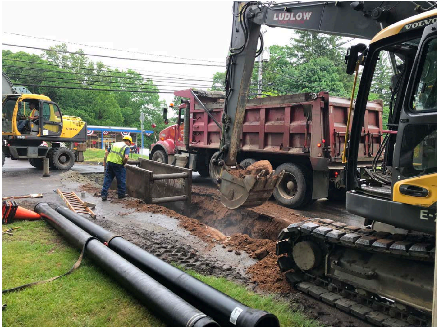
Picture 8: Ludlow placing 8" DIP on Talcott Lane. View to the southeast. Durham, CT.
