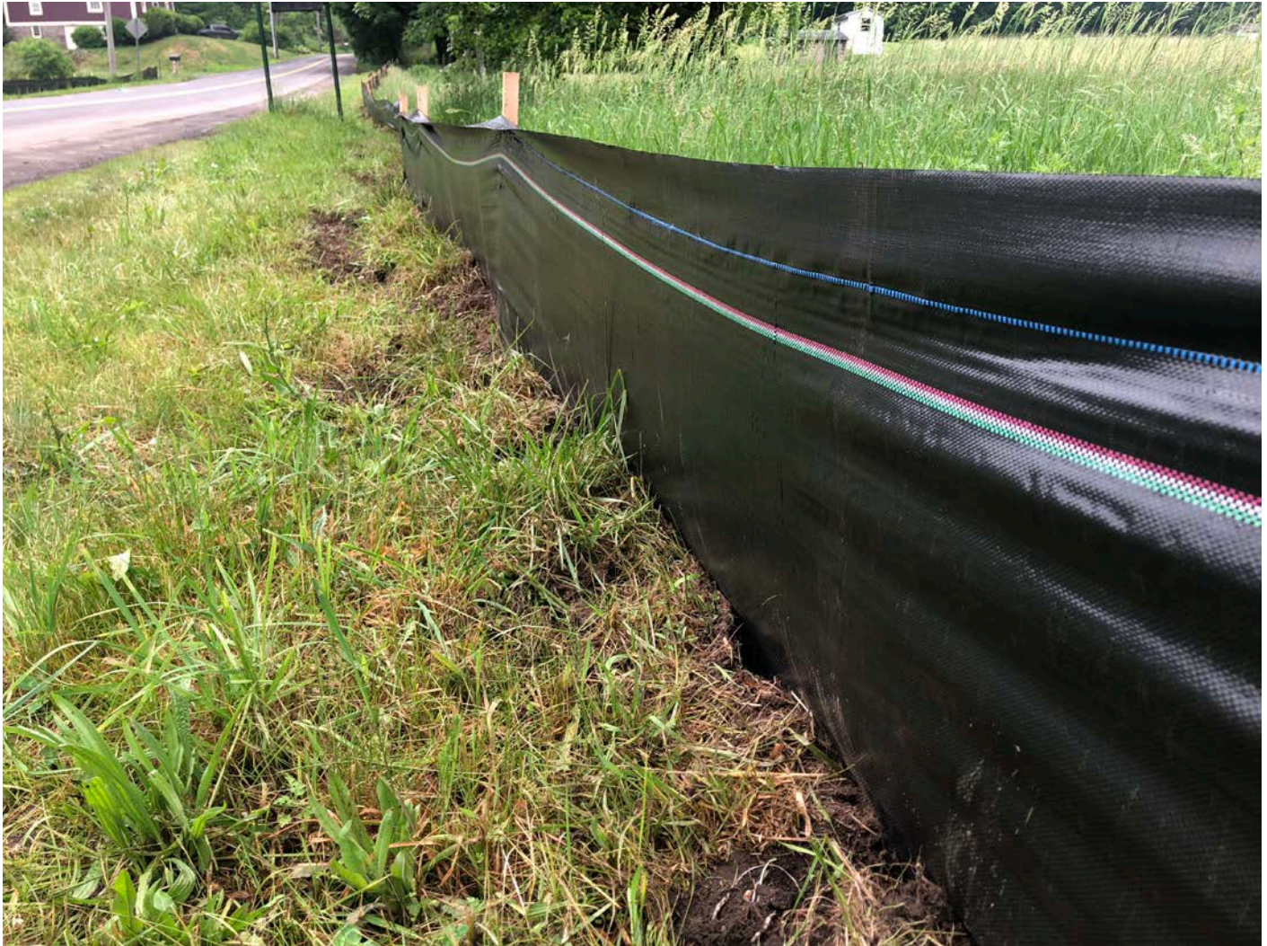
Picture 4: Bottom of silt fence secured below grade by Ludlow. View to the west. Maiden Lane, Durham, CT.
