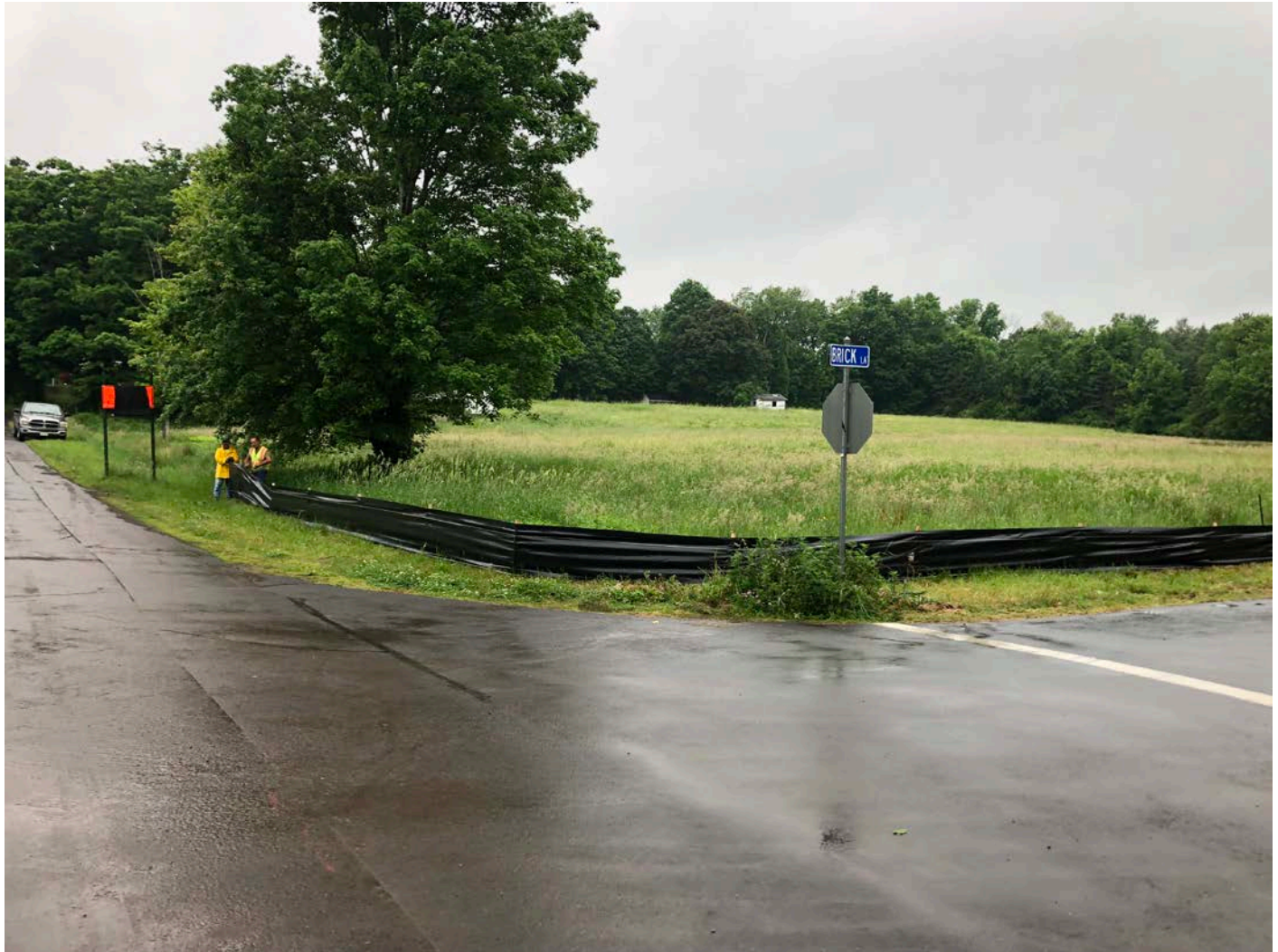
Picture 3: Ludlow at the intersection of Brick Lane and Maiden Lane, placing silt fence. View to the west. Durham, CT.
