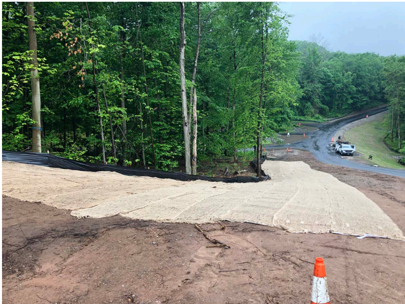
Picture 2: South side of the shared access driveway after being seeded and having erosion control blankets placed over seed. View to the west. Middletown, CT.
