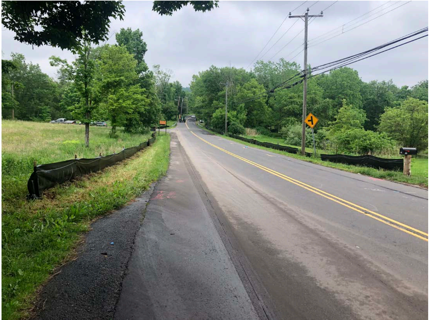
Picture 5: Silt fence placed by Ludlow on Maiden Lane. View to the east. Durham, CT.
