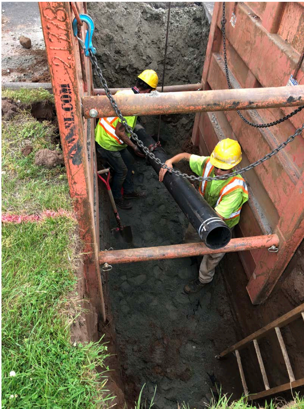
Picture 6: Ludlow installing 6" DIP as part of hydrant installation at Station 169+72, southbound lane of Main Street, Durham. View to the east.
