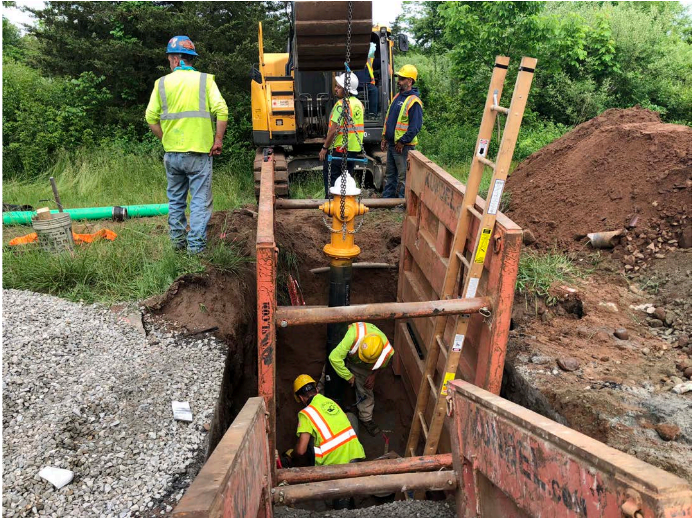
Picture 3: Ludlow installing hydrant on Main Street, Durham, at Station 161+00. View to the west.
