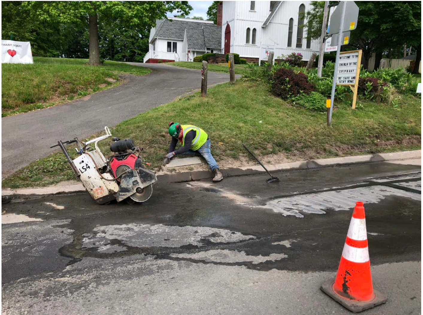
Picture 1: NY-CONN installing a traffic loop at Station 201+10. Main Street, Durham. View to the west.
