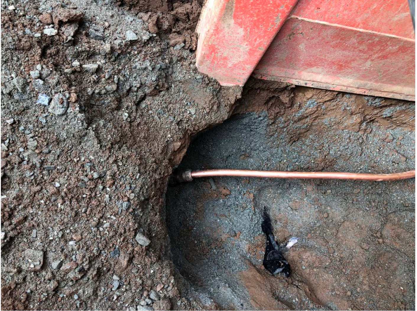
Picture 4: 1" copper water line connected to corporation stop on 16" main water line. Station 122+53, South Main Street, Middletown.
