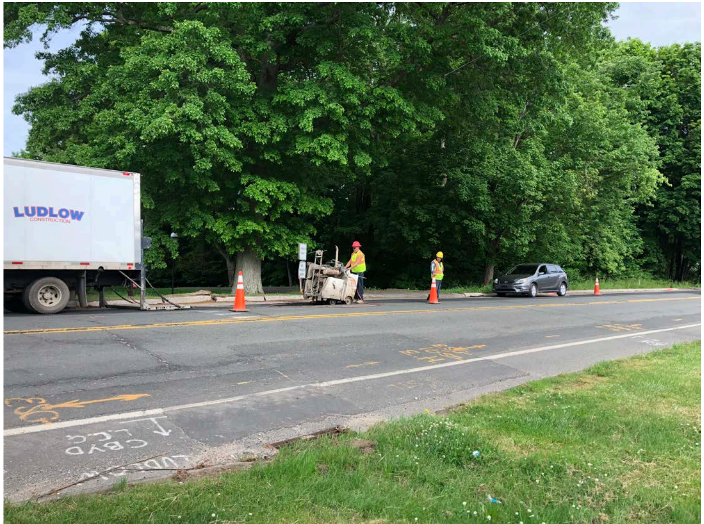
Picture 2: Ludlow saw cutting pavement on the southbound lane of Main Street in Durham at Station 183+50.
