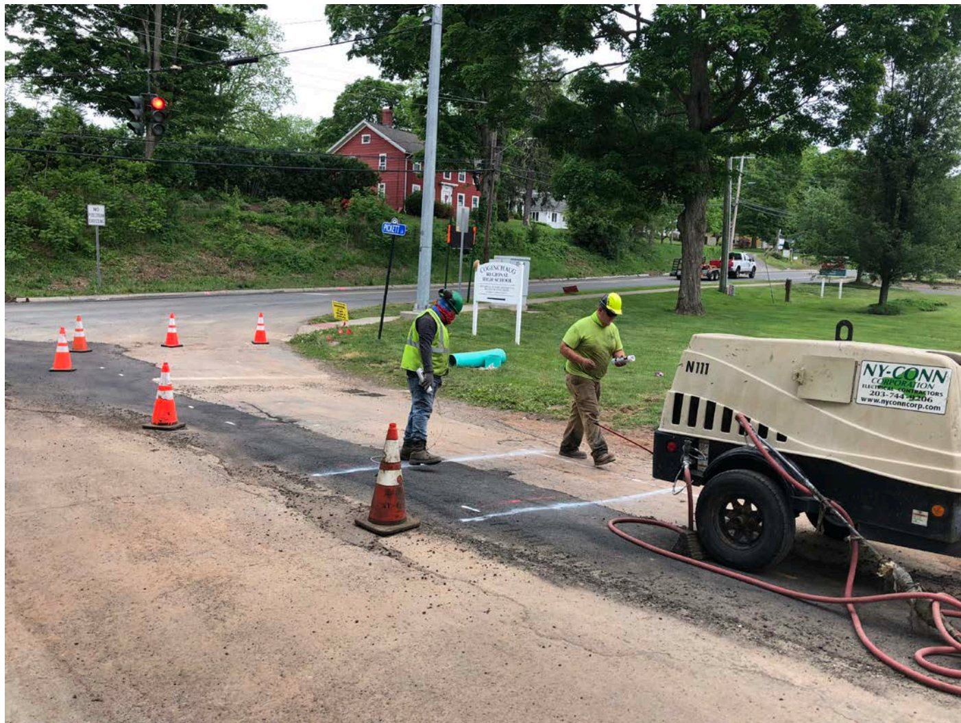
Picture 5: NY-CONN installing a traffic loop at ~Station 500+25. Pickett Lane, Durham. View to the northwest.
