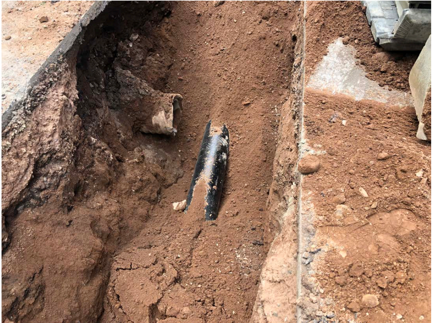
Picture 6: Storm drain pipe that was cut during the installation of 12" DIP on Pickett Lane at ~Station 500+55. View to the west.
