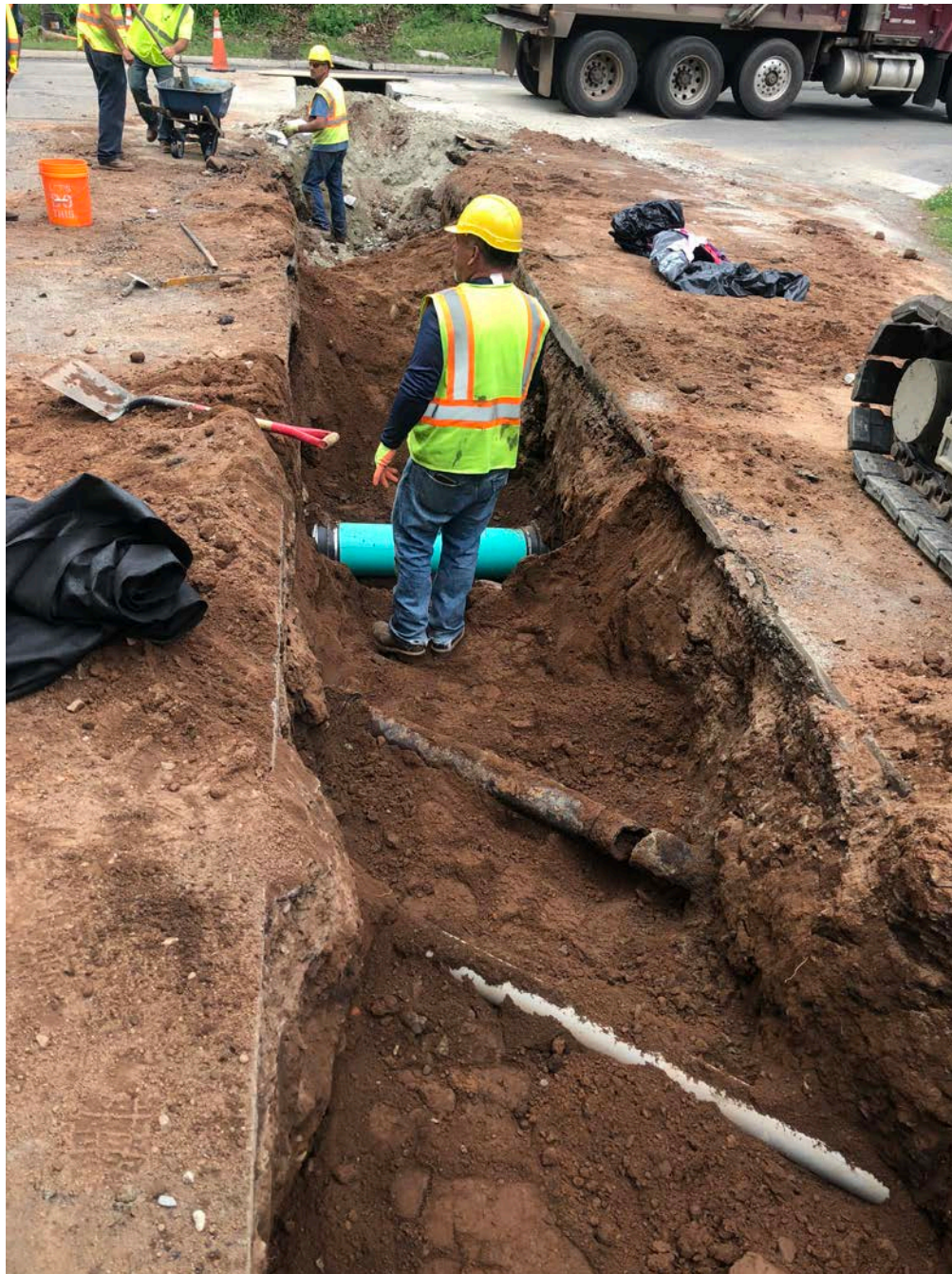
Picture 8: PVC conduit and broken cast iron conduit daylighted at ~Station 500+65 during the installation of 12" DIP on Pickett Lane, Durham. View to the west.
