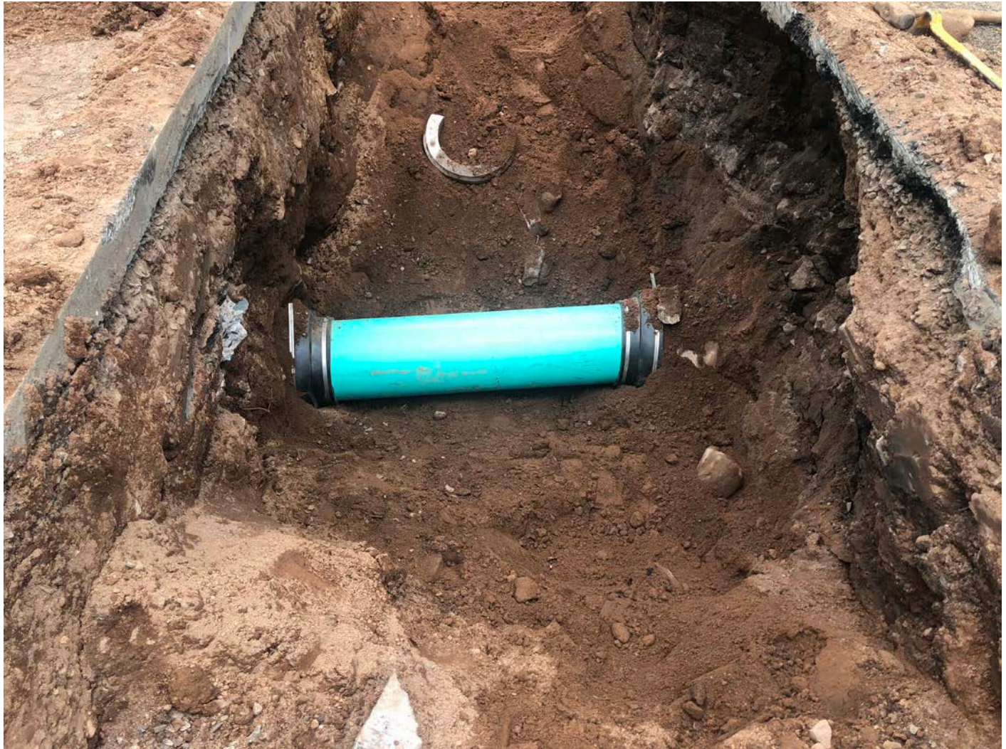
Picture 7: Repair of corrugated steel storm drain pipe that was cut during the installation of 12" DIP on Pickett Lane at ~Station 500+55. View to the west.
