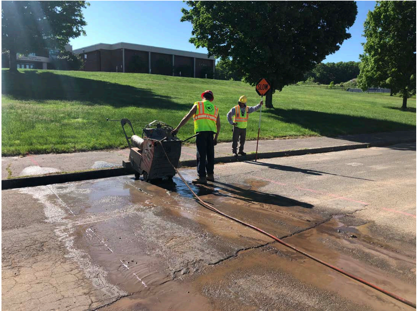
Picture 2: Ludlow saw cutting on Pickett Lane, Durham. View to the southeast.
