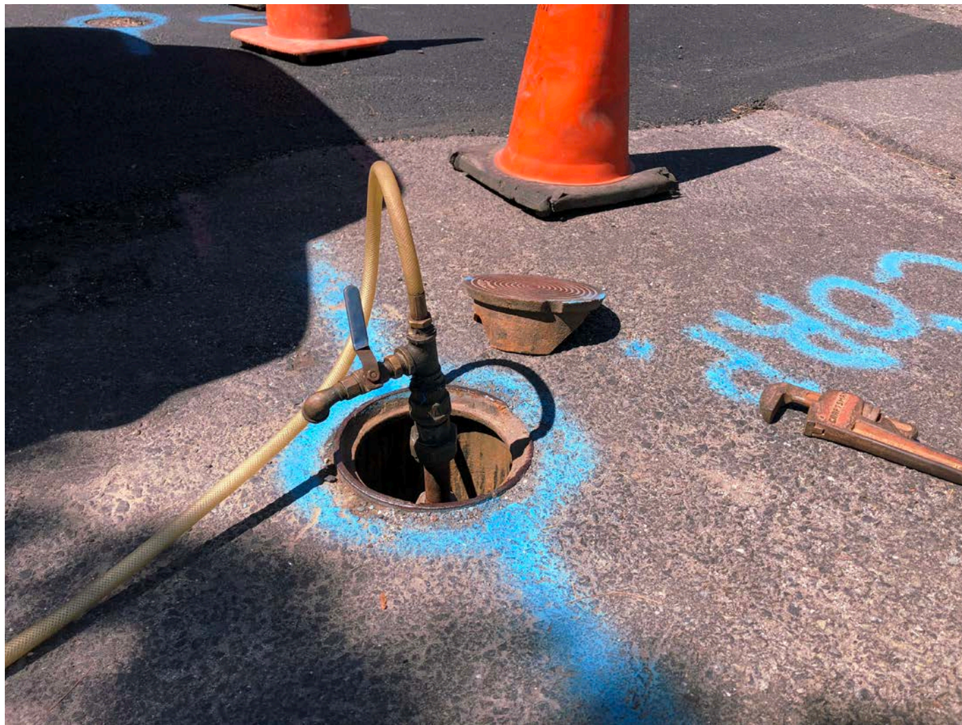
Picture 5: JWS Connections injecting sodium hypochlorite into water line at intersection of Talcott Ridge Drive and Main Street. View to the southwest.
