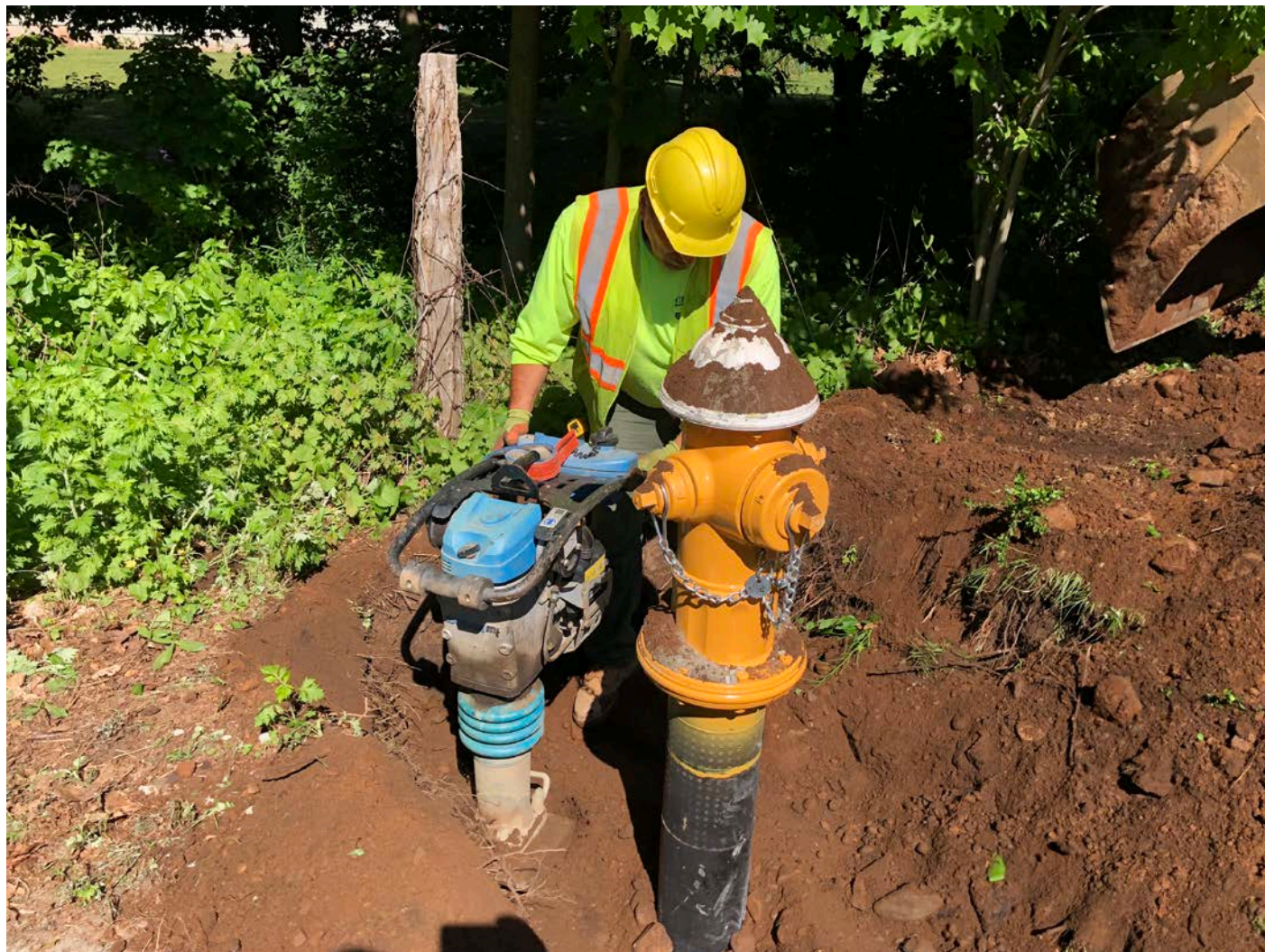
Picture 4: Ludlow compacting backfill around hydrant installed at Station 534+30. Pickett Lane, Durham. View to the northwest.
