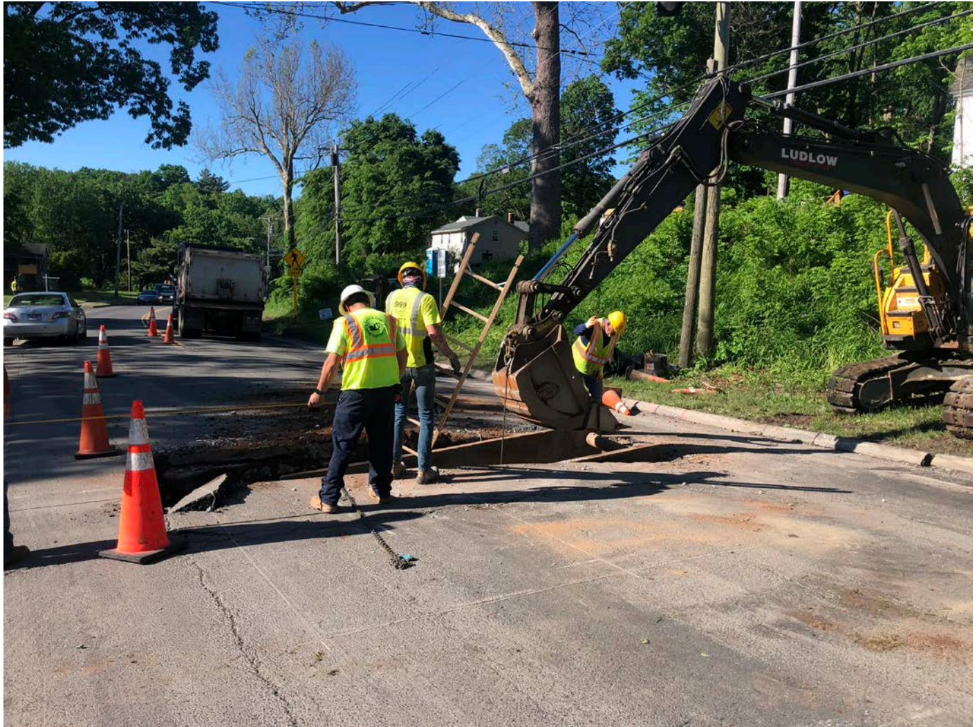
Picture 1: Ludlow begins excavation for placement of 12" DIP at intersection of Pickett Lane and Main Street. Station 500+03, Main Street, Durham. View to the southwest.
