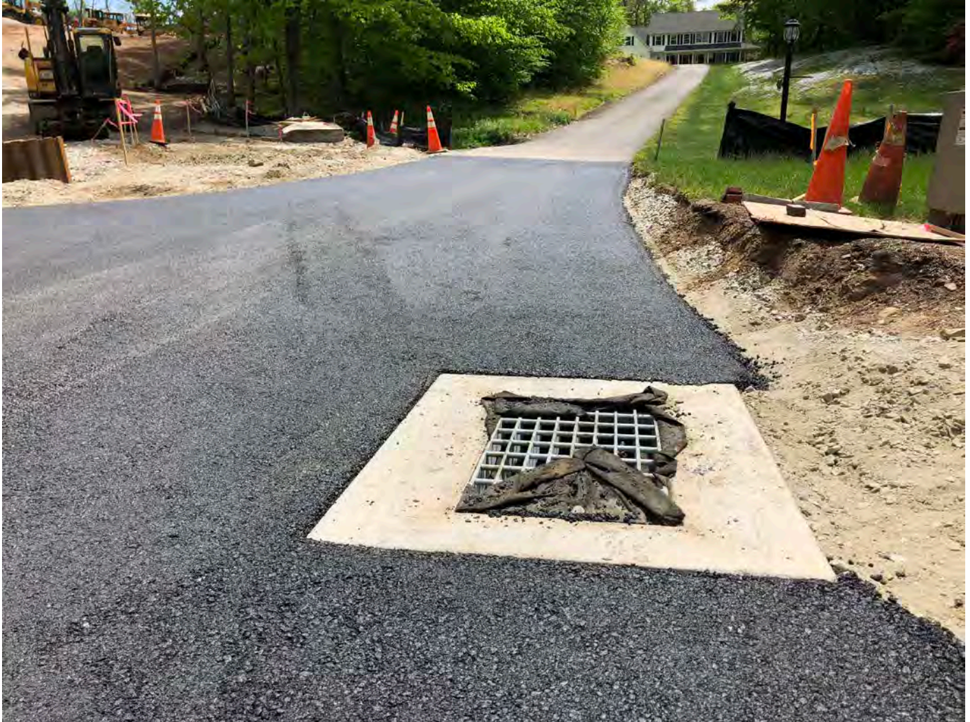
Picture 7: Base coat of pavement surrounding catch basin next to the driveway entrance for 214 Talcott Ridge Drive.. View to the southeast. Middletown, CT
