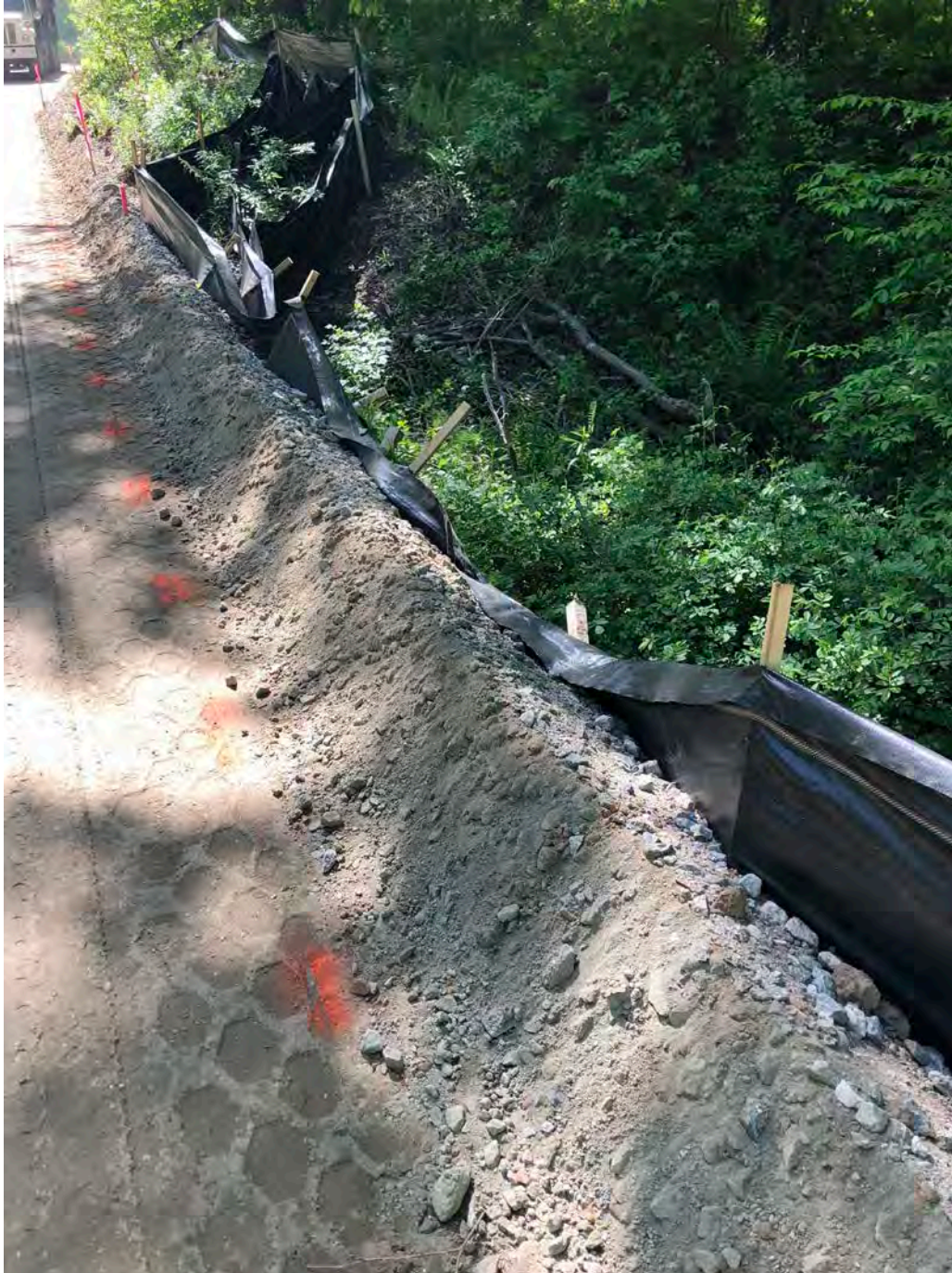
Picture 3: Silt fence on the south side of the Shared Access Driveway at Station 19+85 showing encroachment from fill. View to the east. Middletown, CT.
