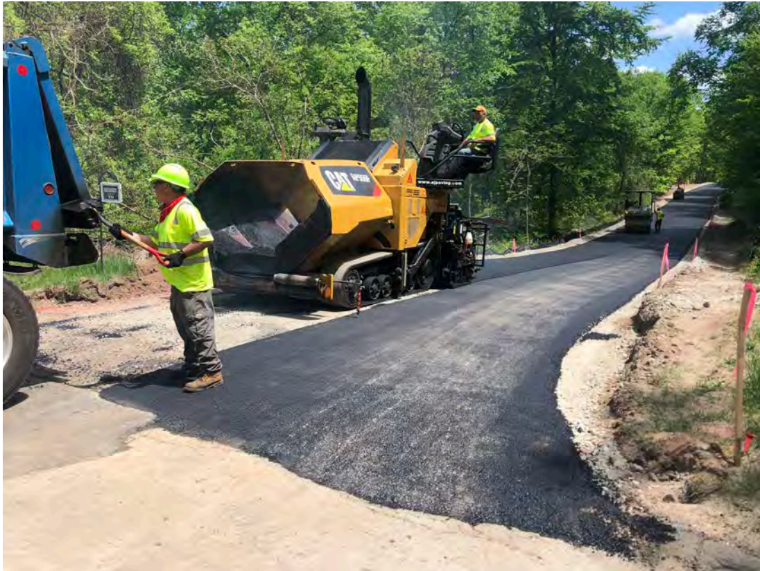
Picture 8: A&J Construction finishing the paving of the Shared Access Driveway. View to the east. Middletown, CT
