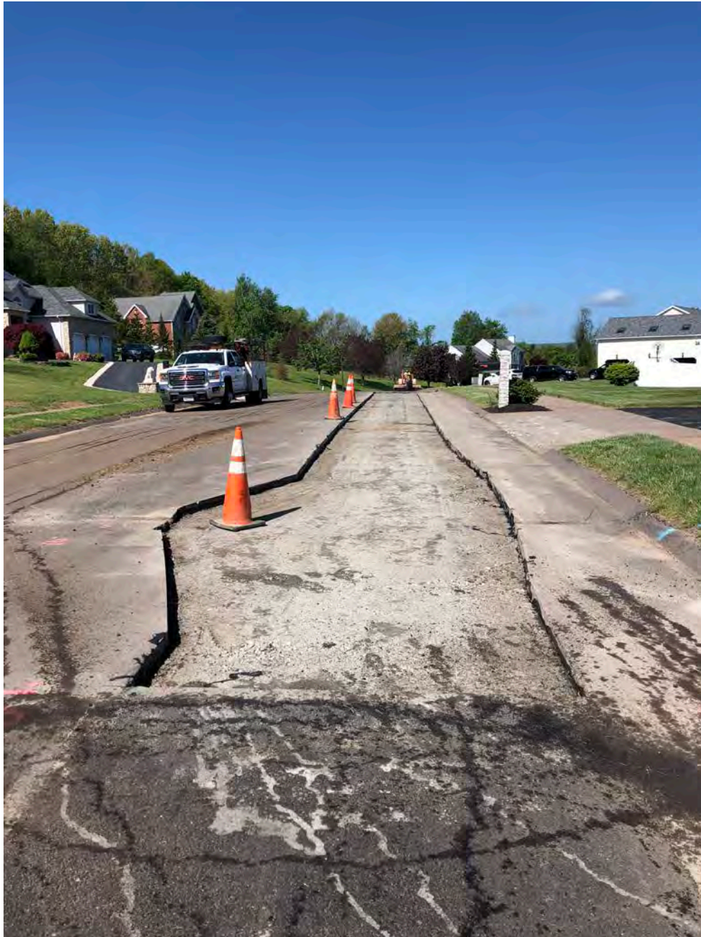
Picture 2: Asphalt removed from 12" cutbacks on Watch Hill Drive from Stations 603+06 to 604+44. Middletown, CT.
