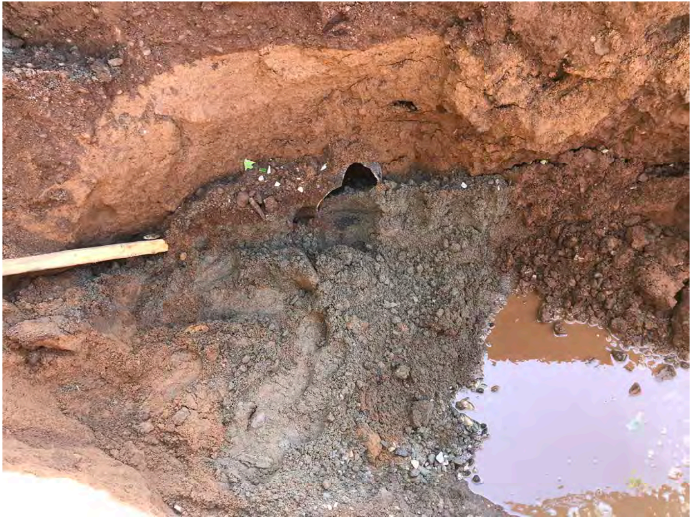
Picture 1: 8" PVC sewer pipe that Ludlow encountered at Station 275+86. Pickett Lane, Durham, CT.
