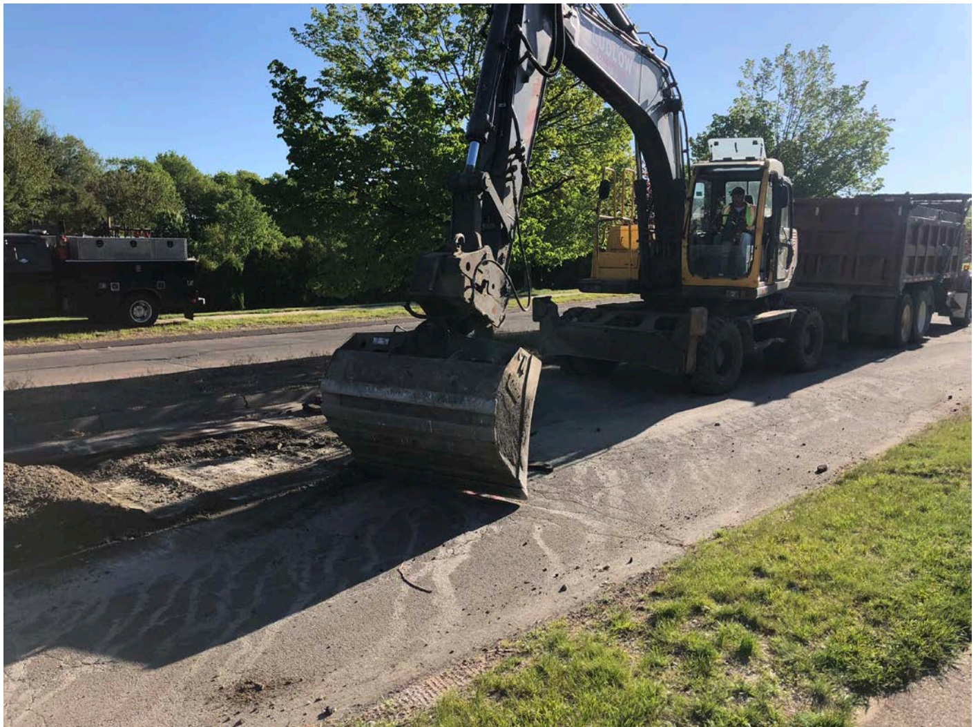
Picture 1: Ludlow peeling asphalt back from trench on Talcott Ridge Lane at ~Station 49+50. Middletown, CT.
