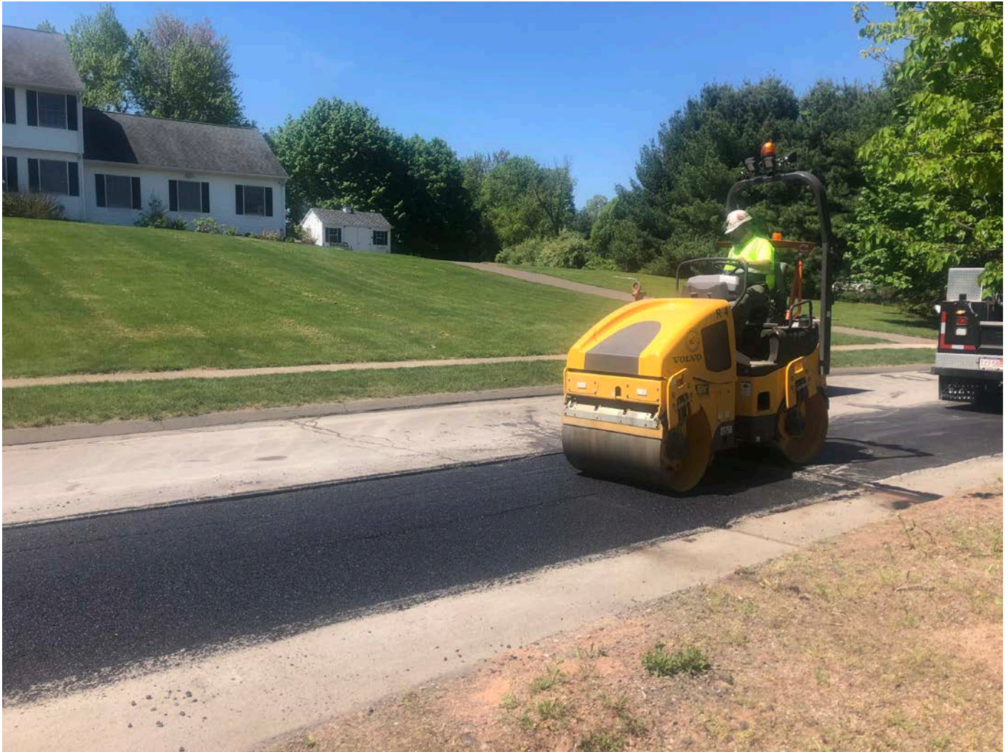
Picture 6: Ludlow compacting first lift of asphalt at ~Station 51+00.
