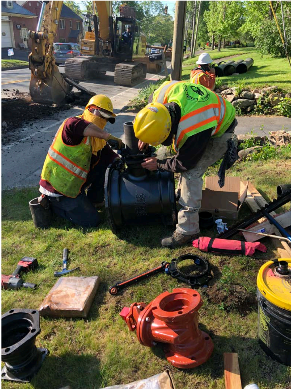
Picture 4: Ludlow assembling 16" x 16" x 4" M.J. TEE for placement at Station 198+02.
