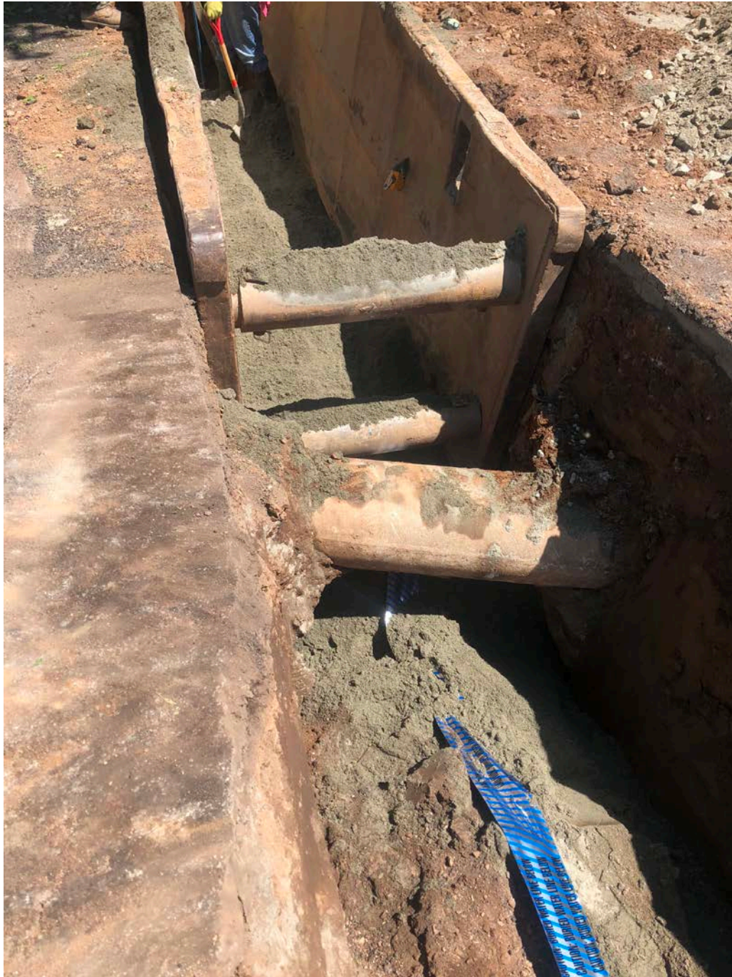
Picture 7: Ludlow daylighting a storm drain pipe at approximately Station 525+95. View to the south. Pickett Lane, Durham.
