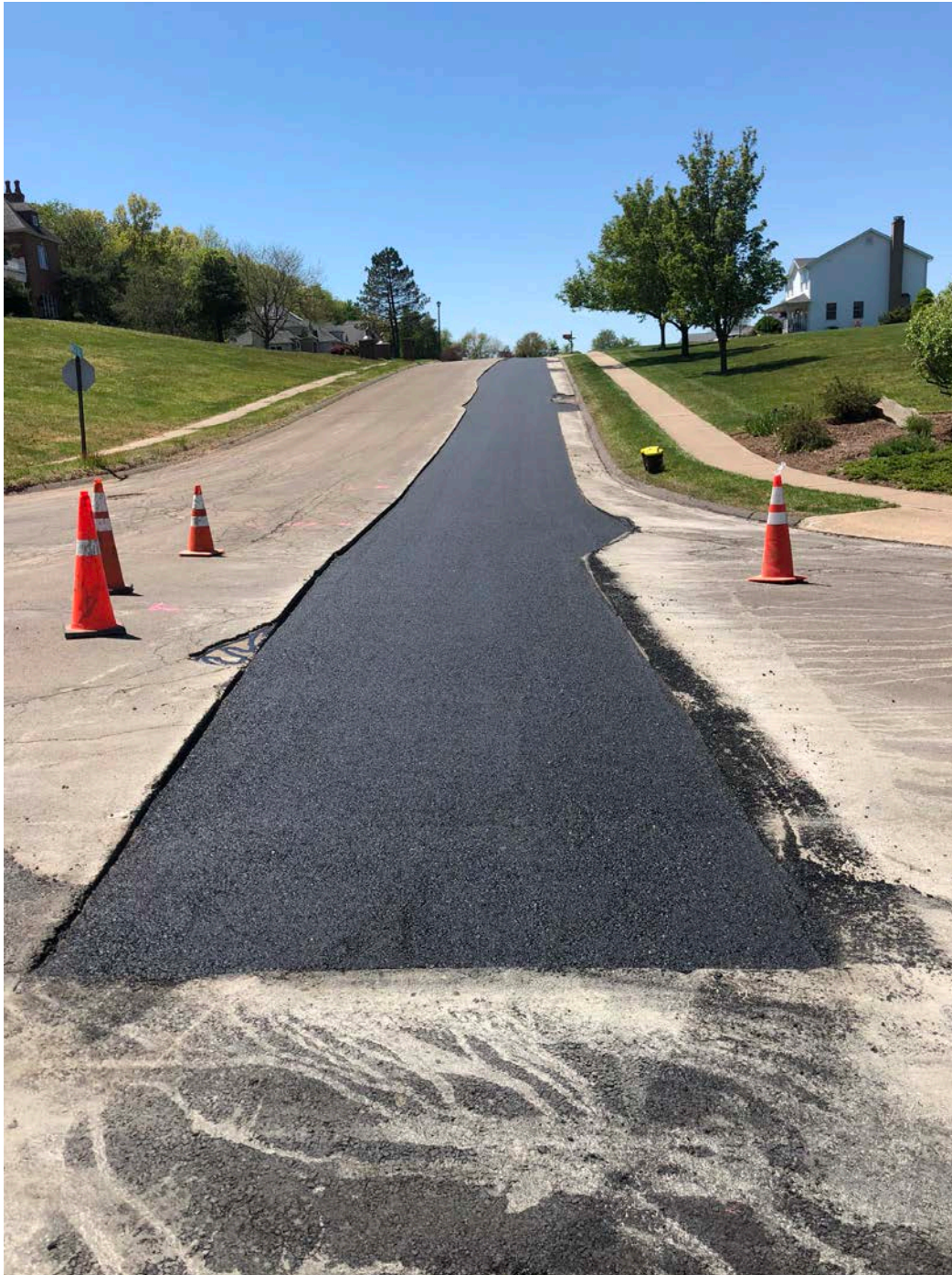
Picture 8: View of first lift of asphalt placed from Station 600+00 to 603+00. View to the west. Watch Hill Drive, Middletown, CT.
