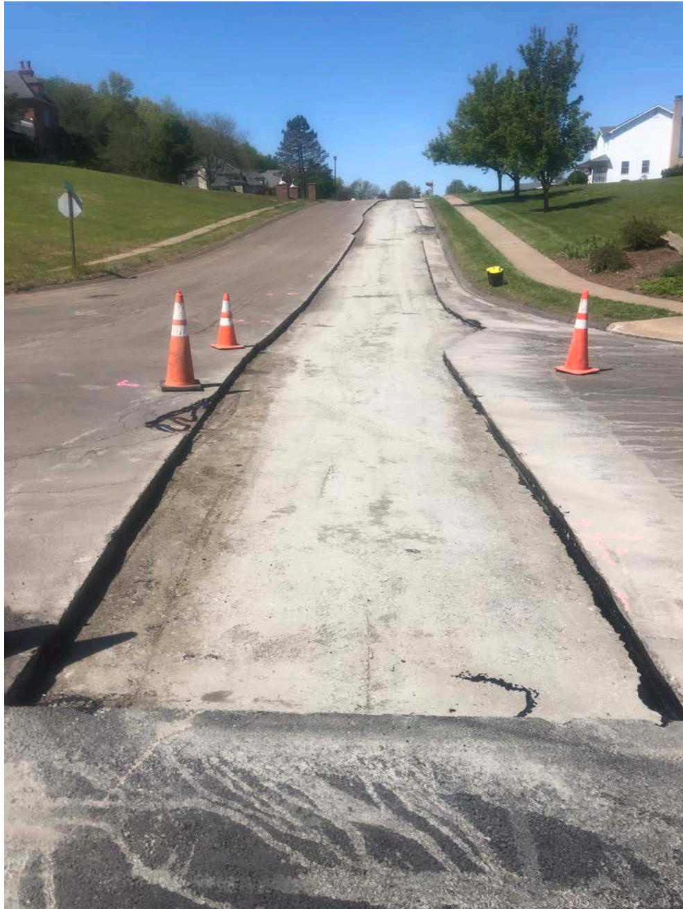
Picture 3: View of asphalt cut back prior to first lift of asphalt. Watch Hill Drive from Station 600+00 to 603+00. Middletown, CT.
