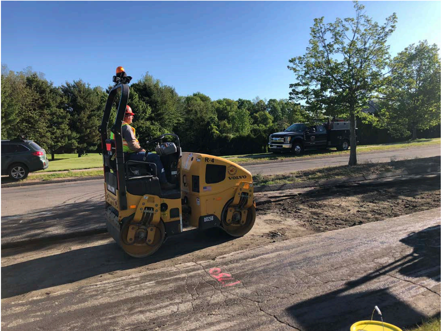
Picture 2: Ludlow compacting road base on Talcott Ridge Drive at ~Station 51+50 after removing temporary asphalt patch. Middletown, CT.
