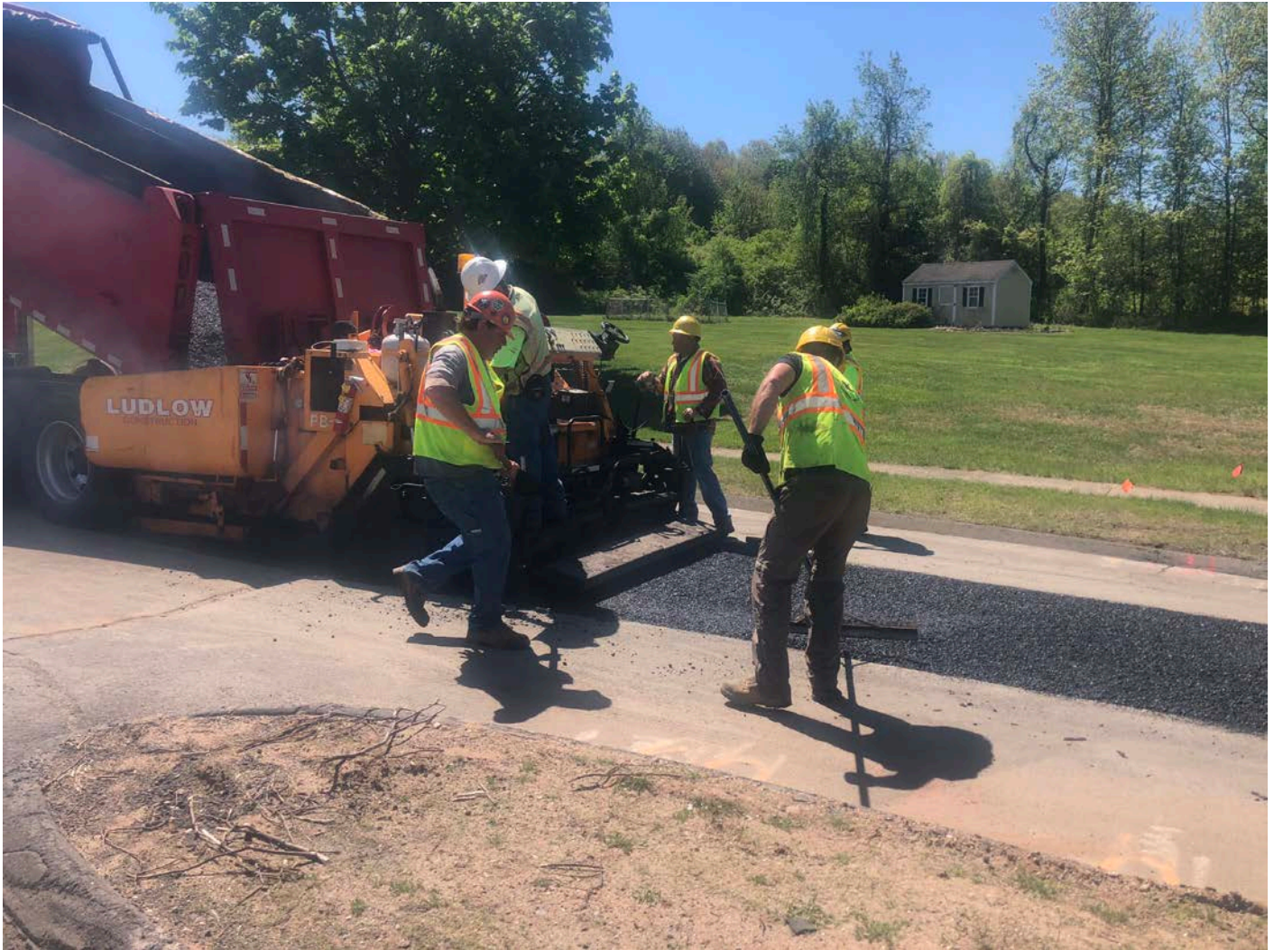
Picture 5: Ludlow placing first lift of asphalt from Station 50+00 to ~Station 47+50. Middletown, CT.
