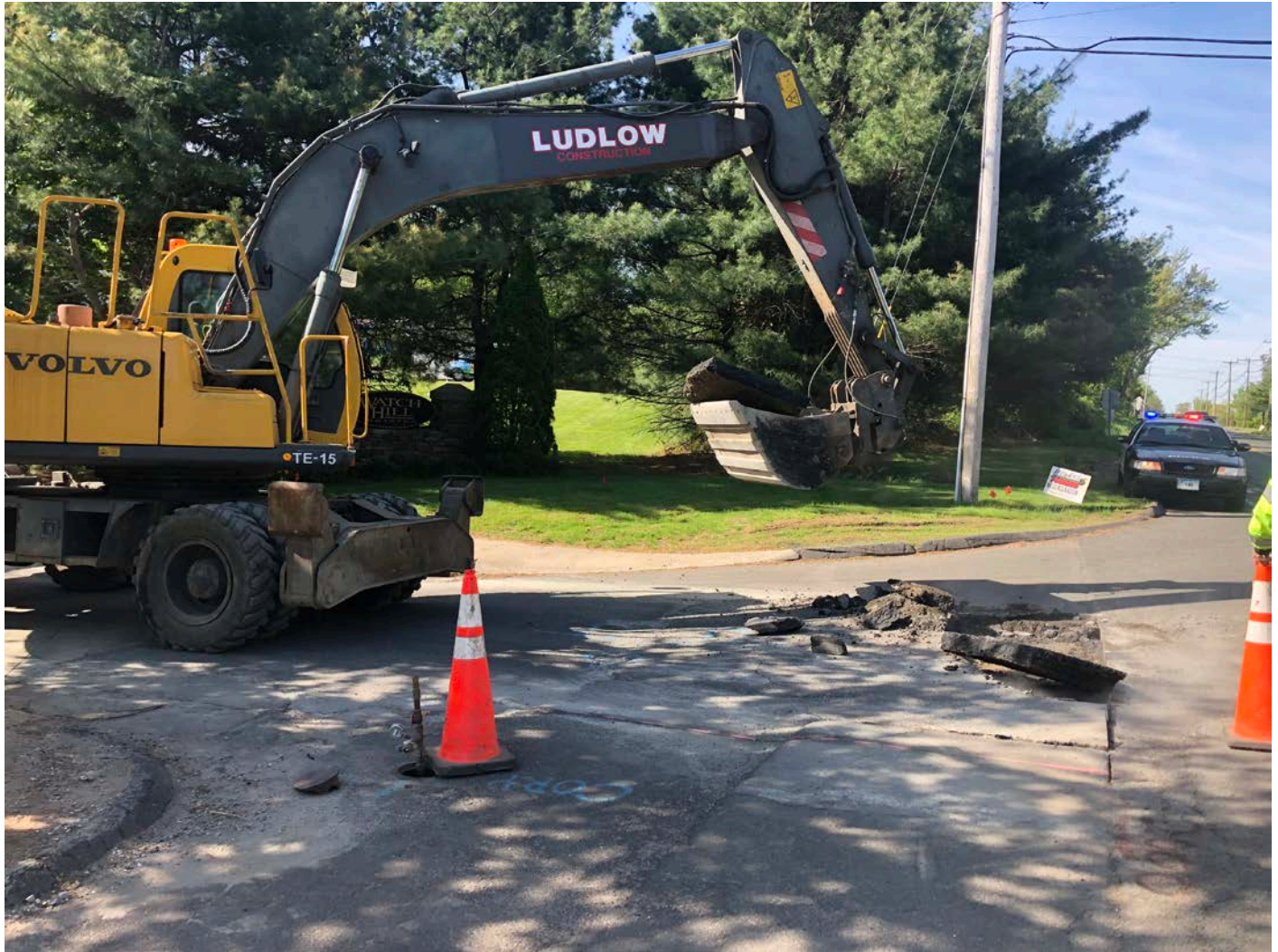
Picture 2: Ludlow peeling asphalt back on 12" cutbacks at the intersection of Talcott Ridge Drive and South Main Street. View to the south. Middletown Connecticut.
