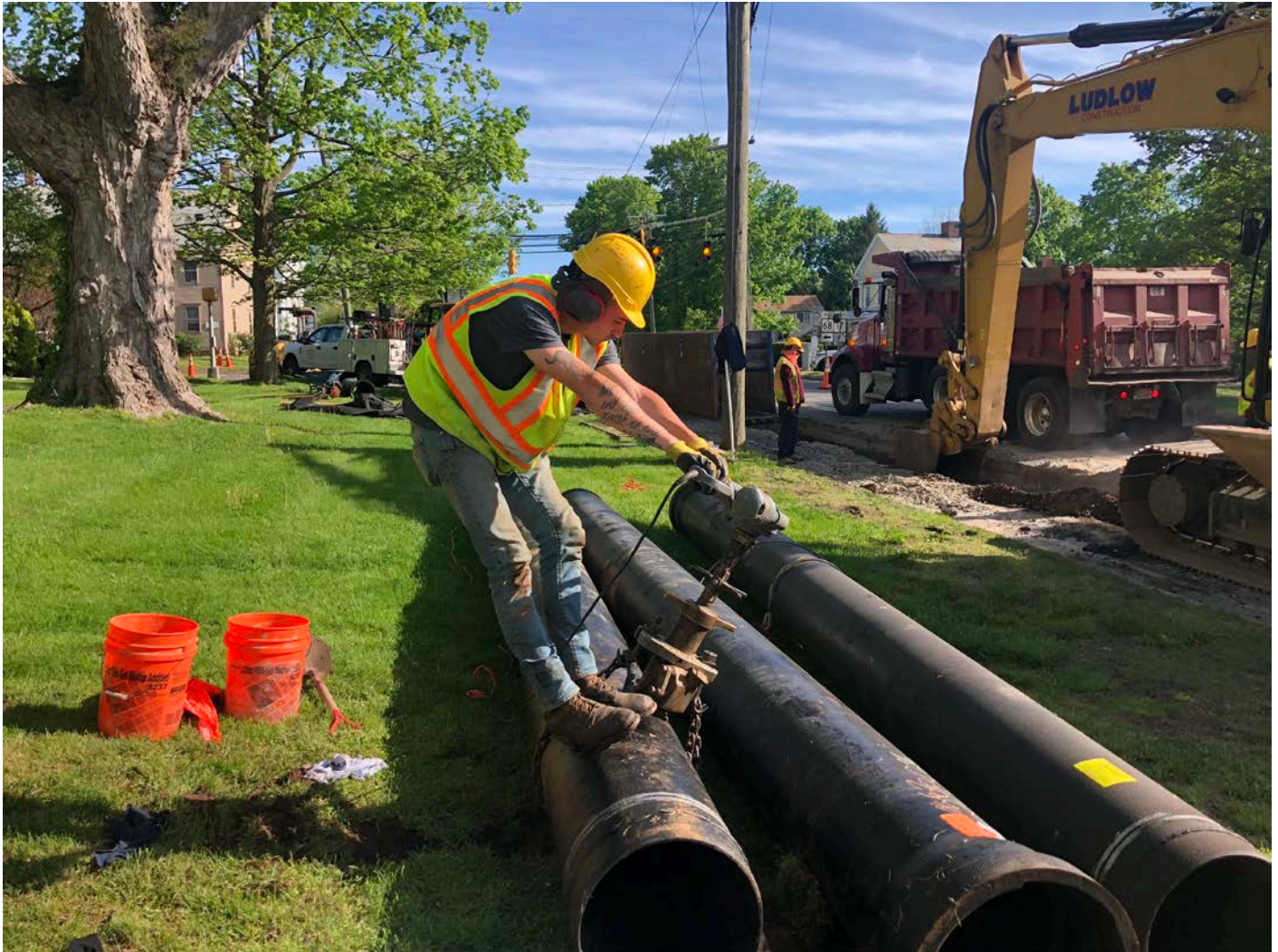
Picture 1: Ludlow taps 16" DIP to add a corporation stop. Main Street, Durham, CT.
