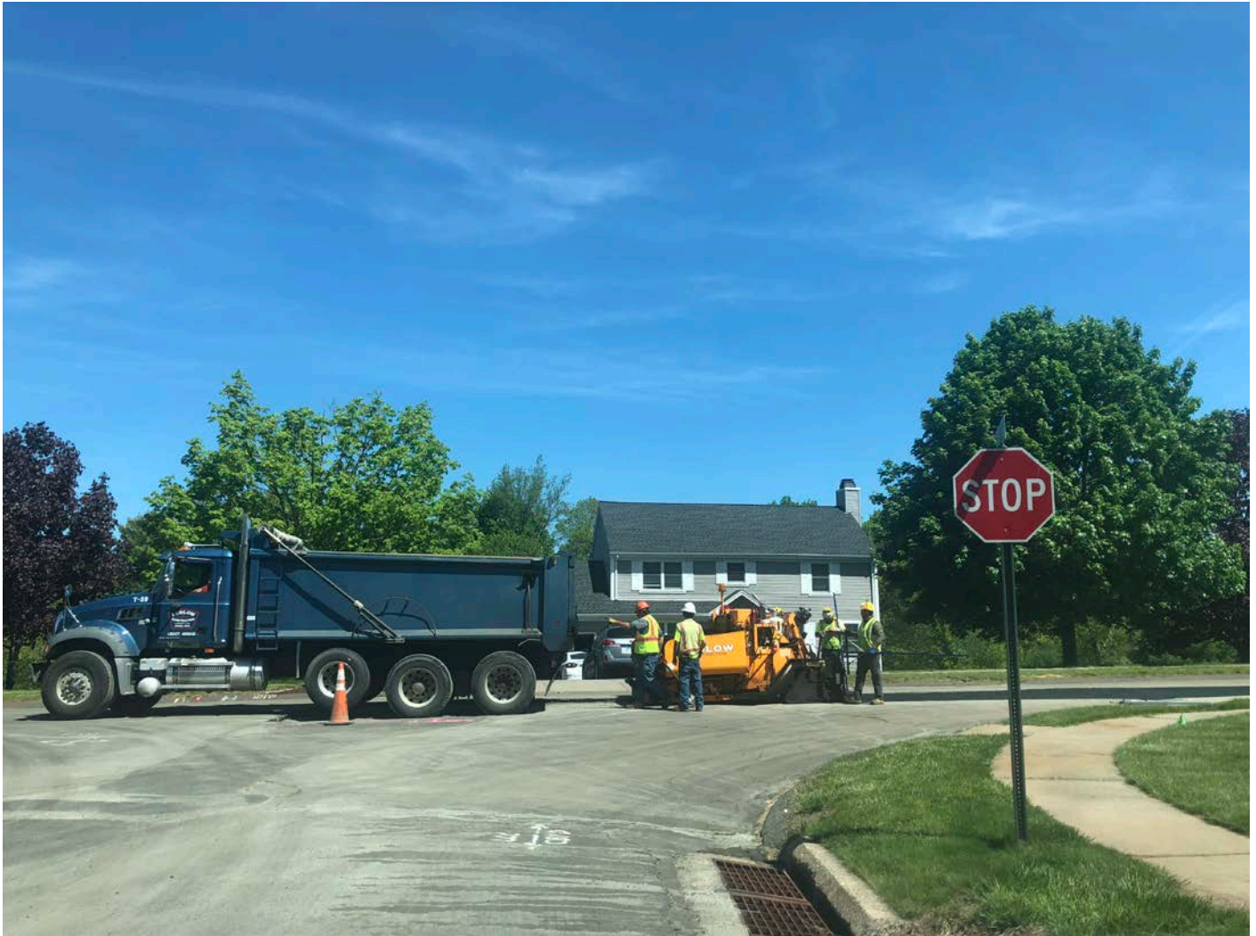
Picture 4: Ludlow placing first lift of asphalt at 12" cut back on Talcott Road intersection of Watch Hill Drive in Talcott Ridge Drive. View to the north, Middletown, CT.
