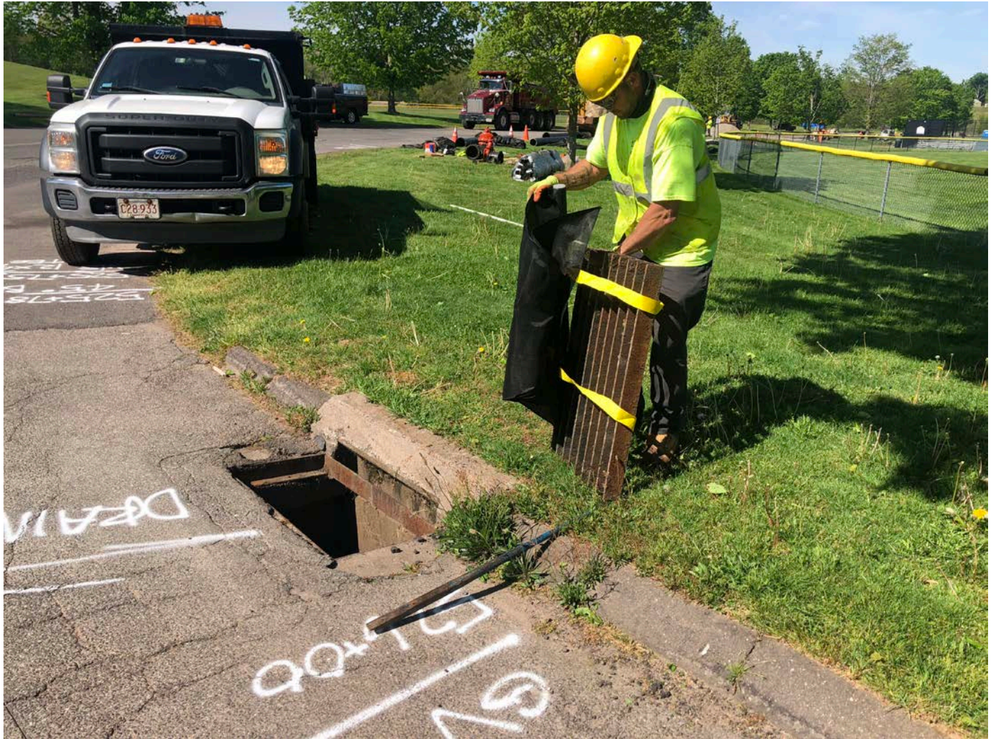
Picture 3: Ludlow placing silt sock on catch basin at Station 526+00. Pickett Lane, Durham, CT.
