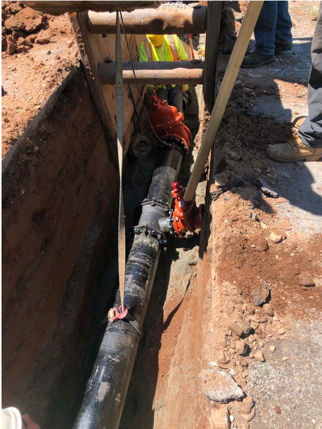
Picture 7: Ludlow placing hydrant assembly at Station 524+70. Pickett Lane, Durham, CT
