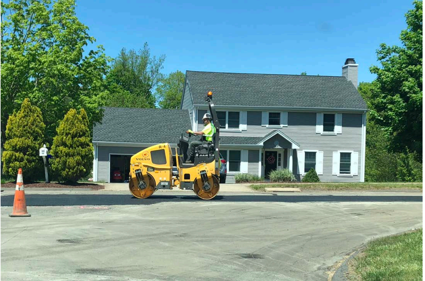
Picture 8: Ludlow rolling second lift of asphalt on 12" cut back at approximately Station 47+15. View to the north. Middletown, CT.
